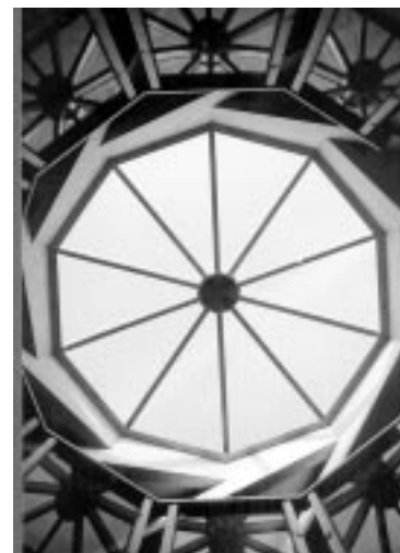
Innovative ecological design from Out of Nowhere at Darnaway. The reciprocal frame design is patented by company founder Graham Brown.
