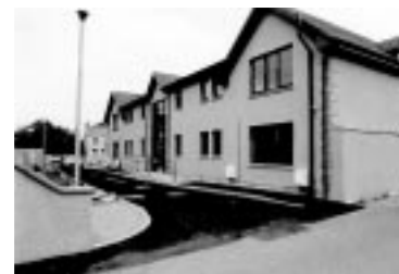
New flats in Buckie by Keith Edmonds Architect
