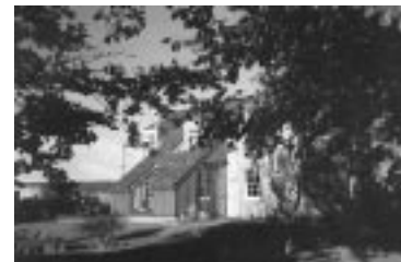
Alterations to Croy House, Pluscarden by LDN Architects, Forres.
