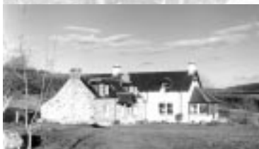
Extended traditional house at Curlusk, Mulben. LDN Architects, Forres.
