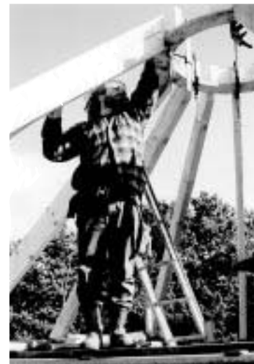
Grania Oi, Findhorn by Edge Architecture and Design. Framing of roof and central rooflight.
