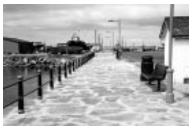
Burghead Harbour improvements
