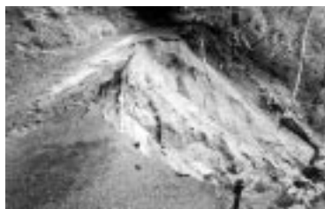
Road infrastructure damage 1997
