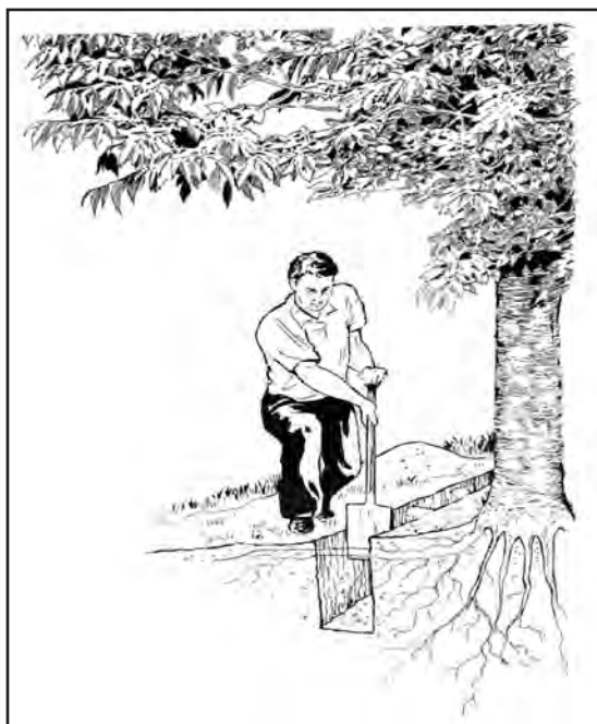
Fig 3: Disruption to roots is minimised by hand digging the routes of the utilities.
