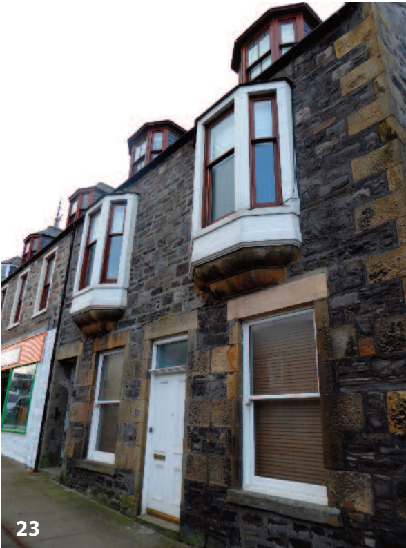
Photograph 23: An example of Oriel windows on Seafield Street that add character to the streetscape. However, the wood staining on the sash and case windows is not a traditional finish.
