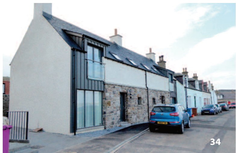
34 Photograph 34: An example of new development at the harbour front of the Seatown. The site previously contained ruined commercial properties from the Seatown’s commercial fishing past. The wall from the existing building was incorporated into the principle elevation of the new development, which maintains links to the historic past as well as adding character to the townscape. Notice how the building also reflects the building line, height and massing so that it does not disrupt views of the streetscape. A good example of how new contemporary development on a gap site can enhance the Conservation Area.
