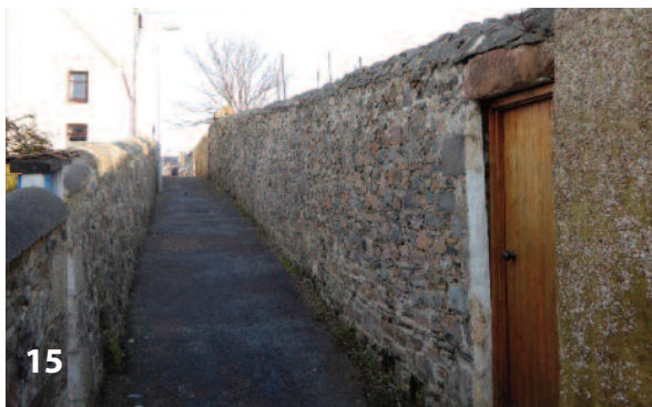
Photograph 15: A characteristic of the grid iron street pattern is straight, narrow lanes that run between larger streets. It highlights how the regular, planned street pattern creates private gardens and is the main contributing factor as to why the Planned Town has very little open space.
