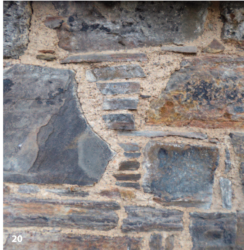
Photograph 19: An example of sneck harling that has had the render “lined out” to imitate ashlar blocks. If this finish is used it is important that the lines are horizontal.
