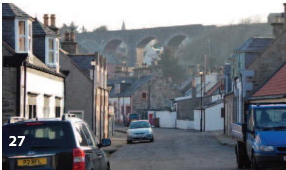
27 Photograph 27: Roof dormers in their various styles are prevalent throughout the Conservation Area and streetscape.
