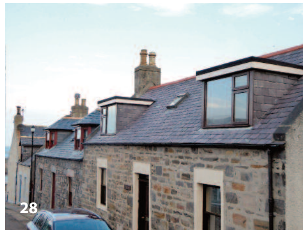
28 Photograph 28: Inappropriate flat roofed box dormers in the Conservation Area disturb the continuity and rhythm of the roofscape. Modern window designs also detract from the traditional character of the Conservation Area.
