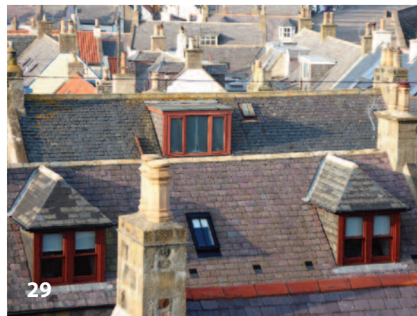
29 Photograph 29: Due to the prominent visibility of the Seatown's roofscape, inappropriate box dormers can be seen from several key vantage points.
