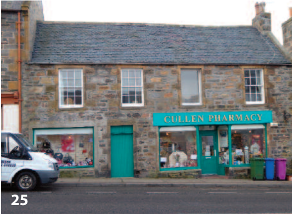
Photograph 25: An example of how the removal of a traditional window can have a negative effect on the appearance and visual balance of a building. It also highlights the important role that astragals have to the visual character of a building.
