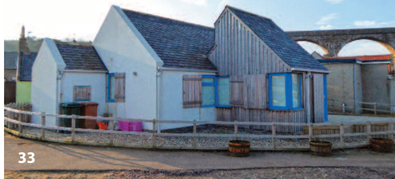
33 Photograph 33: An example of new development in the Seatown. An example of how new development can be contemporary but still respect the traditional appearance of the Conservation Area. The massing and height is respectful of the surrounding townscape and the use of traditional materials reflects the traditional character of Cullen. The use of colour around the windows is a characteristic that was identified as enhancing the appearance of the Conservation Area.
