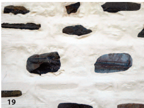
Photograph 19: An example of sneck harling that has had the render “lined out” to imitate ashlar blocks. If this finish is used it is important that the lines are horizontal.
