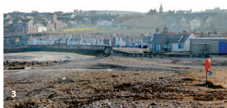
Photograph 3: View from the West looking towards the Conservation Area. The low lying Seatown is in the foreground while the Planned Town is situated on higher ground behind the viaduct. The viaduct, the church steeple, and cottages with their gables fronting the sea are all visible and are integral characteristics to the character and townscape of the Conservation Area.
