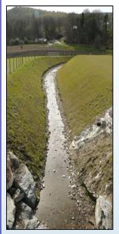
A network of ditches will be constructed to convey surface water runoff from the fields to the north of Back Street, away from the village into the Burn of Kinminitie. Access to these fields will be accommodated where possible during the works. Traffic management will be in place while work is undertaken in this area. However, access to properties on Back Street, Sand Lane and Kinminitie Farm will be maintained throughout the construction period.
