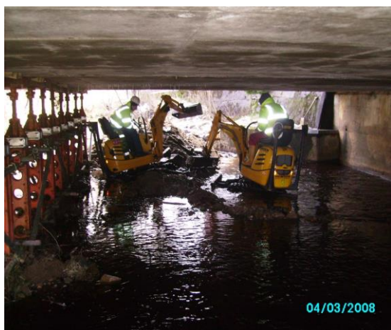
Burn of Rothes – Sediment Removal
