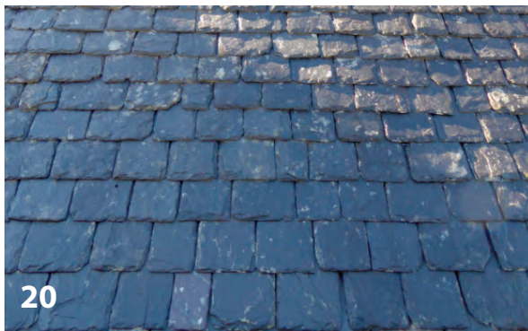
Photograph 21: An example of more uniform and smoother Welsh slate
