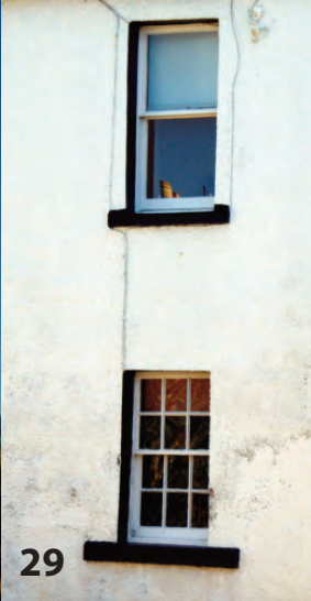
Photograph 29: The visual balance and character of a building can be negatively affected where different astragal patterns are used
