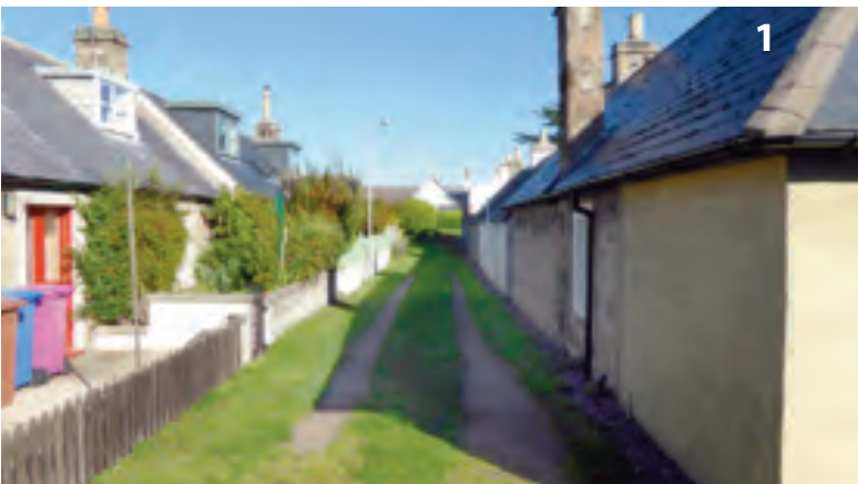
Photograph 1: Rows of single storey terraces have remained a feature of the townscape for over 100 years. Notice the small plot size and how the row of South facing properties have claimed part of the lane as garden ground to take advantage of the sun.
