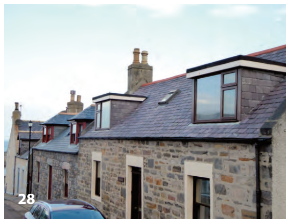
Photograph 28: Inappropriate flat roofed box dormers in the Conservation Area disturb the continuity and rhythm of the roofscape. Modern window designs also detract from the traditional character of the Conservation Area.
