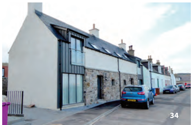
Photograph 34: An example of new development at the harbour front of the Seatown. The site previously contained ruined commercial properties from the Seatown’s commercial fishing past. The wall from the existing building was incorporated into the principle elevation of the new development, which maintains links to the historic past as well as adding character to the townscape. Notice how the building also reflects the building line, height and massing so that it does not disrupt views of the streetscape. A good example of how new contemporary development on a gap site can enhance the Conservation Area.
