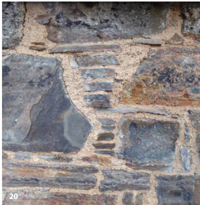
Photograph 19: An example of sneck harling that has had the render “lined out” to imitate ashlar blocks. If this finish is used it is important that the lines are horizontal.
