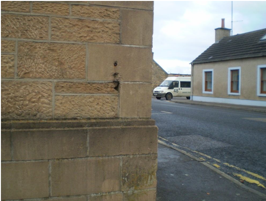
Available visibility to north of access at 2.4 metres, from the edge of the carriageway.
