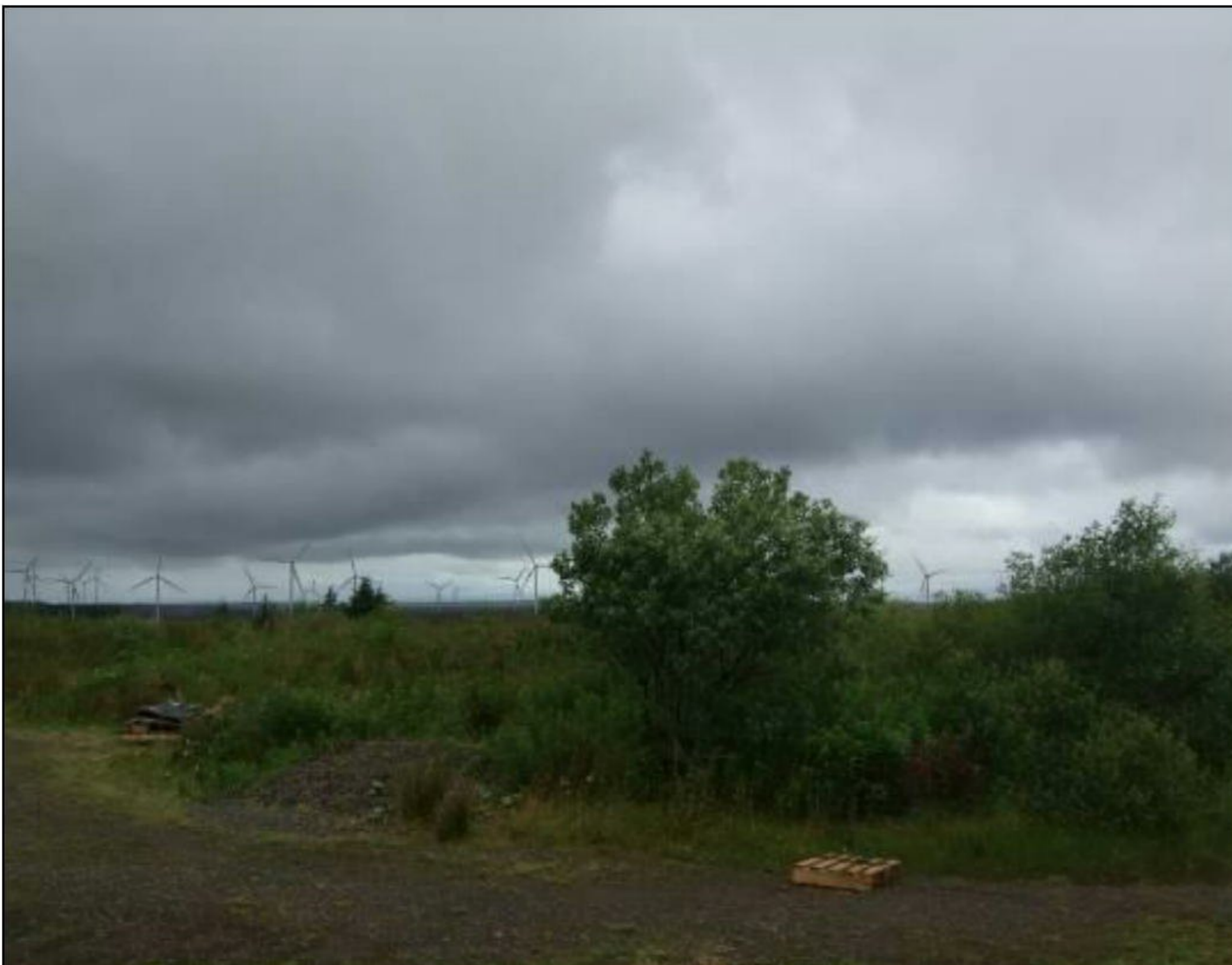
Viewing WNW from the Wind Turbine under test on Test Pad No. A6.
