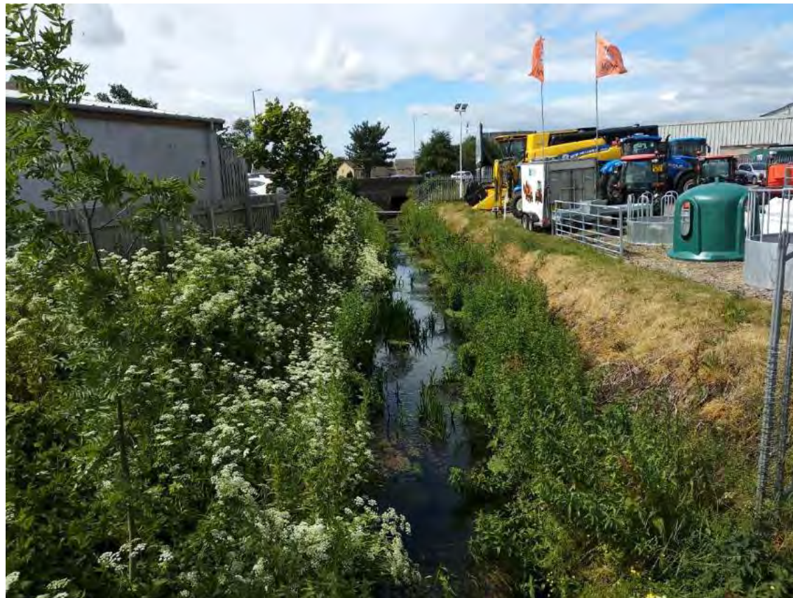
Photography 36. Section XS33, Moycroft road culvert, view from the bridge to upstream.
