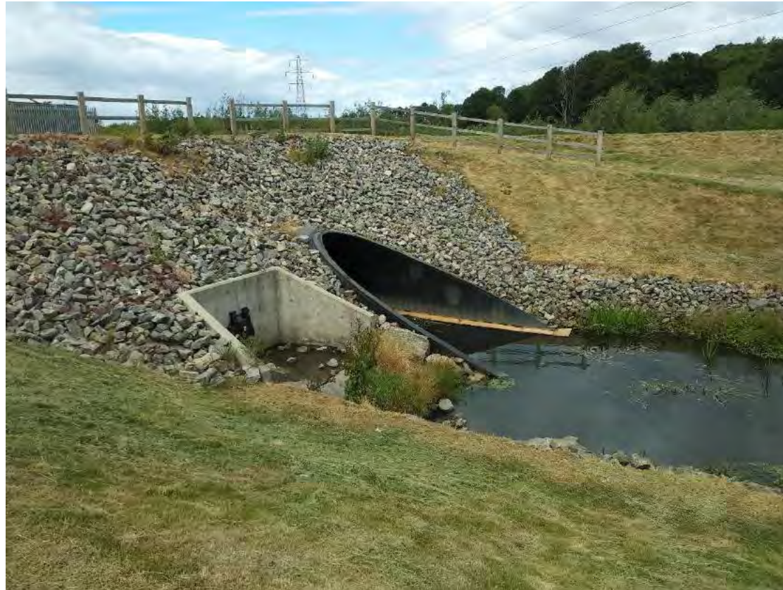
Photography 38. Section XS35 culvert outlet.
