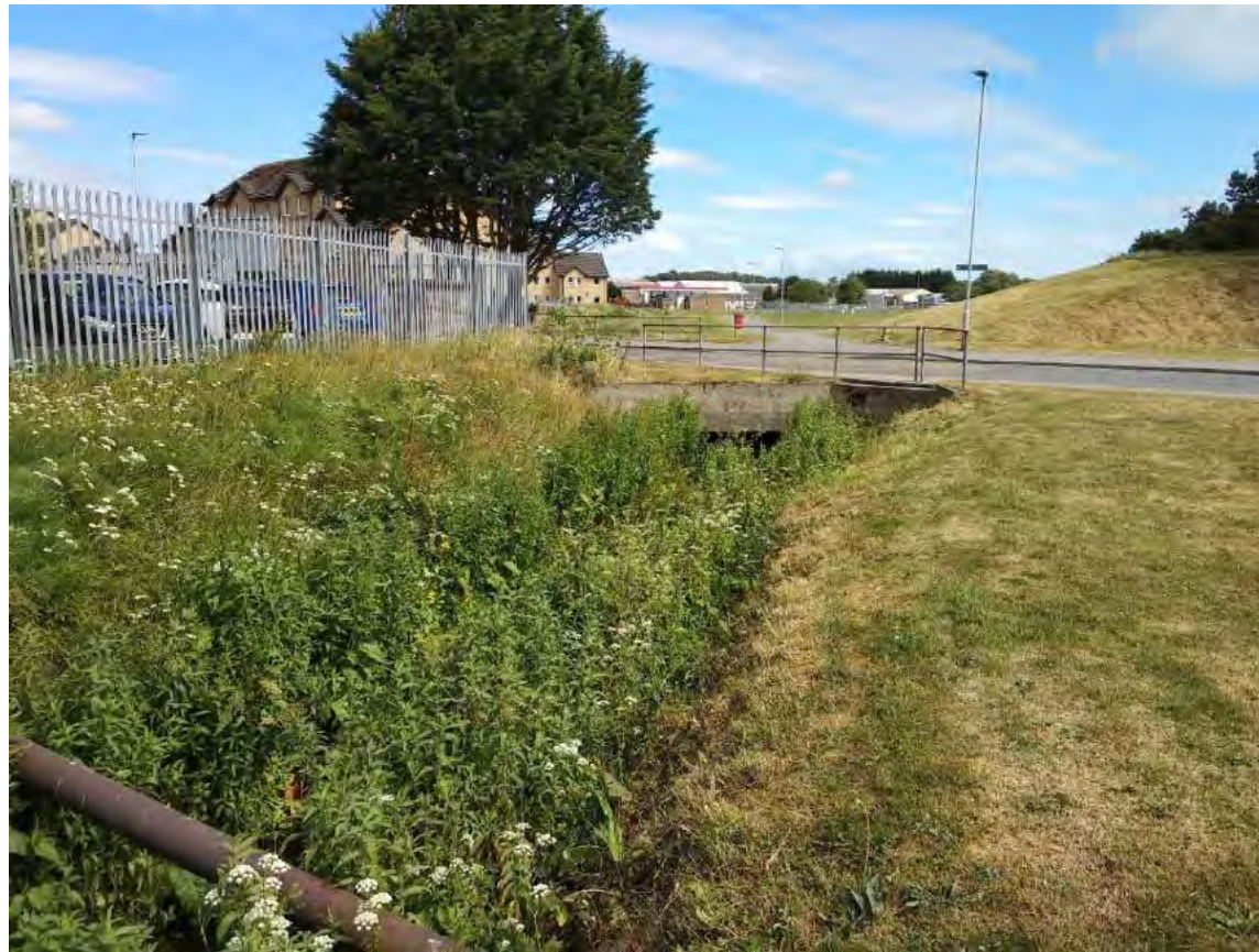
Photography 30. Section XS29 upstream, Ashgrove Road culvert inlet.
