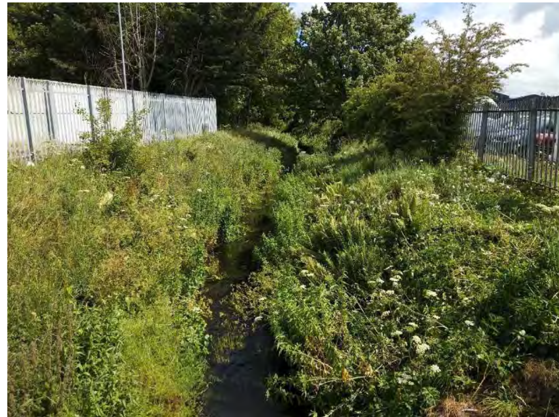
Photography 37. Section XS34, Moycroft road culvert, view from the bridge to downstream.
