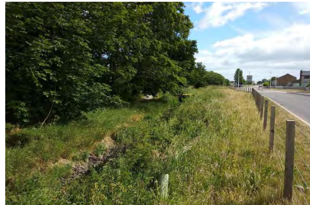
Photography 4. Section between XS5 and Bridge XS6, view from west to east.
