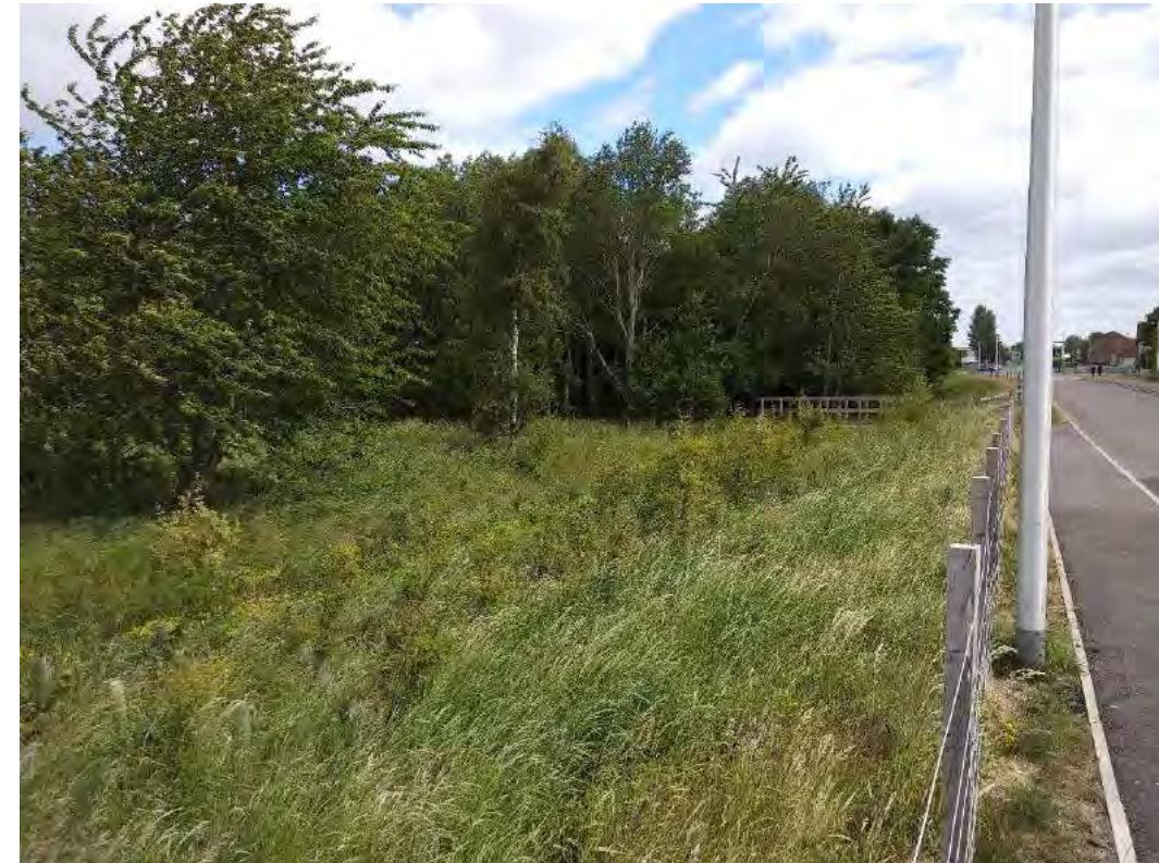
Photography 2. Bridge at Section XS4, view from west to east.
