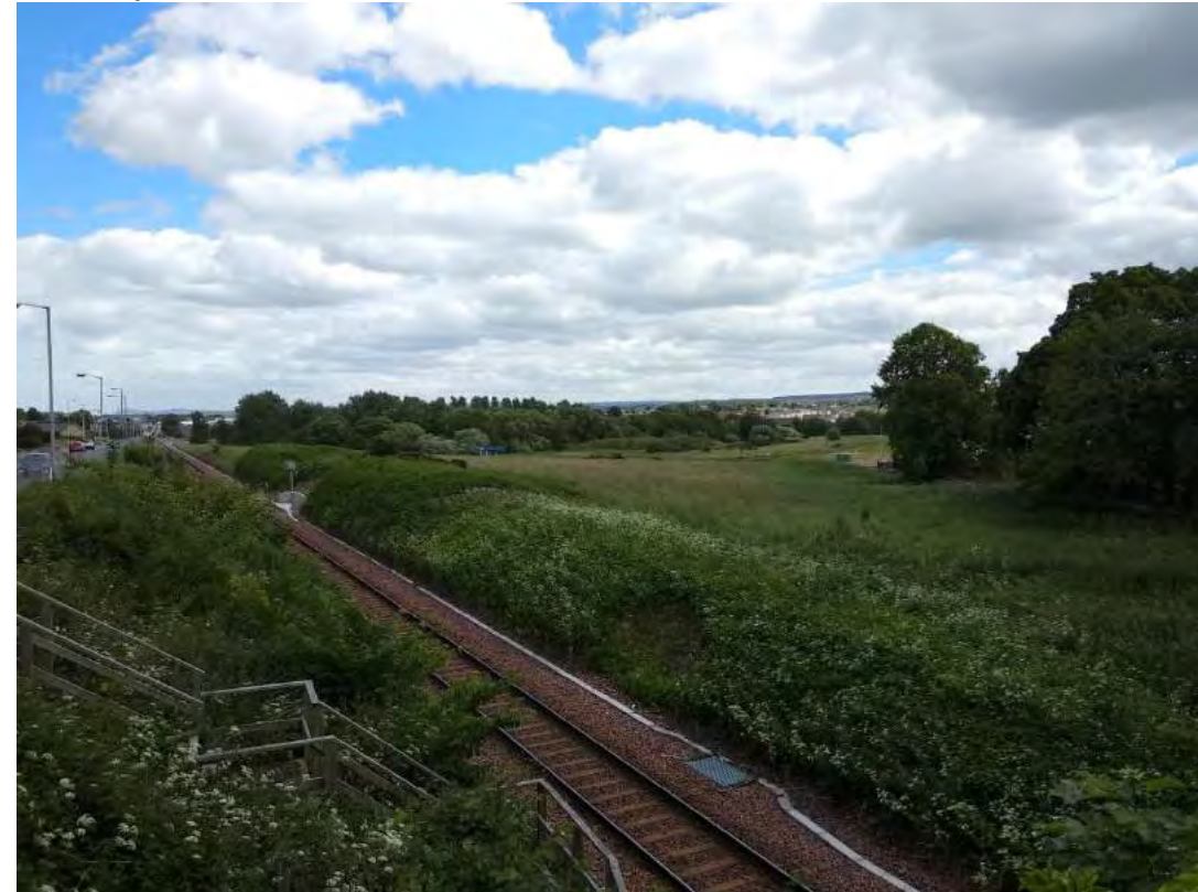
Photography 45. View from west to east at the Mayne Road bridge showing levels raising, south to north, at the proximity of the railway tracks and the low area at the east site boundary.
