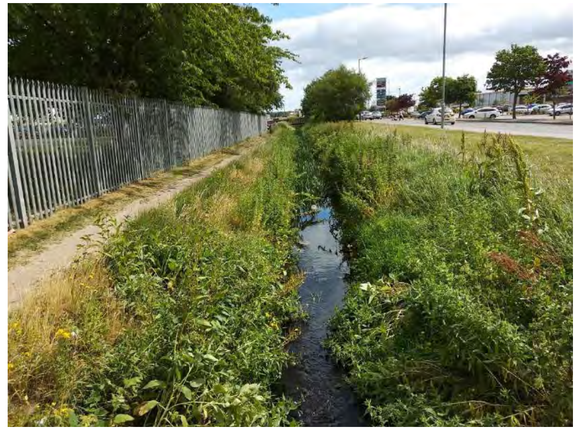
Photography 25. Section XS22 bridge downstream.
