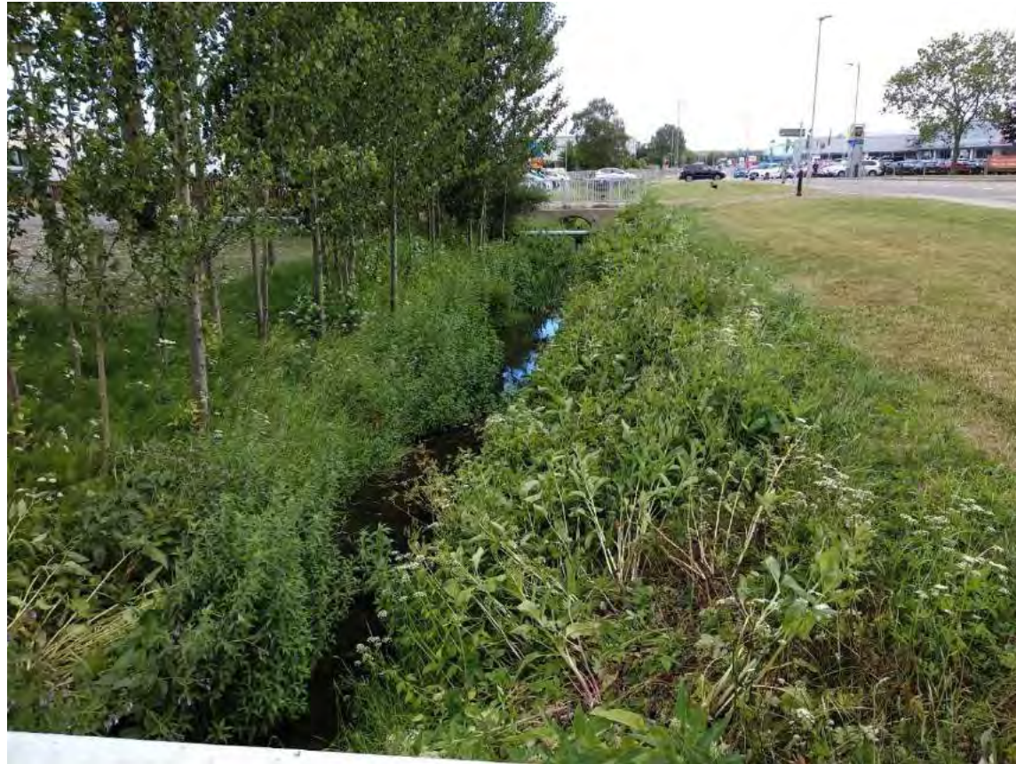
Photography 7. Section XS9 culver outlet showing culvert at Section XS10.
