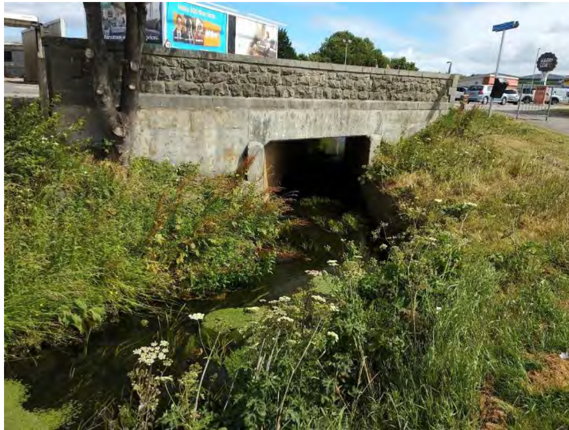
Photography 34. Section XS31, East road bridge upstream.
