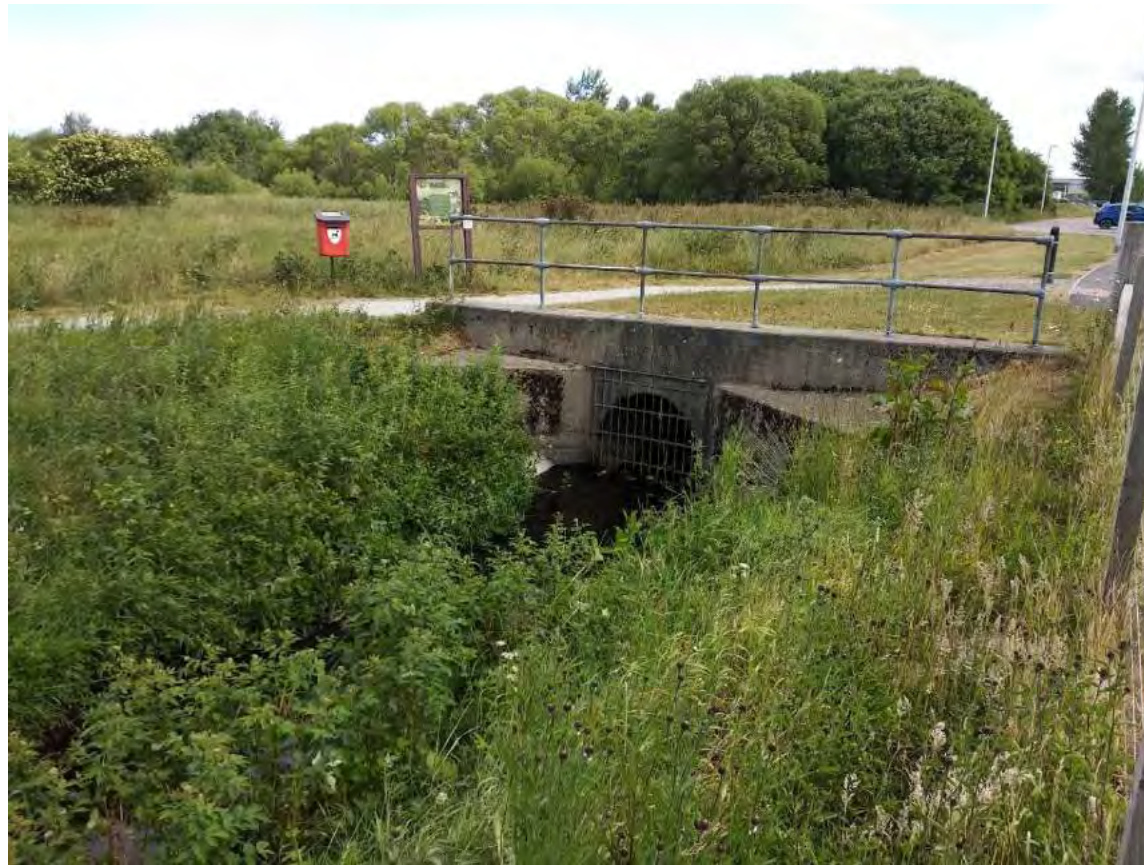
Photography 5. Section XS8 culvert inlet.
