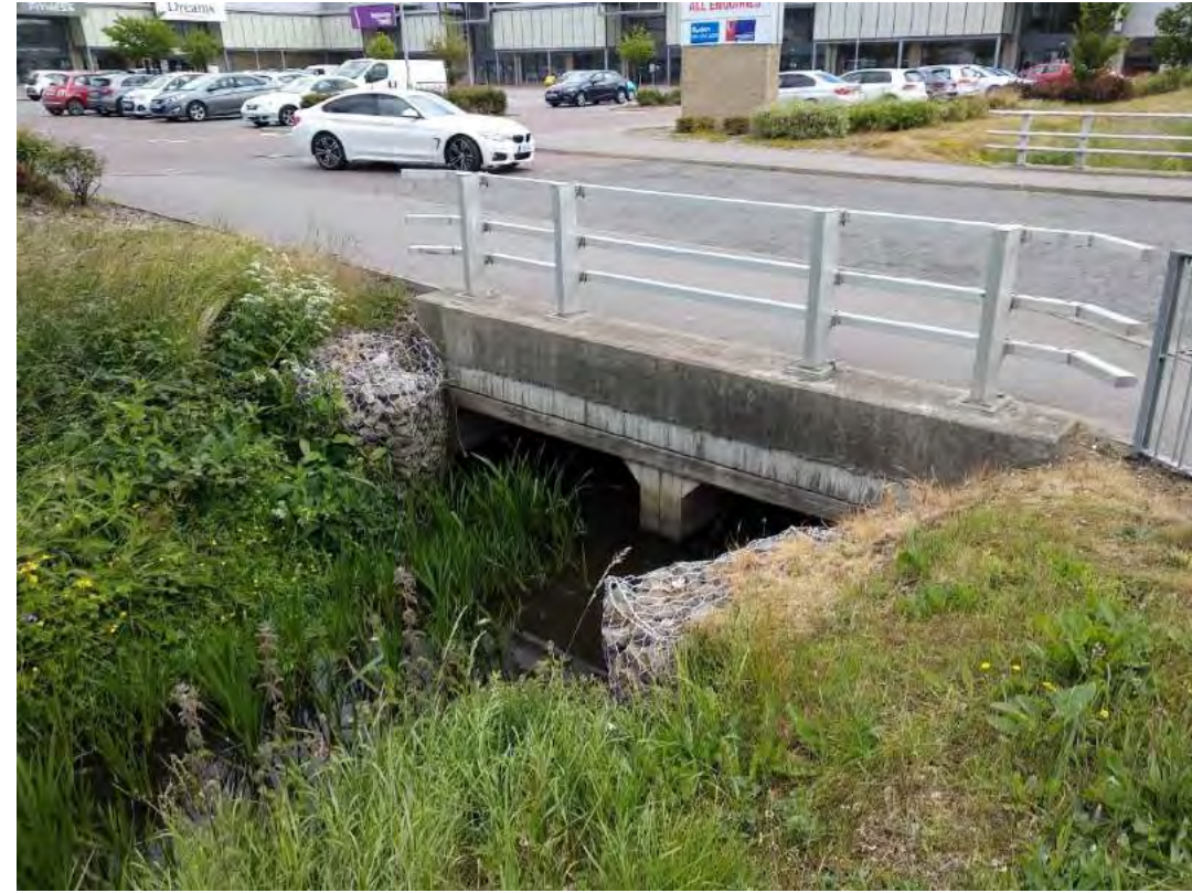
Photography 14. Section XS15 dual culvert inlet.
