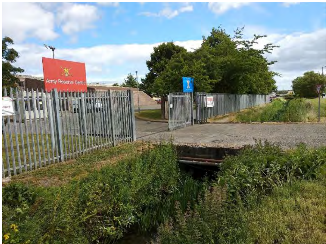
Photography 24. Section XS22 bridge upstream.
