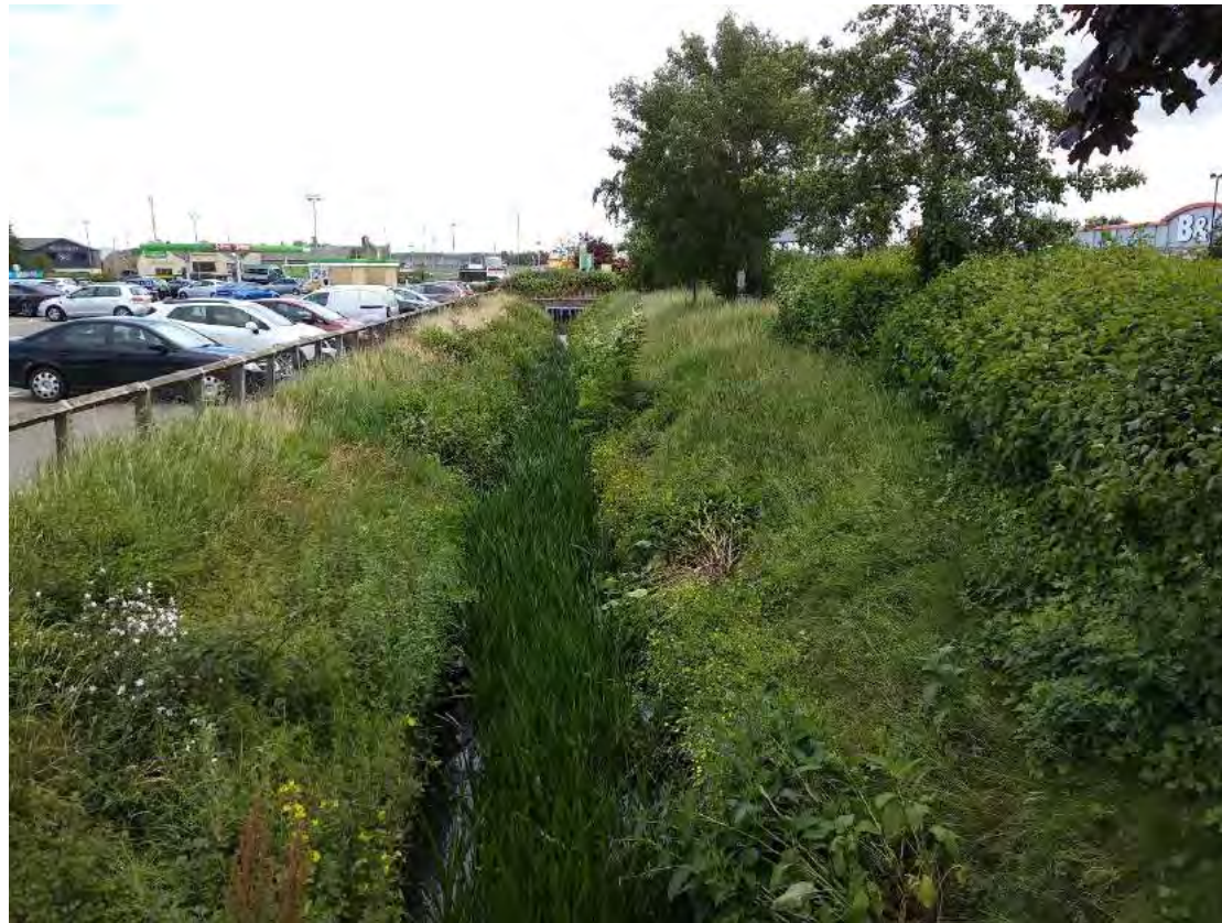
Photography 26. Section XS24 bridge downstream, showing the XS25 culvert inlet.
