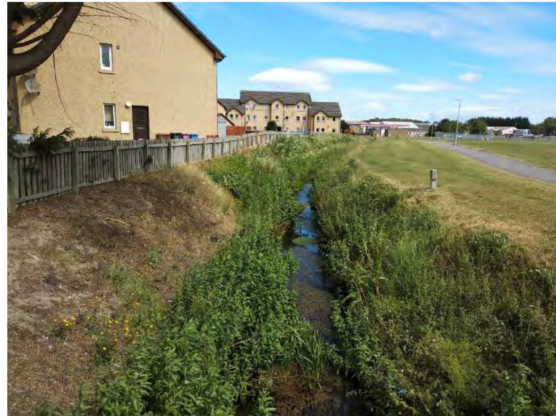
Photography 31. Section XS30 downstream, Ashgrove Road culvert outlet.
