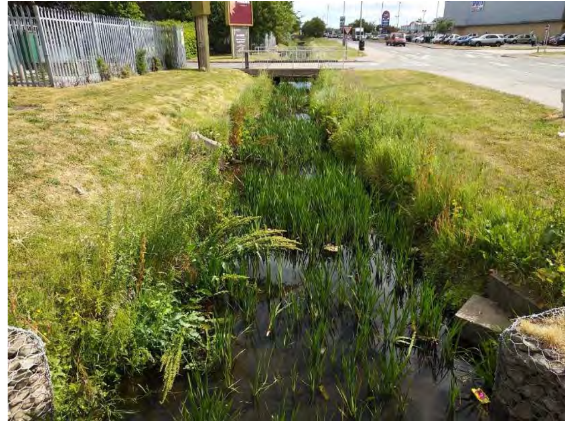
Photography 19. Section XS19 downstream, culvert outlet.
