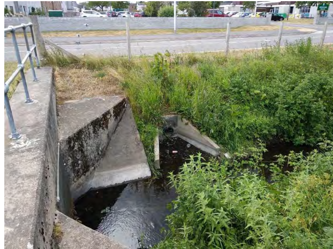
Photography 6. Section XS8 culvert inlet and surface water point of discharge.
