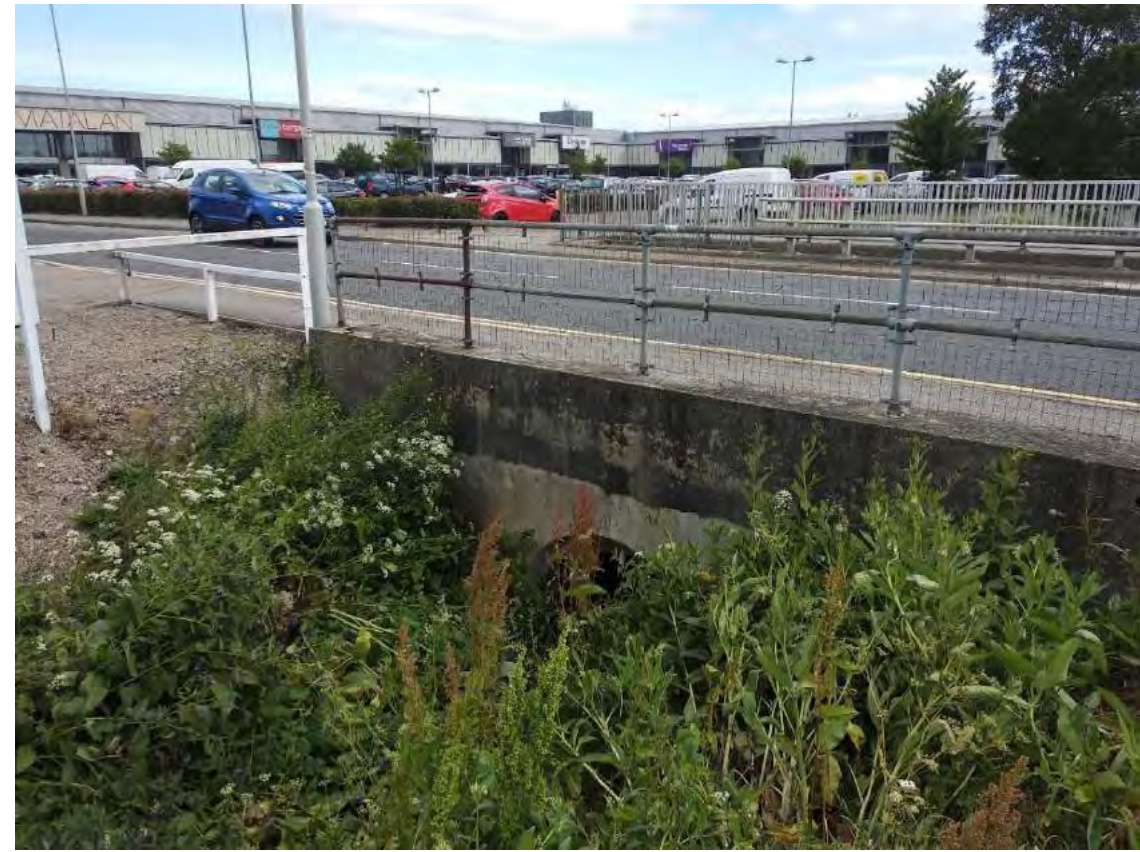
Photography 10. Section XS12 culvert inlet.
