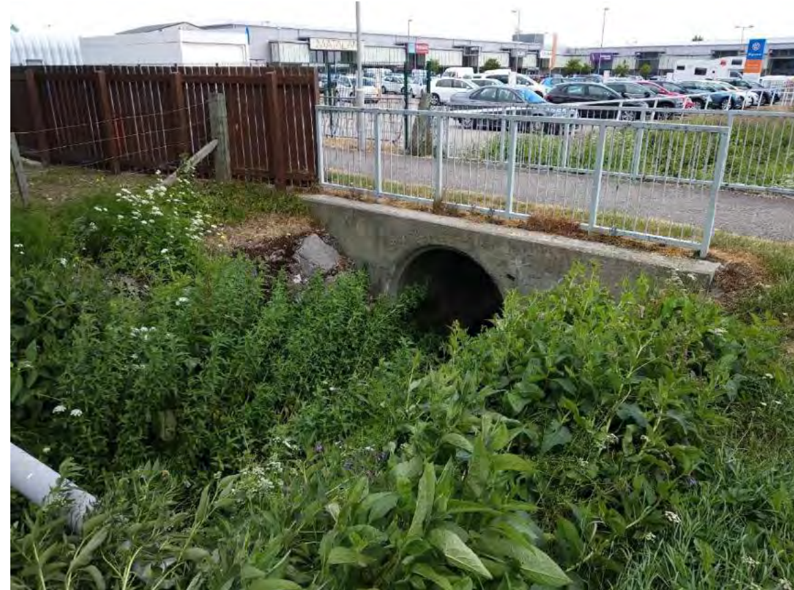
Photography 8. Culver inlet at Section XS10.
