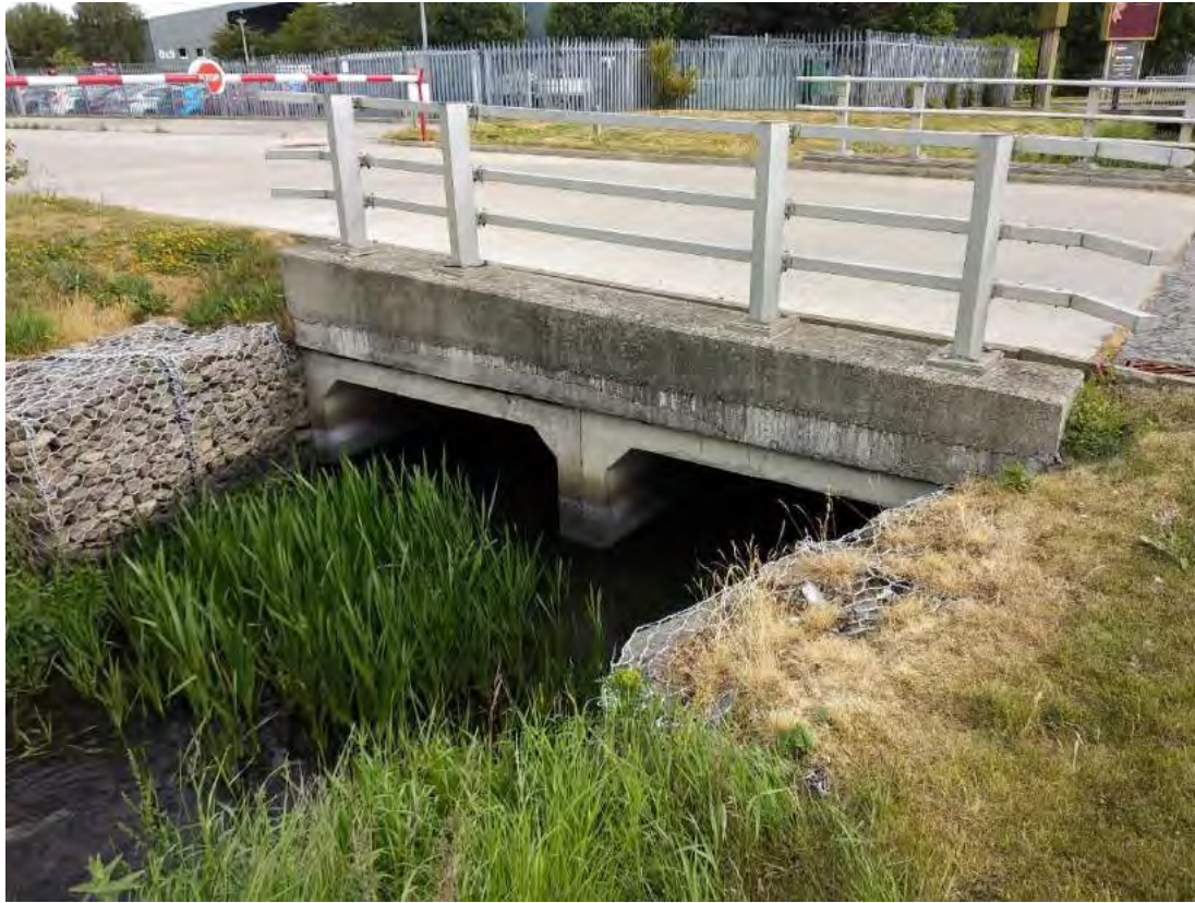
Photography 18. Section XS18 dual culvert inlet.
