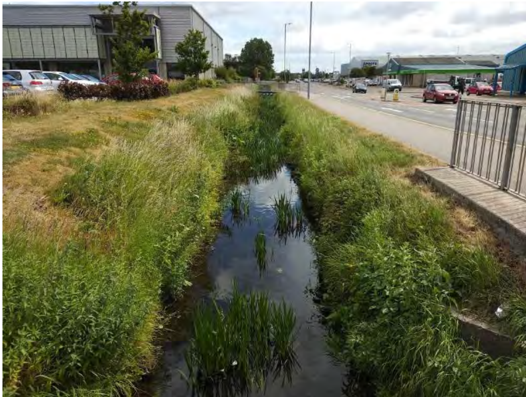
Photography 16. Section XS16 downstream, culvert outlet.
