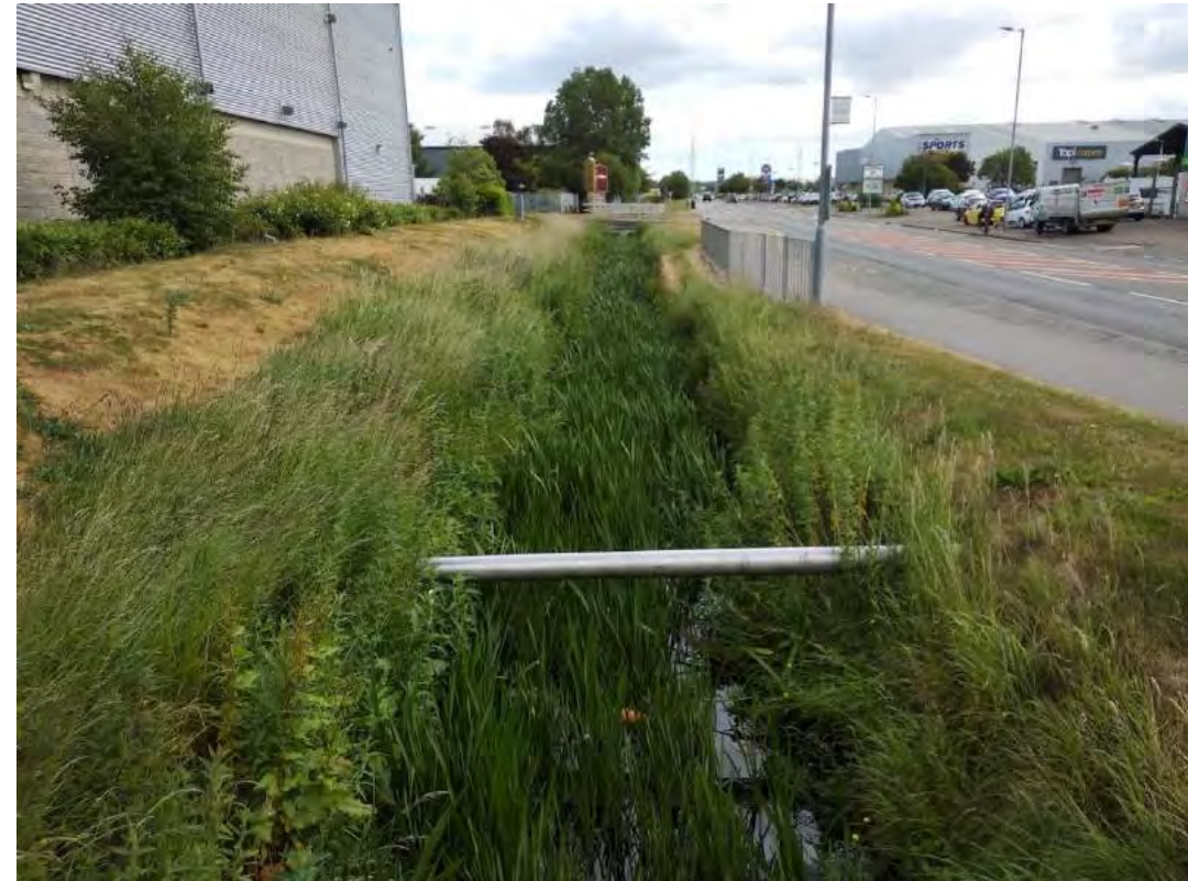
Photography 17. Section XS17 bridge downstream.
