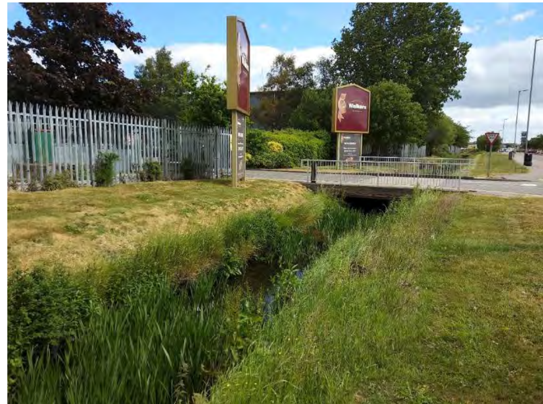
Photography 21. Section XS20 bridge upstream.
