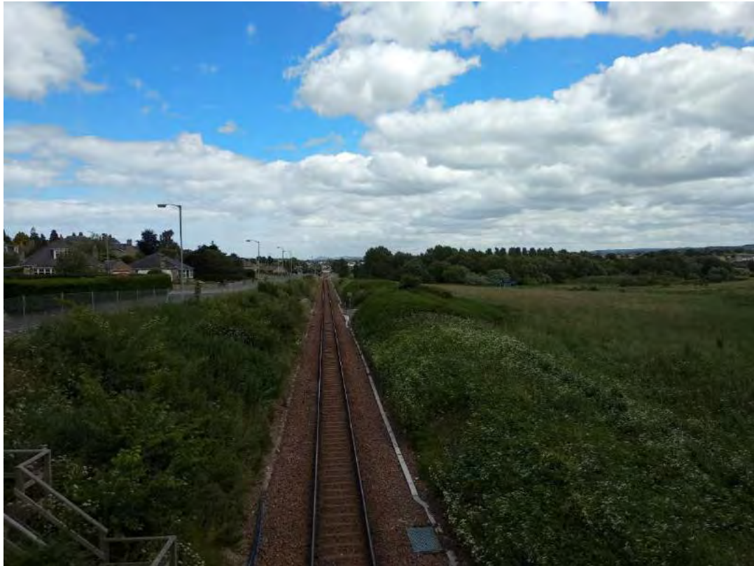
Photography 44. View from west to east at the Mayne Road bridge showing levels raising, south to north, at the proximity of the railway tracks and the low area at the east site boundary.
