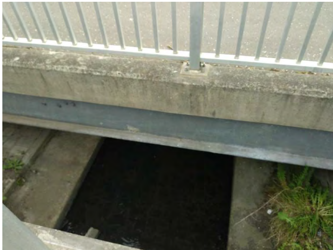
Photography 11. Section XS12 culvert outlet and Section XS13 bridge upstream.
