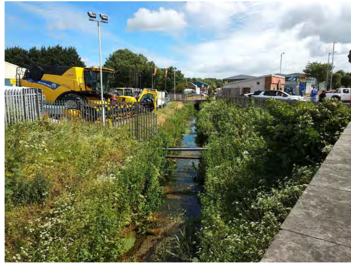
Photography 35. Section XS32, East road bridge downstream.
