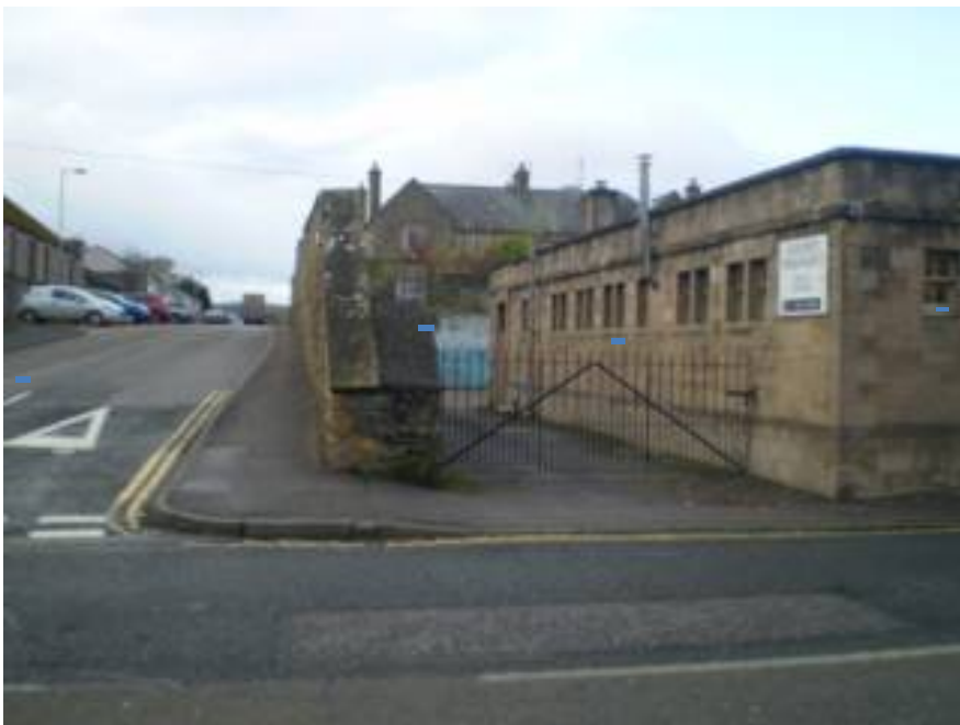
Access to parking area at rear of 'Golden Pheasant'
