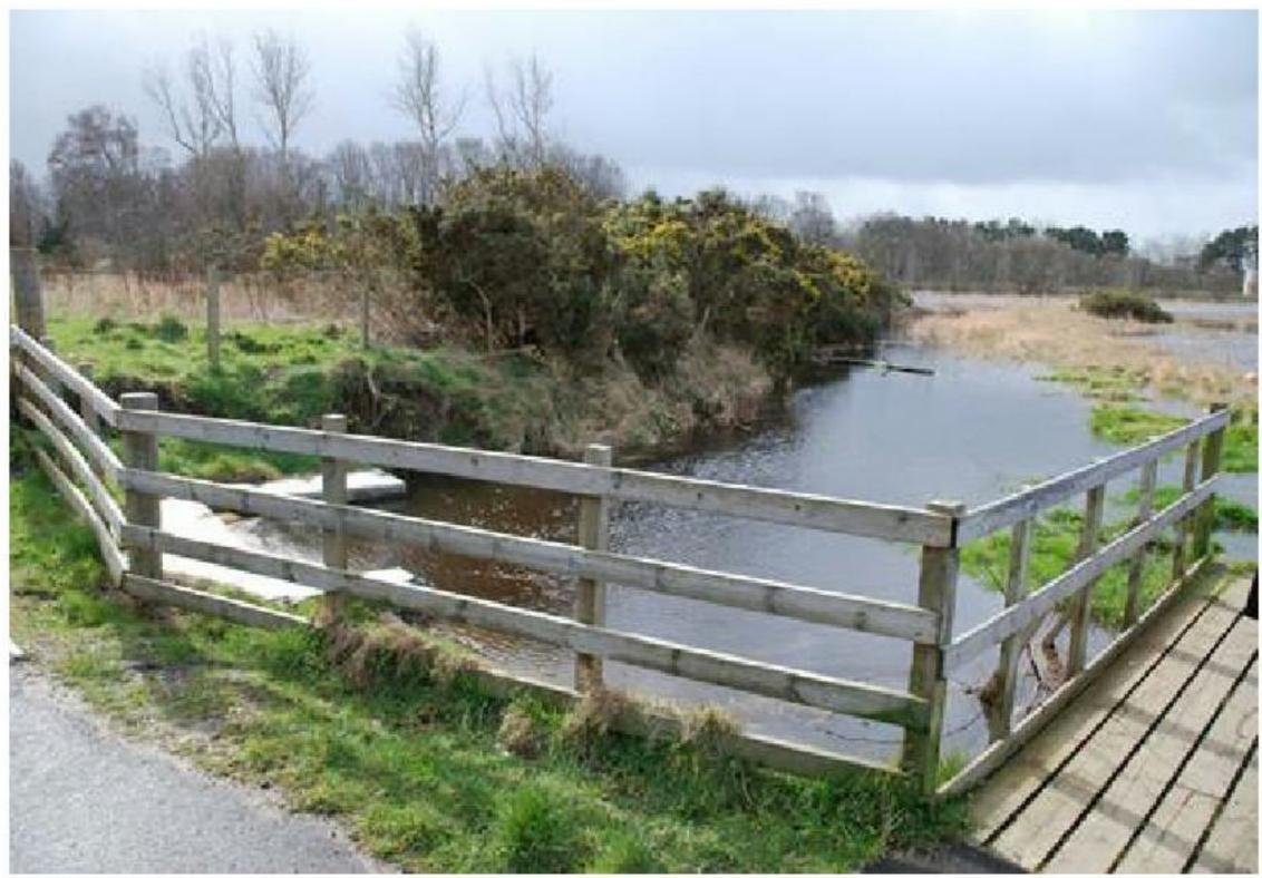
Figure 1 - Airfield Drainage Ditch (bank has recently eroded to expose the sandy soil of R2) [copyright MJT]
