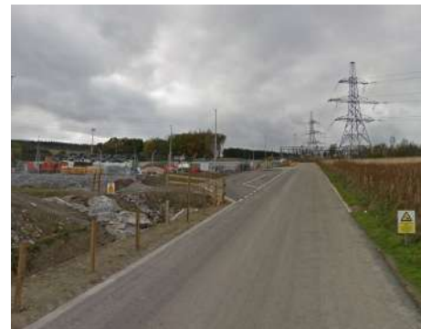
3f - view to Blackhillock Substation*
