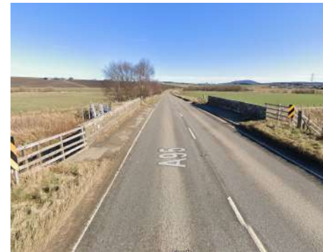
2c - bridge over railway line
