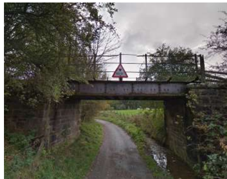
3e - railway overbridge*
