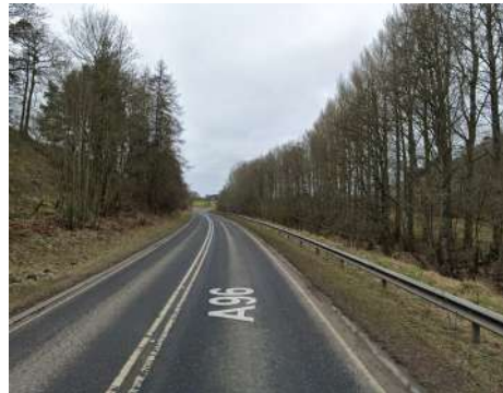
1a - single carriageway, safety barriers
