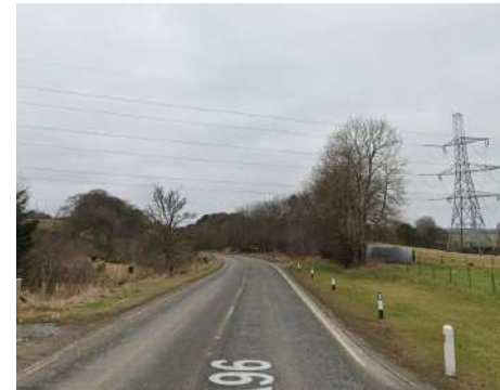
1c - overhead transmission lines
