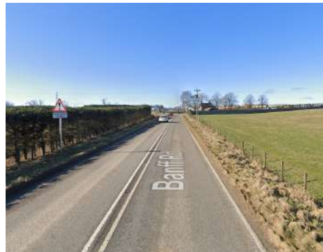
2a - single carriageway into Keith
