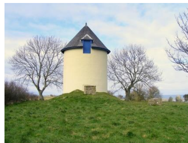
Community Asset Transfer (CAT) for Garmouth Water Tower
