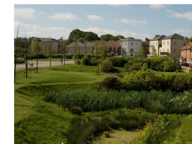
Swales and drainage, open space
