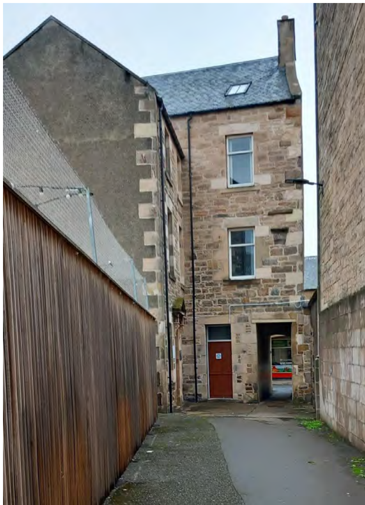
REAR VIEW OF 30-32 HIGH STREET
