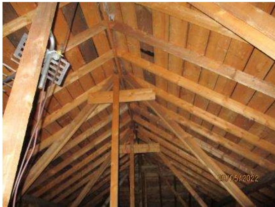
1. Roof structure – Teaching north
