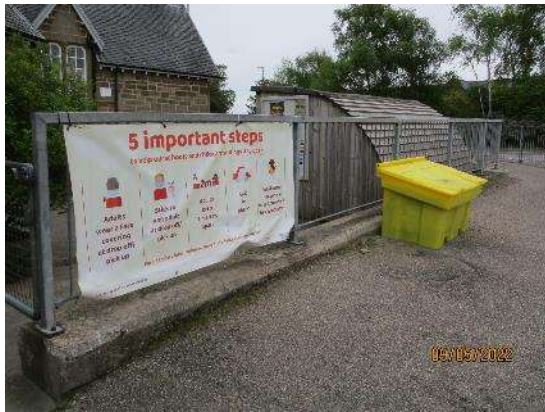
206. Galvanised rail fencing
