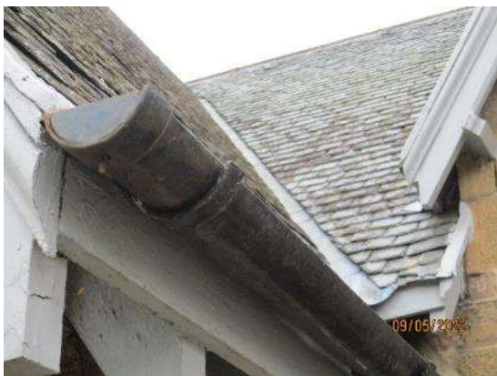
29. Half round cast iron gutters
