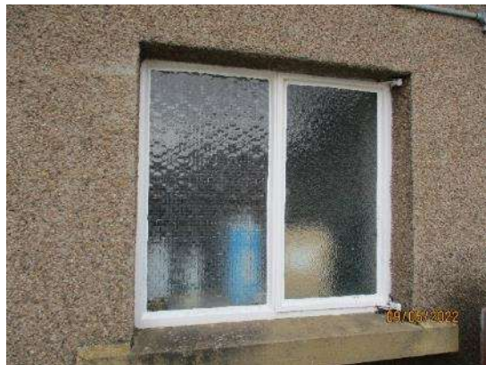
64. Crittall window to Plant Room
