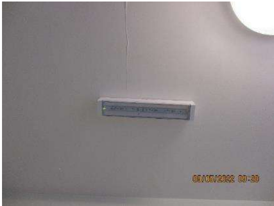
160. Emergency light fitting teaching block class.
