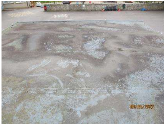
19. GRP roof above boiler room
