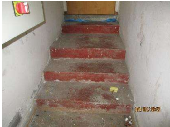
93. Concrete steps to Plant Room
