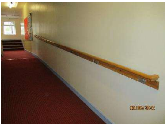
94. Timber handrails to ramps
