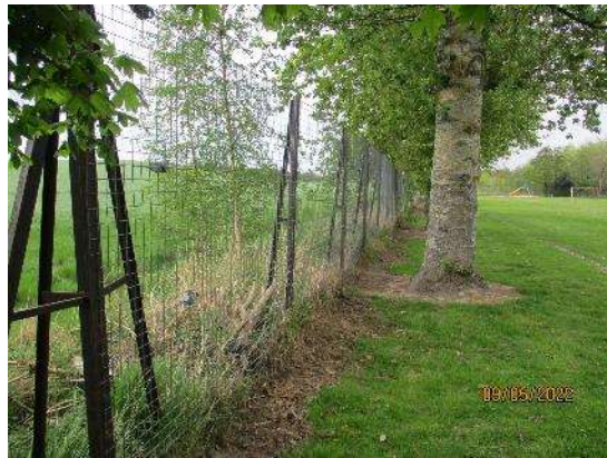
207. Chain link fencing
