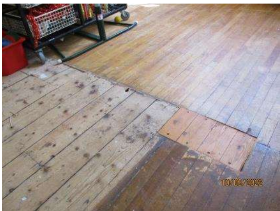
88. Patch repaired timber boards
