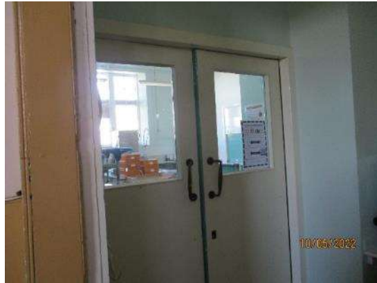
114. Internal double doors
