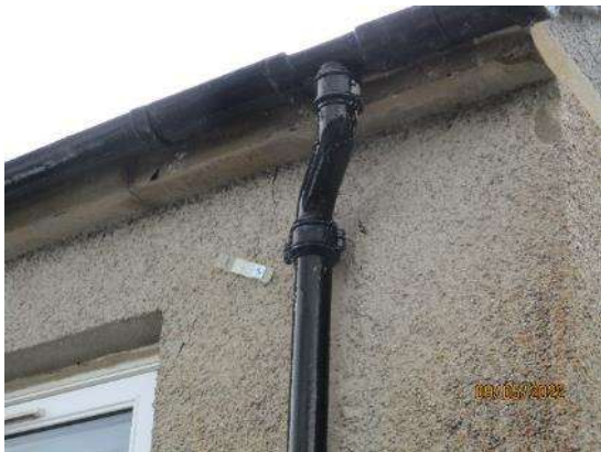
33. Cast iron downpipes
