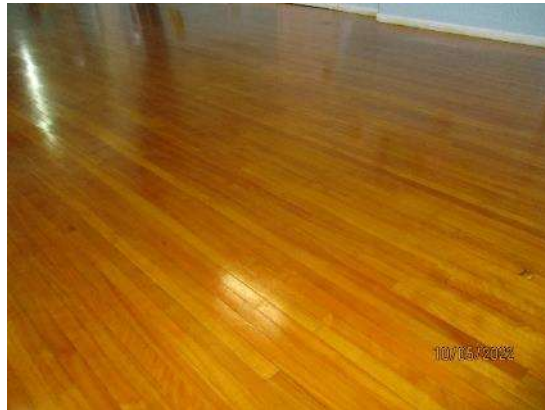
87. Varnished floor boards
