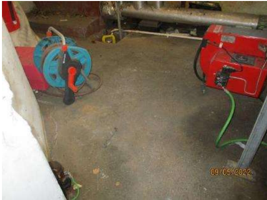
90. Concrete floors to Boiler & Plant rooms
