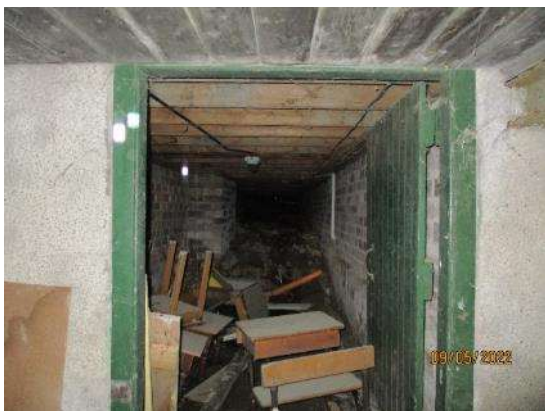
82. Below timber suspended floor – Teaching south
