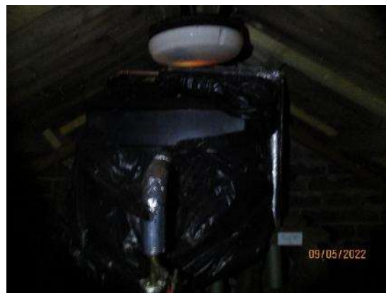
139. Heating feed and expansion tank. Teaching block attic.
