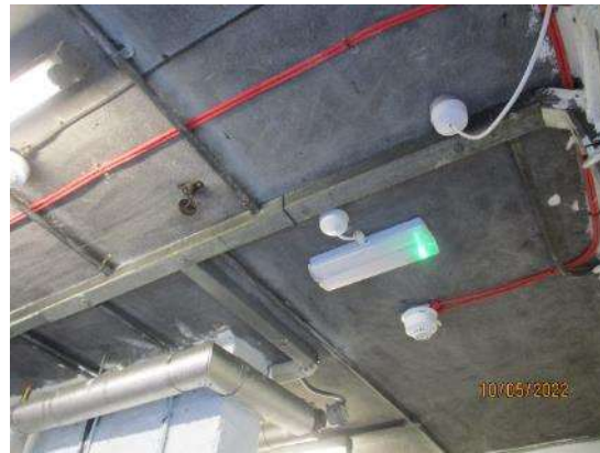
8. Boiler room – concrete flat roof structure
