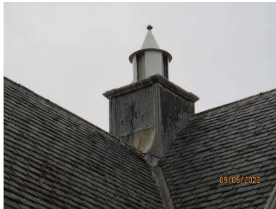
38. Roof vents to Dining block
