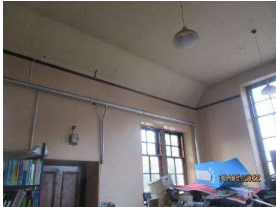
199. Pipework and lighting – external store building. (Assumed disconnected supplies)
