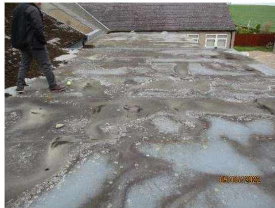
16. GRP roof above pupil toilets
