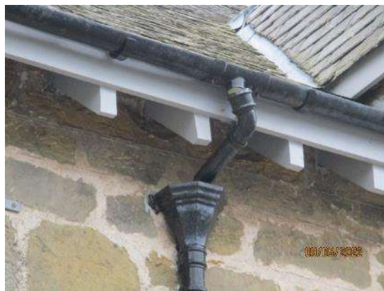
30. Downpipe to hopper heads
