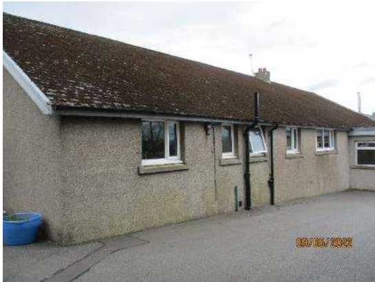
43. Masonry walls – Teaching south
