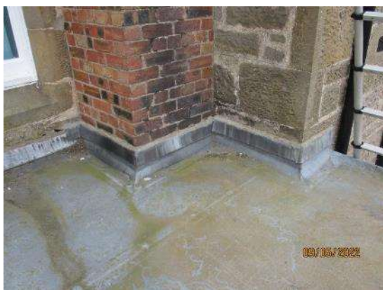
36. Brick chimney to boiler room
