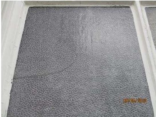
67. Cracked glazing
