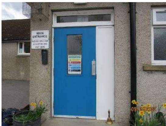
54. Main entrance door – Teaching block
