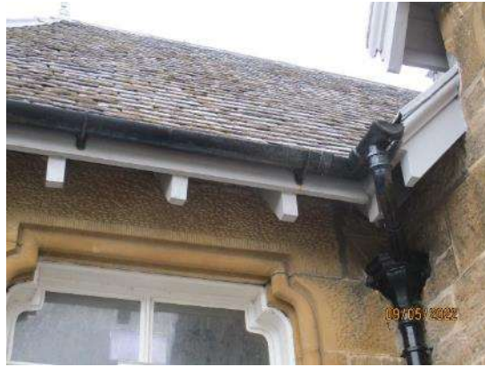
26. Rafter feet and fascia board
