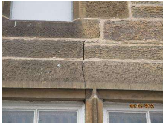
46. Isolated cracking
