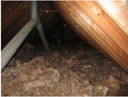
25. Mineral fibre to Dining block
