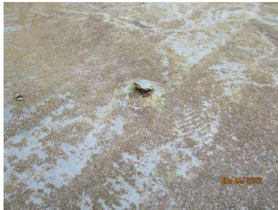
20. Fixings punching through GRP surface
