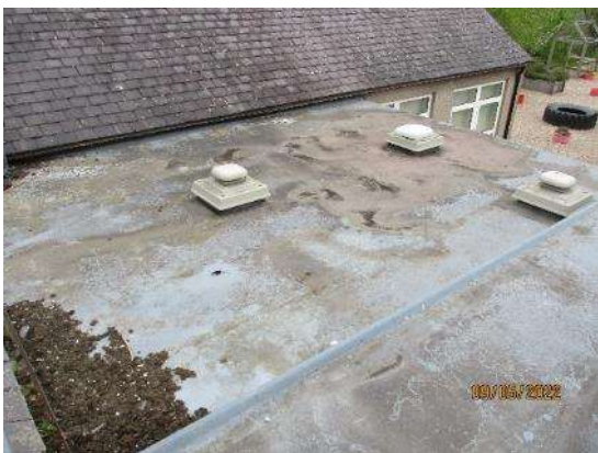
17. GRP roof above staff toilet
