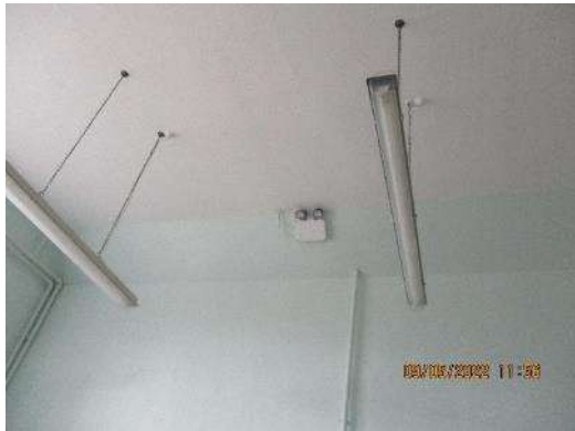
192. Lighting – dining block kitchen.
