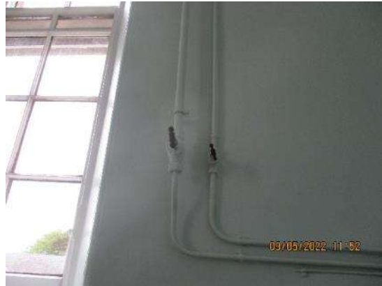
181. Hot water copper pipework – dining block example.
