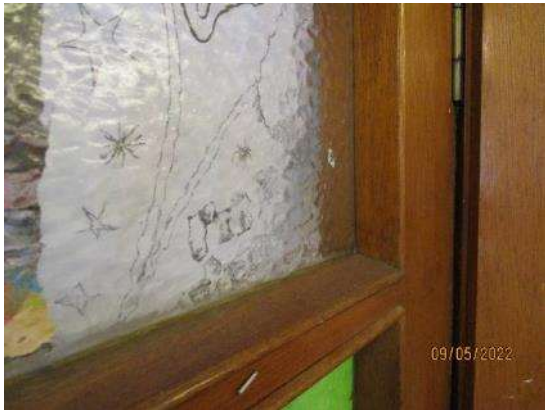
115. Single glazing to doors
