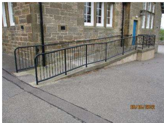
77. Ramps and guard rails
