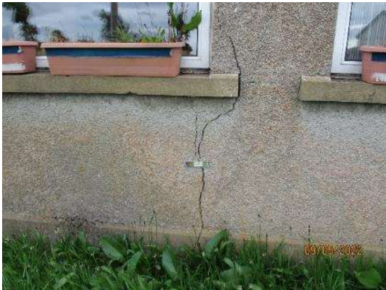
39. Masonry walls – Teaching north
