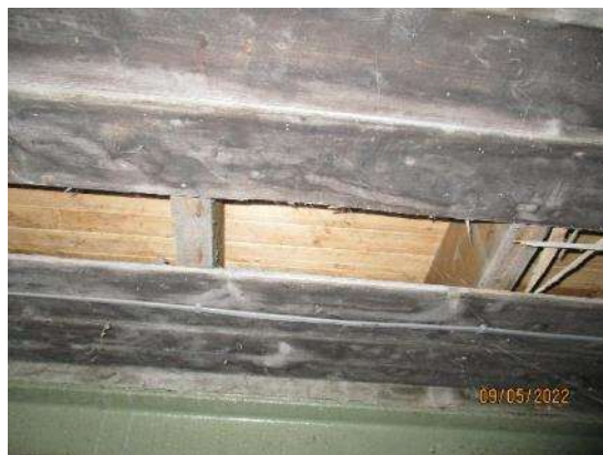
83. Timber suspended floor
