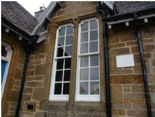
61. Timber sliding sash windows
