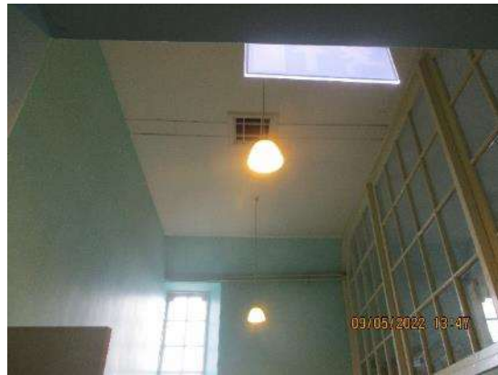
193. Lighting – dining block classroom.
