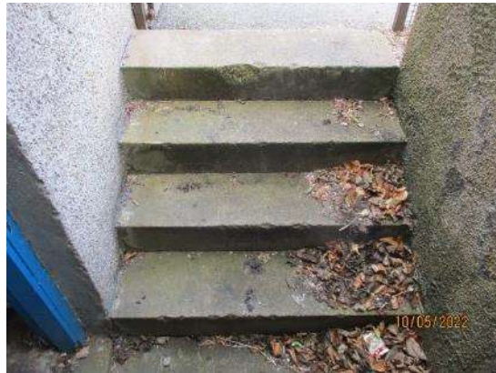
75. Concrete steps to Boiler House
