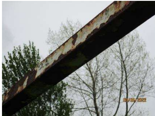
232. Surface corrosion
