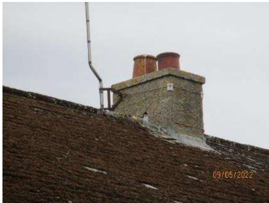
37. Brick/roughcast chimney to Teaching block
