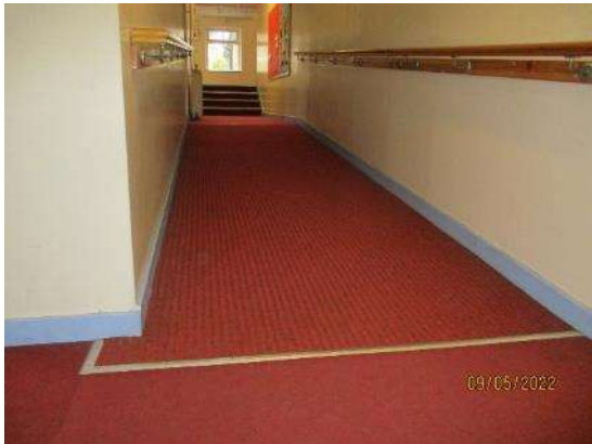
92. Ramps to Teaching corridor
