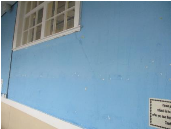
70. Lath & plaster walls
