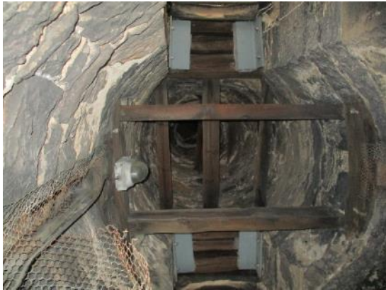
7. Timber structure within the steeple
