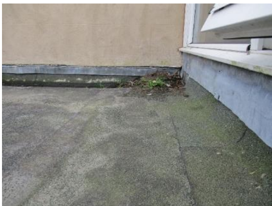
23. Felt roof box gutters
