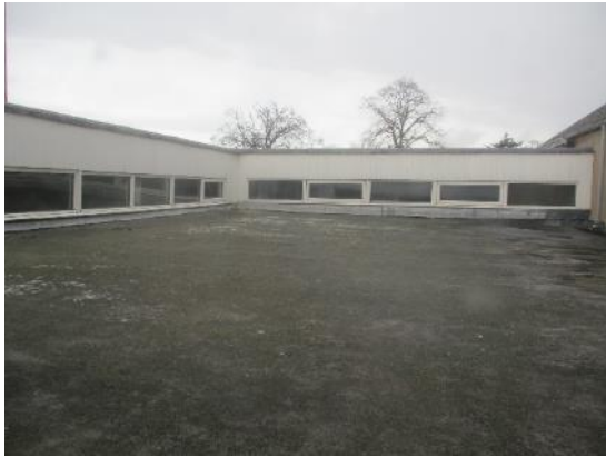
3. Mineral felt roof above Gym Hall
