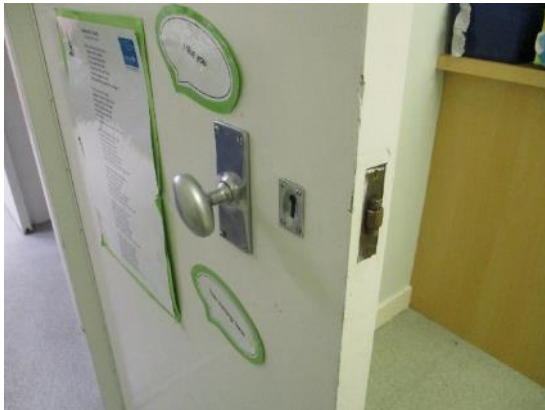
90. Roller ball catches to some doors
