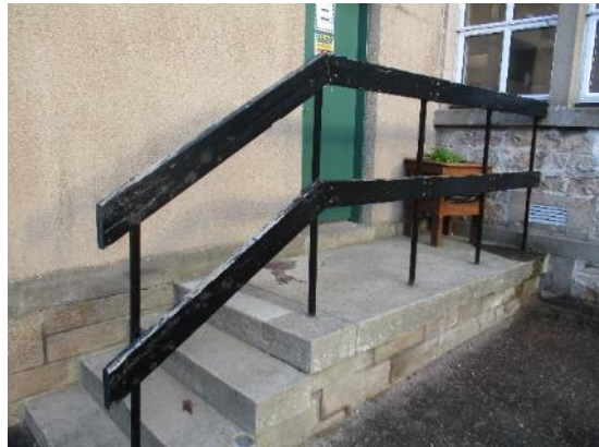
61. Timber handrail to Kitchen side door
