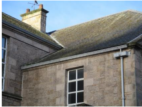
14. Cast iron ogee gutters
