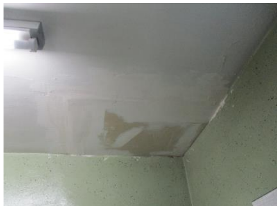
63. Repairs to plasterboard
