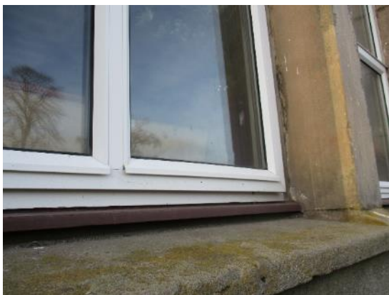
48. Timber window sills
