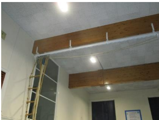
68. Gym Hall glulam beams and ceiling tiles
