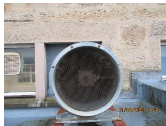
136. Specialist extract mechanical ventilation kitchen fan 1/11
