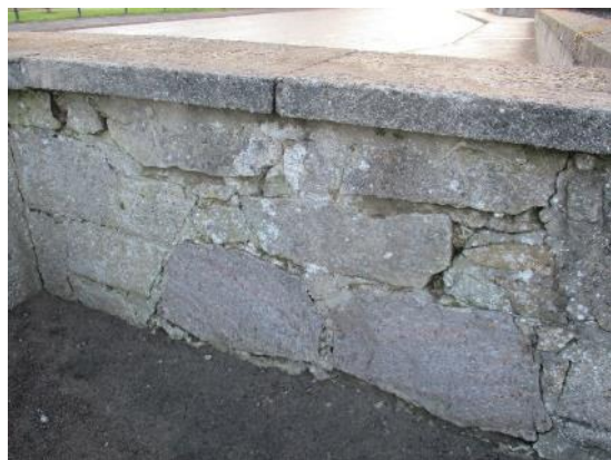
172. Perimeter wall pointing
