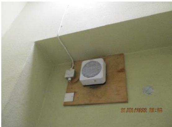
133. General extract mechanical ventilation 1/2a
