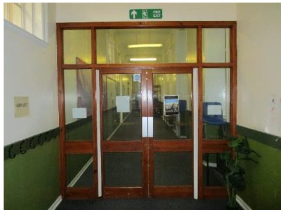
79. Corridor screen partitions
