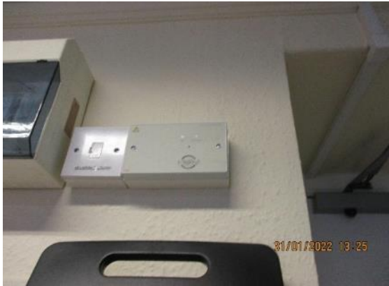
155. Disabled alarm system receiver unit - reception
