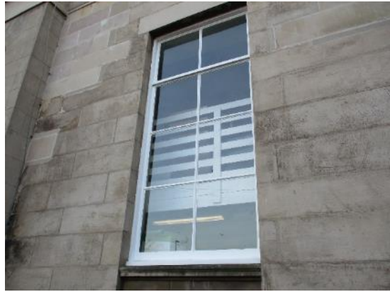
45. Timber framed windows
