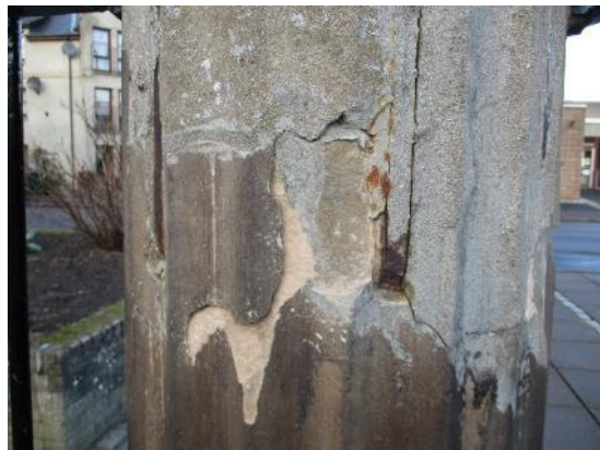
170. Exposed reinforcement
