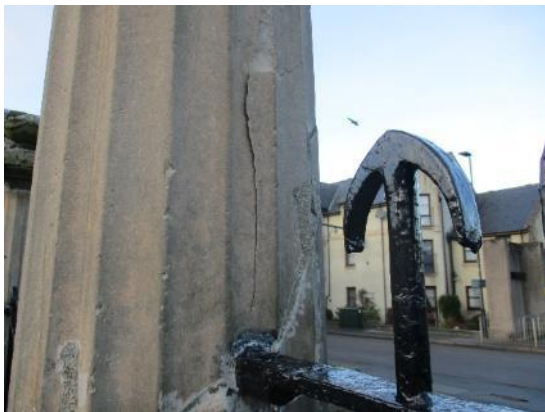
169. Stone cracking
