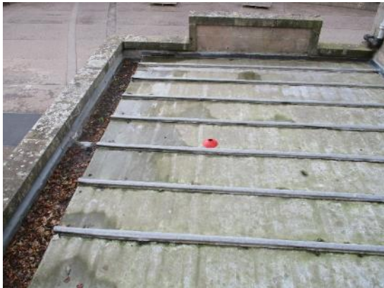
21. Lead roof box gutters
