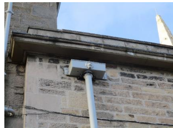
18. Cast iron hopper heads
