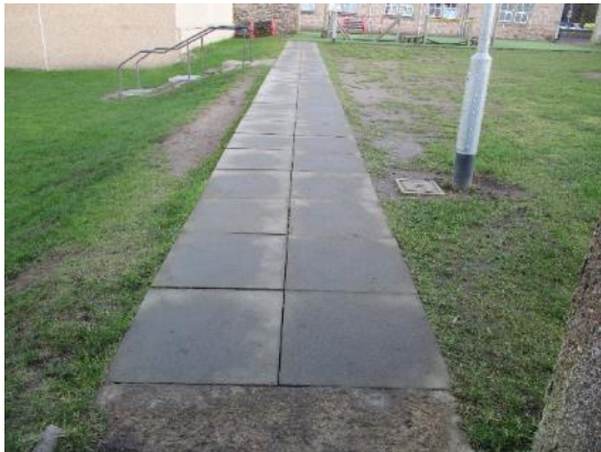
163. Paving slab footpath
