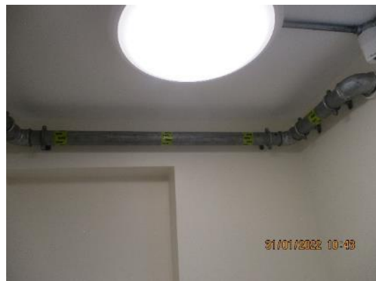
130. Gas supply (part) to kitchen internal 1/33
