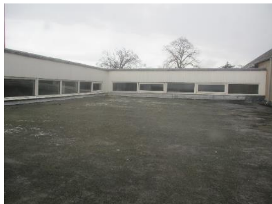
24. Parapet wall to felt roof
