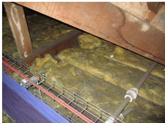
12. Mineral insulation over lath & plaster
