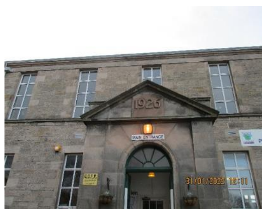
160. External CCTV camera main entrance
