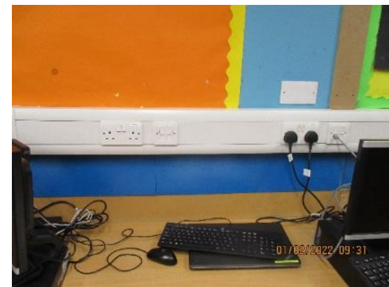
142. General wiring and dado trunking – class 2/30
