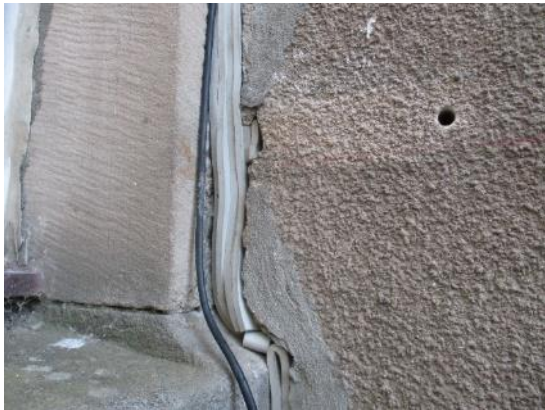
34. Expansion tape filling the gap
