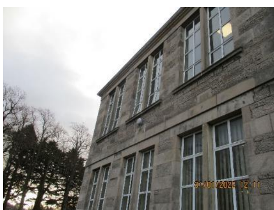
154. Period bell system (external bell)
