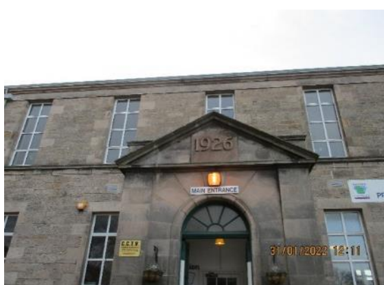
147. External building lighting
