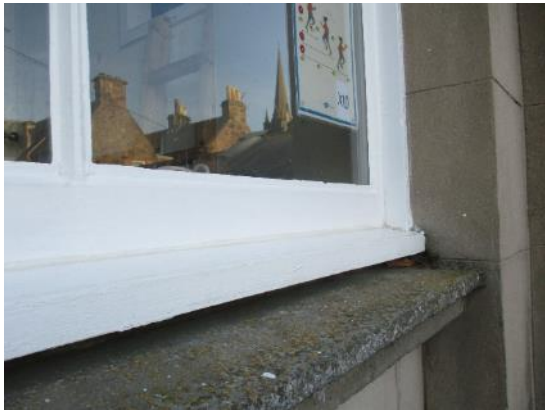
46. Timber window sills
