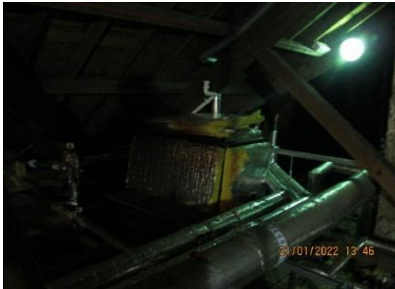
127. Cold water storage tank attic space
