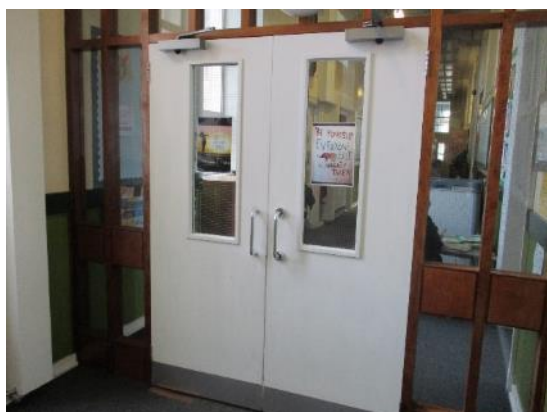
82. Timber double doors
