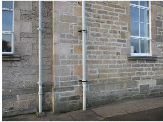
20. Cast iron down pipes
