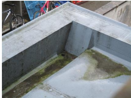
22. GRP roof box gutters
