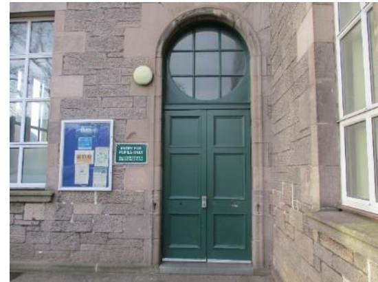
41. Timber fire escape doors
