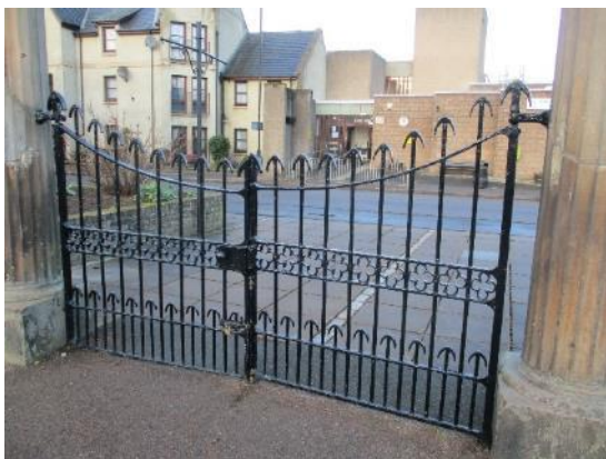
165. Cast iron gate (Listed)
