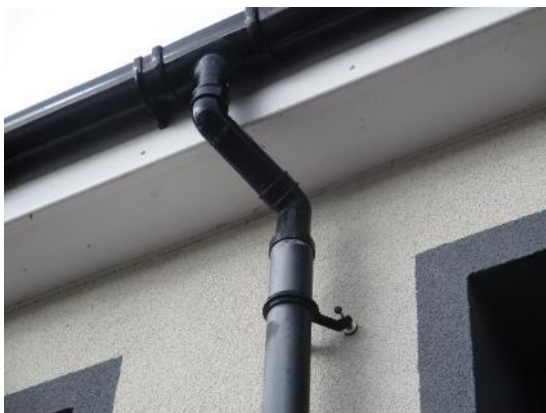
29. Various pipe diameters
