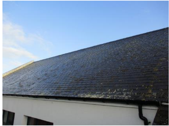
2. Slate roof above Assembly Hall
