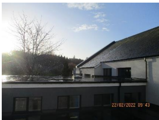
123. Specialist ventilation – kitchen canopy fan roof
