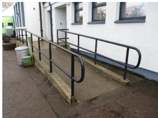
48. External ramps and handrails
