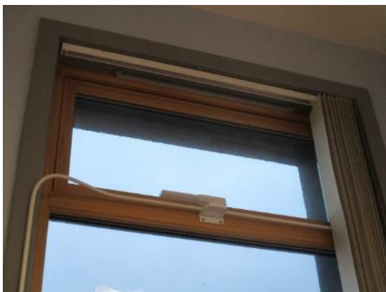
47. Mechanical top hopper mechanism
