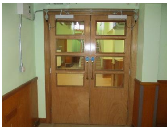
86. Replacement double doors
