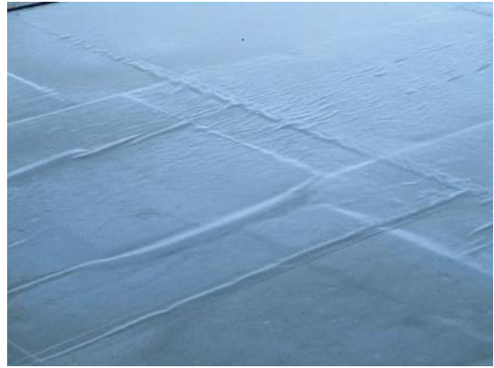
8. Wrinkled single ply membrane
