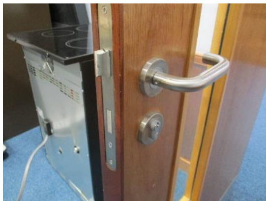
88. Replacement aluminium ironmongery
