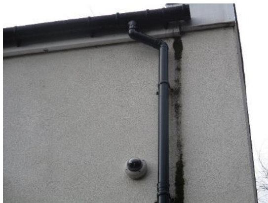
22. Leaking gutters
