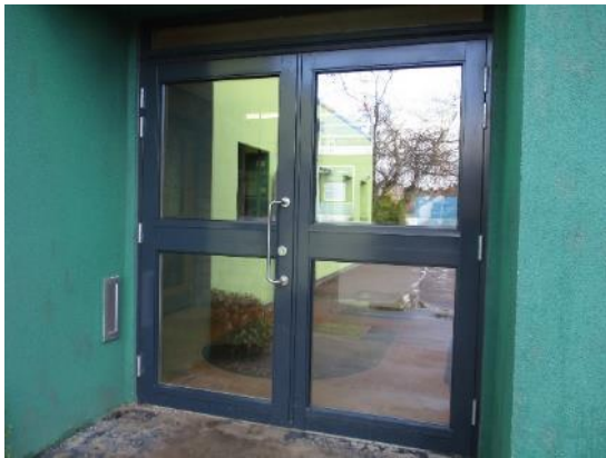
37. Main entrance doors
