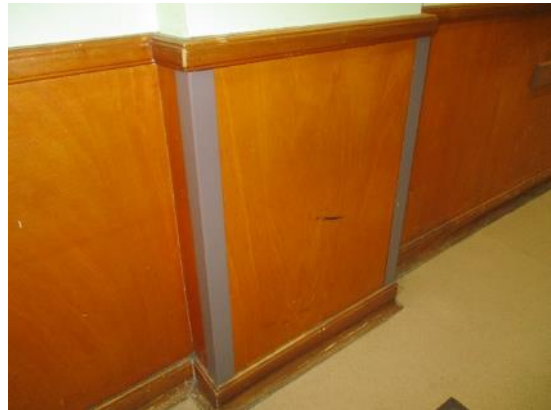
76. Timber panelling at low level
