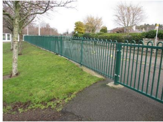
166. Metal railings to rear
