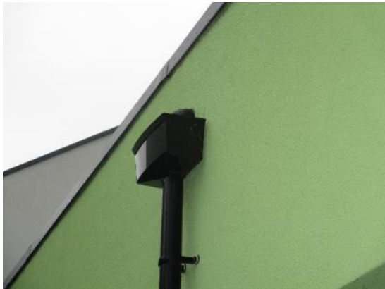
27. Flat roof hopper collection
