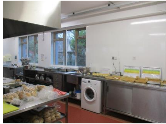
80. Wetwall in Kitchen
