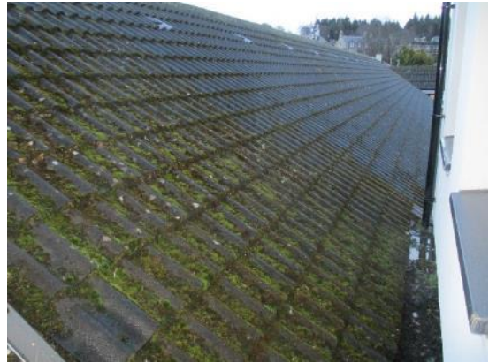
4. Tiled roof above SEN
