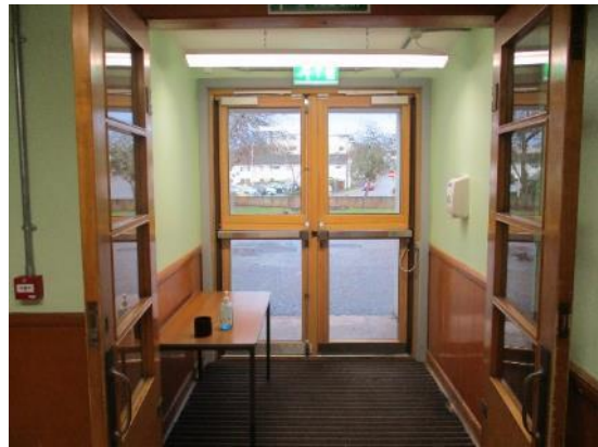
38. External doors internally
