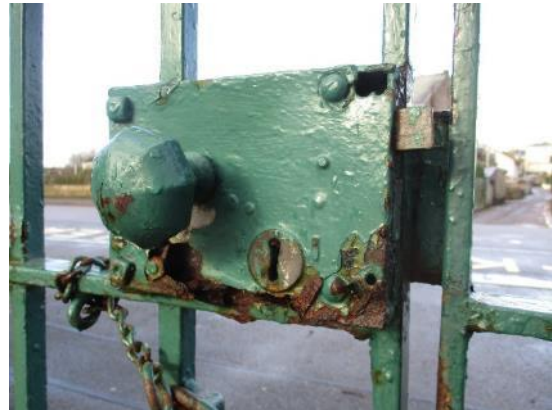
168. Extensive corrosion
