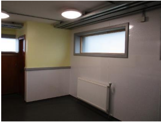
79. Wetwall in toilets
