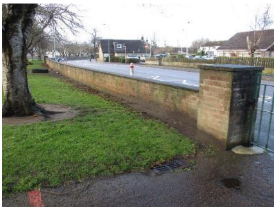
169. Brick wall to front
