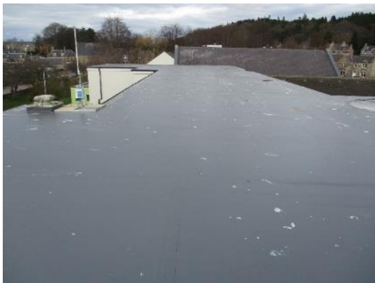
15. Two storey flat roof
