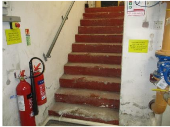
62. Concrete stairs to Boiler House
