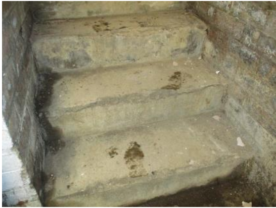
61. Concrete stairs to Basement Store
