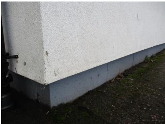
33. External wall insulation
