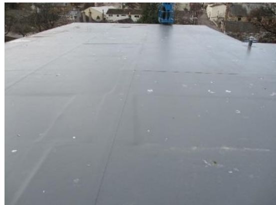
16. Insulation joints visible
