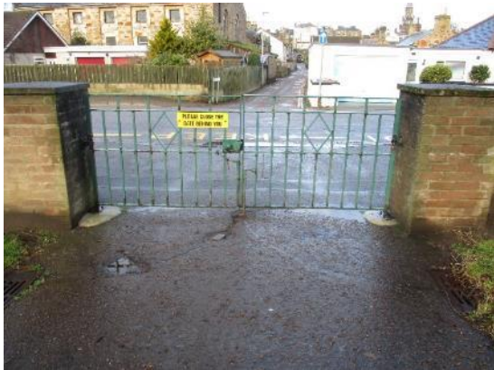
167. Typical metal gate
