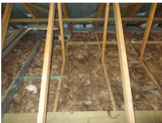
19. Mineral fibre insulation
