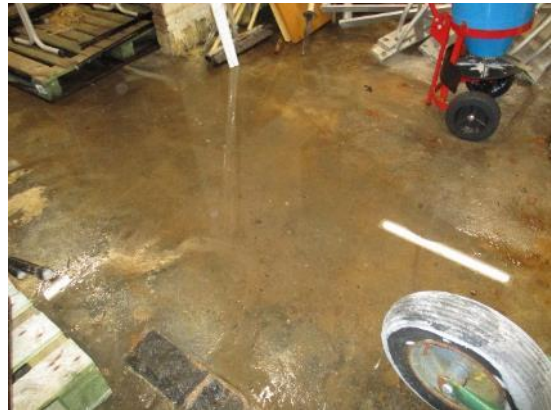
58. Concrete floor – Basement Store
