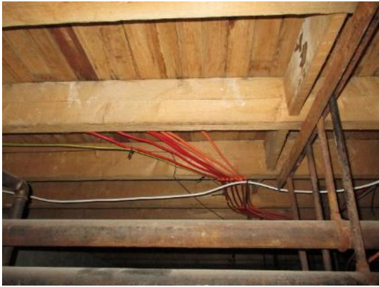
49. Suspended timber floor
