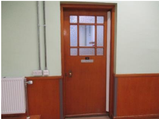
81. Original timber doors
