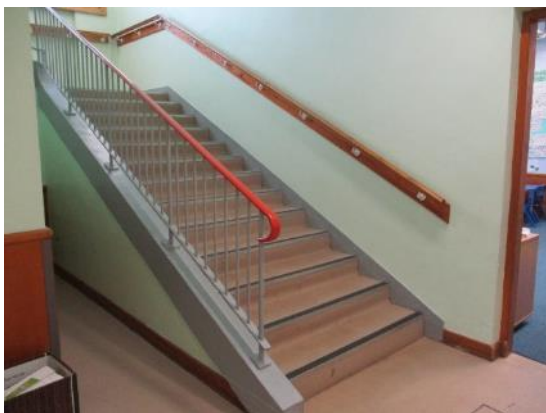
65. Timber and PVC handrails
