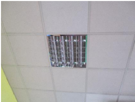
50. Classroom light main school.
