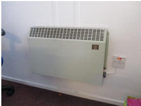
25. Portacabin electric convector
