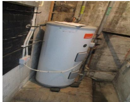
70. Unvented hot water storage cylinder
