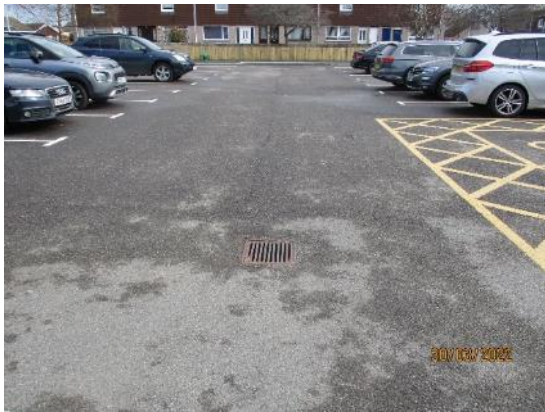
167. Tarmacadam car park
