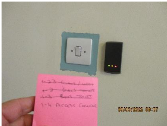
133. Security door card reader unit access corridor.
