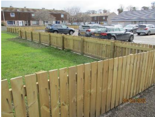
173. Timber fence to car park
