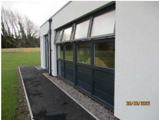
39. Large screen windows
