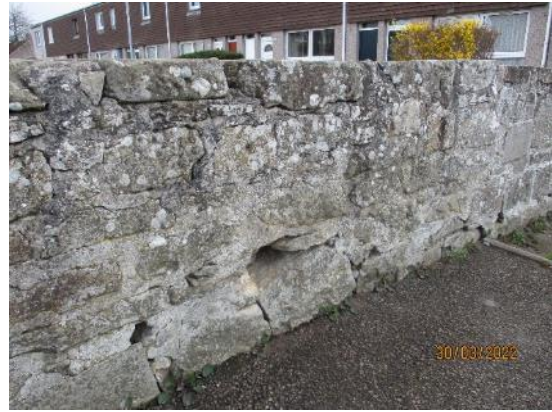
180. Stone wall to East boundary
