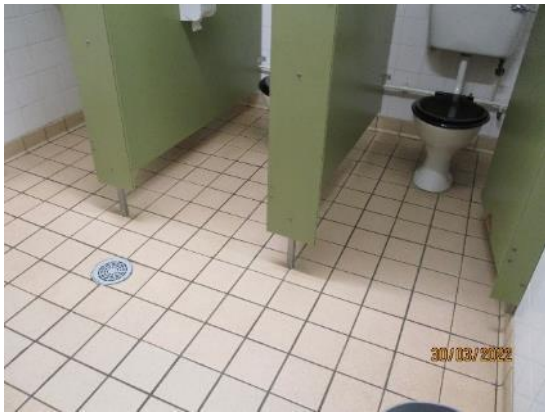
54. Quarry tiles in toilets
