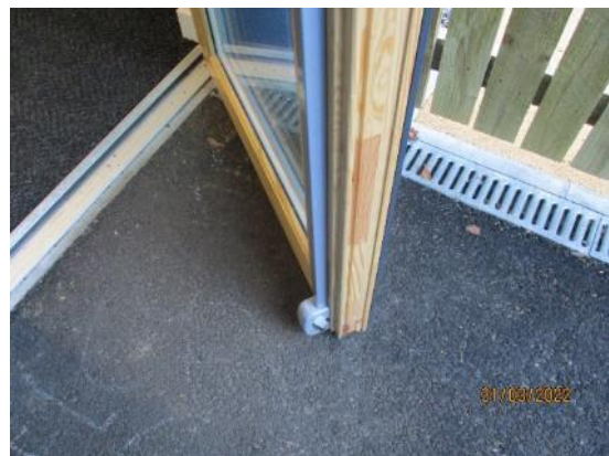
30. Timber doors with aluminium face
