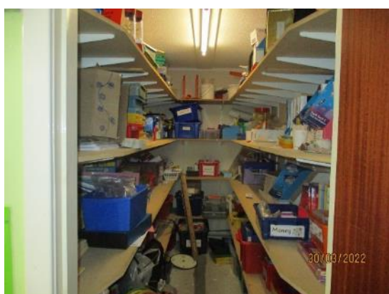
94. Cupboards lined with chipboard shelving
