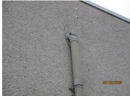
14. Games Hall downpipes
