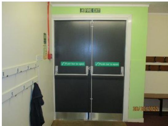
27. Fire exit doors internally
