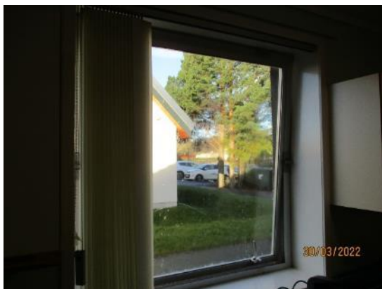
35. Centre pivot windows
