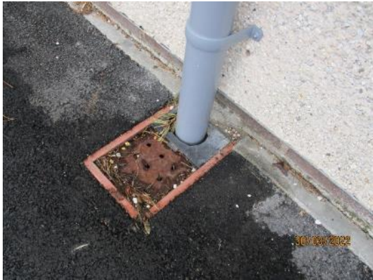
13. Downpipes to back inlet gullies
