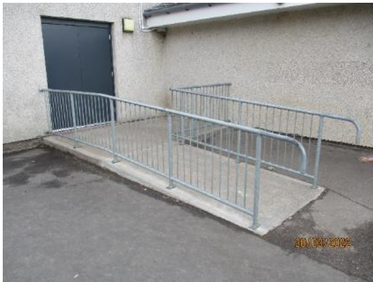
49. Ramped fire exit and galvanised guardrail
