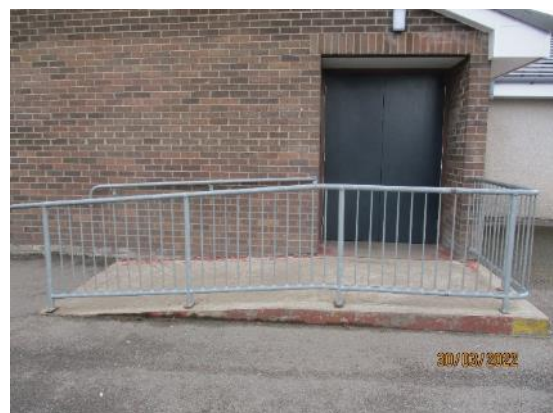
48. Concrete ramp and galvanised guardrail
