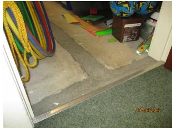
55. Concrete screed in cupboards
