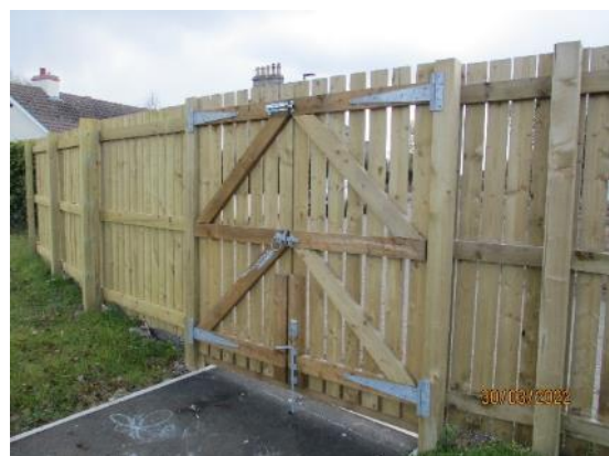
178. Timber gates to Annexe
