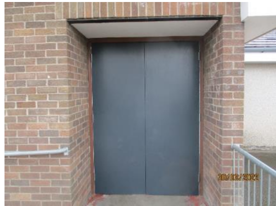
26. Fire exit doors
