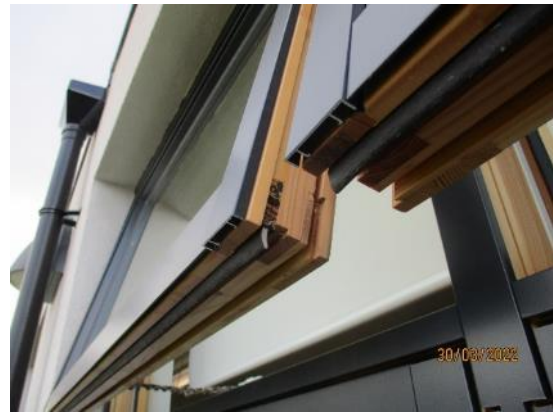
38. Timber with aluminium face
