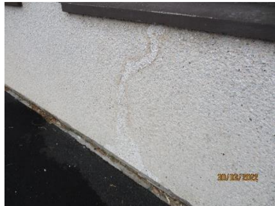
20. Roughcast repairs
