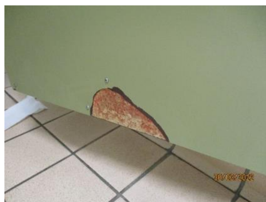
91. Chipped and broken surface
