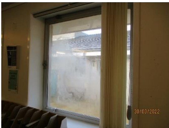
41. Blown double glazing – Primary School
