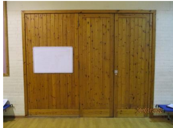
75. Timber lined doors in Gym Hall
