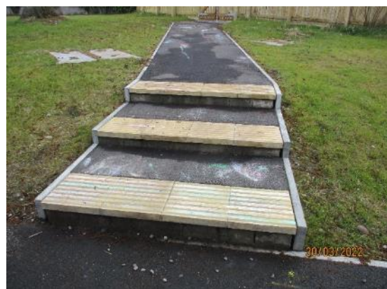
172. Steps to rear of Annexe
