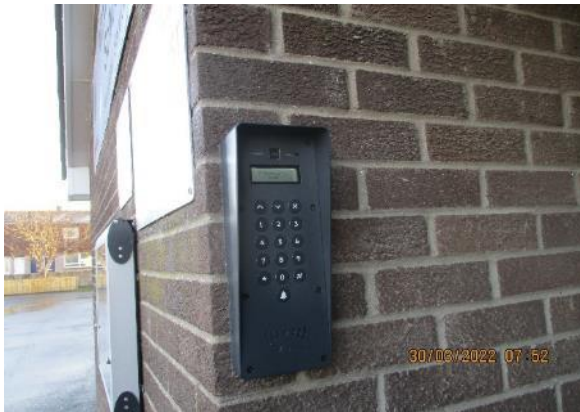
131. Door entry keypad and camera. Main entrance.
