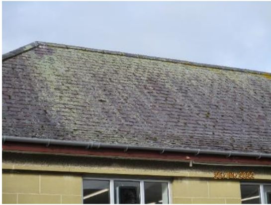
7. Dining Hall slate roof
