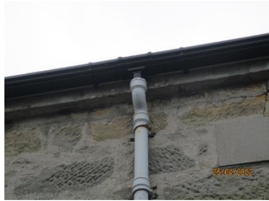
26. UPVC ogee gutter to school and Gym Hall
