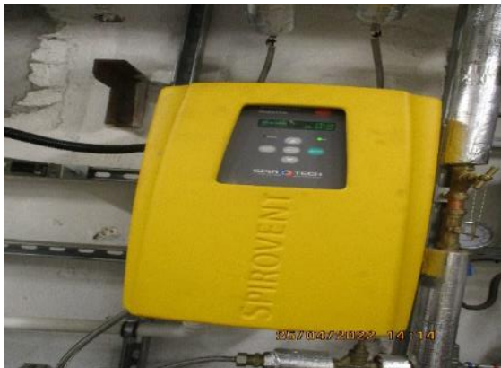
143. Spirovent fill and degasser unit – heating. 0/1
