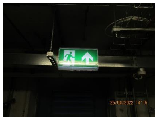
168. Emergency exit lighting – typical.
