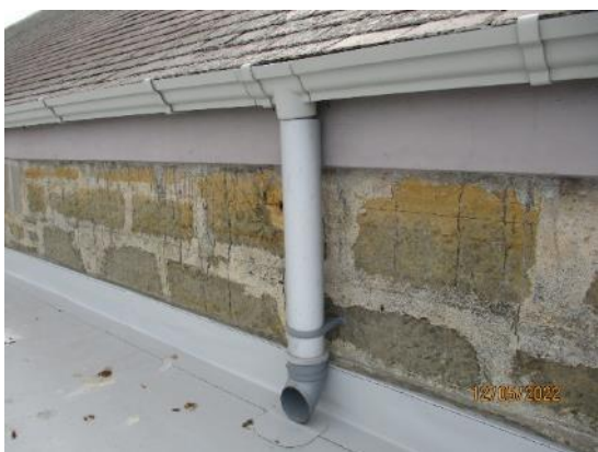
23. Steel ogee gutter to main school
