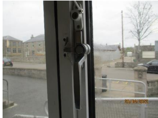
62. Defective/missing ironmongery
