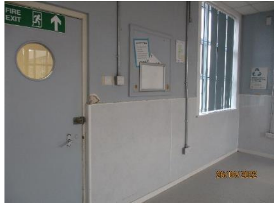
108. Wetwall to Dining Room walls
