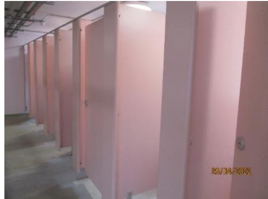
126. Composite cubicle partitions
