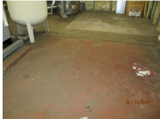
85. Boiler room painted concrete floor
