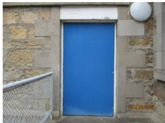
65. External timber doors
