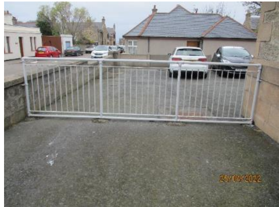
228. Metal railing fence
