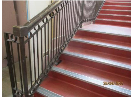
91. Timber handrails and metal balustrades
