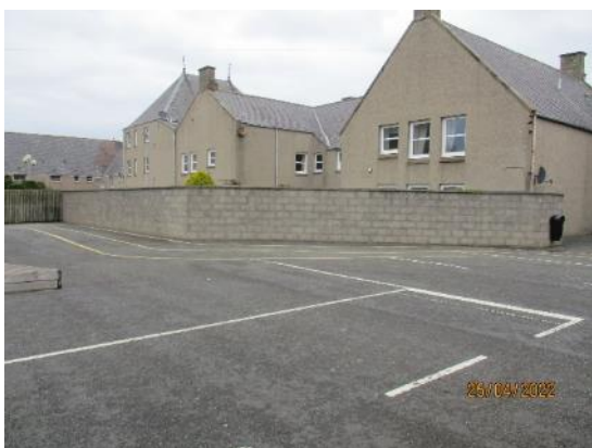
235. High blockwork wall
