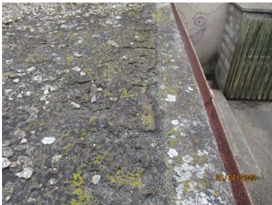
15. Felt cracking and crazing
