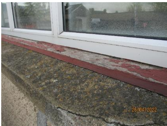
64. Timber window sills
