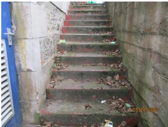
70. Concrete stair to Boiler Room
