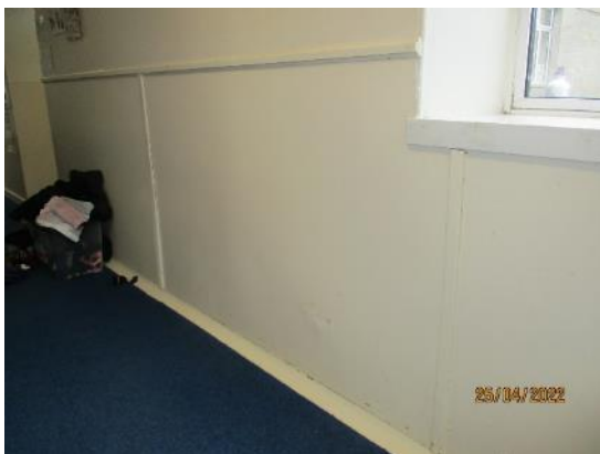
105. Fibreboard linings
