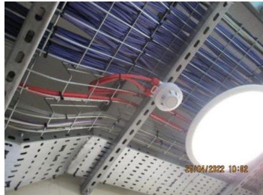
174. Fire alarm system wiring – typical.
