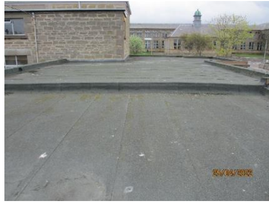
8. Mineral felt to single storey flat roofs
