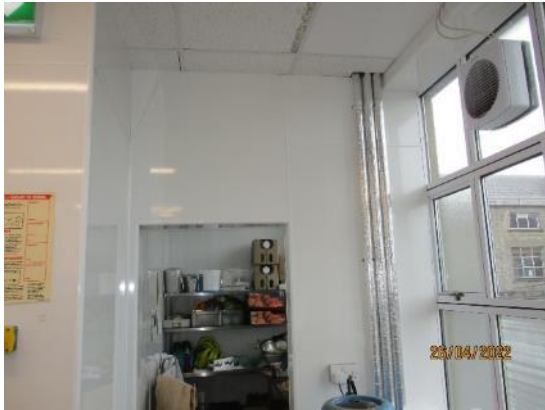
107. Wetwall to Kitchen walls
