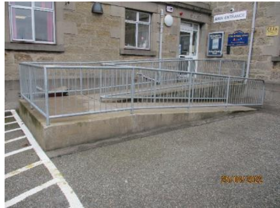
75. Galvanised guardrails
