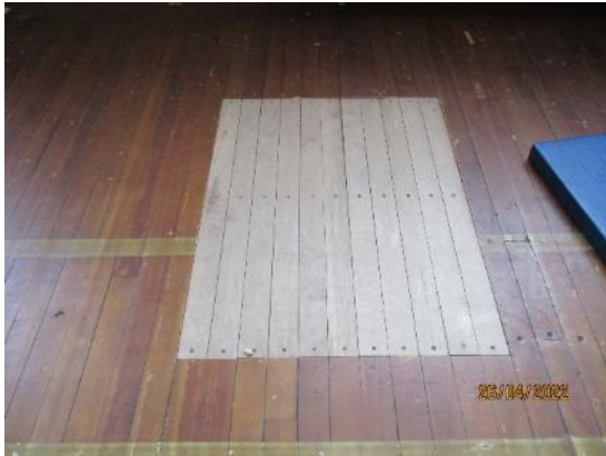
84. Timber flooring repairs
