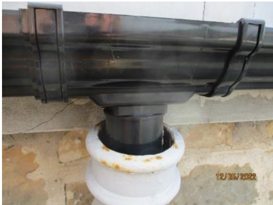
27. UPVC ogee gutter outlets
