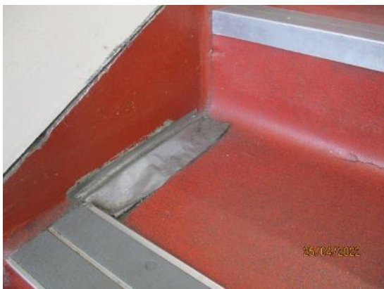
88. Vinyl taped repairs
