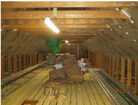
3. Dining Hall roof structure
