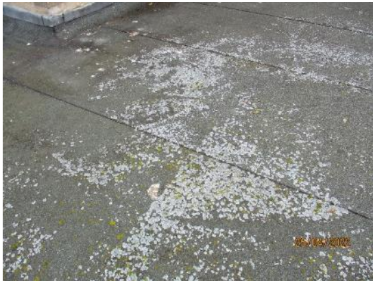
9. Lichen on the surface of felt roofs
