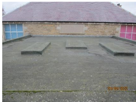
6. Slated roof to Gym Hall
