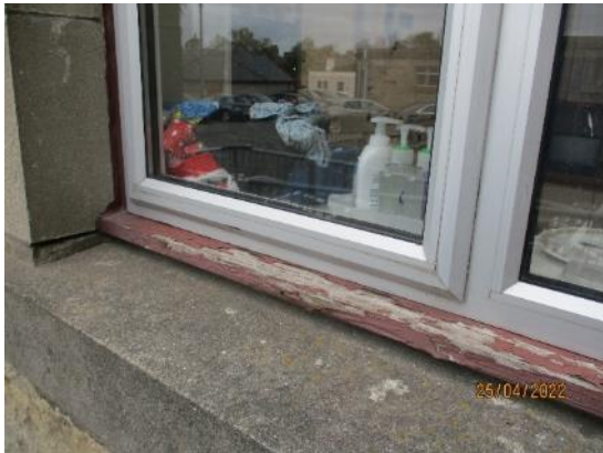
57. Timber window sills
