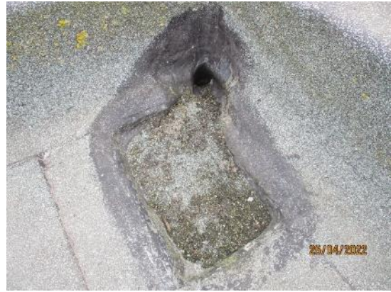
32. Small outlets to felt roofs
