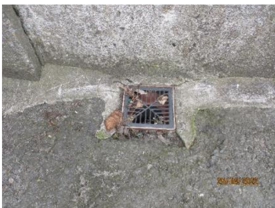
241. Car park gully
