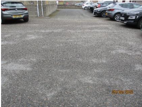
219. Tarmacadam car park
