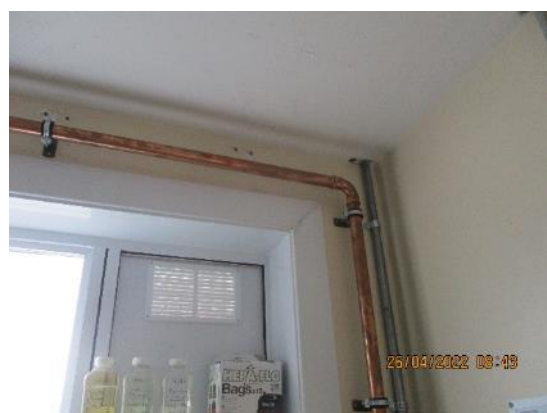
200. Gas pipework – copper distribution plant room 1/50
