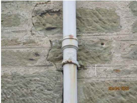
66. Cast iron rain water goods
