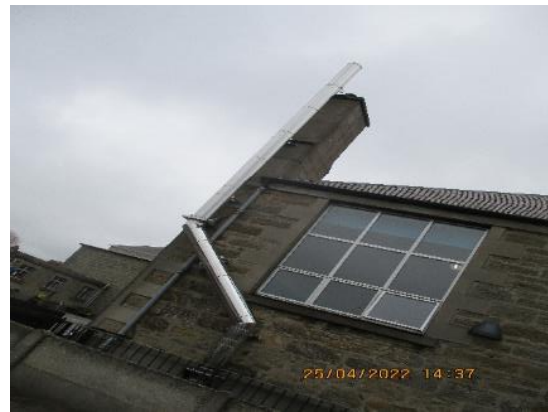
142. Boiler common flue external.
