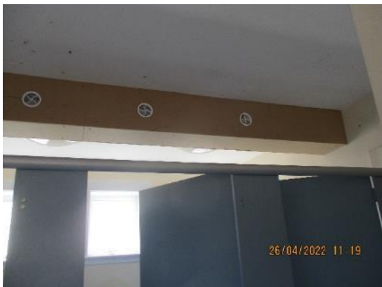
193. Boiler flue. Boxed in through boys toilets 1/52.
