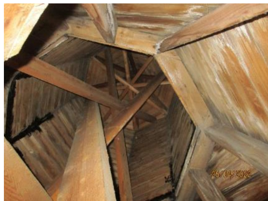
36. Tower's timber structure
