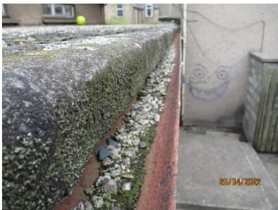
29. 1/2 round cast iron gutter to Dining Hall
