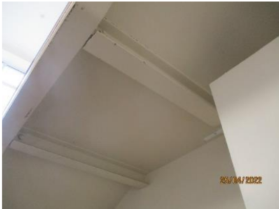
86. Steel and concrete staircases
