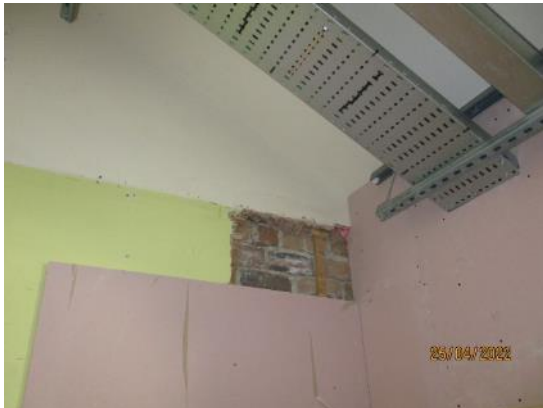
97. Brick and plastered internal walls
