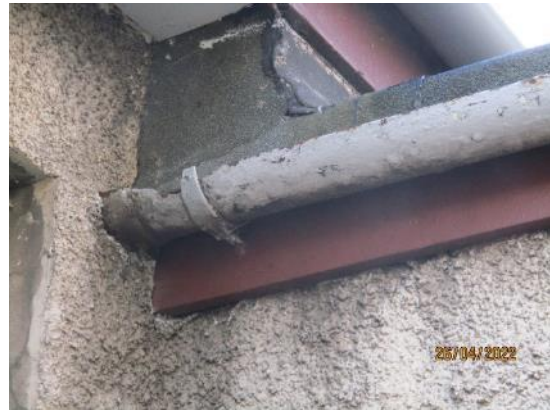
28. 1/2 round cast iron gutter to Dining Hall
