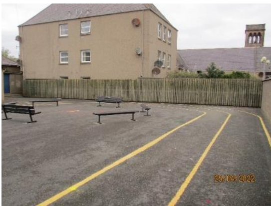
229. High, close boarded fence
