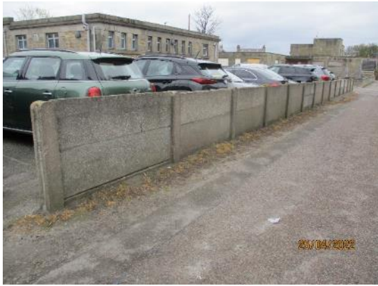
225. Concrete post and panel fence
