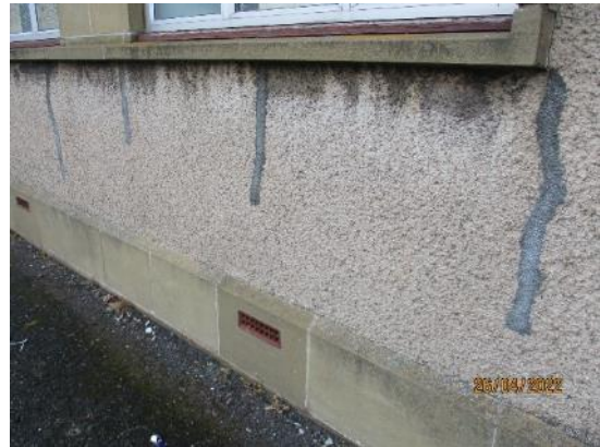
46. Dining Hall, repairs to roughcast
