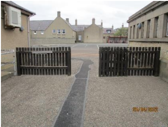
227. Timber fence and gate
