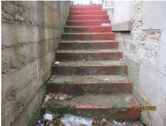
72. Concrete stair to Boiler Room
