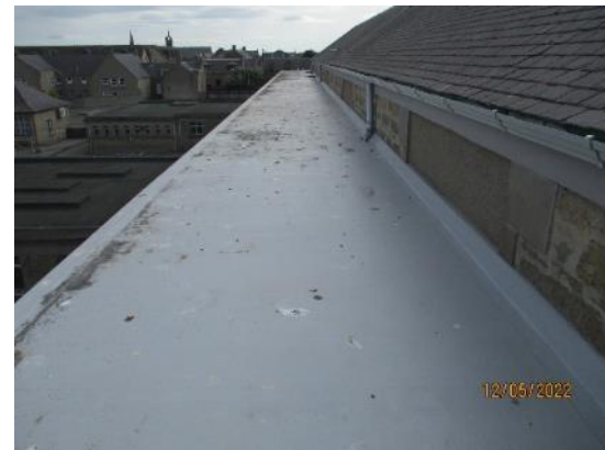
16. Single ply membrane to high level flat roof
