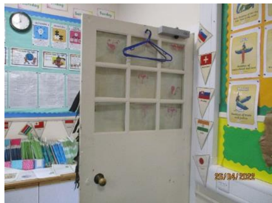
112. Timber classroom doors with glazing panels
