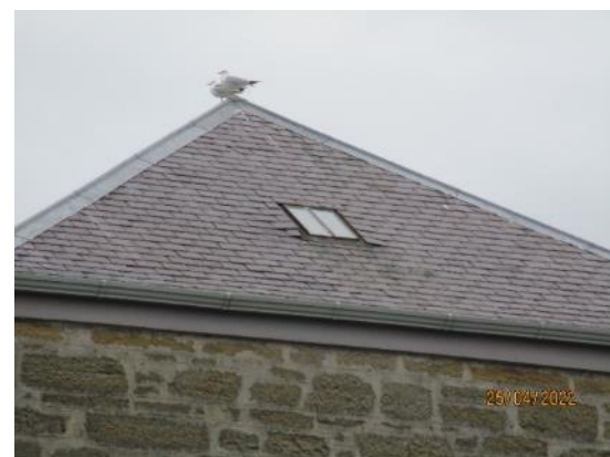
18. Skylight to main school roof
