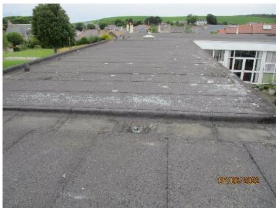
5. Steps in felt roofing
