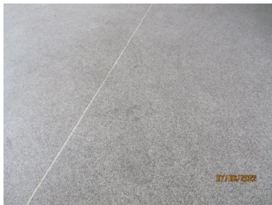
48. Sheet vinyl to toilets
