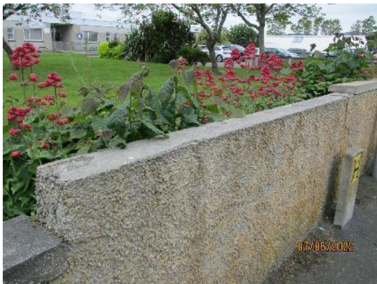
181. Missing coping stones
