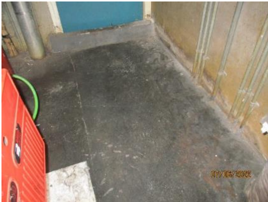
57. Concrete screed to boiler room
