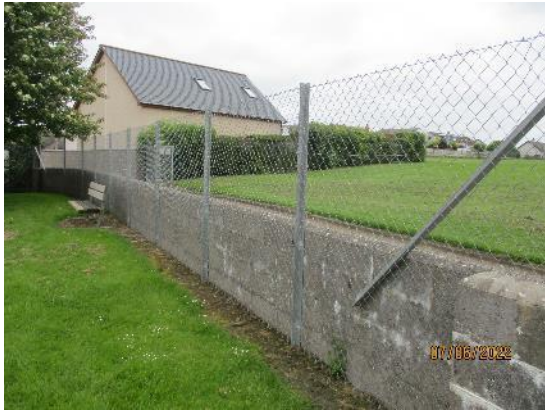
173. Chain link fence to rear wall
