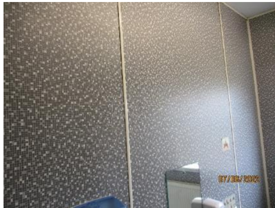
67. Wetwall in toilets
