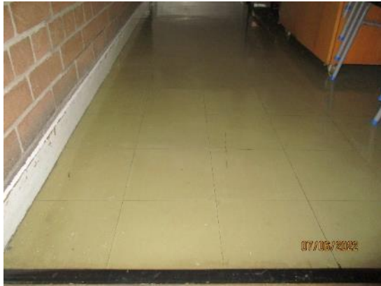
49. Vinyl tiles to corridor
