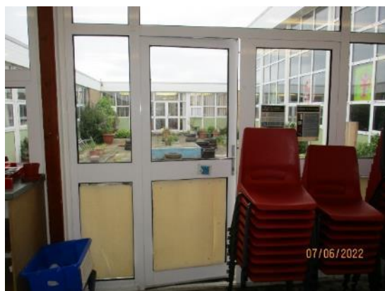
24. Courtyard door and screen
