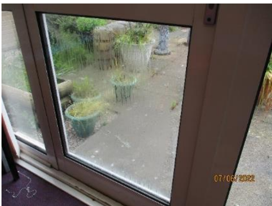
41. Blown double glazing units
