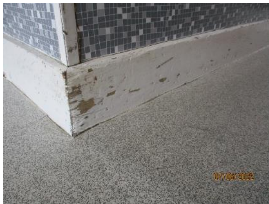
94. Timber skirting boards
