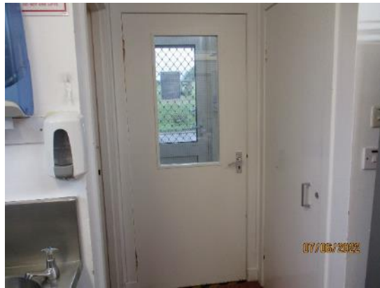
73. Timber doors with vision panels
