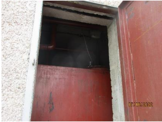
113. Oil storage tank. 1-36
