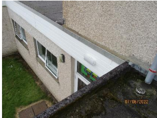
138. External emergency exit light typical. Kitchen.
