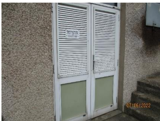
23. Boiler house double doors
