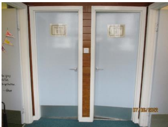
76. Timber doors to toilets
