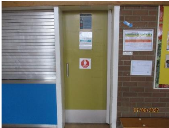
72. Timber internal doors
