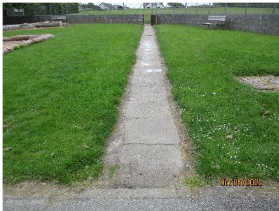
169. Paving slab footpath
