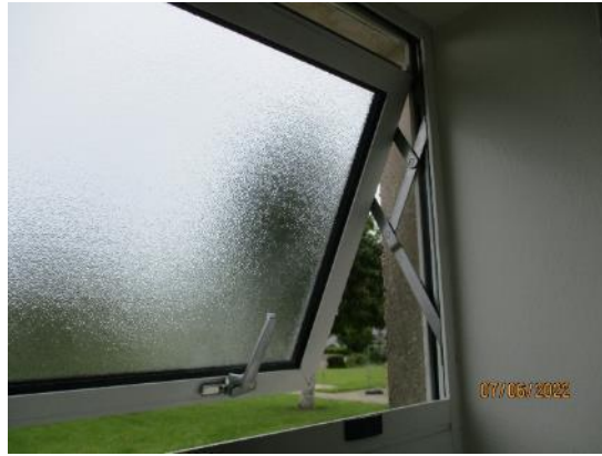
32. Friction hinge mechanism
