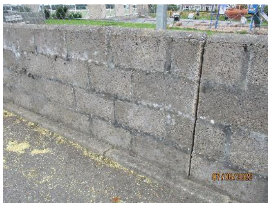
183. Rear blockwork wall
