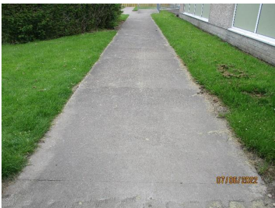
165. Cast in-situ concrete footpath
