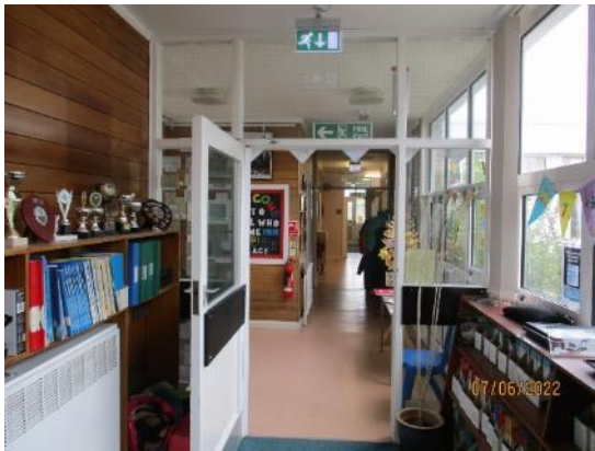
78. Corridor screen doors
