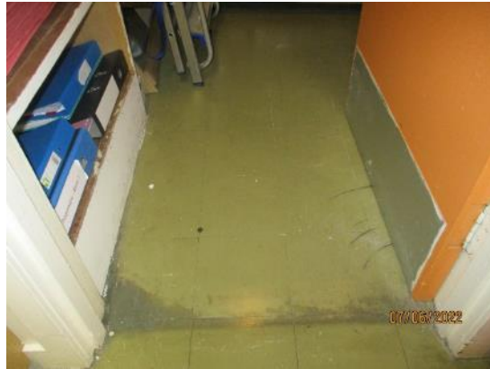
50. Vinyl tiles to cupboards
