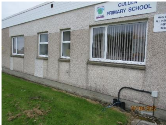
15. Patch repairs to roughcast
