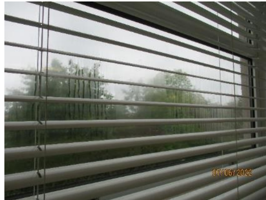
40. Blown double glazing units
