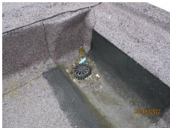
12. Deep box gutters
