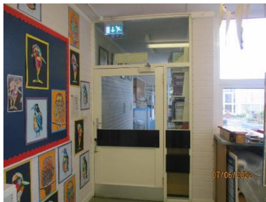
77. Corridor doors with glazed screen
