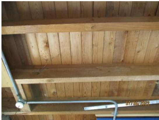
1. External store roof
