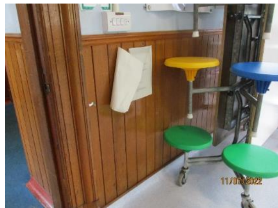
95. Timber linings to dado level
