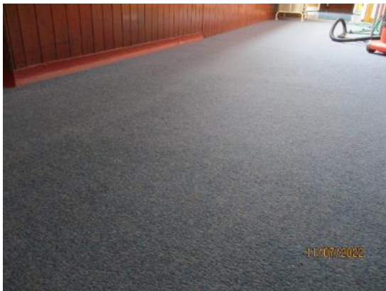
62. Concrete ground floor with raised ridge
