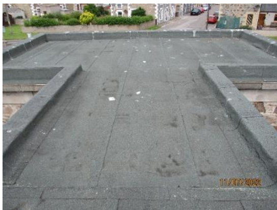
5. Felt roof above toilets
