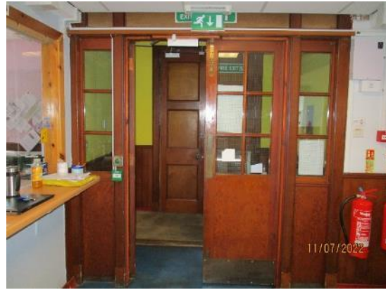
103. Vestibule timber doors and side screens
