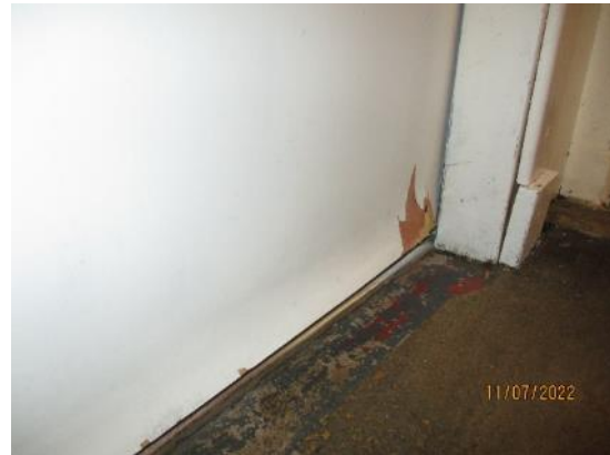
39. Rot and lamination to bottom edge
