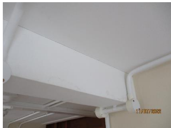
83. Plastered ceilings with concrete beams
