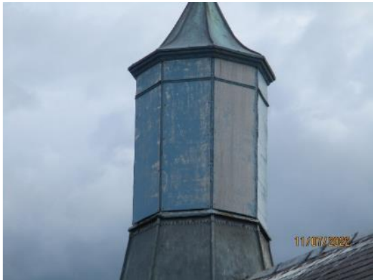
27. Timber cladding to belltower
