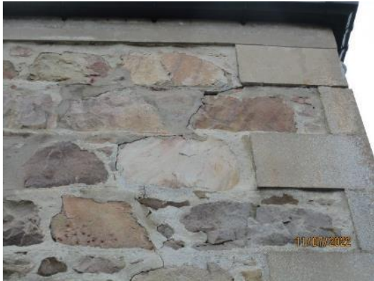
30. Isolated cracking
