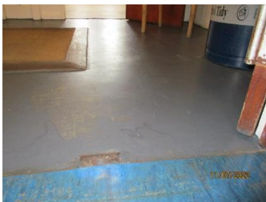
72. Painted concrete floors
