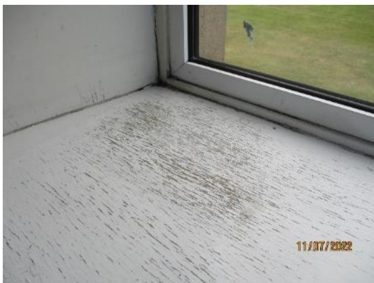
100. Plywood window sills
