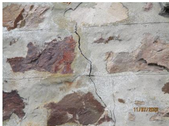
29. Vertical cracking
