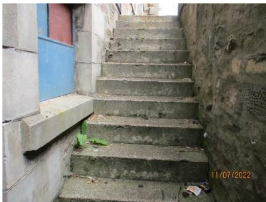
58. Concrete steps to Boiler House
