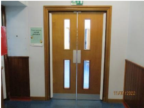
104. Replacement timber double doors
