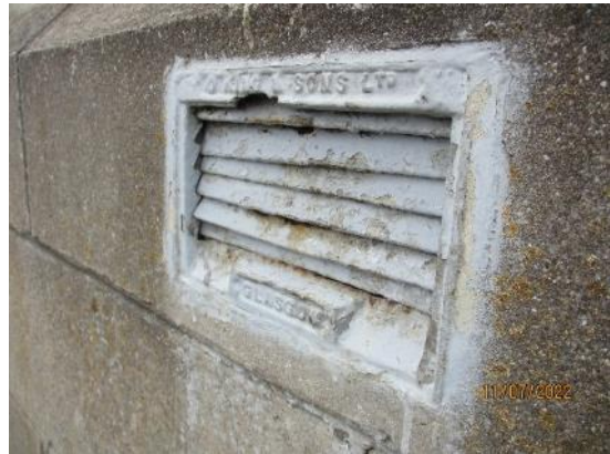
33. Damaged vents
