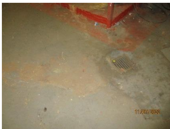
73. Boiler House concrete floor
