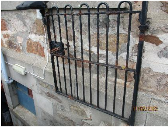
199. Metal framed gate
