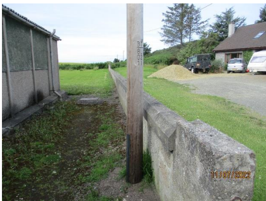
215. Timber utility pole
