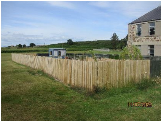
193. Timber boarded fencing
