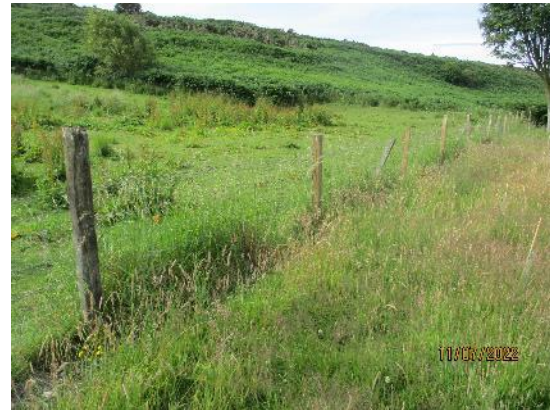
194. Timber post and wire fencing
