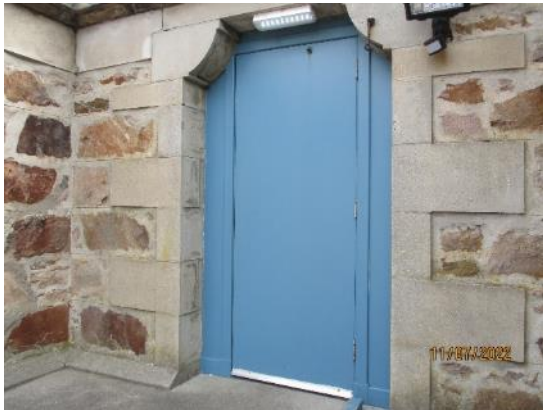
38. Timber fire escape doors
