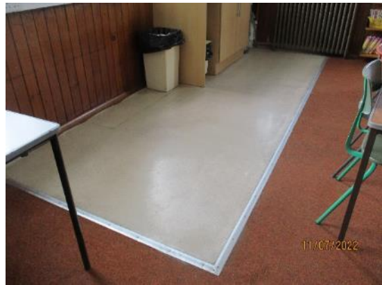
67. Sheet vinyl to kitchen sink areas
