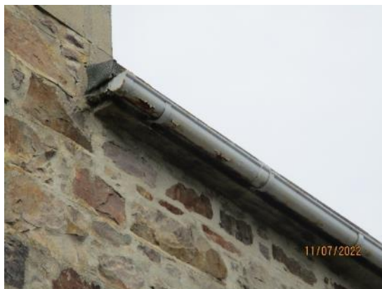
16. Cast iron gutter to first floor corridor
