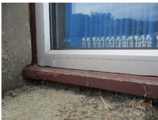
52. Timber window sills
