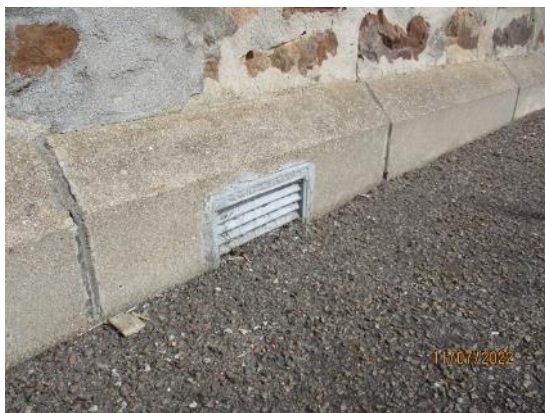
34. Ground level to rear
