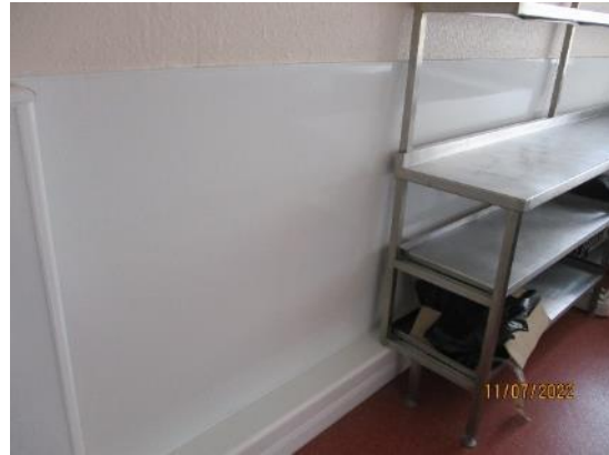
97. Wet wall to various walls
