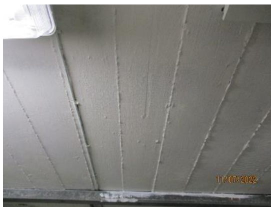
89. Concrete ceiling in Boiler House
