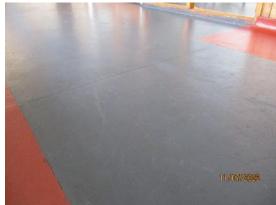
63. Concrete first floor with paint finish
