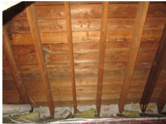
2. Timber sarking boards
