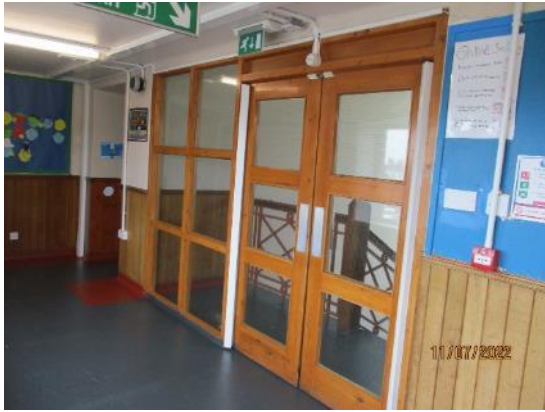
102. Timber doors and screens to stairs
