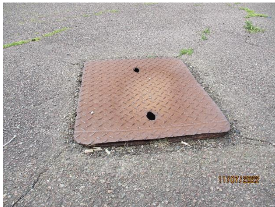
207. Raised playground inspection chamber
