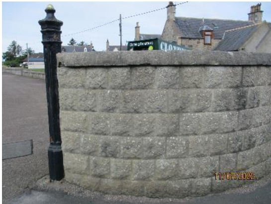
201. Concrete block walls
