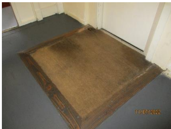
74. Timber frame to coconut matting
