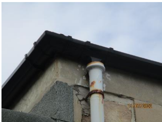
15. UPVC ogee gutter to Games Hall
