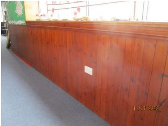
96. Timber linings to corridors
