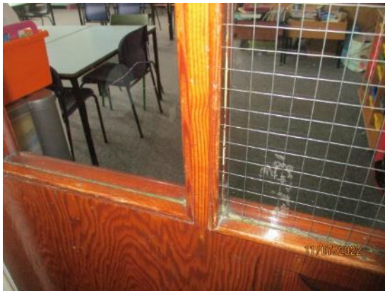
108. Mixed glazing to some doors
