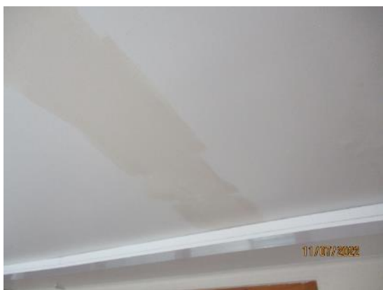
88. Patch repair to plasterboard ceiling
