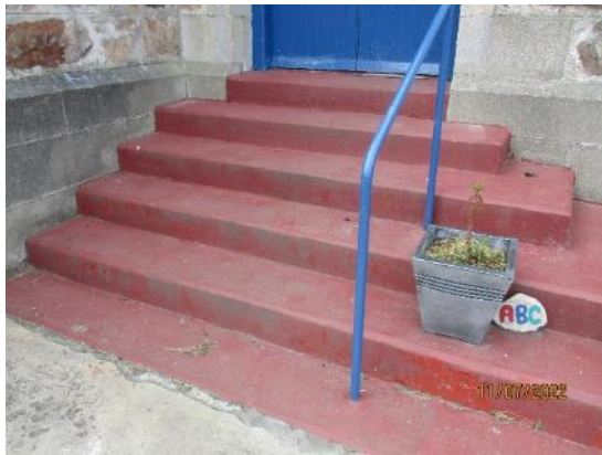
54. Concrete steps to front entrance
