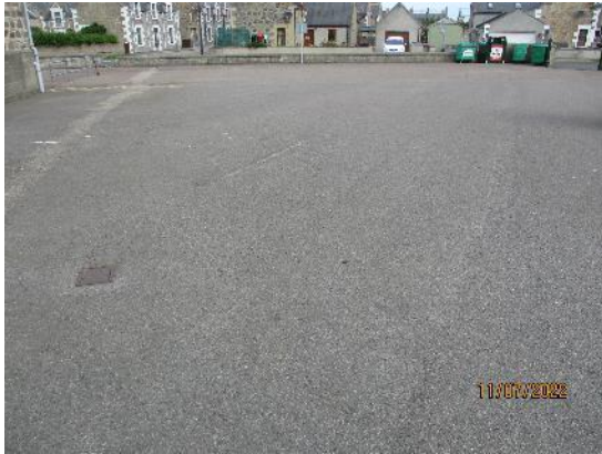
185. Tarmacadam car park
