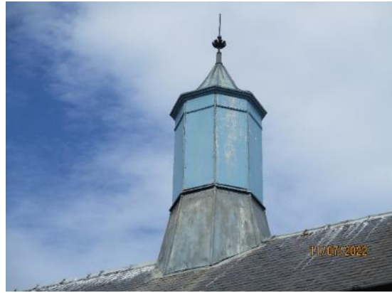
26. Octagonal bell tower with metal capping and skirt
