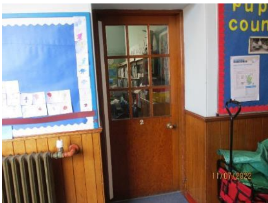
106. Timber doors to classrooms
