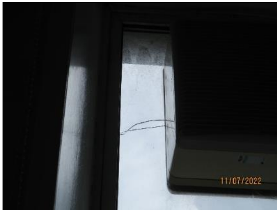
48. Broken double glazing unit
