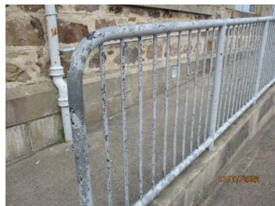
53. Railings and guard rails
