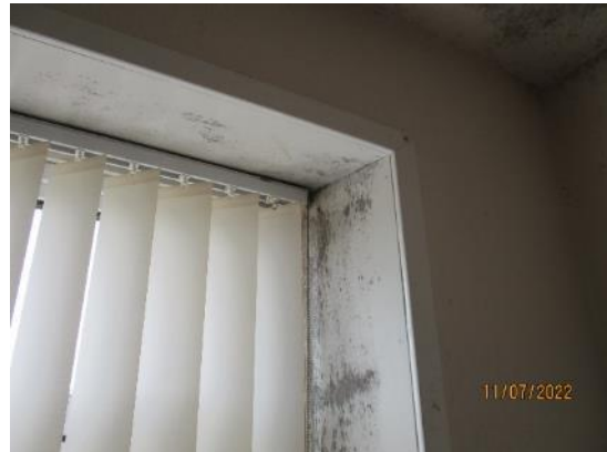
99. Plywood window reveals
