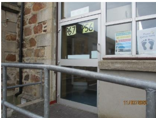
40. Aluminium doors to ramped access
