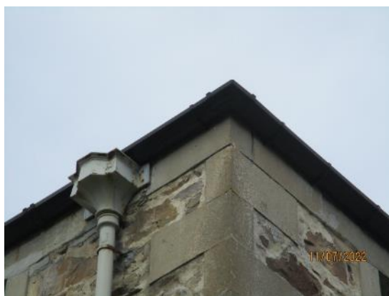
14. UPVC ogee gutter to main building
