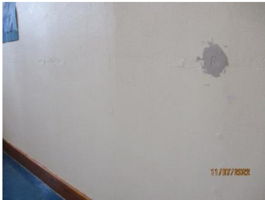
90. Repairs to plasterboard walls
