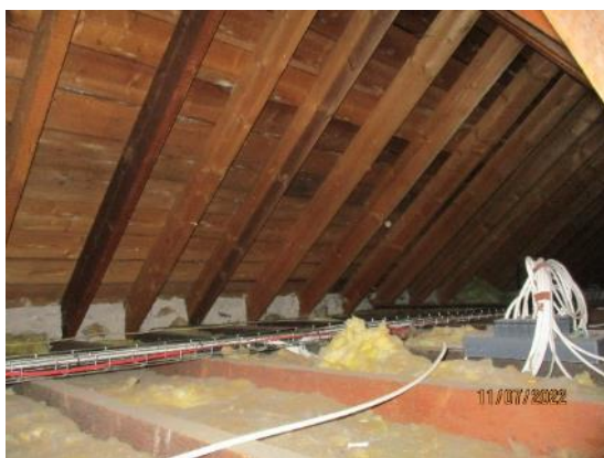
13. Insulation between ceiling ties
