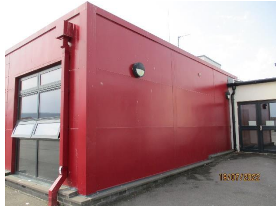
26. Smooth metal cladding to pods extension
