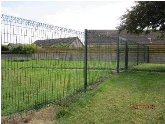
210. Security mesh fencing
