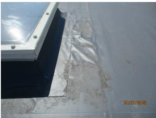
5. Wrinkled single ply membrane
