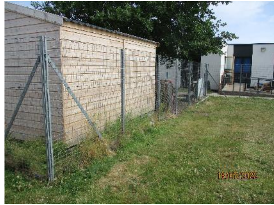
209. Galvanised mesh fencing
