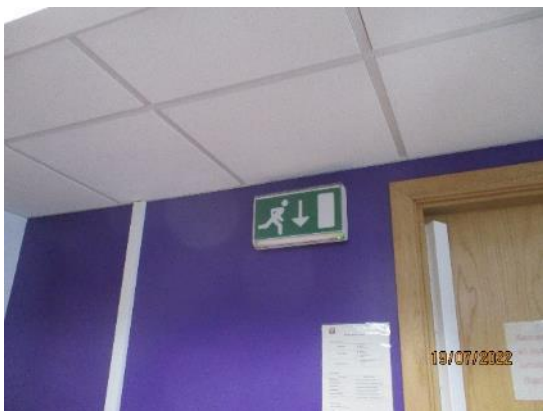
176. Emergency exit non maintained sign light – typical.
