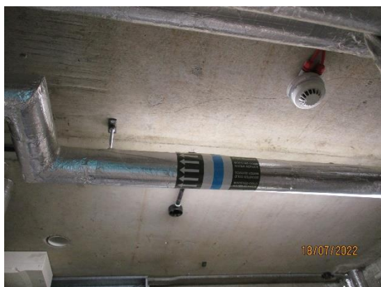
77. Concrete ceilings to plant rooms
