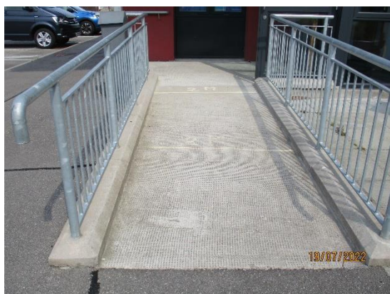
43. Concrete ramp to main entrance
