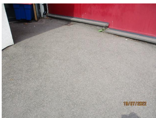
47. Tarmac ramp to fire exits
