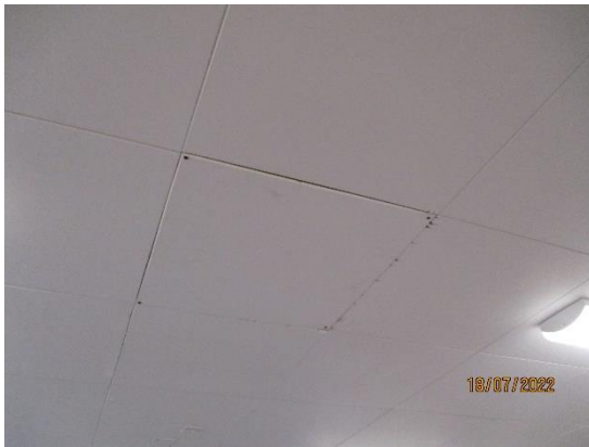
65. Fibre ceiling tiles
