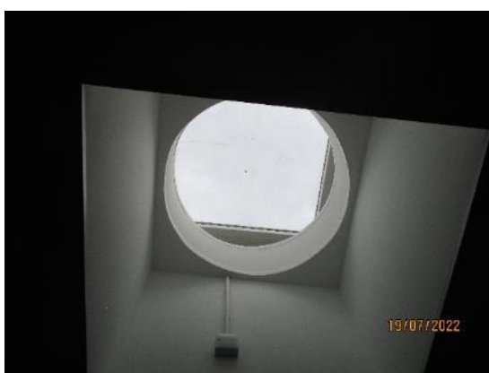
152. Passivents – modular classrooms. Typical.
