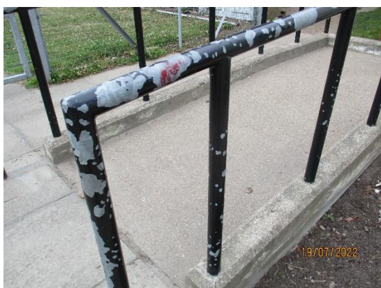
51. Tubular guard rail to Nursery
