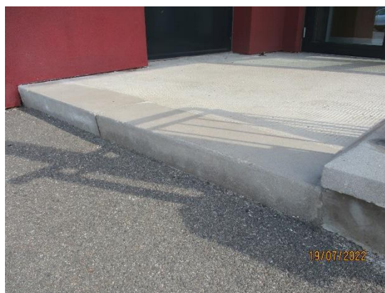
44. Concrete step to main entrance
