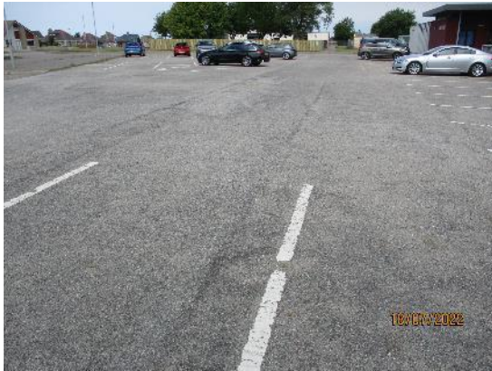
196. Tarmacadam car park
