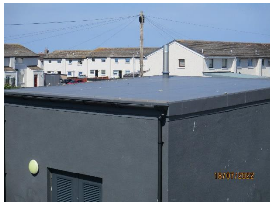
6. Boiler house single ply membrane
