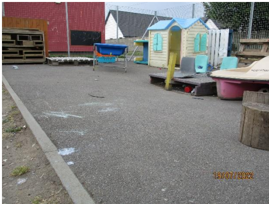
220. Sunken Nursery playground/drainage
