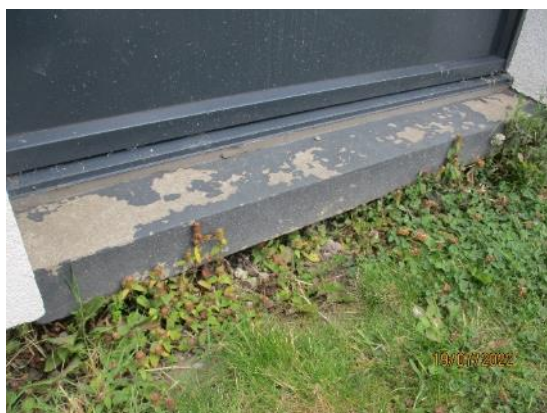
41. Painted concrete sills
