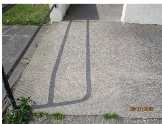
48. Concrete ramps to fire exits
