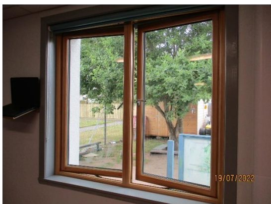
37. Typical window (internally)
