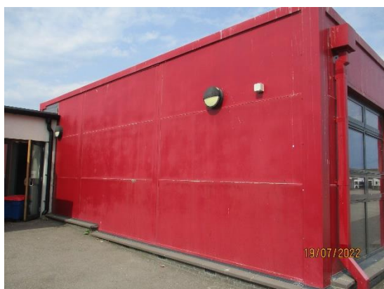
39. Smooth cladding to pods extension
