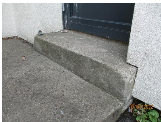
46. Concrete steps to fire exits
