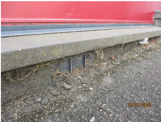
54. Ventilation below suspended timber floor
