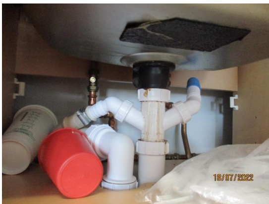
109. PVC waste pipes
