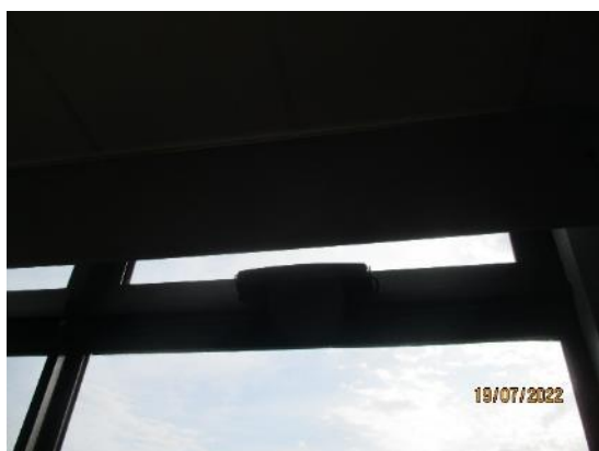
156. Electrically operated windows. Modular classrooms.
