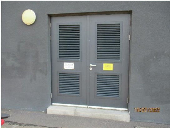
31. Boiler house timber louvred doors
