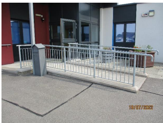
49. Tubular guard rail to front entrance
