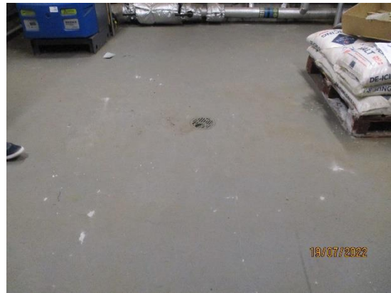
55. Boiler house concrete floor
