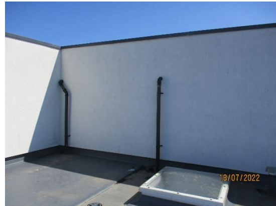
16. Downpipes from Games Hall roof
