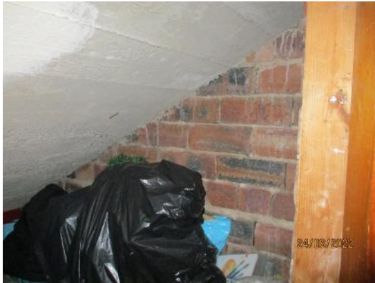
109. Brickwork below staircases
