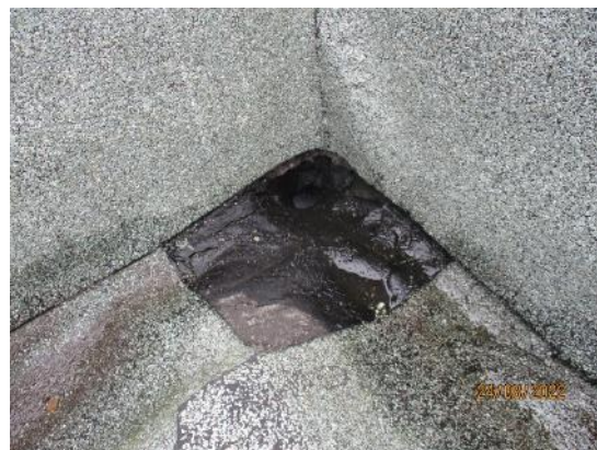
18. Felt lined box gutters
