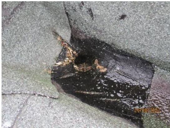
19. Narrow outlets from flat roofs
