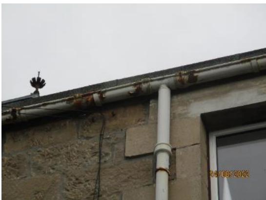
17. Cast iron gutters to first floor corridor
