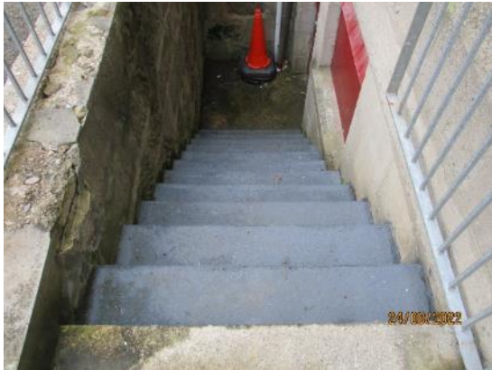
62. Concrete steps to Boiler House
