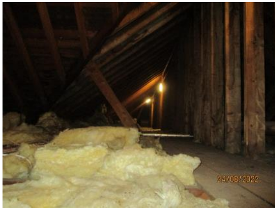
1. Main school trussed roof
