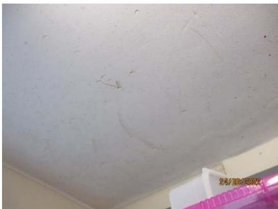
107. Polystyrene sheet to store ceiling 1/19
