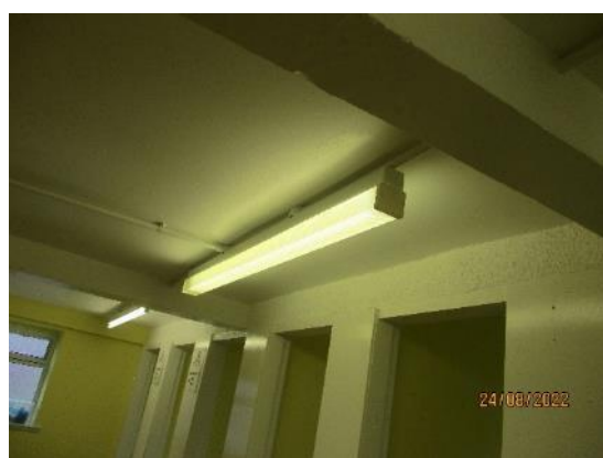
212. Lighting – pupils toilets.
