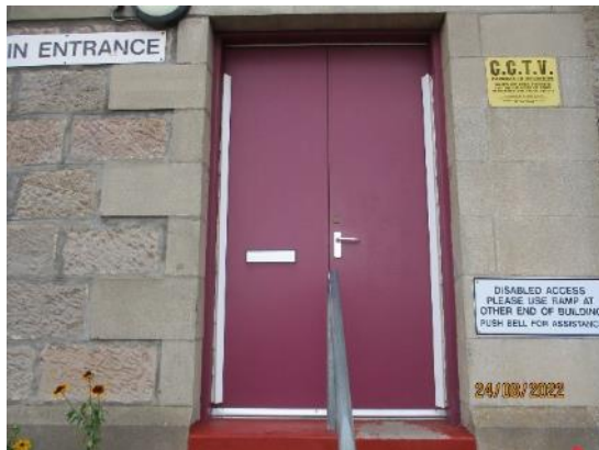
33. Timber entrance doors
