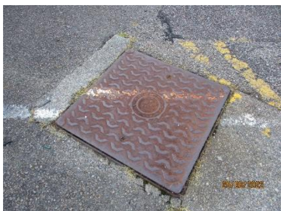
259. Raised drainage cover
