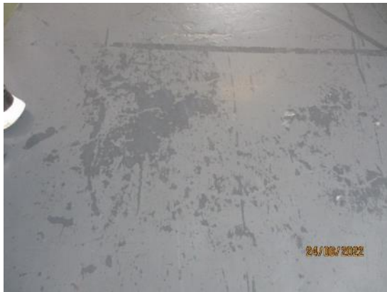
86. Painted concrete floor – 1 st floor corridor
