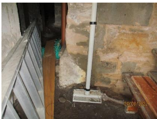
73. Temporary support bearing on the floor
