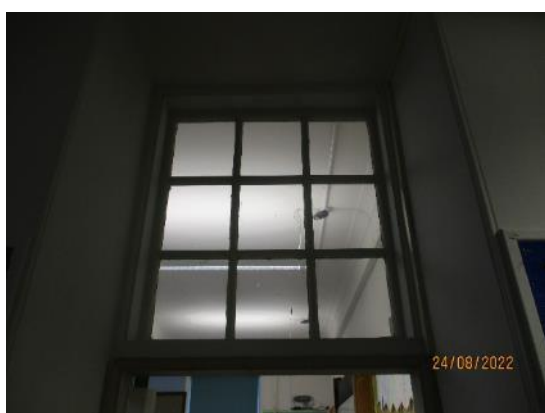
143. Borrowed lights above classroom doors
