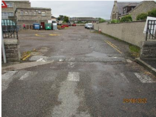
232. Tarmacadam access road
