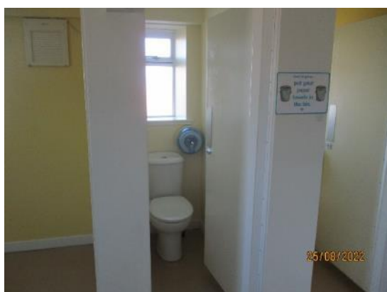
139. Timber doors to toilet cubicles
