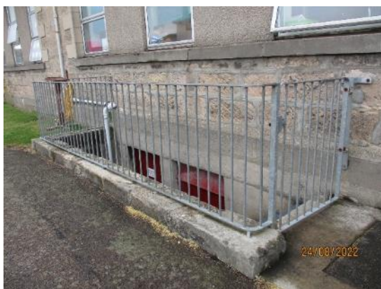
248. Galvanised fence to Boiler House
