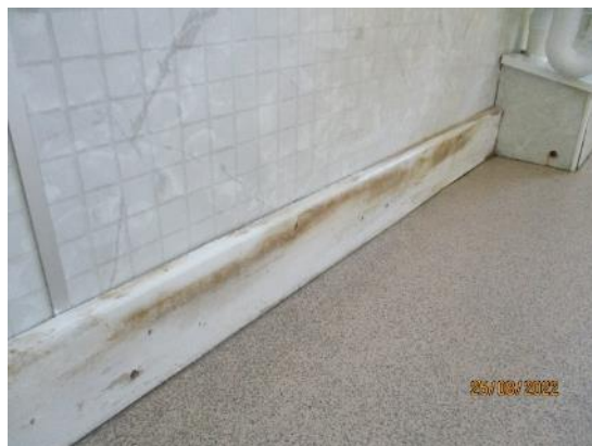
179. Timber skirting boards
