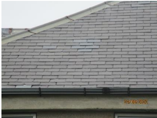
15. UPVC ogee gutters
