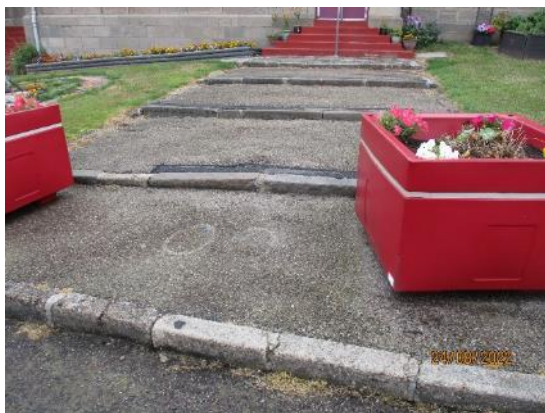
60. Steps to front entrance
