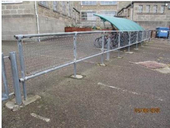
240. Tubular rail and mesh fencing
