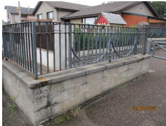
245. Metal railings above block walls
