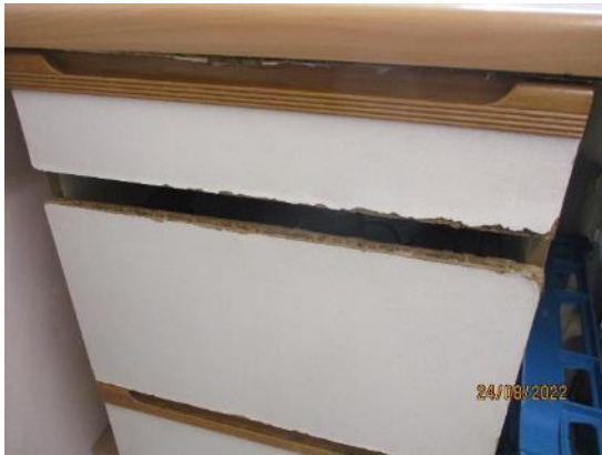
165. Damaged base units
