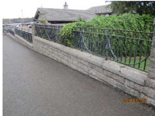
253. Block walls to playground
