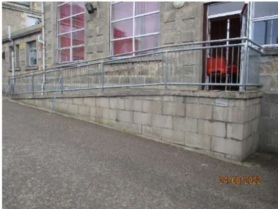
64. Fire escape ramps
