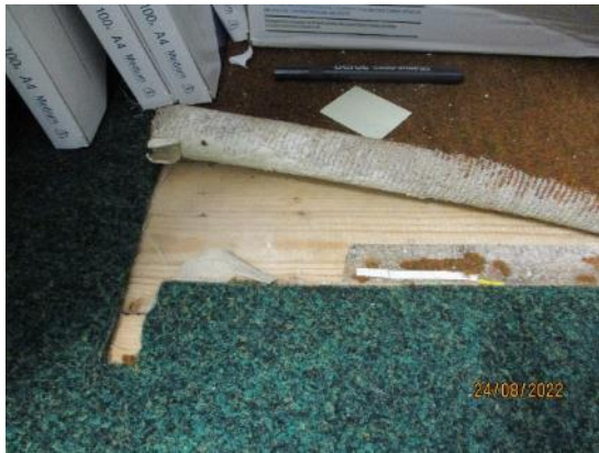
74. Suspended timber floor
