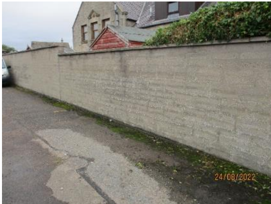
252. Blockwork wall to north
