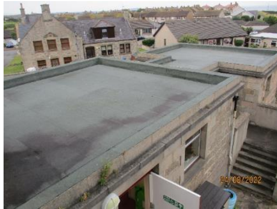
8. Felt covered flat roofs
