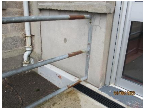
71. Surface corrosion
