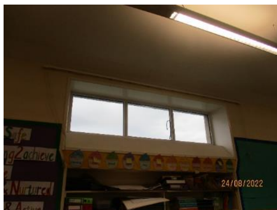
44. High level windows on 1 st floor
