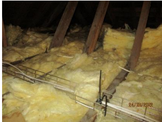
14. Mineral fibre insulation to main school
