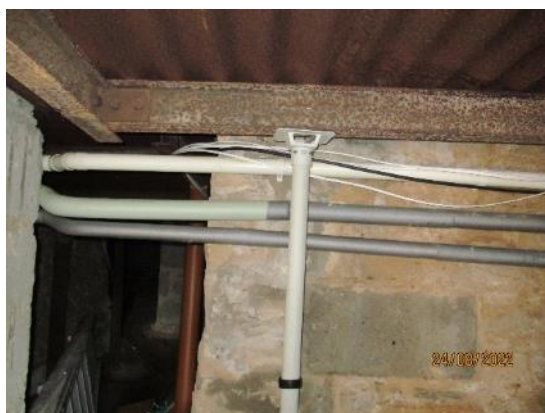
72. Cellar steel frame with temporary support
