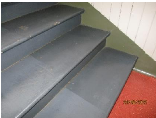
91. Painted concrete treads
