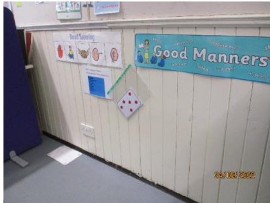
118. Timber lining boards to walls
