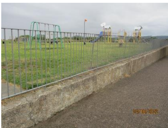
254. Rendered block walls to sports field
