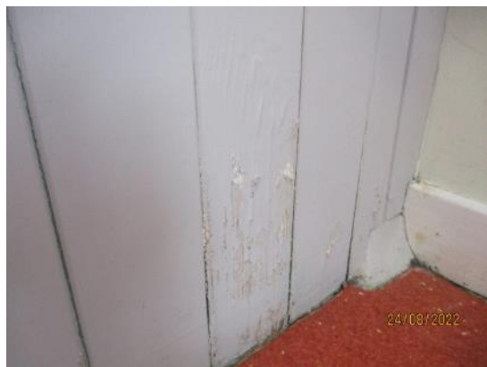
173. Timber lining boards
