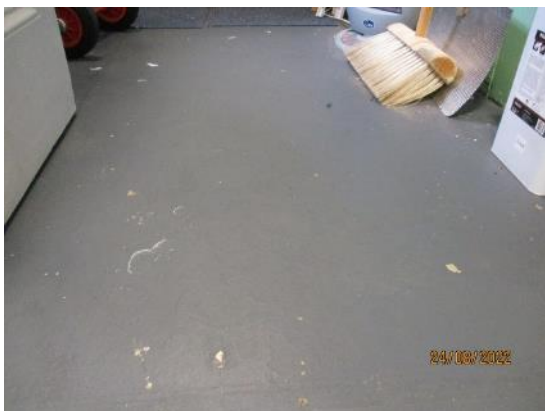
84. Painted concrete floor
