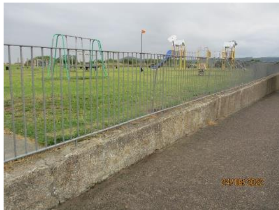
247. Galvanised railings above blockwork walls
