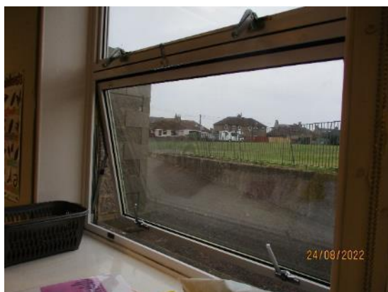
43. Aluminium windows internally
