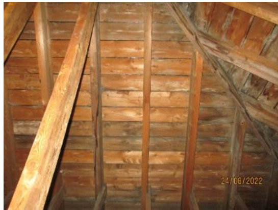
2. Timber sarking boards
