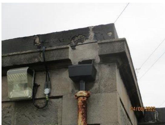
23. Replacement upvc hopper heads
