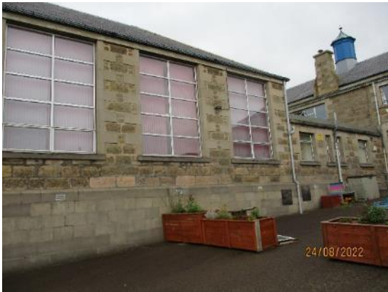
39. Large aluminium framed windows
