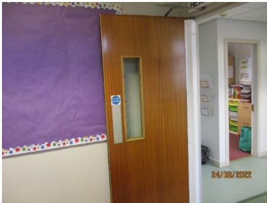
133. Timber doors to offices, stores etc
