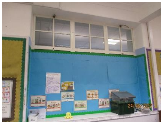
126. Timber borrow lights – Classroom/corridor
