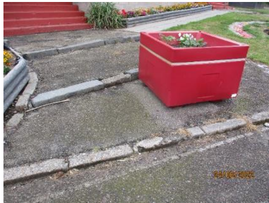
93. External concrete kerb steps
