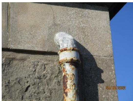
24. Lead outlet to cast iron downpipes
