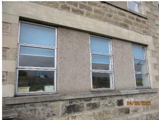
32. Roughcast panels between windows (south)
