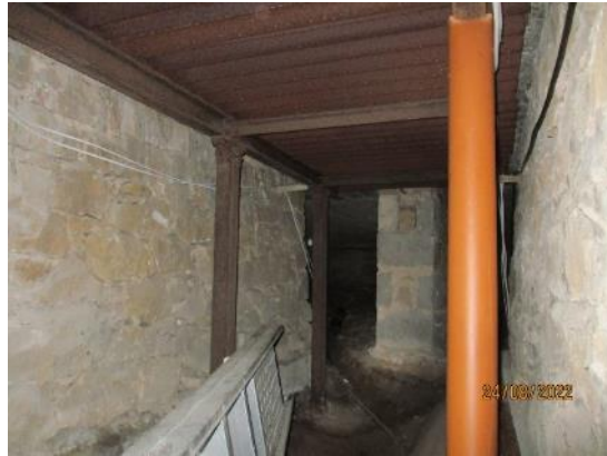
110. Cellar blockwork walls
