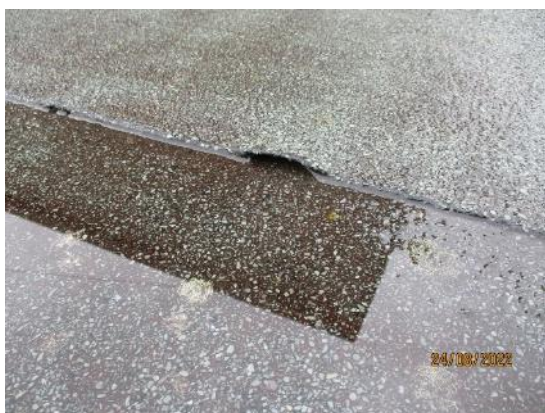
12. Open felt joints
