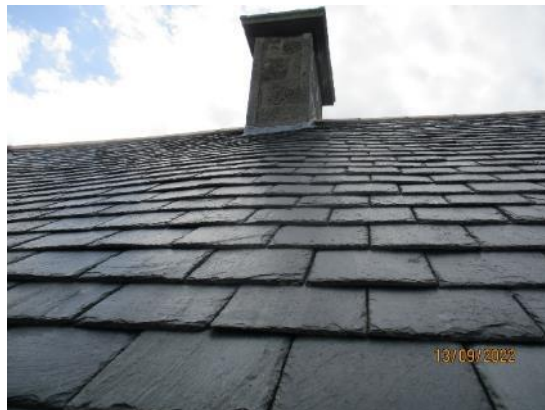
10. Raised roof surface
