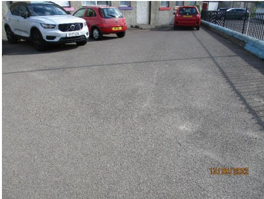
252. Tarmacadam car park
