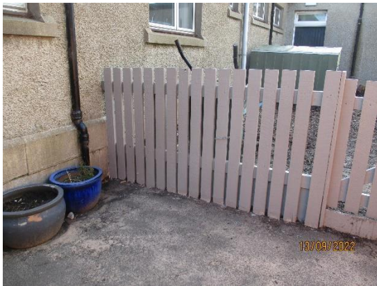
264. Timber fence to playground
