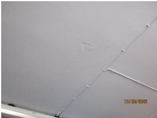
126. Repairs to plaster ceilings
