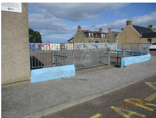
262. Galvanised railings to playground
