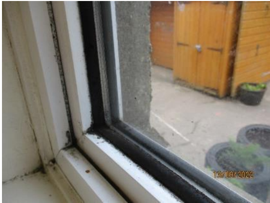
79. Double glazing to aluminium windows
