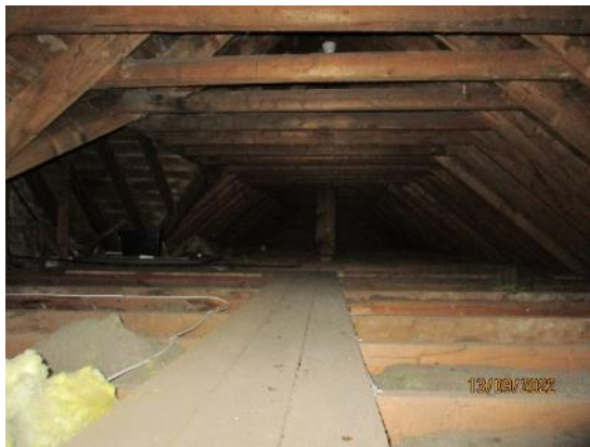
3. Roof structure, south pitch
