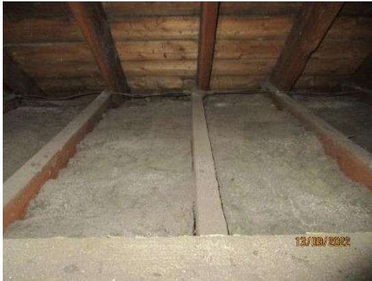
31. Insulation above Dining Hall
