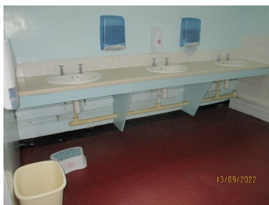
182. Vanity basin worktop (Boys Toilet)
