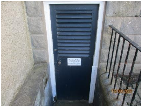
67. Timber louvre door to Boiler House
