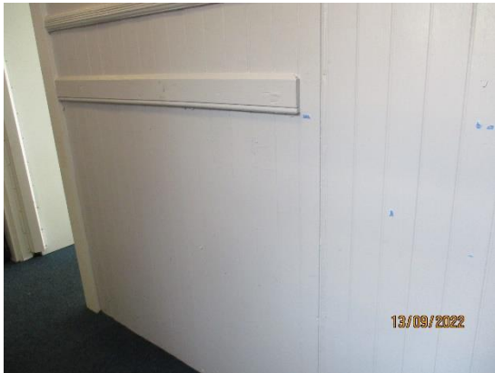
140. Timber linings to dado level
