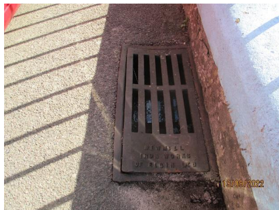
281. Car park road gully
