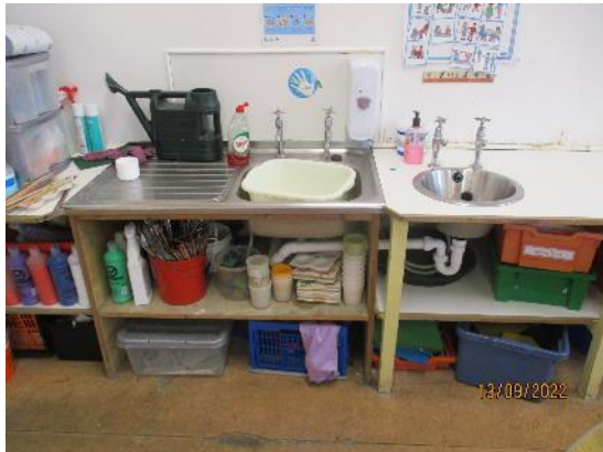
201. Worktop only, no base units
