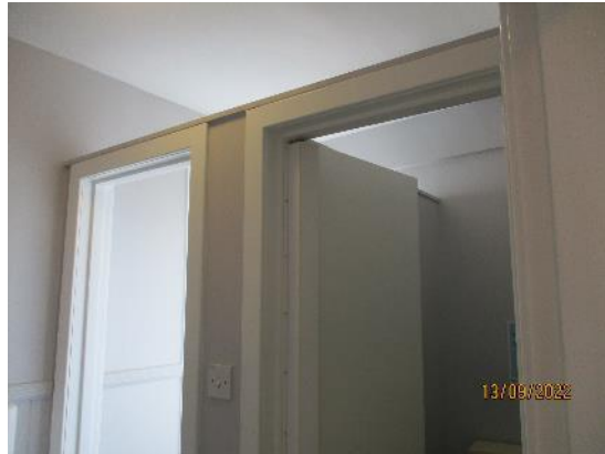
158. Toilet cubicle timber doors
