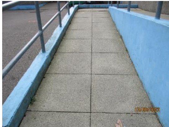
94. Paving slab ramp
