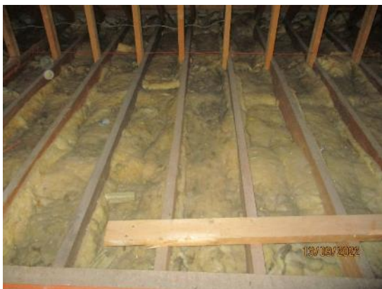
29. Insulation to south pitched roof
