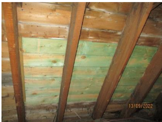
5. Replacement sarking boards
