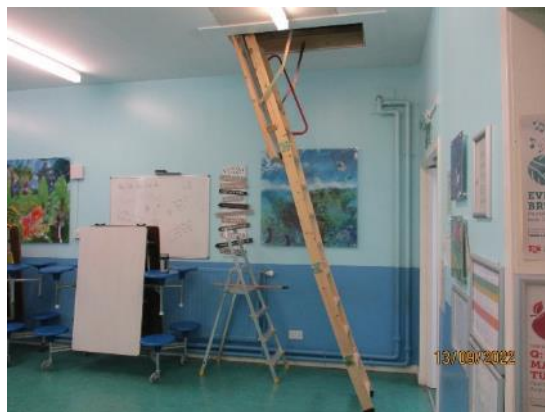
6. Roof space access above Dining Room
