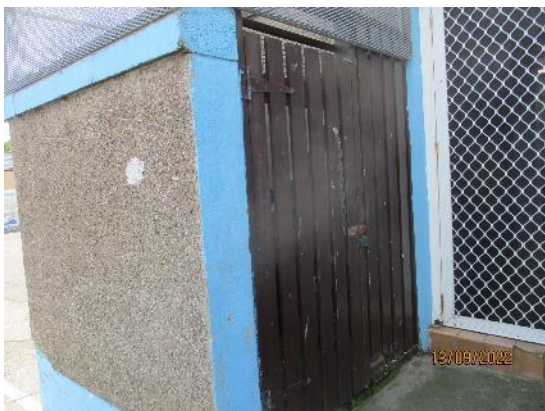
286. Bin store enclosure
