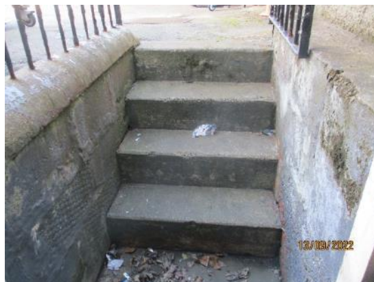
90. Steps to Boiler House
