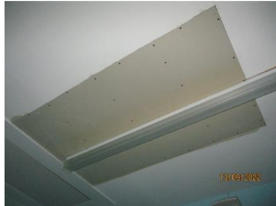
121. Plasterboard repairs
