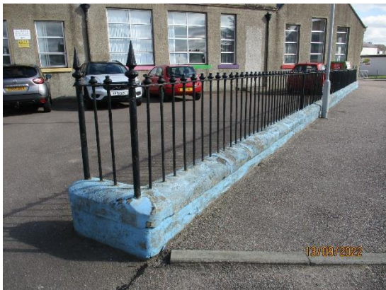
260. Metal railings to car park
