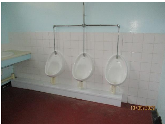
142. Ceramic wall tiles – Boys toilet
