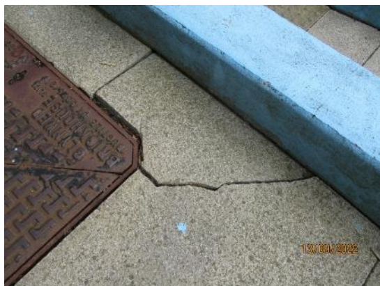
95. Damaged slabs
