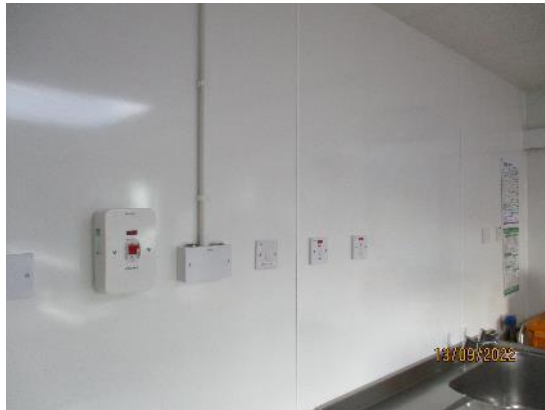
141. Wetwall to the Kitchen
