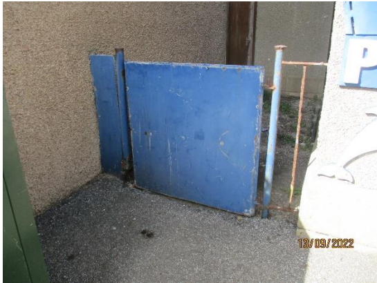
270. Metal gate from car park
