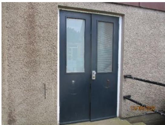
59. Timber doors to Nursery
