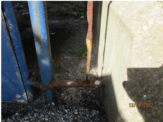
272. Extensive corrosion
