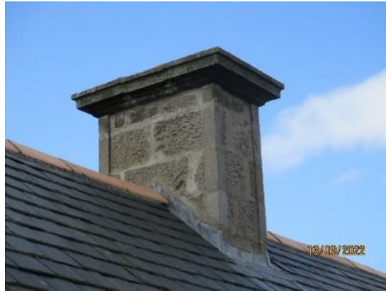
44. Redundant stone chimneys
