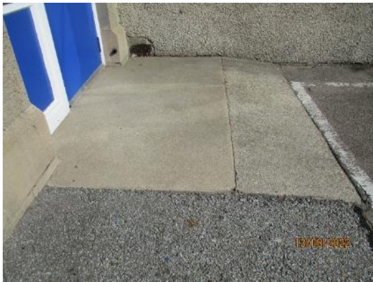
91. Concrete ramp to front entrance
