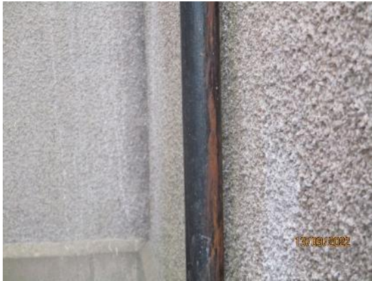
85. Cast iron rainwater goods
