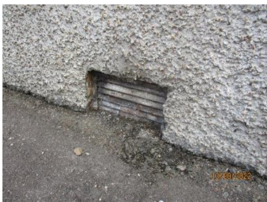
53. Some underfloor vents at ground level
