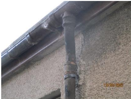
37. Cast iron downpipes
