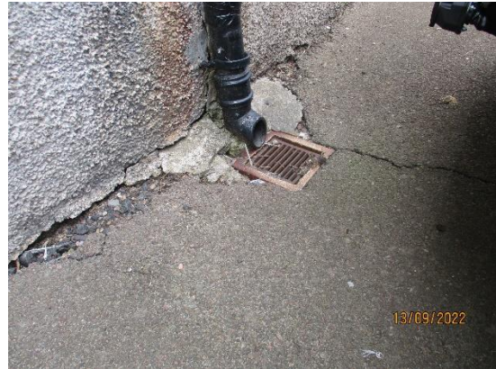
253. Surface cracking
