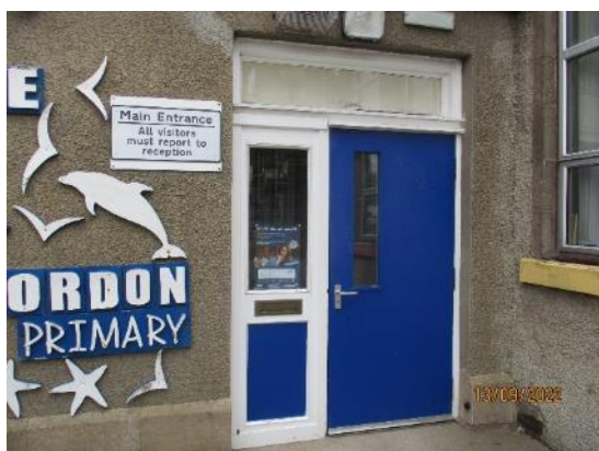
63. Timber front entrance door
