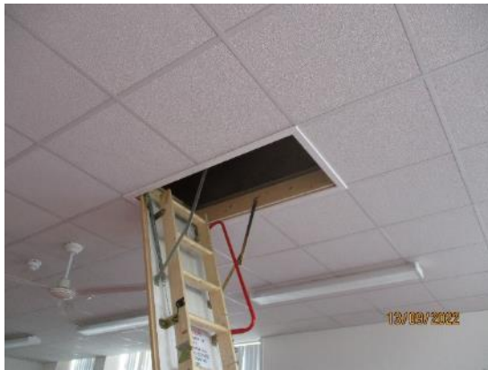
1. Roof space access above P1, 2 & 3
