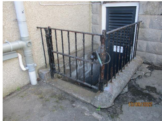
265. Boiler House metal railings
