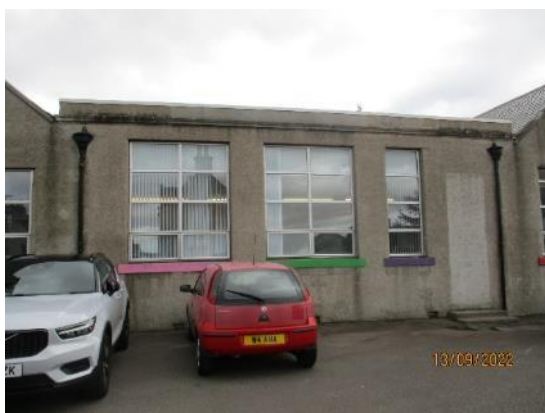
54. Roughcast external walls
