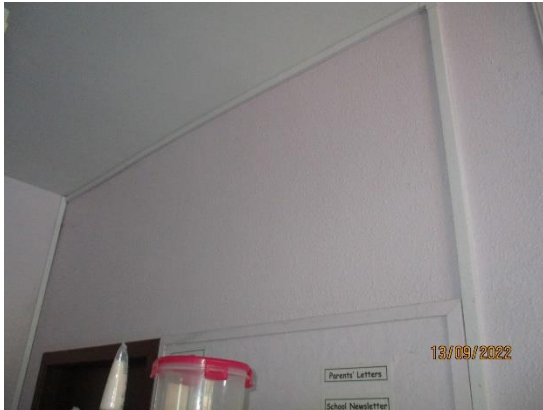
132. Plastered walls with wallpaper
