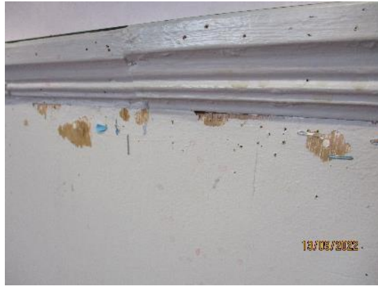
139. Plywood wall linings
