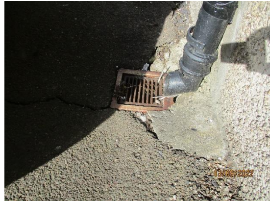
283. Surface water gullies at downpipes
