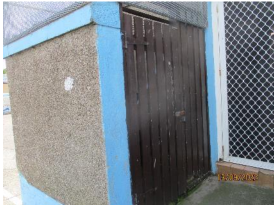
273. Timber gates to bin store
