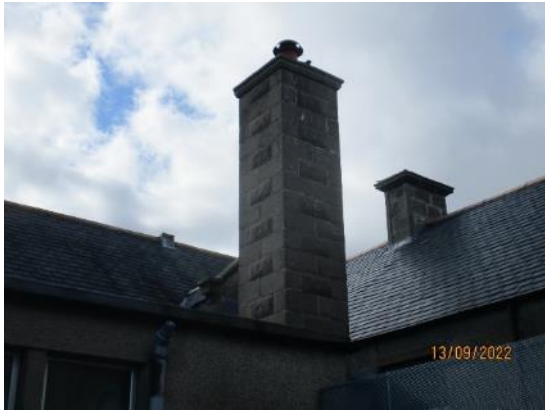
43. Boiler House chimney
