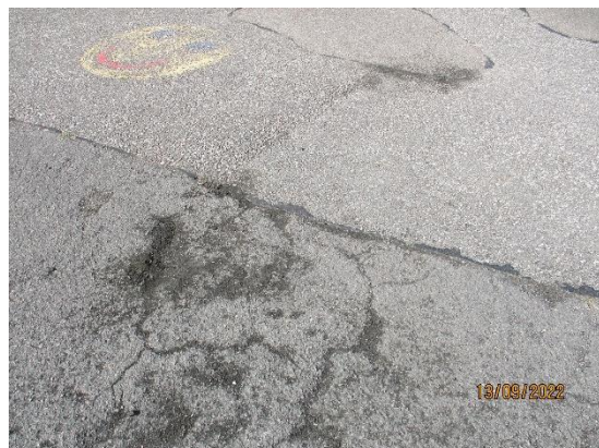
257. Surface cracking
