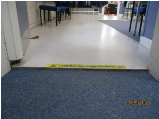
99. Sloping timber floors
