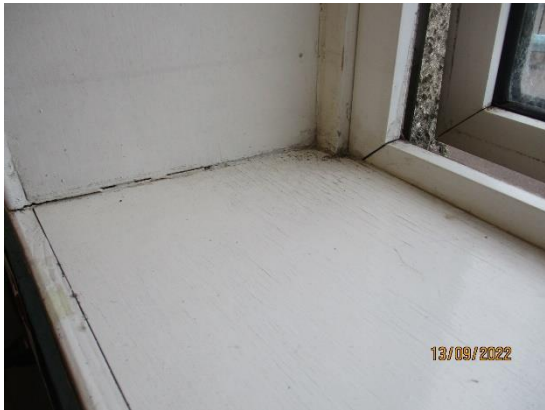
146. Timber window sills and surrounds
