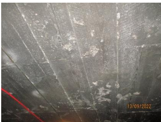
130. Concrete ceilings – Boiler House
