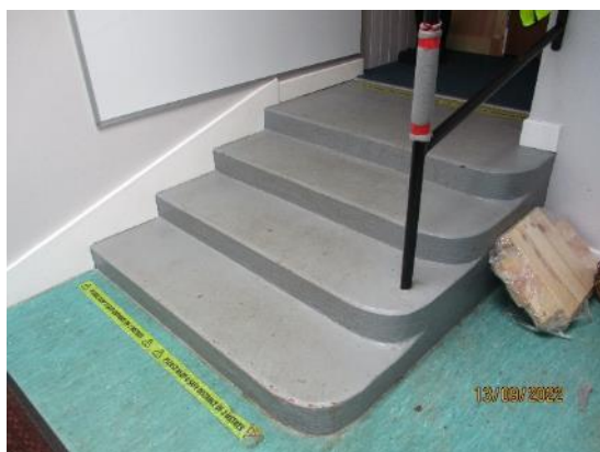
115. Concrete steps - Nursery
