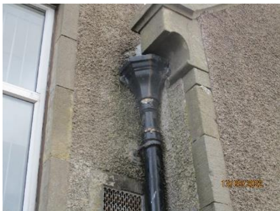
36. Cast iron hopper heads and downpipes
