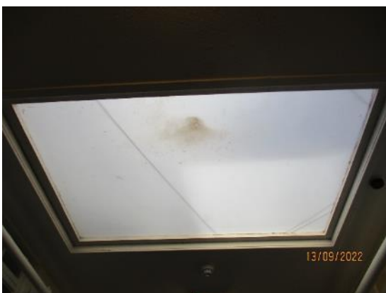
131. Borrowed lights – Central corridor
