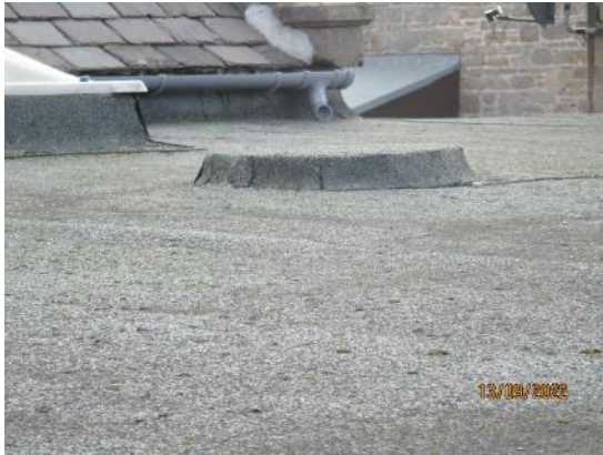
25. Vent cap above staff toilet
