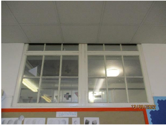
144. Timber framed borrowed lights
