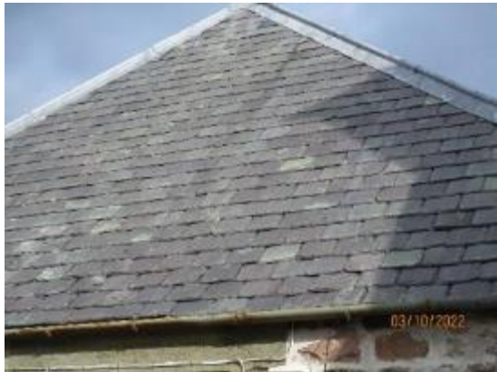
10. Slated roof to main school
