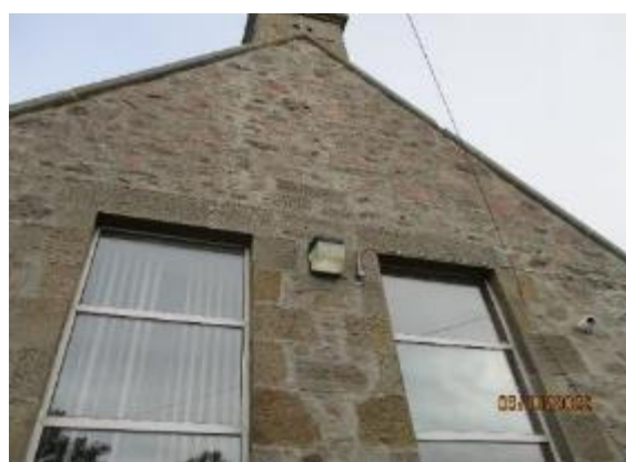
210. External lighting typical.
