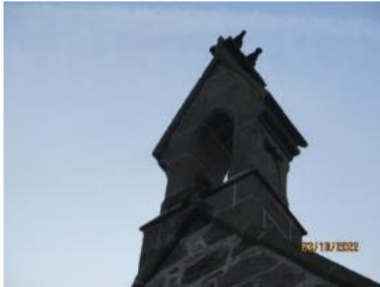
44. Stone bell tower to school
