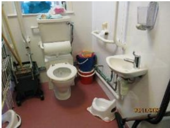
152. Accessible toilet in the Nursery
