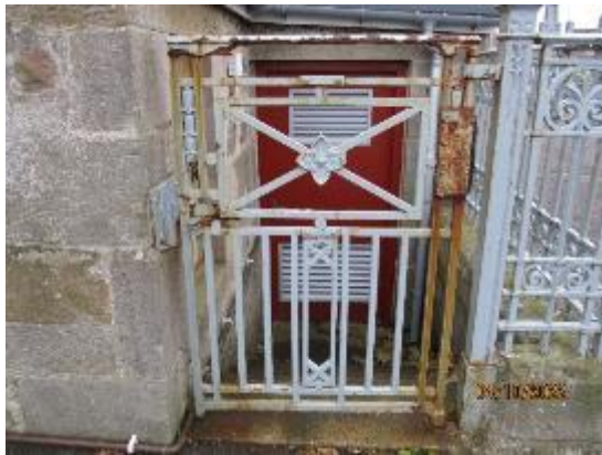
260. Metal gate to Boiler House
