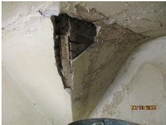
102. Lath & plaster ceilings
