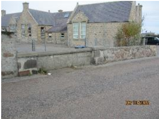
268. Stone wall to south boundary
