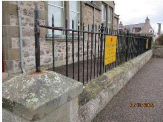
249. Metal railings to east boundary
