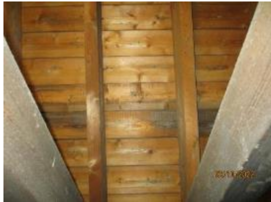
4. Timber sarking boards
