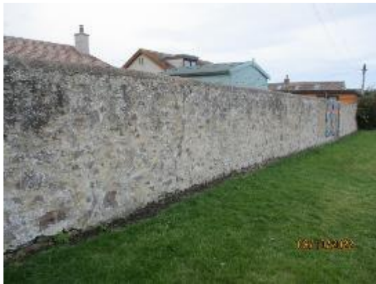
272. Stone wall to sports field
