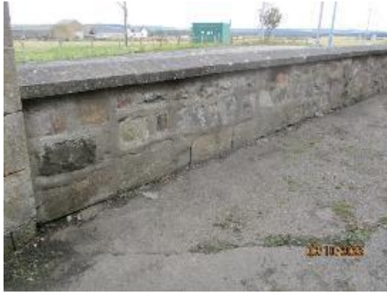
267. Stone wall to south east boundary
