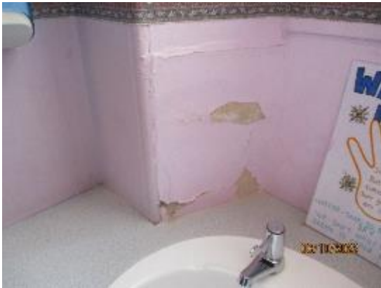
166. Lath & plaster walls
