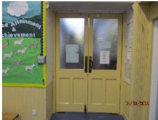
126. Timber panelled double doors
