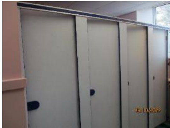
153. Composite cubicle partitions
