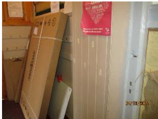
116. Timber linings to walls in the Nursery
