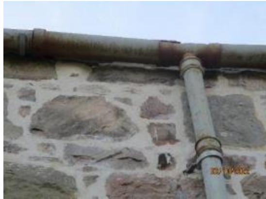
32. Cast iron downpipes
