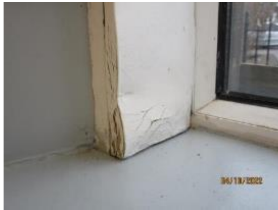
120. Laminated MDF window linings
