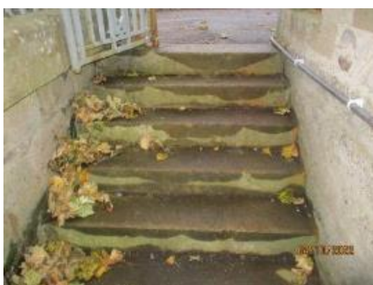
77. Concrete steps to Boiler House
