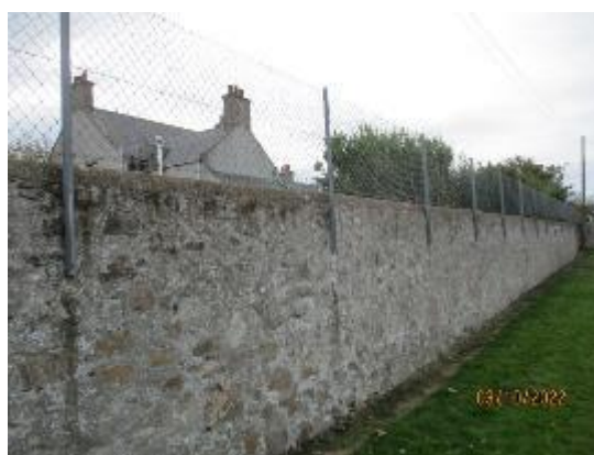
255. Chain link fence above wall to sports field
