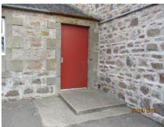
54. Timber rear fire exit door
