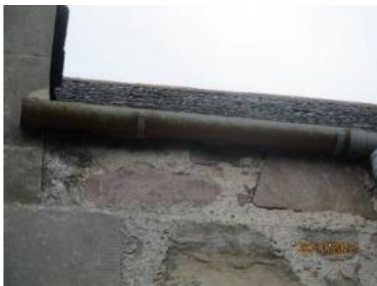
71. Cast iron rainwater goods
