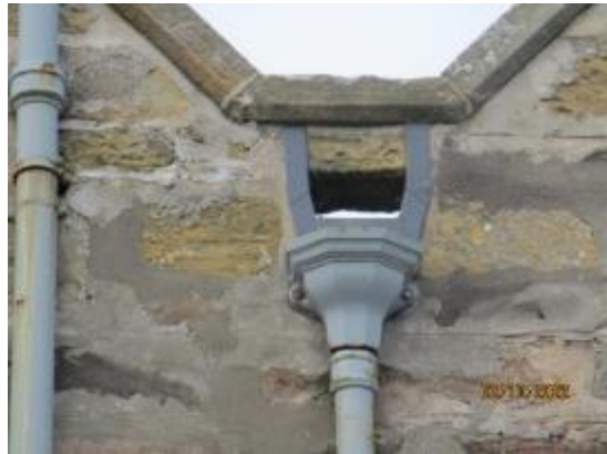
34. Cast iron hopper heads to valley drainage
