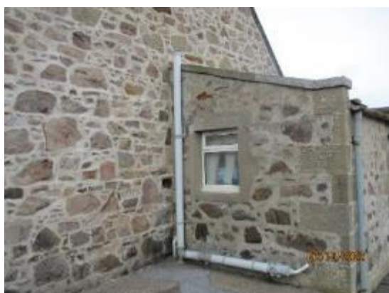
39. UPVC soil vent pipes to Nursery
