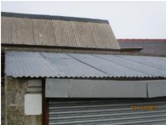
15. Corrugated iron to Nursery external stores
