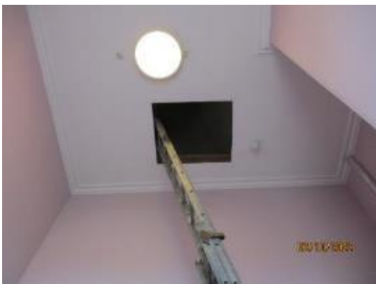
5. Roof access above staff toilets
