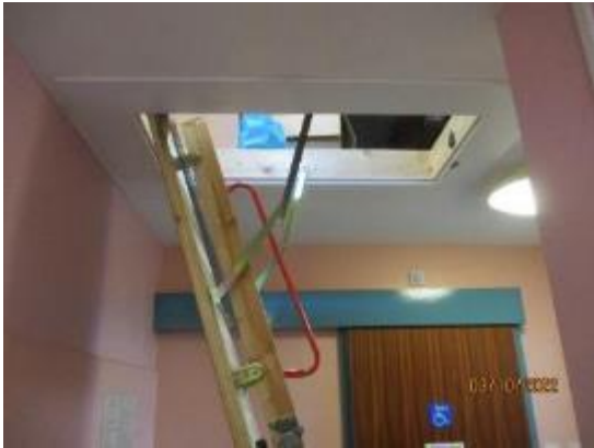
1. Roof access above toilets
