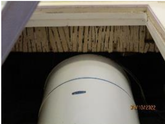
104. Lath & plaster ceilings to Nursery
