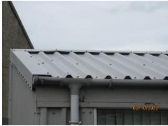
14. Metal profile to Nursery extension
