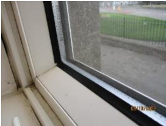
67. Double glazing to all windows
