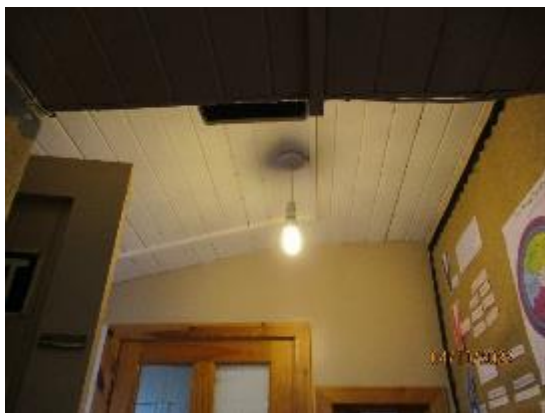
106. Timber linings to ceilings
