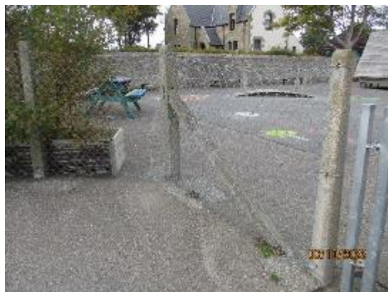
253. Concrete post and chain link fencing
