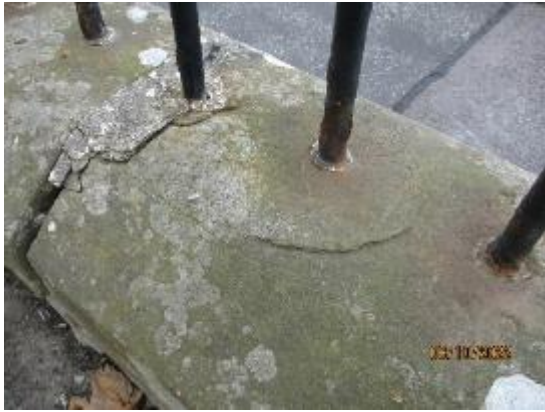
266. Concrete coping stones
