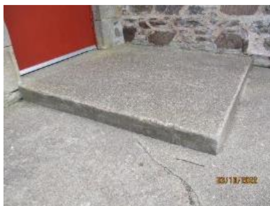
75. Concrete step to back door
