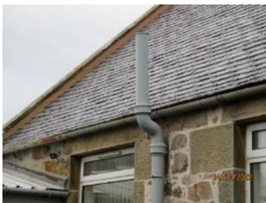
38. Cast iron soil vent pipes to Nursery
