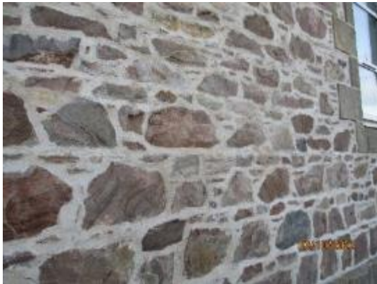
45. Natural stone external walls
