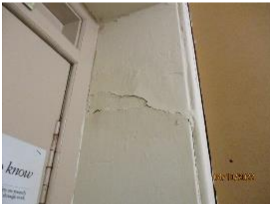
115. Lath & plaster in the Nursery
