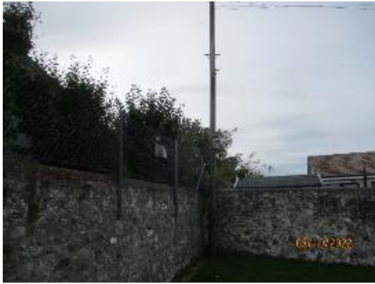
284. Utility pole in corner of sports field
