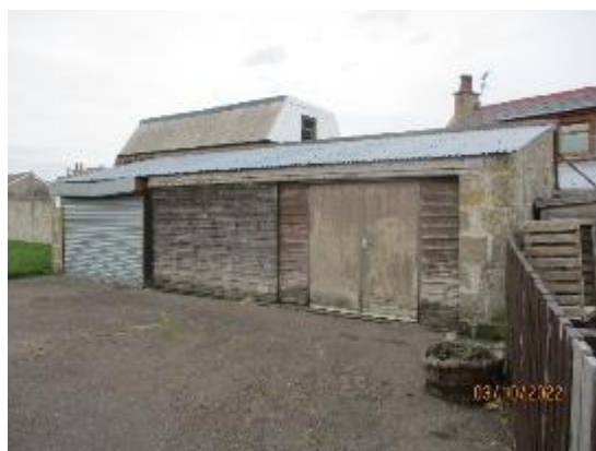
283. Nursery external stores
