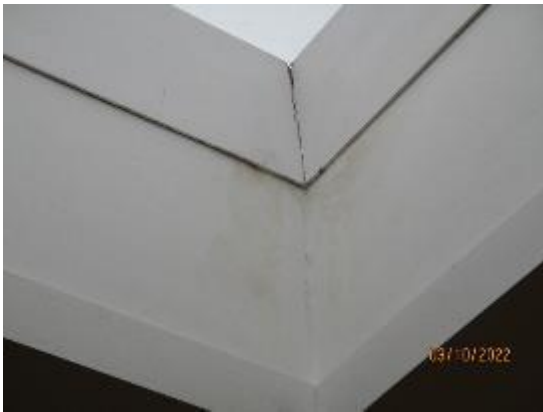
164. Watermarked rooflight linings
