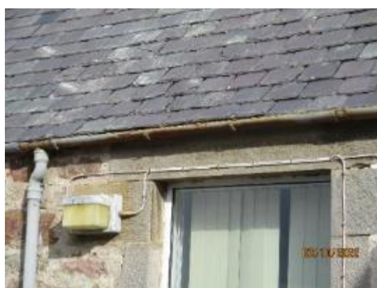
24. Cast iron gutters to school
