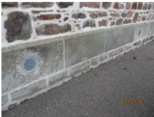
48. Ground level and sub-floor ventilation
