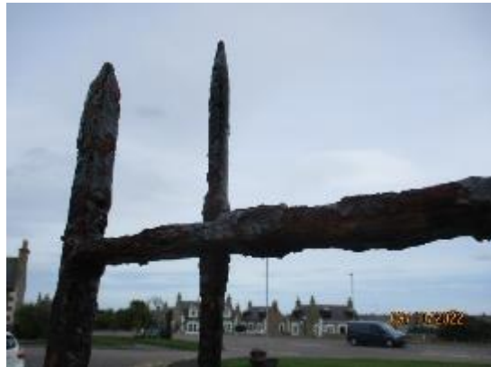
251. Railing corrosion
