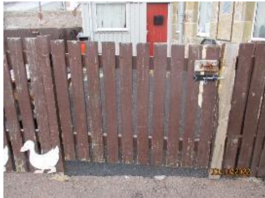
263. Timber gate to Nursery playground
