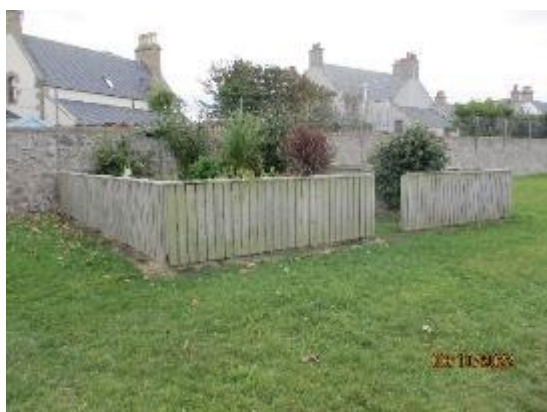
256. Timber fence to school garden
