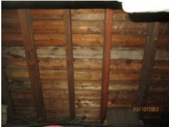
7. Timber sarking boards
