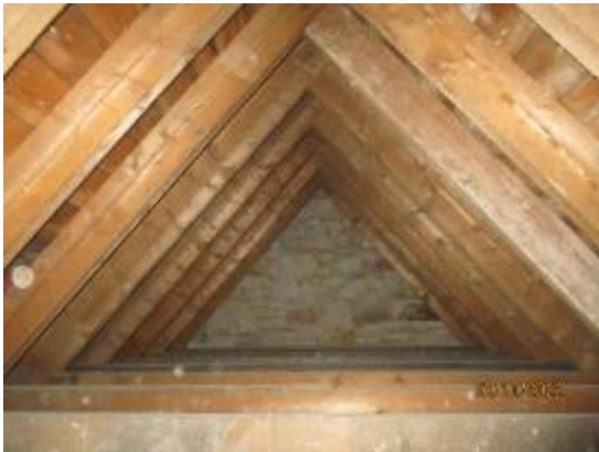
3. Timber roof trusses
