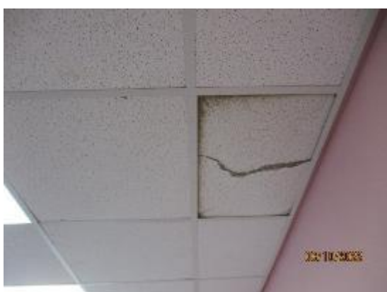
94. Suspended ceiling tiles
