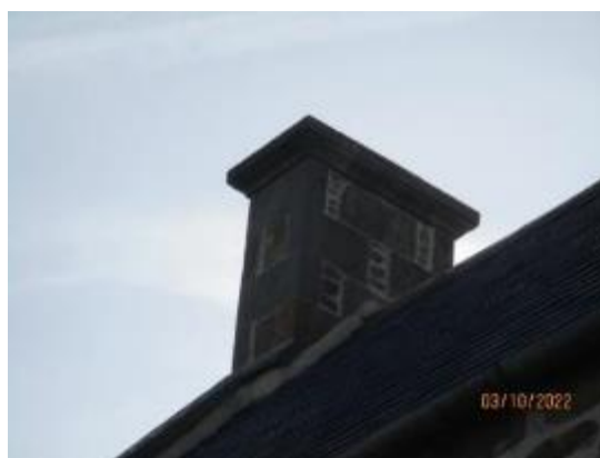
40. Stone chimneys to school
