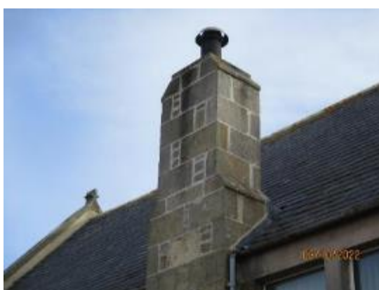
42. Stone chimney to Boiler House
