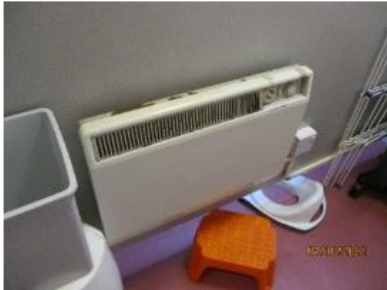
225. Electric convactor heater. Disabled WC.1/B3
