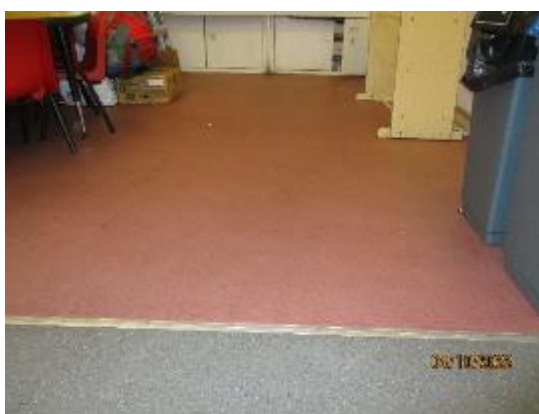
91. Sheet vinyl floors in the Nursery
