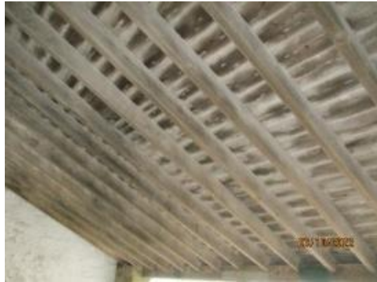
8. External store roof structure
