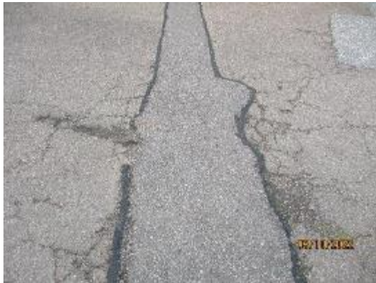
245. Patch repairs to playground surface
