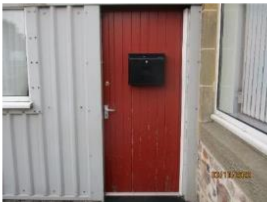
70. Timber external doors
