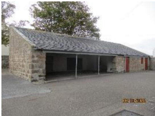
281. External shelter and stores
