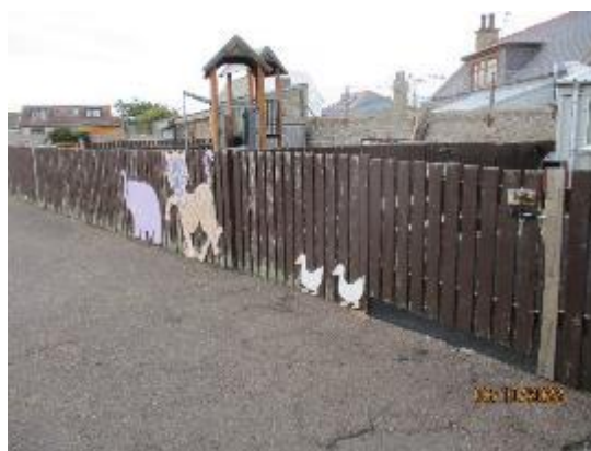
257. Timber fence to Nursery playground
