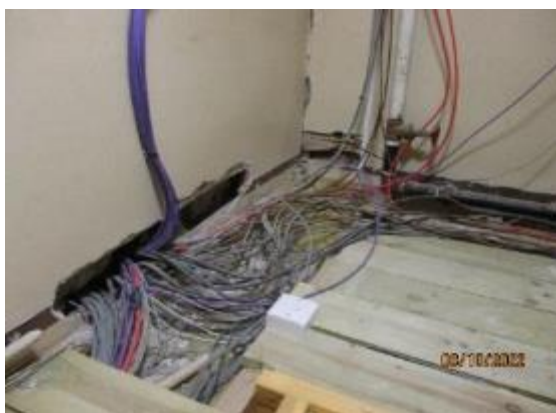
198. General wiring. Void above staff room.
