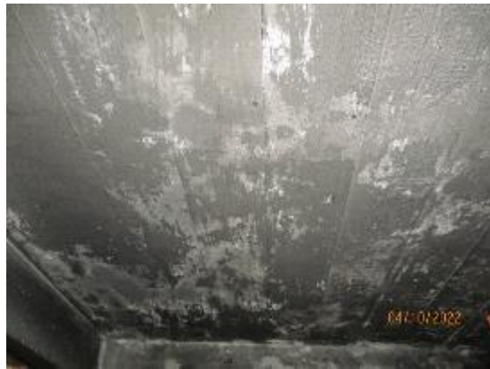
103. Concrete ceiling to Boiler House
