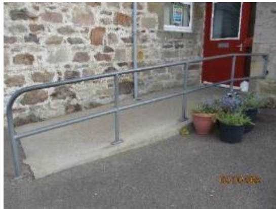
79. Galvanised handrail to ramp
