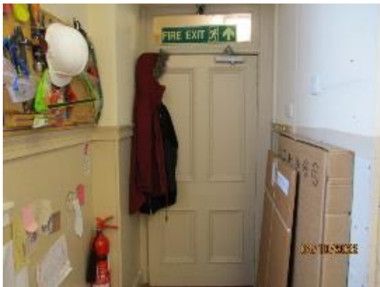
127. Timber panelled doors in the Nursery
