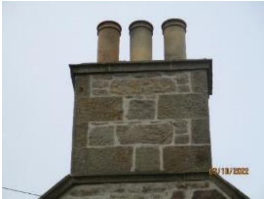
43. Stone chimney to Nursery
