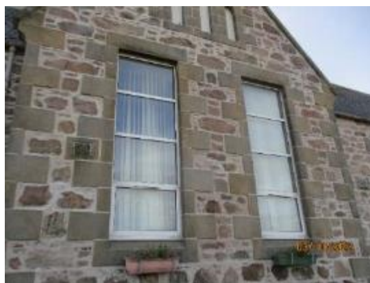
60. UPVC windows to school
