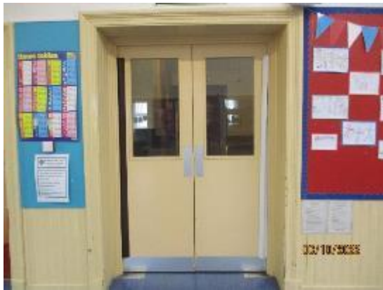
125. Timber double doors
