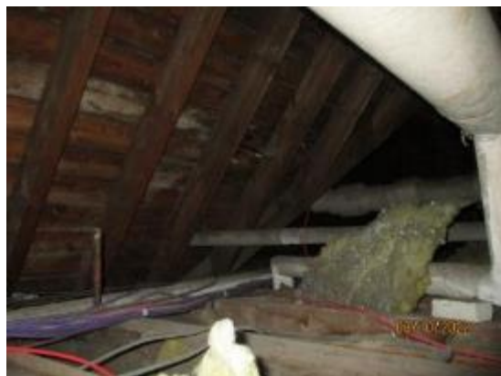
6. Timber roof trusses
