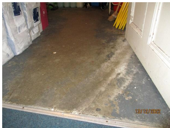
78. Painted concrete floor
