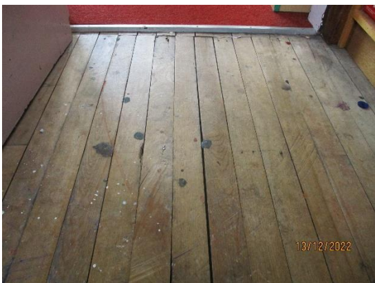
77. Timber boarded floors
