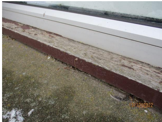
56. Timber window sills
