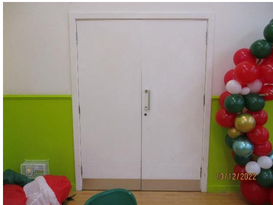
120. Timber flush, double doors
