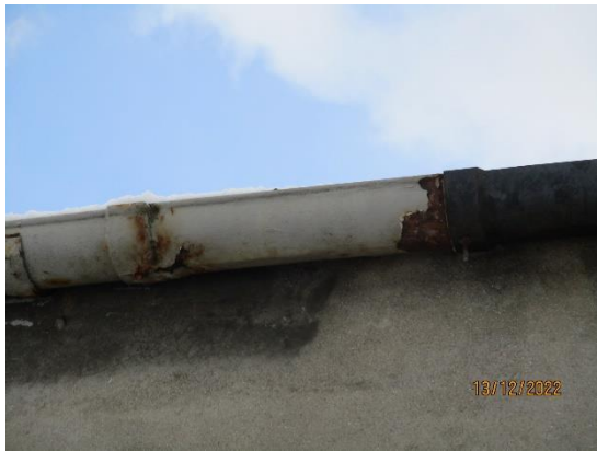
55. Cast iron rain water goods
