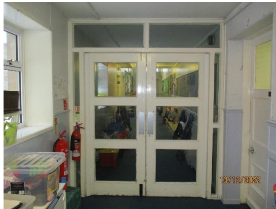
121. Timber doors and glazed screens
