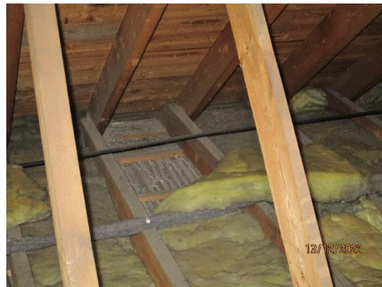
16. Disturbed insulation
