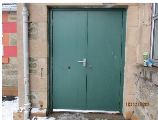
36. Solid core timber doors
