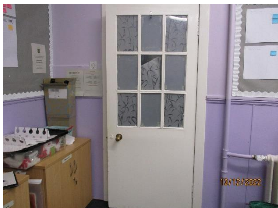
110. Timber panelled classroom doors
