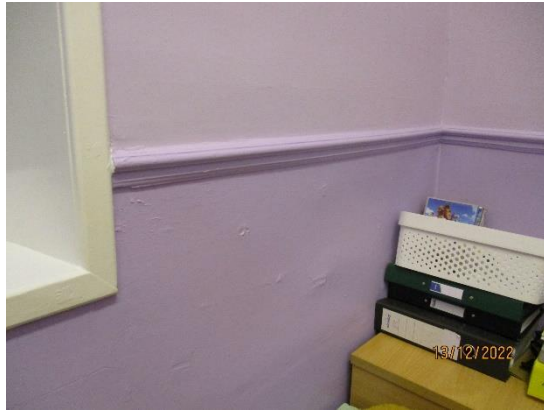
97. Spalling plaster
