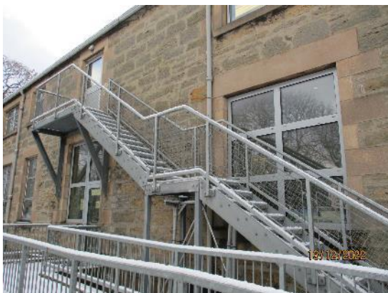
219. Galvanised fire escape
