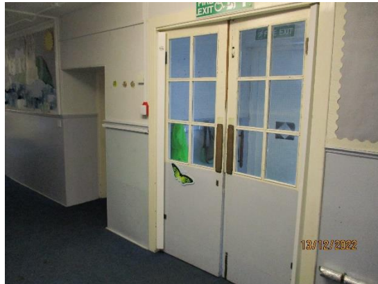
117. Double timber panelled doors
