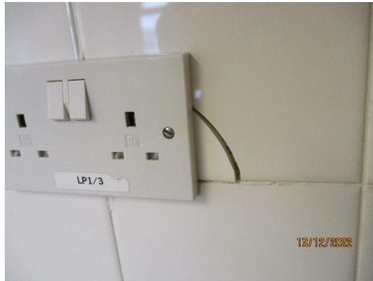
105. Damaged ceramic tiles
