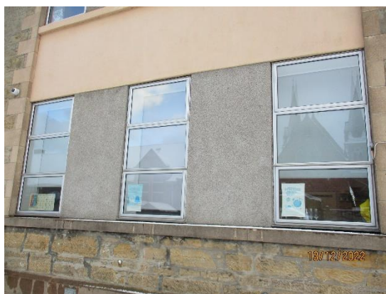
35. Roughcast panels between windows
