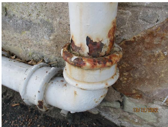
23. Downpipe corrosion
