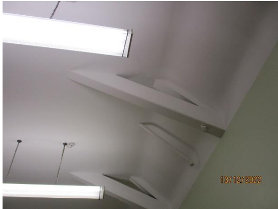
85. Lath & plaster ceilings
