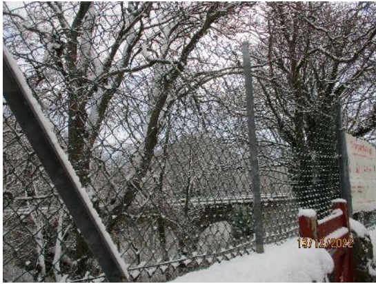
221. Chain link fence above wall
