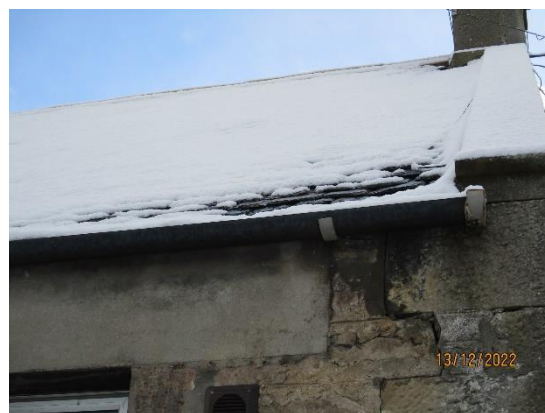
18. Cast iron gutters
