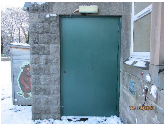
41. Timber solid core fire escape door
