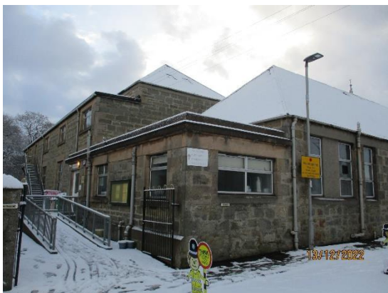
11. Flat roofs east
