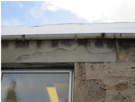
31. Previous repairs to concrete lintols
