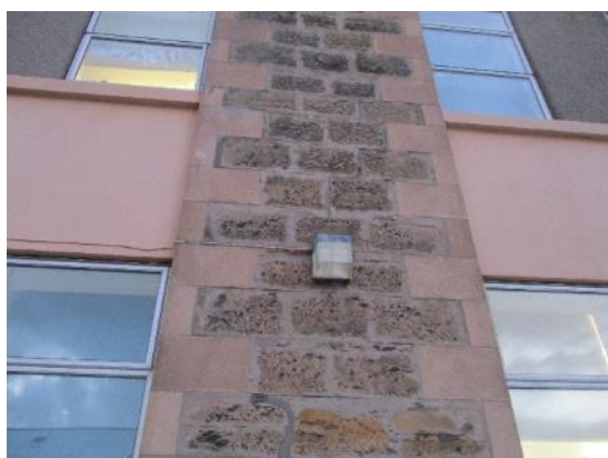
199. External lighting typical.
