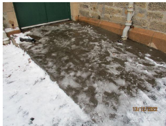
60. Concrete ramps to playground
