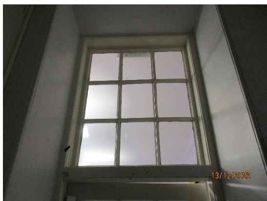
108. Timber framed borrowed lights
