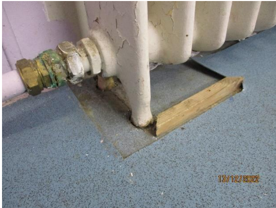
67. Vinyl flooring cut around radiators
