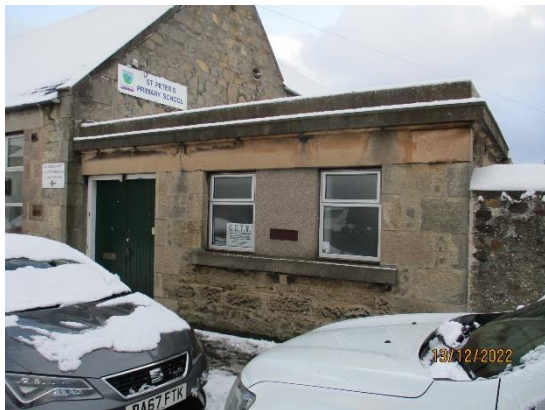
10. Flat roof west
