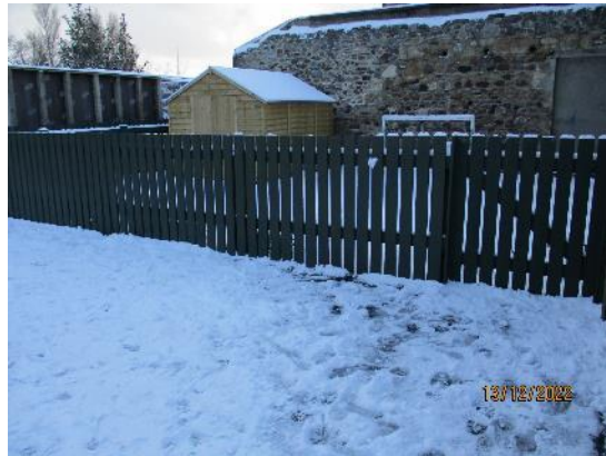
224. Timber boarded fence
