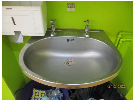
135. Stainless steel wash hand basin
