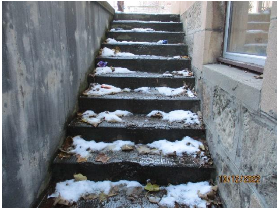
61. Steps to Boiler House
