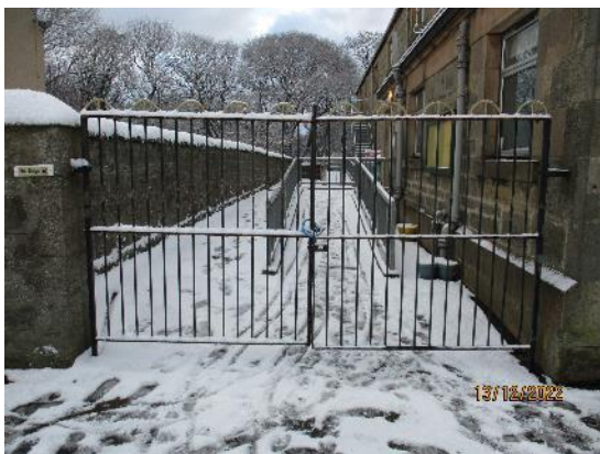
225. Metal entrance gates
