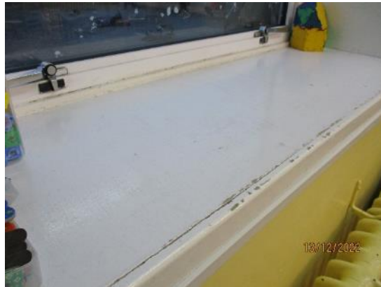
152. Timber window sills
