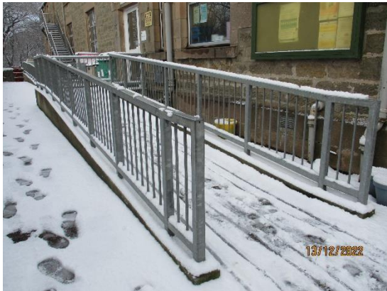
63. Galvanised guardrail
