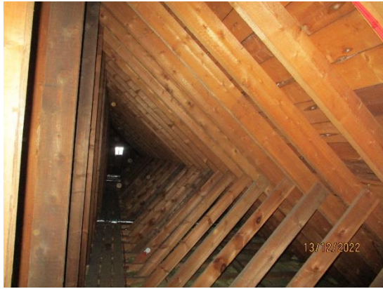
1. Timber roof trusses
