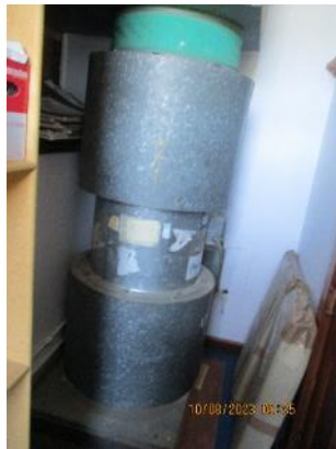
310. Kitchen cooking extract fan and ductwork 2/45b.
