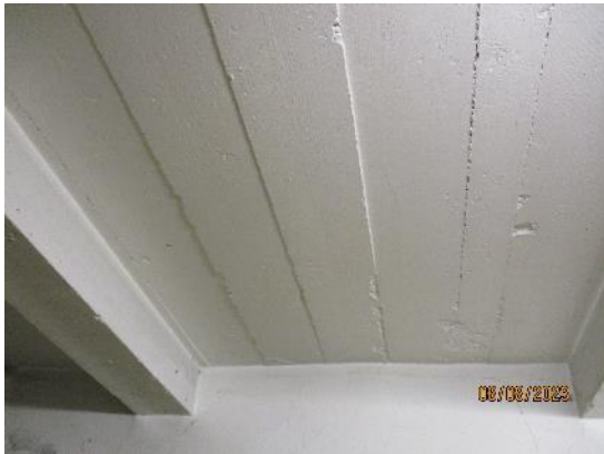
182. Concrete ceiling to Boiler Room
