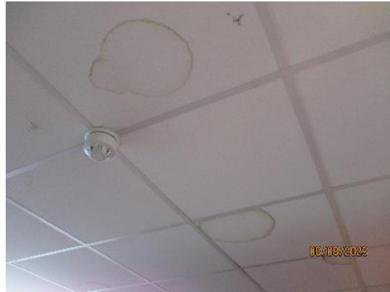
169. Suspended ceiling tiles in Classrooms
