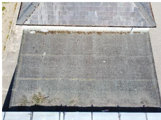
30. Mineral felt flat roof
