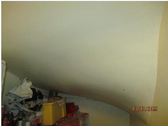
165. Plaster soffits to timber stairs
