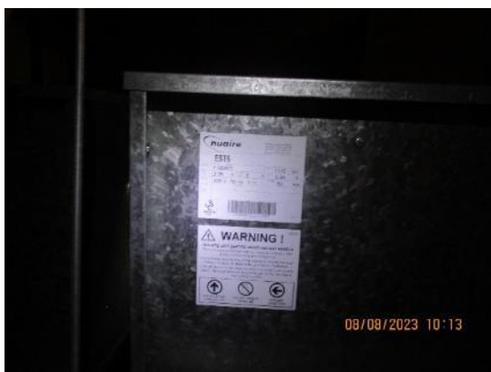
306. Centralised ventilation system (1) unit 2008 extension attic space.
