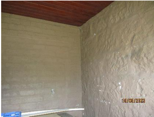
191. Brick and stone to external stores
