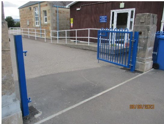
392. Tubular rail vehicle gate
