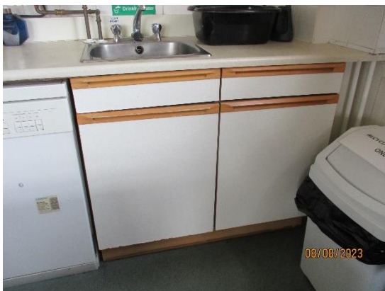
266. Worn sink base units
