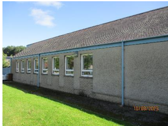
68. Brickwork external walls
