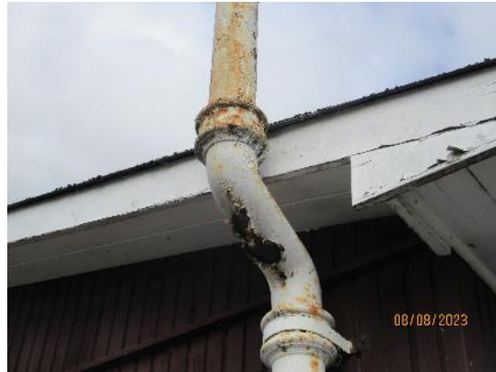
134. Cast iron soil vent pipes
