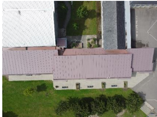
22. Single ply membrane to 2007 extension
