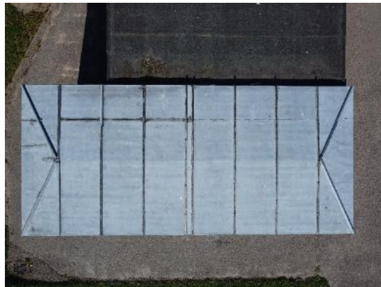
32. Zinc roof to external stores
