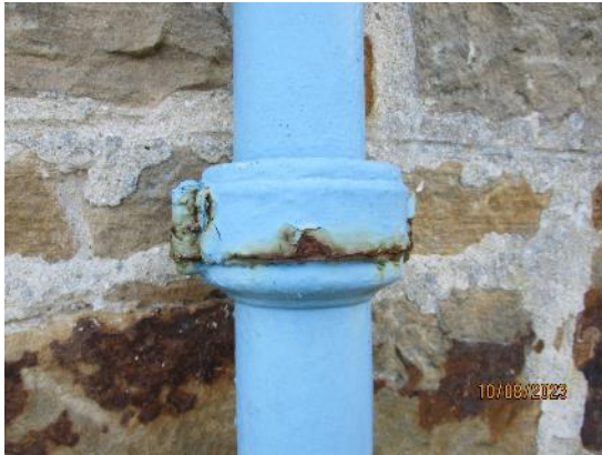
133. Cast iron rainwater goods
