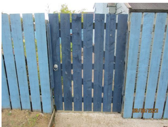
390. Timber boarded gates 1.50m
