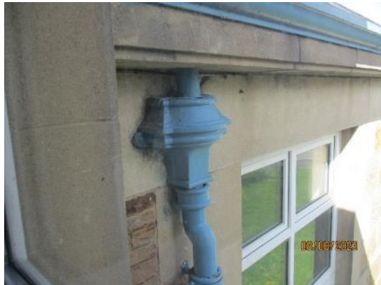
58. Cast iron downpipes
