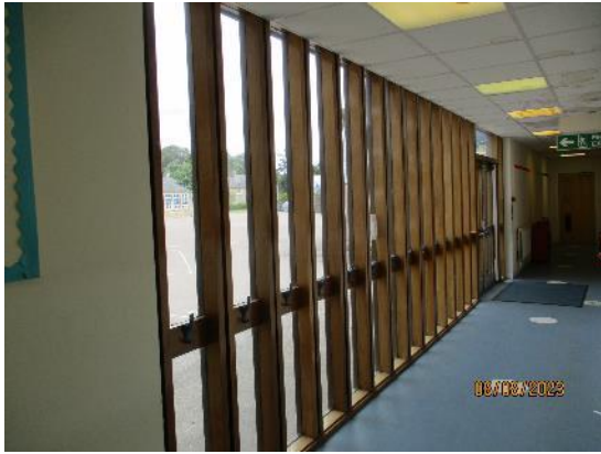
97. Timber screen internally
