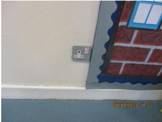
326. Socket – 2008 extension corridor 1/71.
