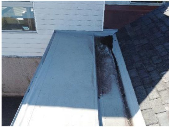
19. Single ply membrane to 1975 extension
