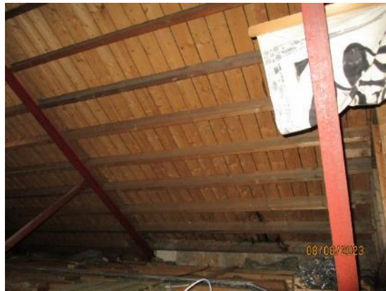
2. Vertical timber sarking boards.
