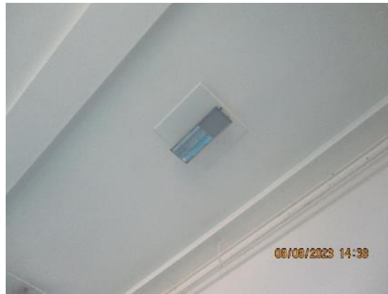
333. Lighting – original school hall.
