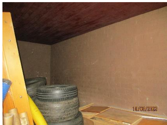
190. Brickwork to external stores
