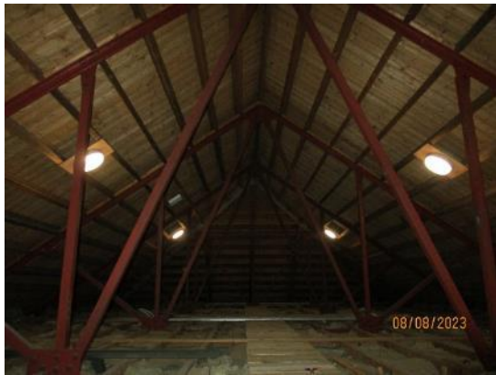
1. Original school, steel framed roof.
