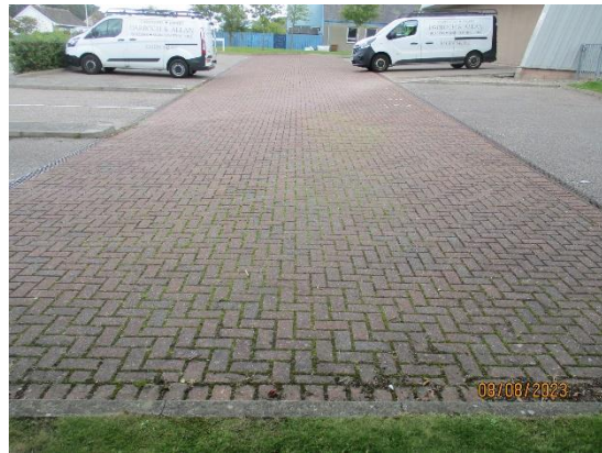
363. Brick pavior car park
