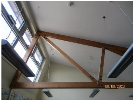
10. Exposed roof trusses
