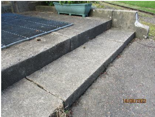
141. Pointing and levelling to concrete steps
