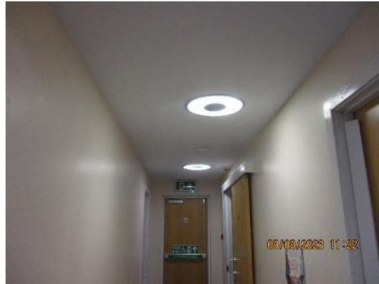
339. Lighting – 2008 extension corridor.
