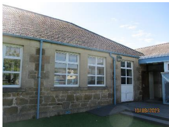
144. Composite ramp and decking
