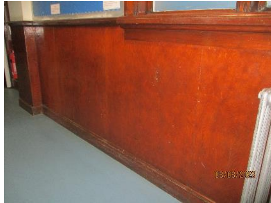
192. Plywood linings at low level
