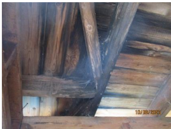
12. External stores timber roof structure
