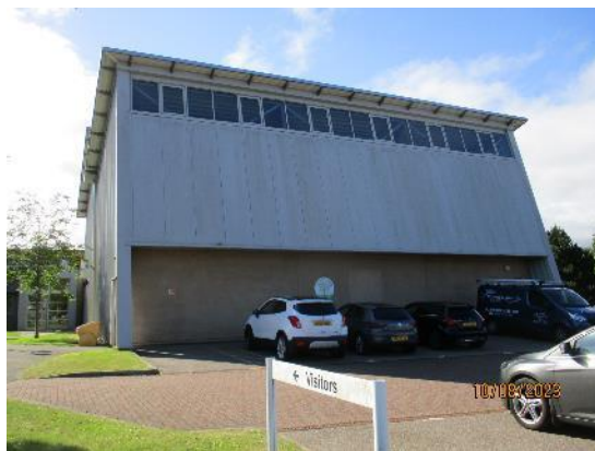
78. Metal profile walls to Games Hall
