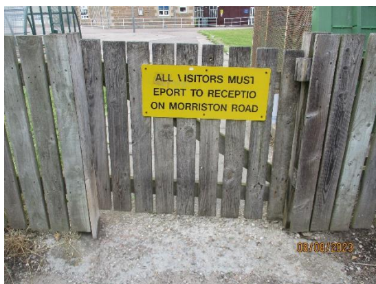
391. Timber boarded gates 0.90m
