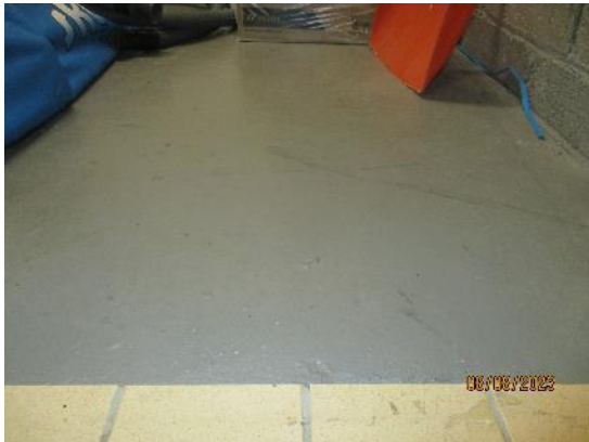
159. Painted concrete floors
