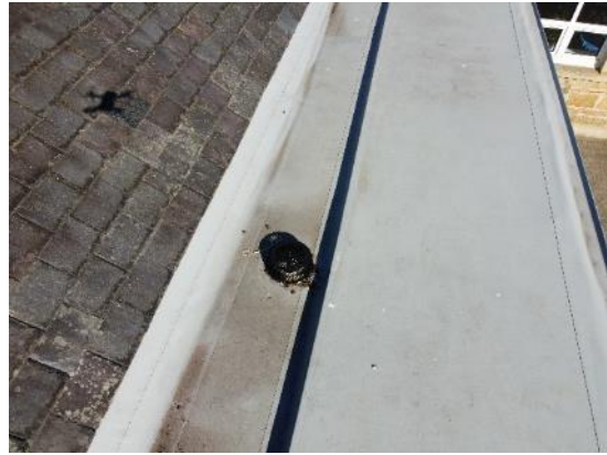
20. Box gutter and internal downpipe
