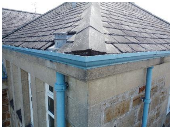
48. Cast iron ogee gutters
