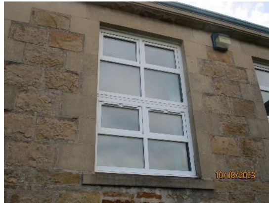
112. Large UPVC windows
