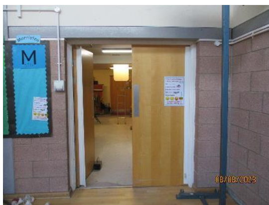
212. Timber double veneered doors
