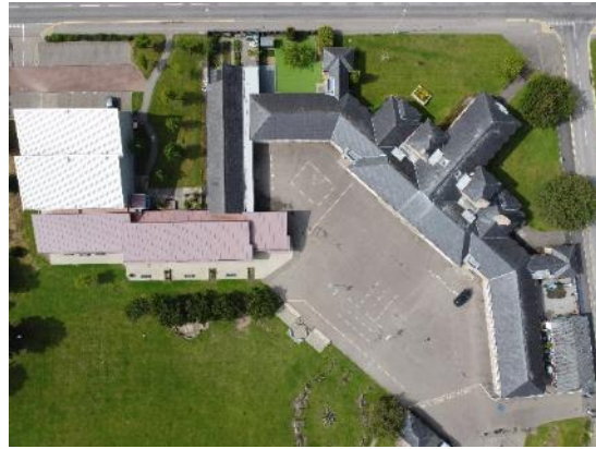
14. School roofs overview
