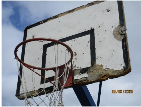
417. Backboards in poor condition
