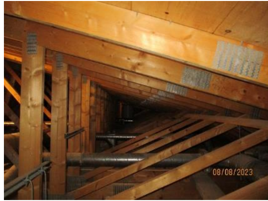
8. 2007 extension timber roof structure
