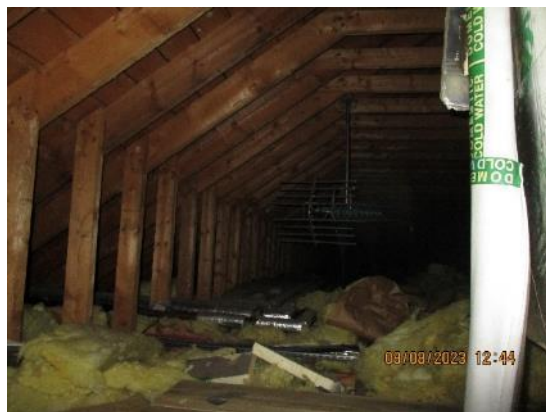
6. 1975 extension roof structure.
