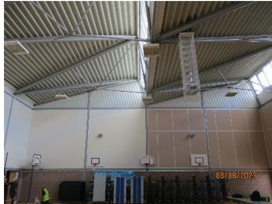
181. Metal profile sheets to Games Hall ceiling
