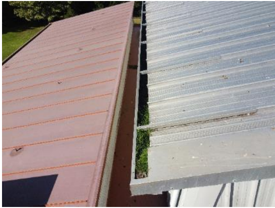
55. Aluminium box gutters
