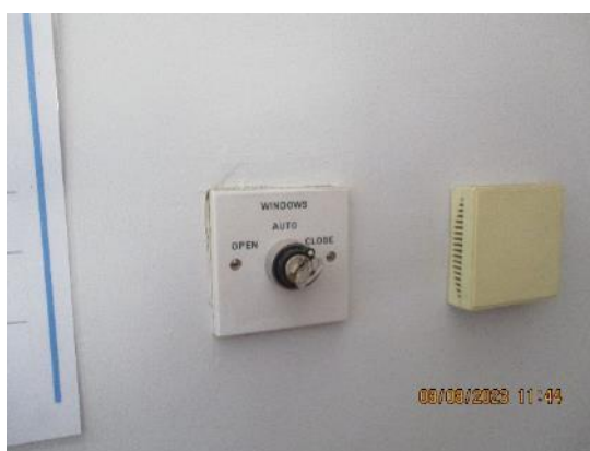
361. Electric window control – 2008 extension classes.
