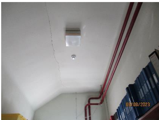
178. Lath & plaster ceilings
