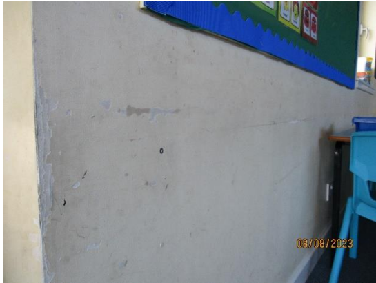
257. Painted plasterboard walls
