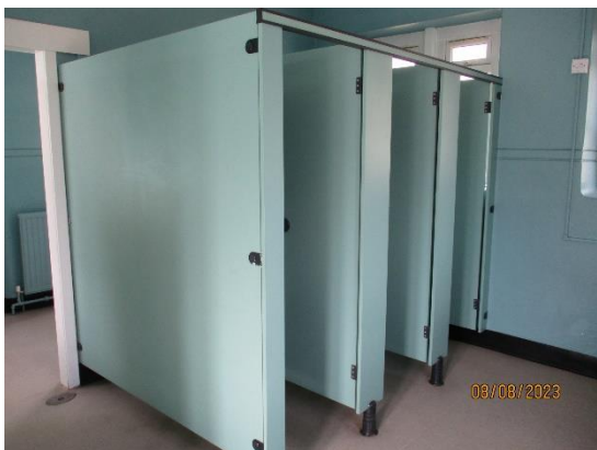
237. Composite panel toilet cubicles
