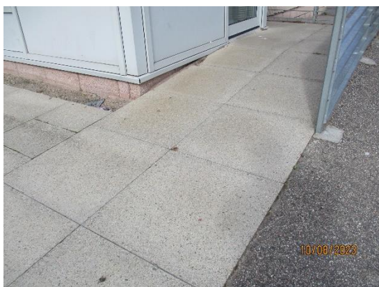
372. Paving slab footpaths
