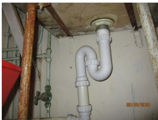
252. UPVC waste pipes to cleaners sinks
