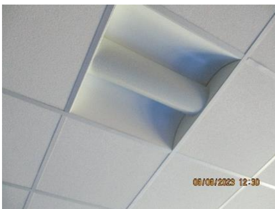
336. Lighting – 1970s extension classroom.
