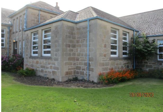
67. Stone external walls
