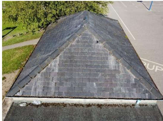
28. External store slated roof
