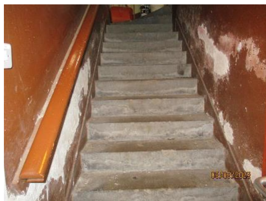
162. Concrete stairs to basement
