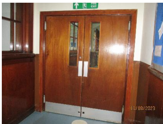
210. Timber solid core doors
