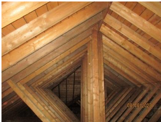
3. Timber framed roof structure
