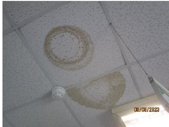
171. Watermarked suspended ceiling tiles
