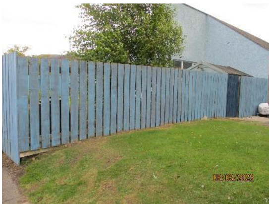
137. Timber fencing and gates
