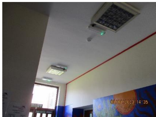
331. Lighting – original school corridor.
