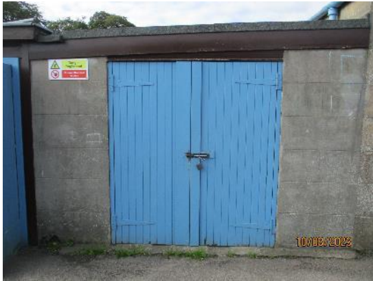
91. Timber double doors to external stores
