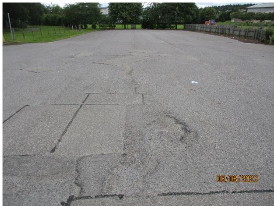
364. Tarmac staff car park
