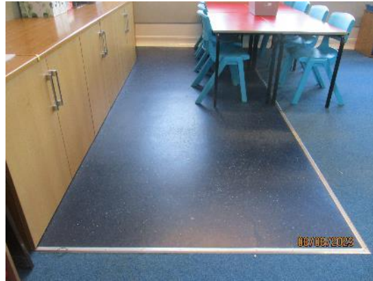
152. Sheet vinyl to sink areas
