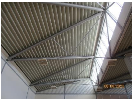
11. Games Hall steel framed roof structure
