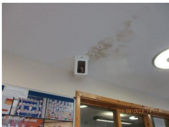
356. CCTV camera – main reception 1/71.
