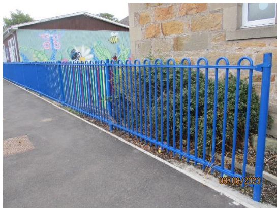
382. Tubular rail fence to Nursery
