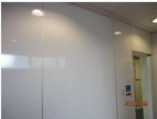
195. Wetwall in Toilets
