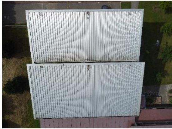
26. Metal profile roof above Games Hall
