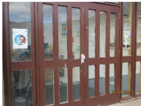
96. Screen with timber double door
