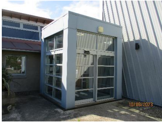
98. Electric automatic powder coated door
