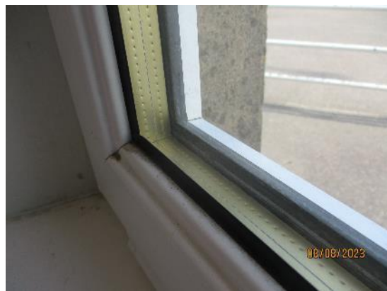
126. Double glazing to original school building
