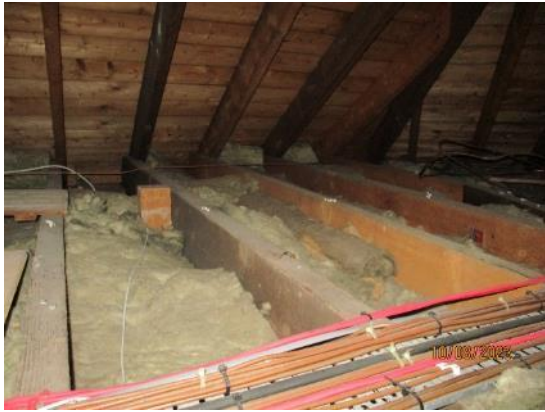
43. Thin insulation above the original school
