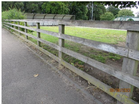
383. Timber horizontal rail fence
