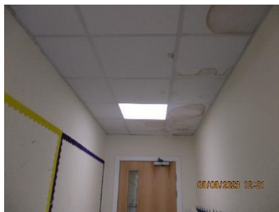
337. Lighting – 1970s extension corridor.
