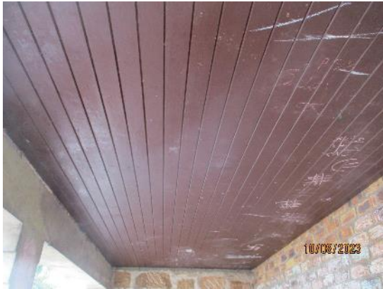
180. Timber linings to external stores
