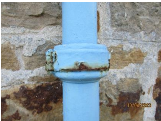
59. Surface corrosion
