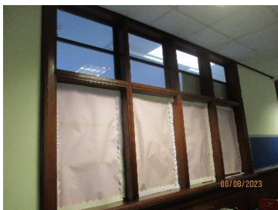
199. Timber borrowed lights in corridors
