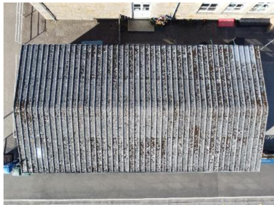
34. Asbestos roof to Nursery
