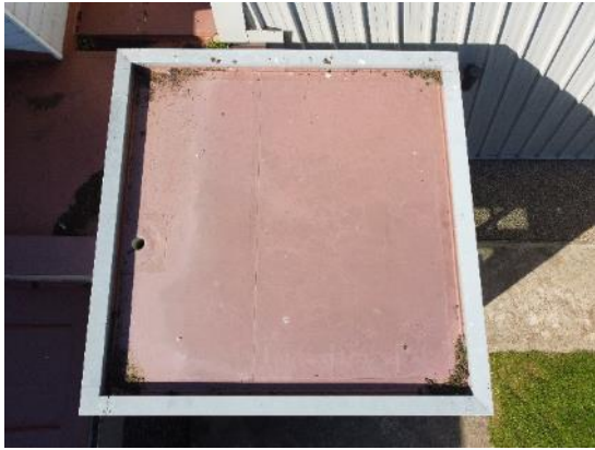
25. Single ply membrane above entrance
