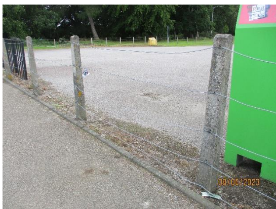
384. Concrete post and wire fence
