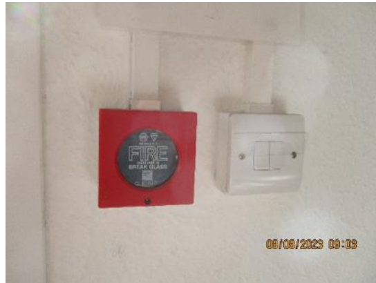
329. Light switch – nursery building typical.
