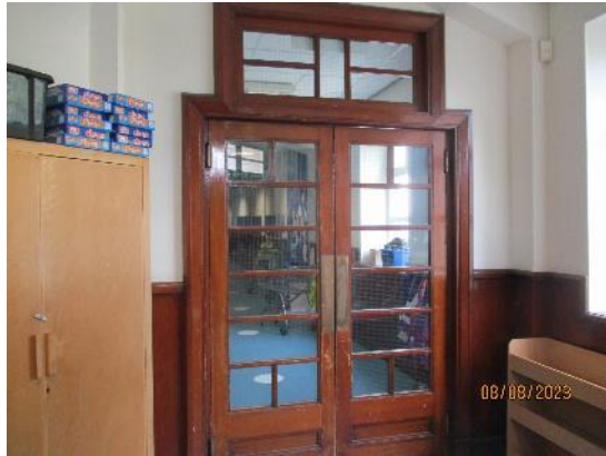
204. Timber panelled double doors
