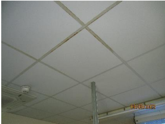
168. Suspended ceiling tiles in the Kitchen
