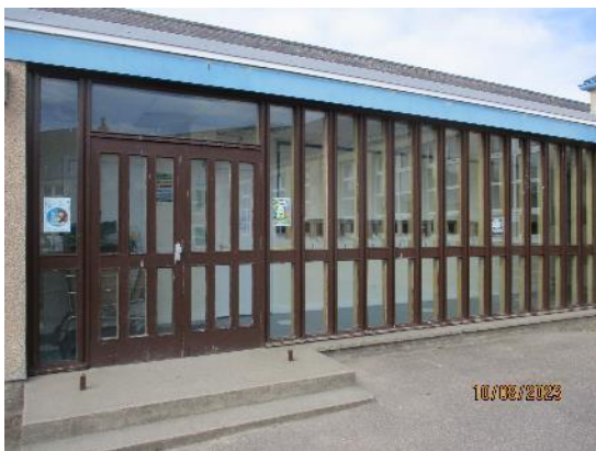
95. Timber screen to 1975 extension
