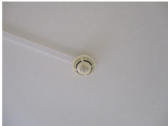
271. Smoke detector block 2 typical.
