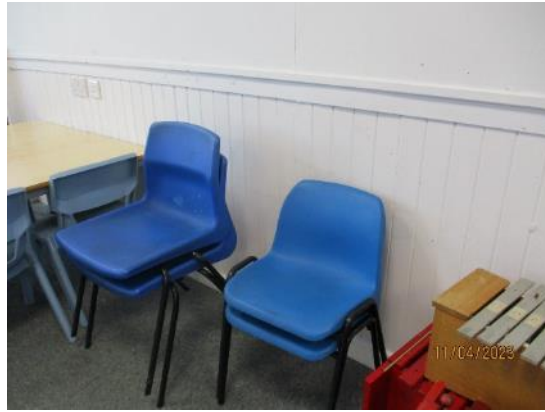
144. Block 1 – Timber linings
