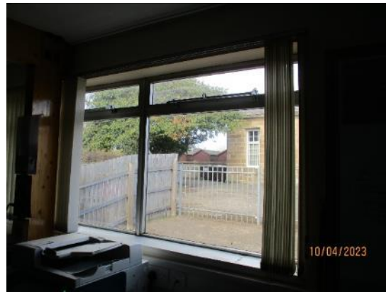
75. Block 2 – Window internally
