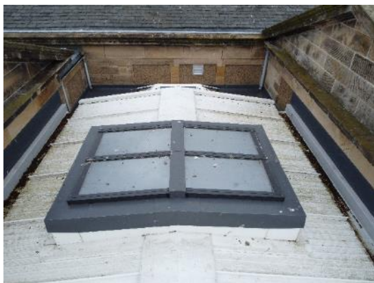
12. Block 1 – skylight over entrance
