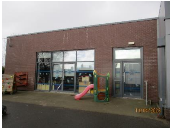
59. Nursery brickwork walls
