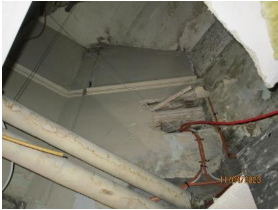
143. Lath & plaster walls
