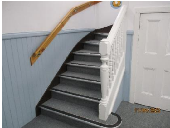
122. Block 1 – Timber staircase
