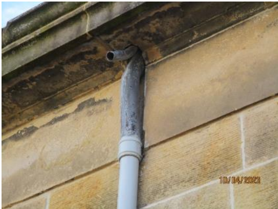
39. Lead / cast iron downpipes
