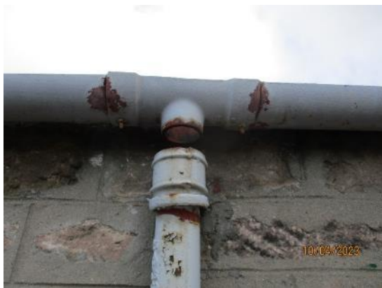
36. Cast iron downpipes
