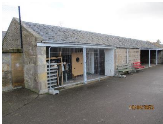
338. External shelter with Heras security fencing
