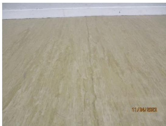
107. Linoleum cracked
