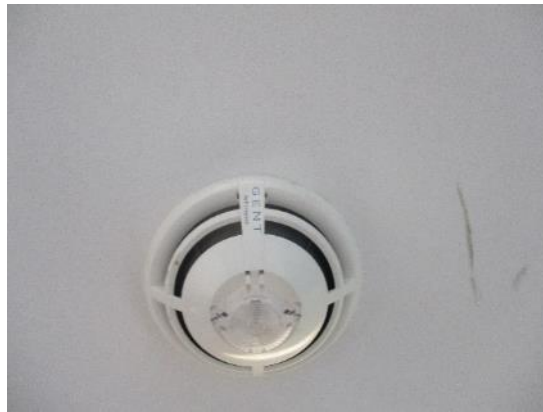
275. Smoke head – block 1 typical.
