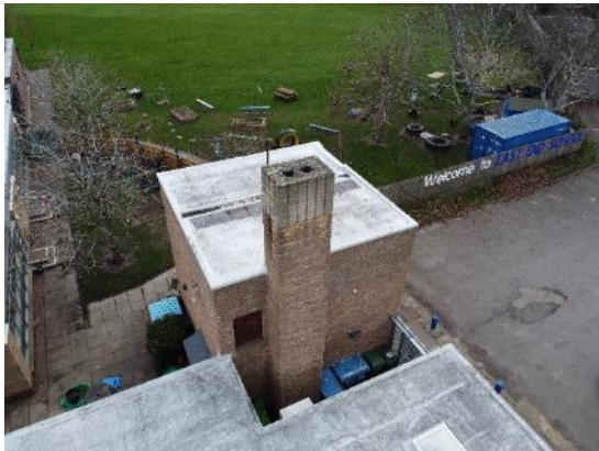
45. Brick boiler flue
