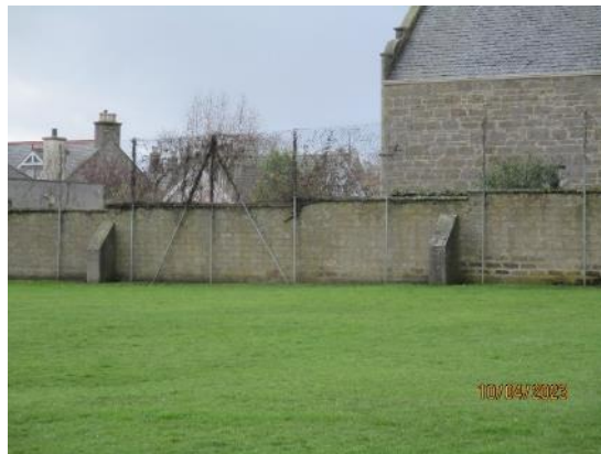
331. Concrete block walls with buttressing
