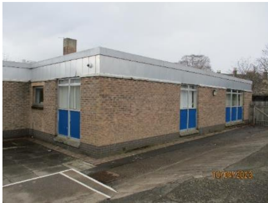
56. Block 2 – Brickwork walls
