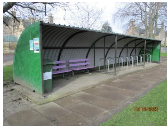
339. Steel framed bike shelter
