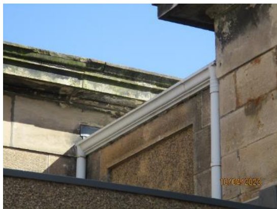
35. Cast iron ogee gutters
