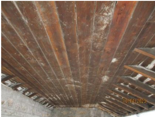
139. External shelter – Timber linings
