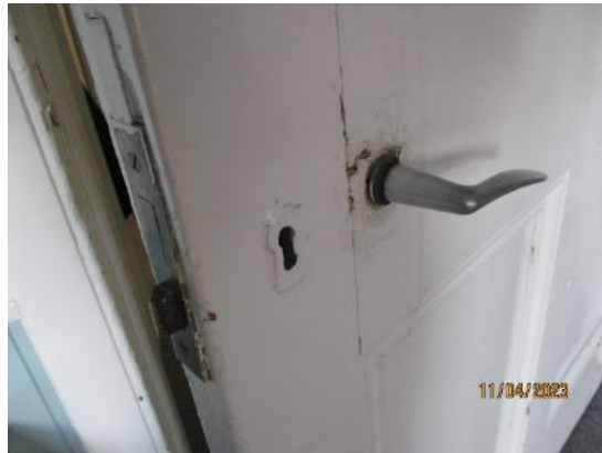
164. Missing aluminium ironmongery
