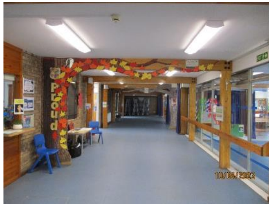
2. Block 2 – Glulam beams
