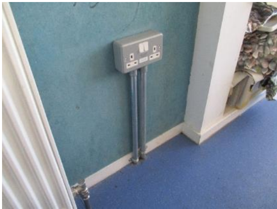
256. Low level surface sockets – block 2 typical.
