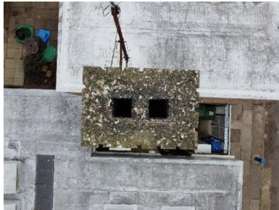
46. Concrete cap to boiler flue
