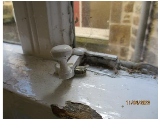
89. Block 1 – window ironmongery
