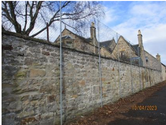
313. High chain link fencing
