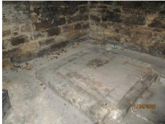
121. Concrete floor and plinths – old Boiler Room
