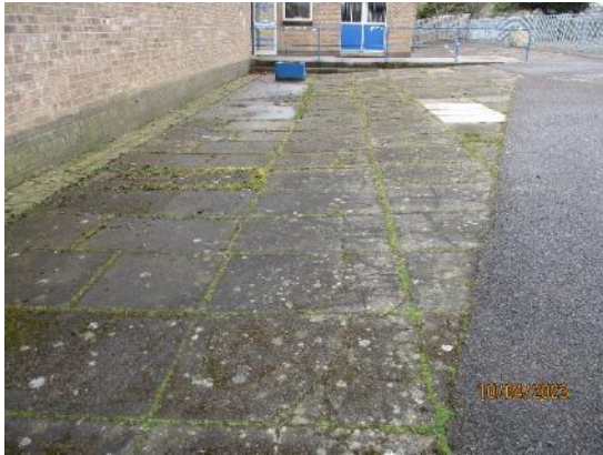
304. Paving slabs to playground
