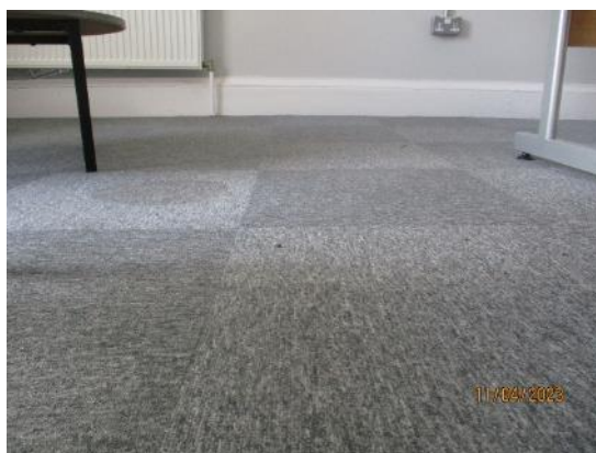
106. Block 1 – Sloping timber suspended floors
