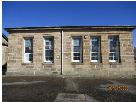
71. Block 1 – Timber sliding sash windows
