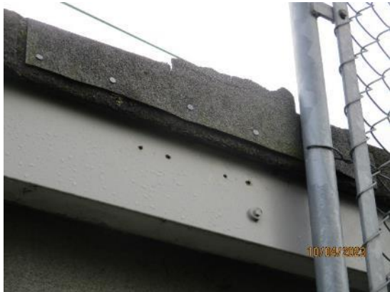
21. External store (former felt roof)
