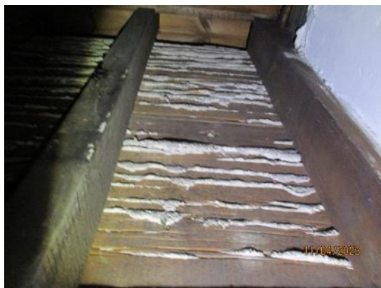
141. Block 1 – Lath & plaster walls
