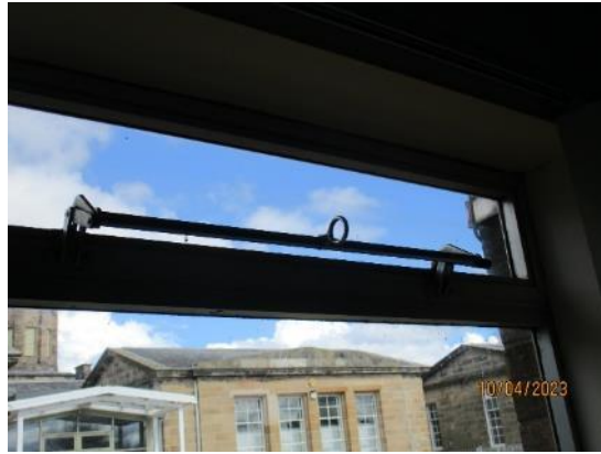
87. Block 2 window ironmongery
