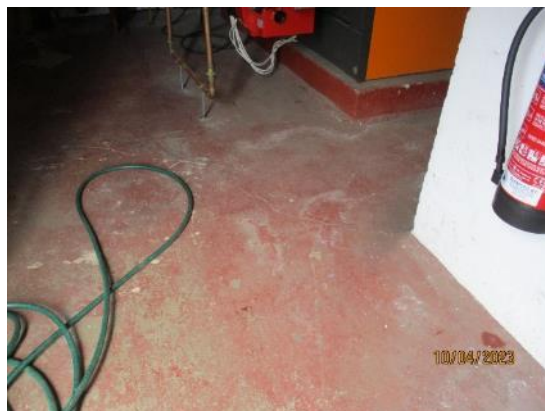
119. Painted concrete floor
