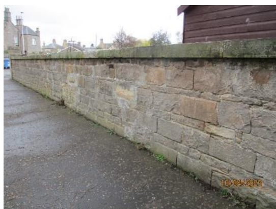
325. Natural stone walls
