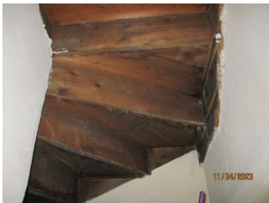
124. Underside of timber staircase
