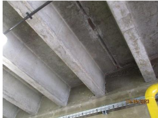
138. Concrete beam ceiling
