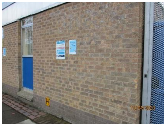
48. Block 2 – Brick walls
