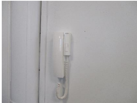
295. Security door audio control handset. Block 1 Annexe.
