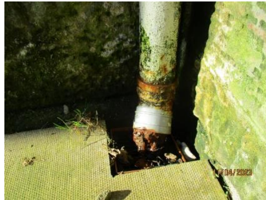
40. Blocked downpipes
