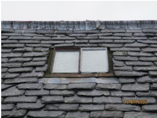
33. External shelter metal skylight
