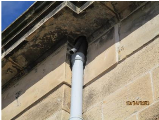
37. Block 1 – downpipes and overflows
