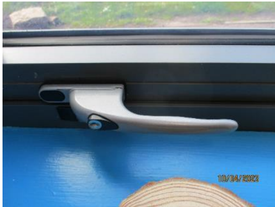
88. Nursery – window ironmongery
