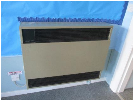
216. Convector heater block 1 annexe typical.
