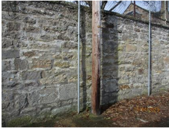
346. Utility pole in car park
