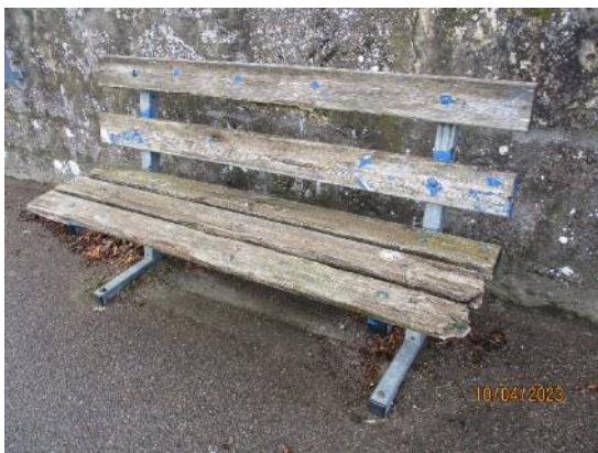
308. Timber benches with timber rot
