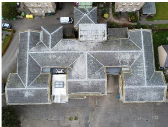
5. Block 1 – Roof overview
