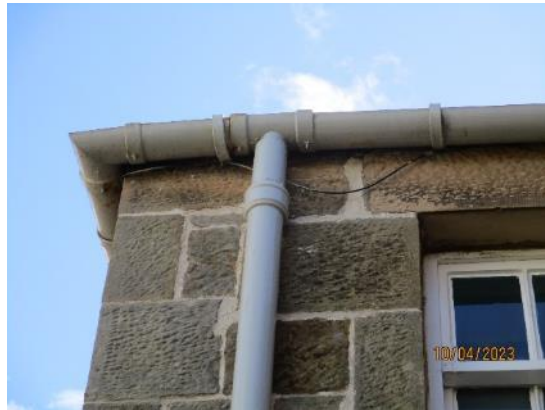
34. Half round cast iron gutters
