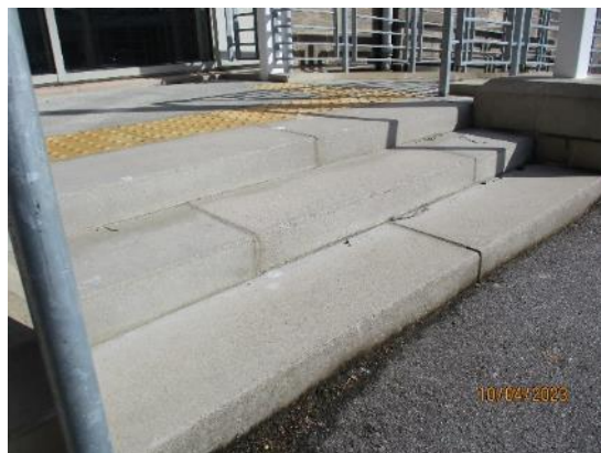
101. Block 1 – Concrete steps
