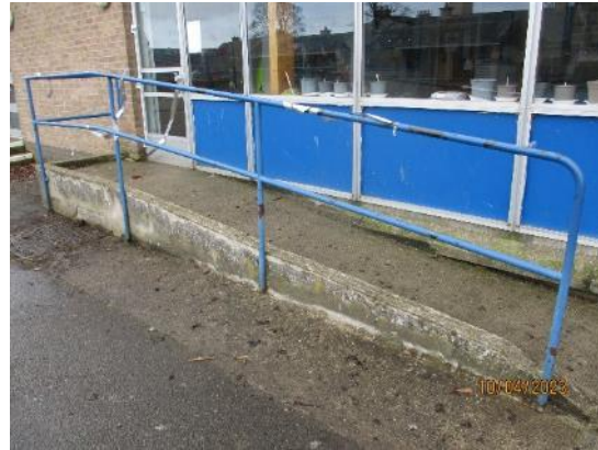
103. Tubular metal handrails
