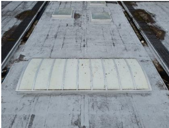
27. Barrel vault rooflights
