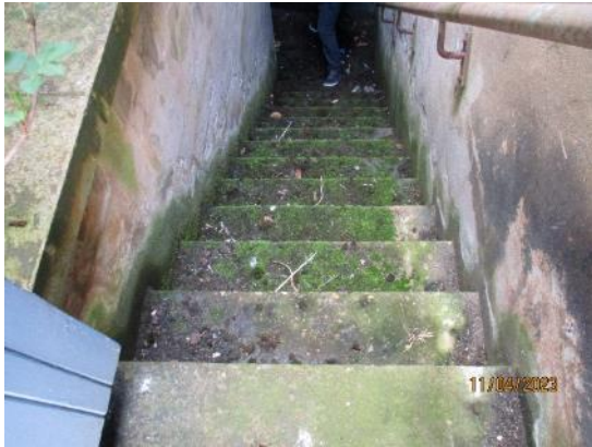
102. Concrete steps to Boiler Room
