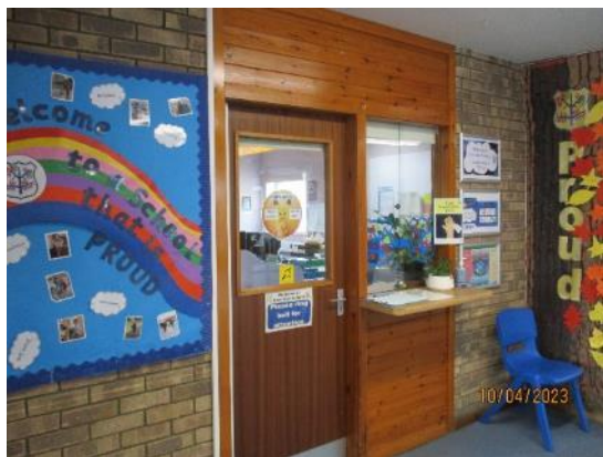
147. Block 2 – Brick walls
