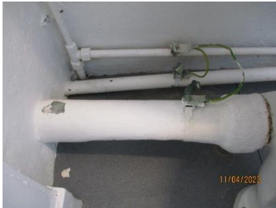
182. Lead waste pipes (Block 1)
