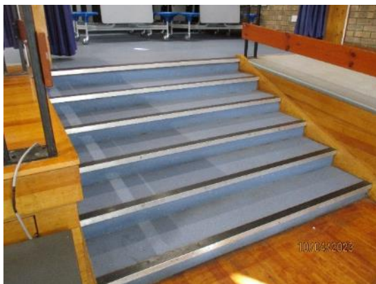
125. Block 2 – Timber stair
