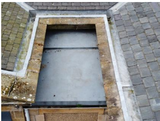
11. Single ply membrane and lead secret gutters
