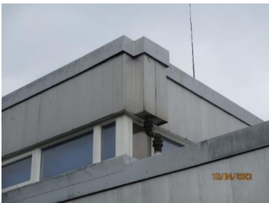
41. Block 2 – Cast iron internal downpipes
