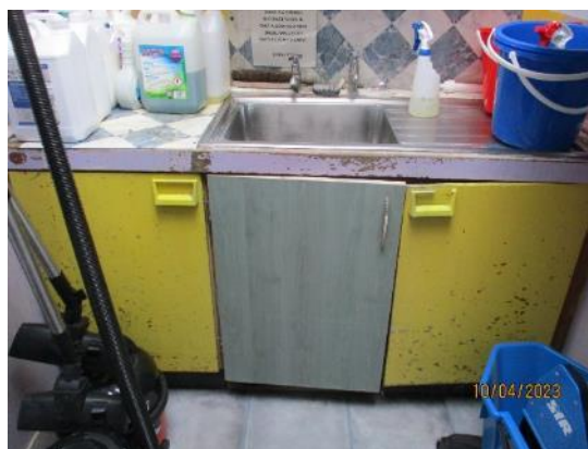
202. Cleaners sink base units
