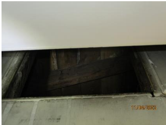
1. Block 1 – Timber trusses
