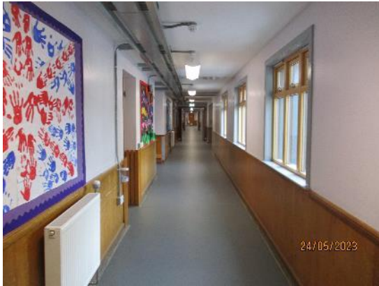
114. Timber wall panelling in the primary school
