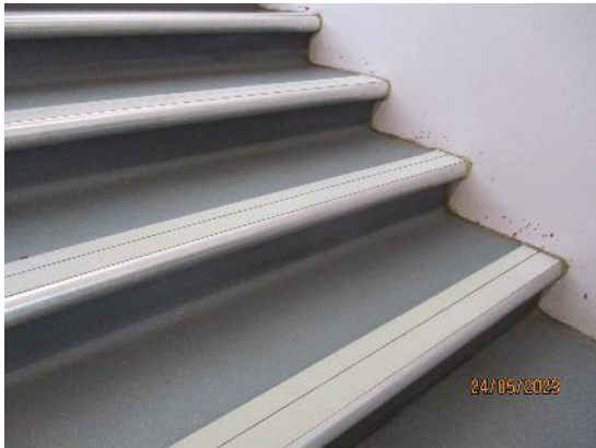
99. Sheet vinyl treads and risers
