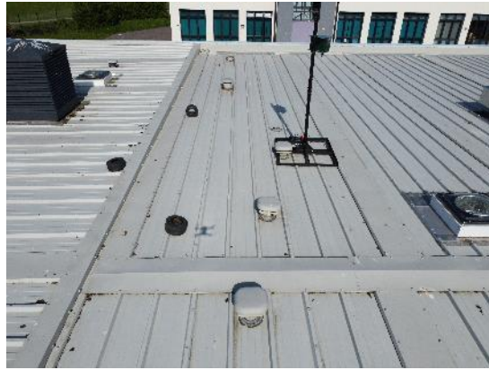
8. Metal standing seam roof with bird scarer
