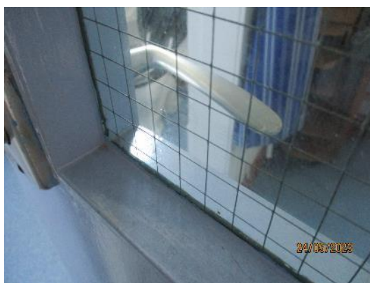
135. Georgian wired glass to some doors
