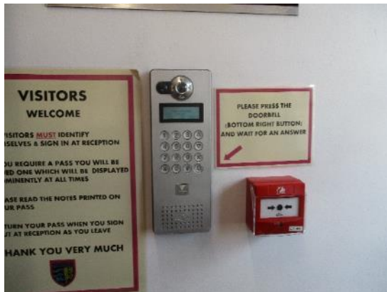
228. Security door entry keypad and video unit main school.
