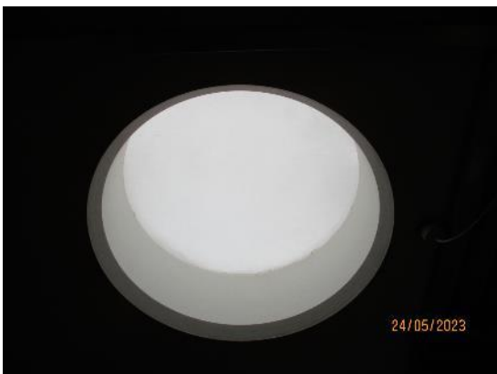
17. Internal view of rooflights
