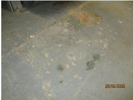
91. Boiler room painted concrete floor
