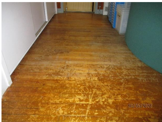
165. Timber floor boards
