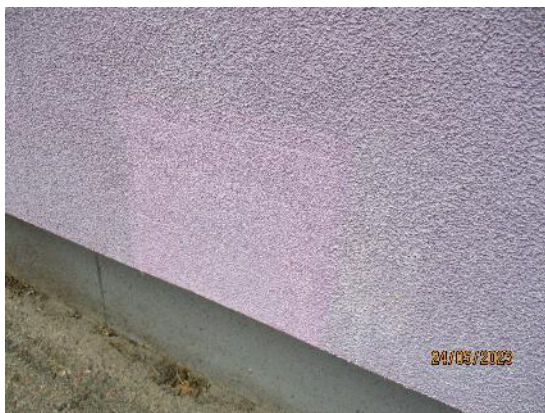
54. Isolated areas of previous repair
