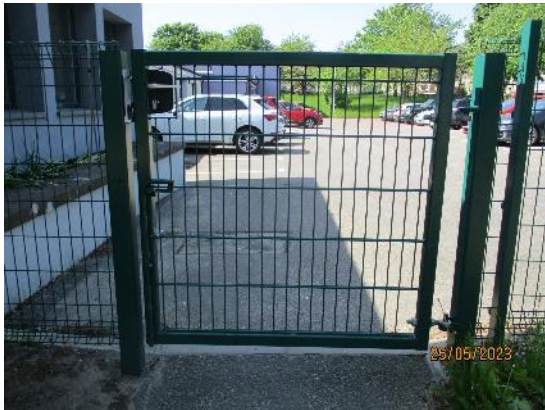
264. Security mesh pedestrian gates
