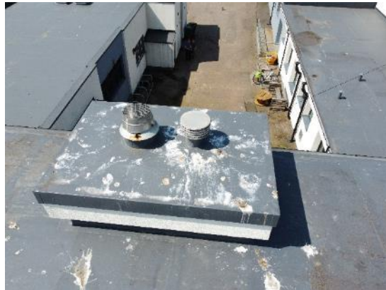
235. Boiler flue termination main school roof level.
