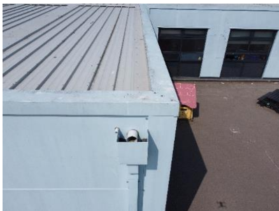
36. Metal roof outlets
