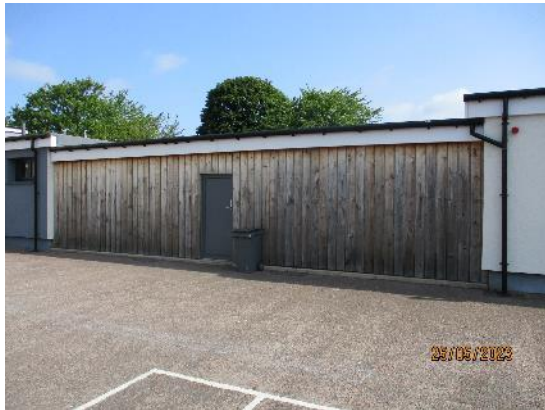
51. Timber lining boards
