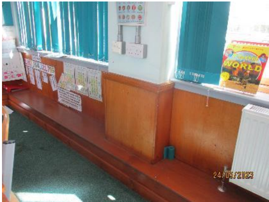
116. Panelling to classroom walls
