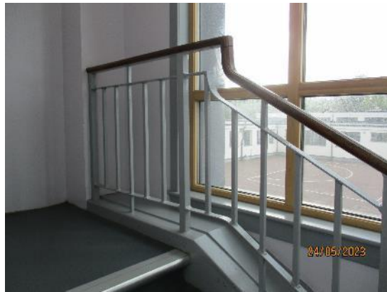
104. Metal balustrades with timber handrails
