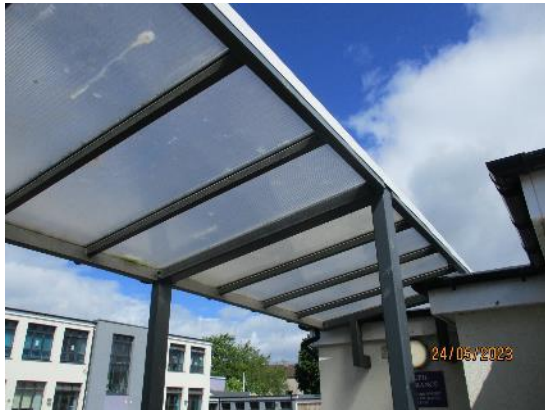
10. Glass canopy roof – School to Nursery
