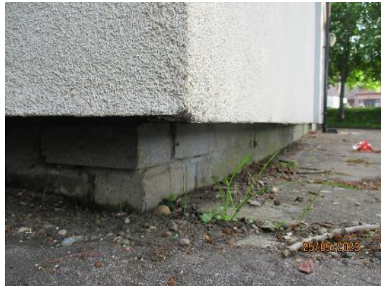
46. Projecting external insulation
