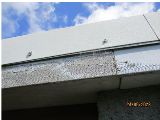
23. Plywood fascia boards
