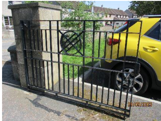
259. Metal bar vehicle gates
