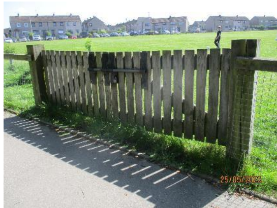
265. Timber boarded gates.
