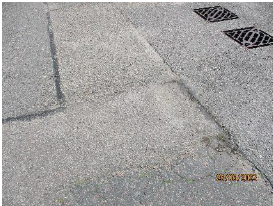
240. Tarmacadam car park
