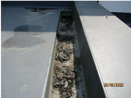
27. Flat roof box gutters
