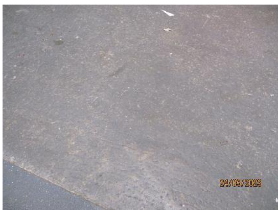
90. Painted concrete floors
