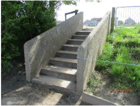
250. Concrete staircase to playing field
