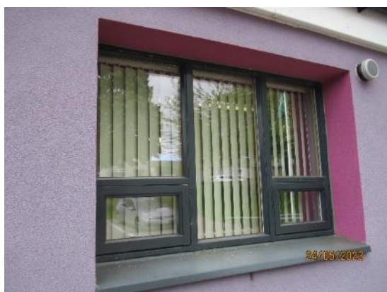
63. Powder coated standard window
