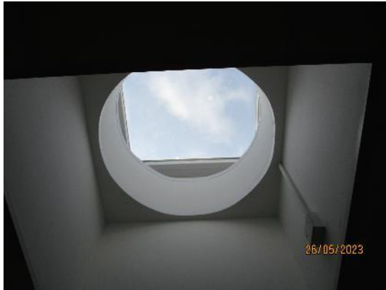
19. Nursery Rooflights internally
