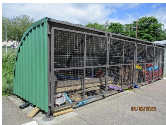
278. Metal profile and caged enclosure
