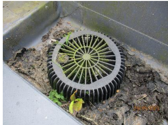
28. Flat roof rainwater outlets
