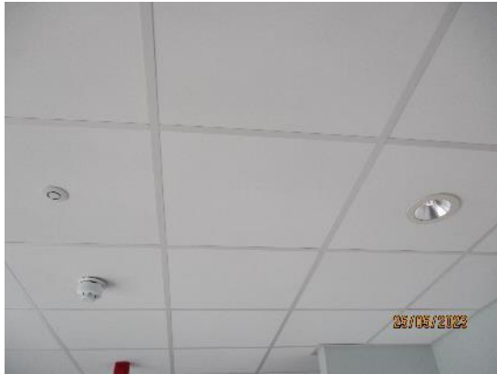
109. Nursery suspended ceiling tiles
