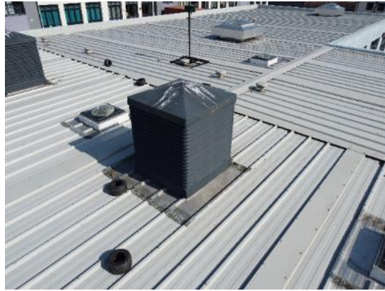
233. Passive windcatcher units – modular nursery.
