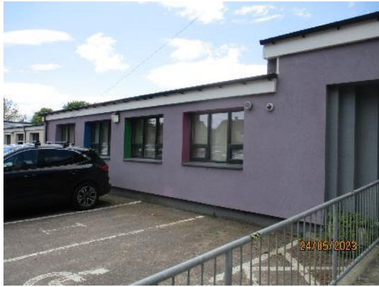
49. Primary school external insulation
