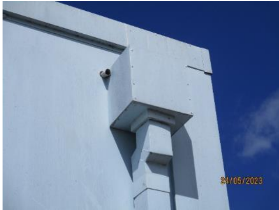
37. Metal hopper heads and downpipes
