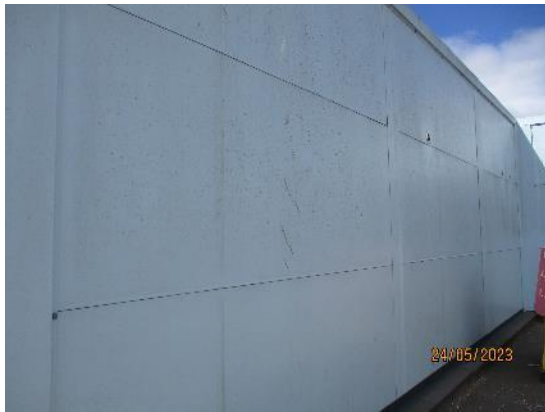
55. Nursery – Metal composite panel walls
