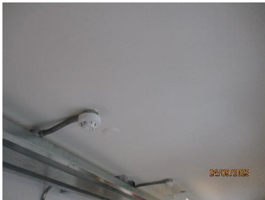
106. Primary school plastered ceilings
