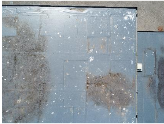
2. Single ply membrane (insulation sheets visible)
