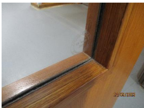
134. Safety glass to replacement doors
