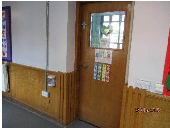
121. Typical timber hollow core door
