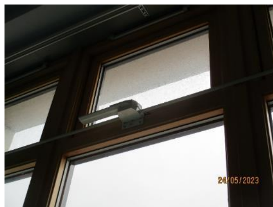
72. High level mechanisms operated by winding handle
