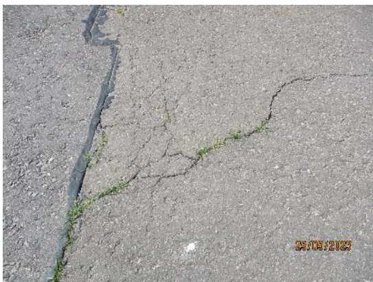
242. Tarmacadam cracking
