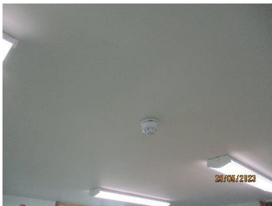
108. Plasterboard ceilings in The Hub
