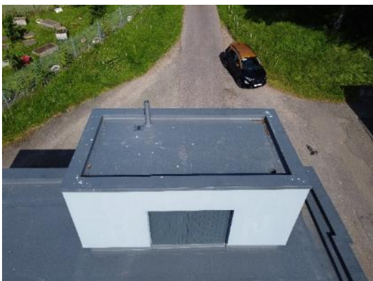
41. Water tank house roof
