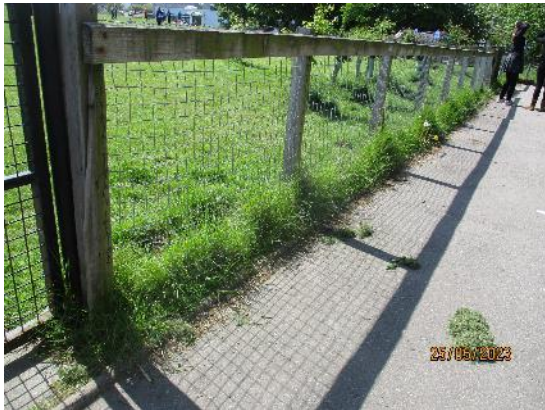
258. Timber post and mesh fencing
