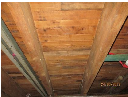
83. Timber suspended floor of the stage
