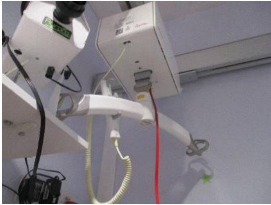
232. Person hoist system – main school.
