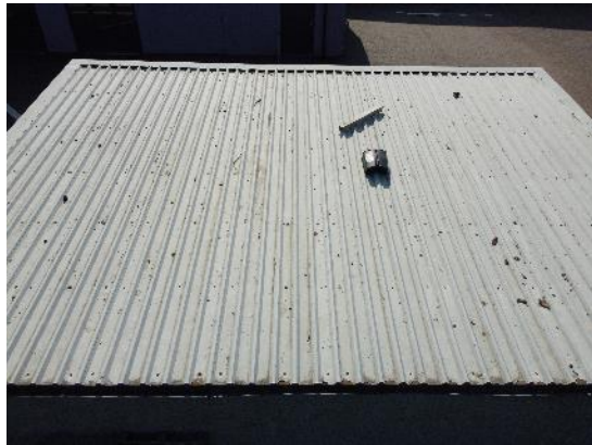
9. Metal profile roof to shelter/garage
