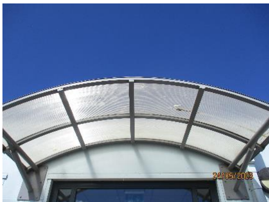
12. Polycarbonate canopy to Nursery entrance
