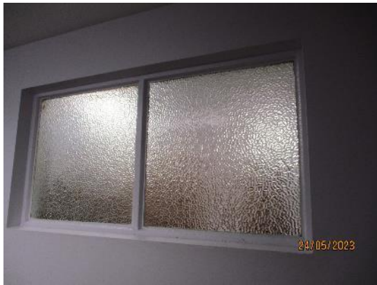
120. Internal borrowed lights (toilets)
