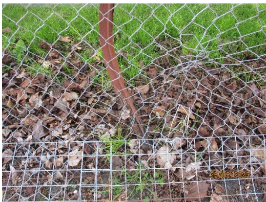
254. Impact damage to steel frame
