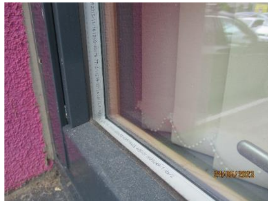
70. All windows are double glazed
