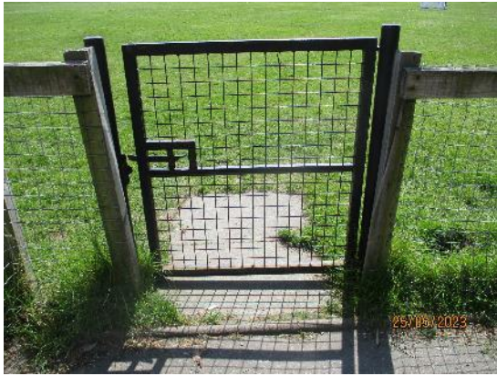
268. Metal framed gates
