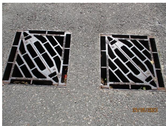
275. Car park and playground drainage
