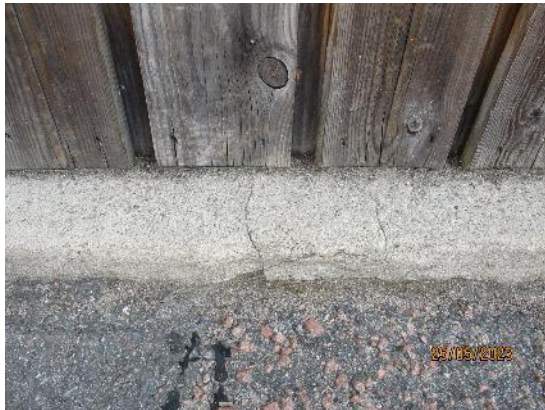
52. Boards close to concrete slab
