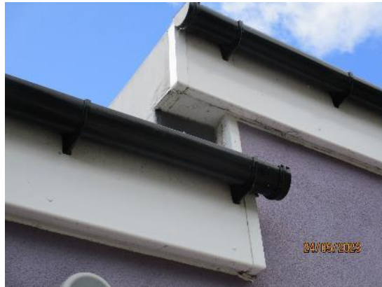
22. UPVC fascia boards
