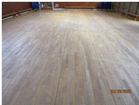
65. Timber sports floor
