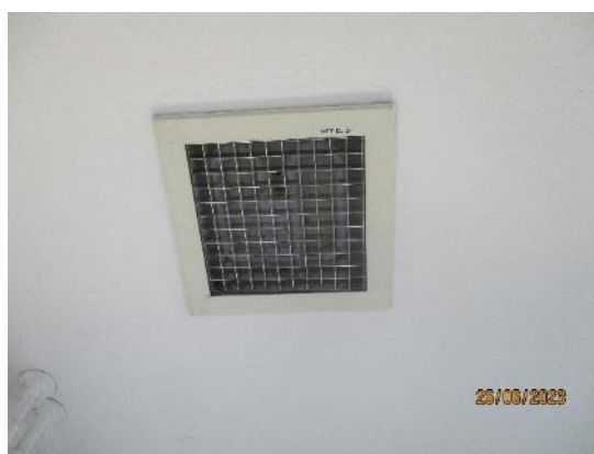
172. Lighting – circulation areas typical.
