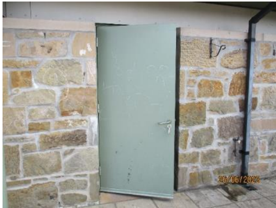
50. Timber external doors
