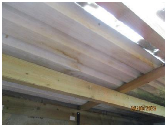
6. External store timber joists
