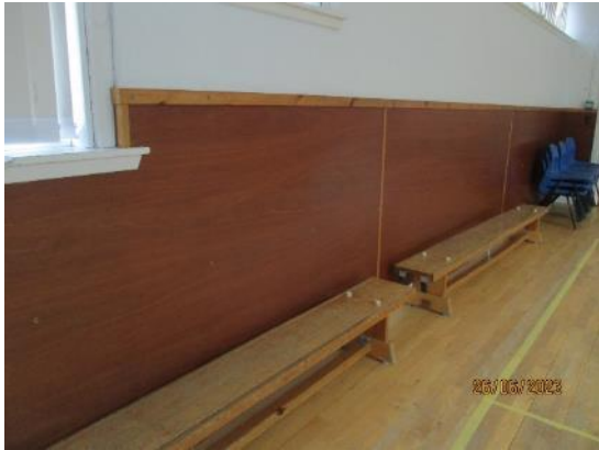
82. Timber linings to Games Hall walls
