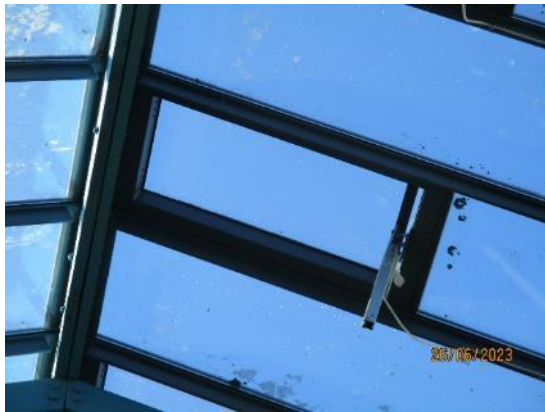
19. Electrically operated skylights
