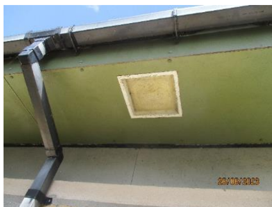
174. External building lighting typical.
