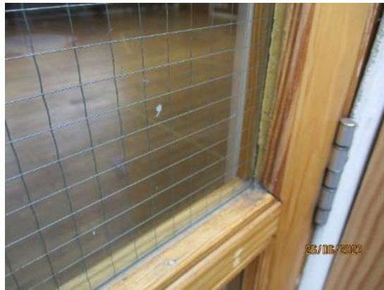
101. Georgian wired glass to doors
