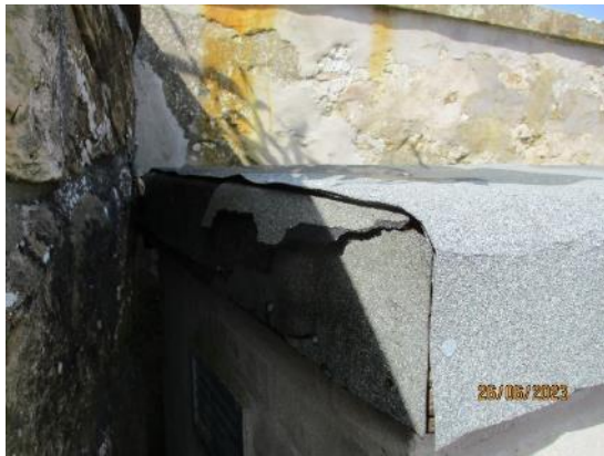
13. Felt roof to gas meter house
