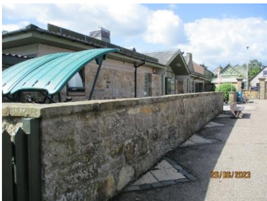
211. Natural stone garden walls
