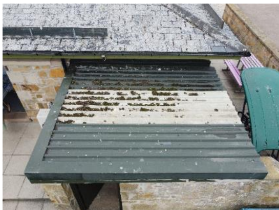
12. Metal profile flat roof (external store)
