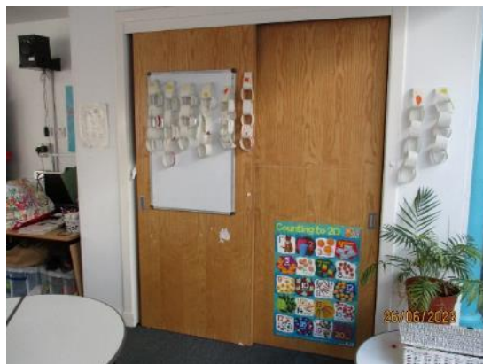
93. Double timber doors
