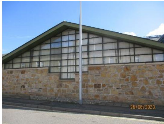
40. Large timber glazed screen
