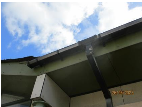
29. UPVC gutters and downpipes
