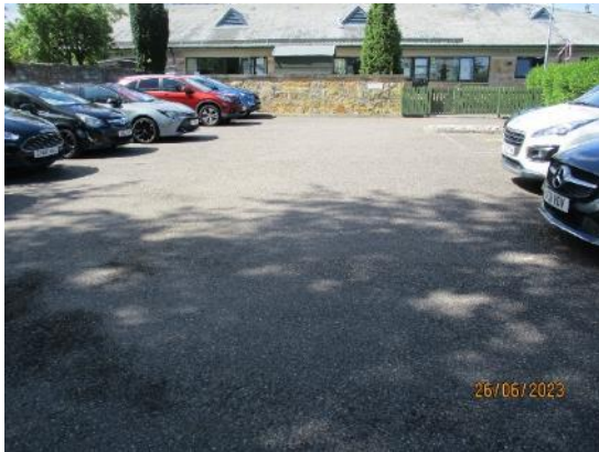
191. Tarmacadam car park
