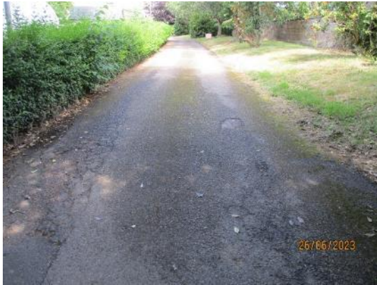
189. Tarmacadam shared access road
