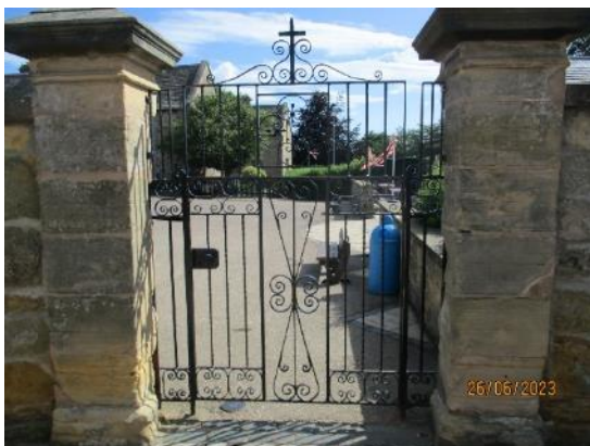
205. Metal rail gate
