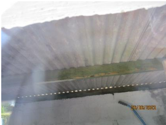
7. Salt store timber joists
