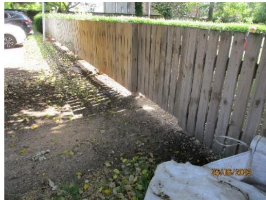
202. Timber boarded fencing
