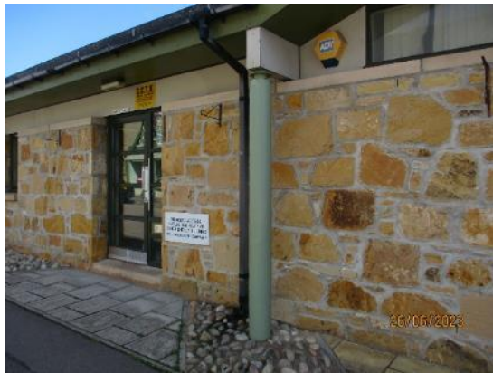
1. Steel frame externally
