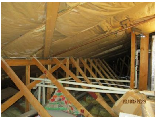
5. Timber trussed roof
