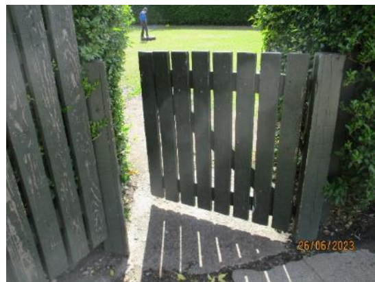
206. Timber boarded gates
