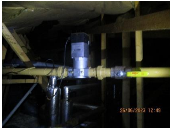
148. Gas pipework – kitchen supply attic space.
