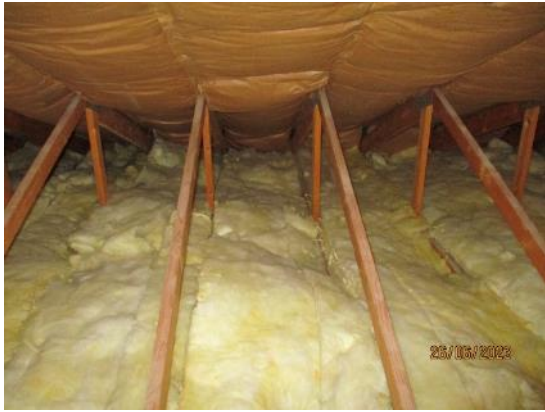
25. Mineral fibre insulation laid on ceilings
