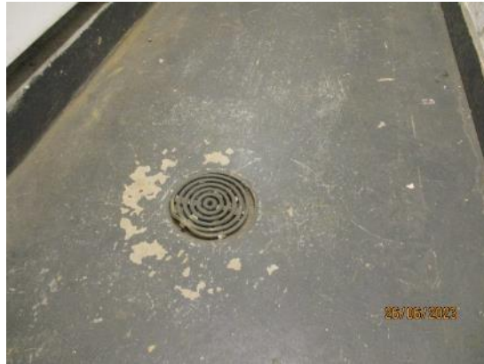
67. Painted concrete floors
