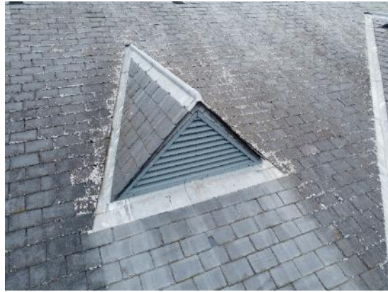
49. Timber roof ventilation grills
