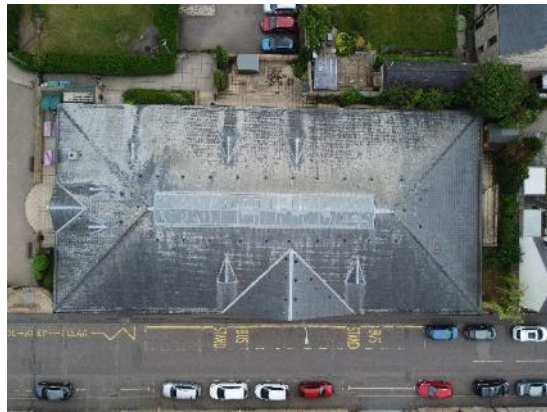
8. Overview of slated roof
