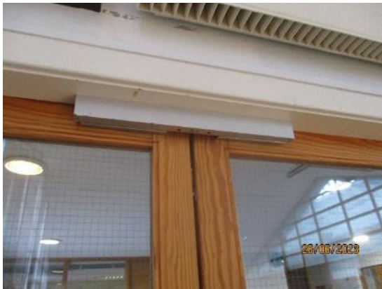
183. Security door electro magnet unit typical.
