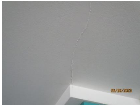
74. Cracking at steel columns
