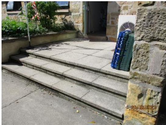
54. Paving slab steps
