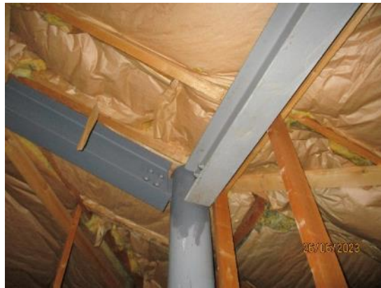
2. Steel columns & beams within roof space
