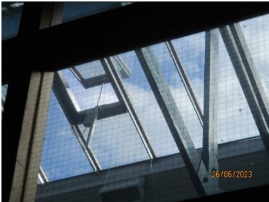
90. Screen glazed with Georgian wired glass
