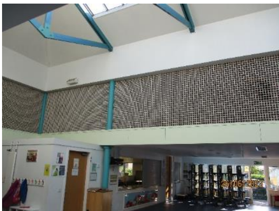
80. High level lattice panelling
