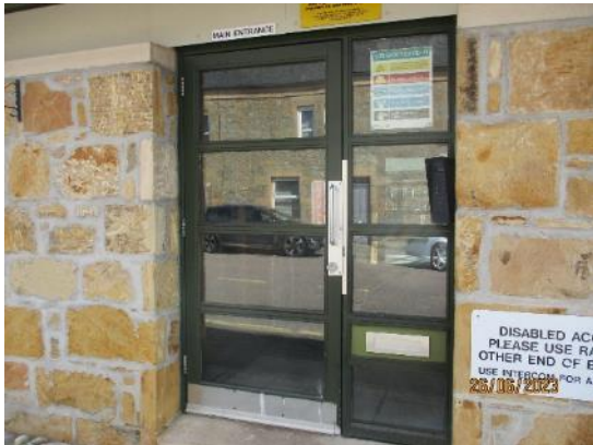
33. Timber glazed entrance door
