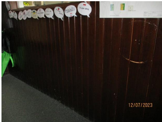
160. Tongued & grooved timber linings
