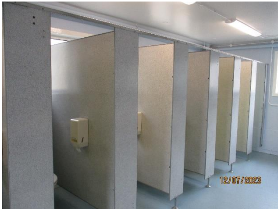
204. Composite panel cubicle partitions
