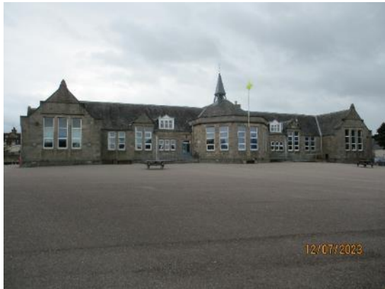
62. Stone walls to school building
