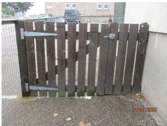
322. Timber boarded gates
