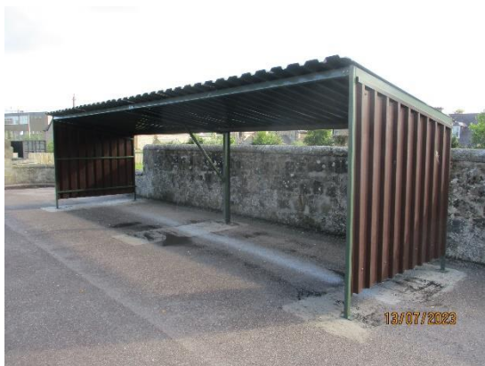
346. East playground shelters
