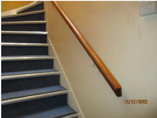
140. Timber handrails to staircases
