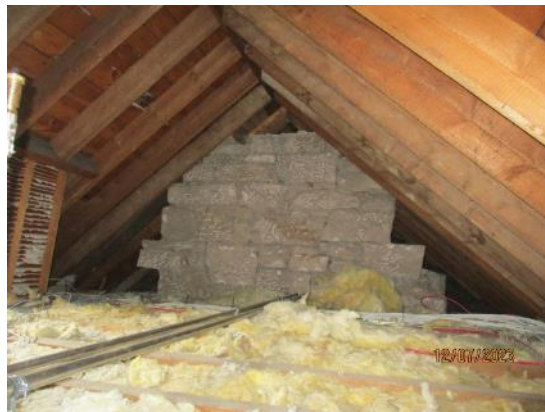
4 Stone chimney breast.
