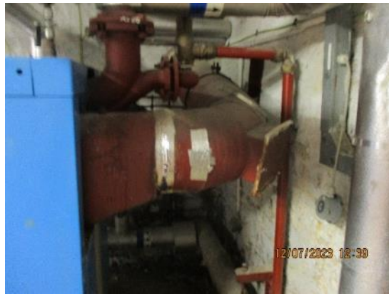
229. Boiler flue into brick chimney 0/1
