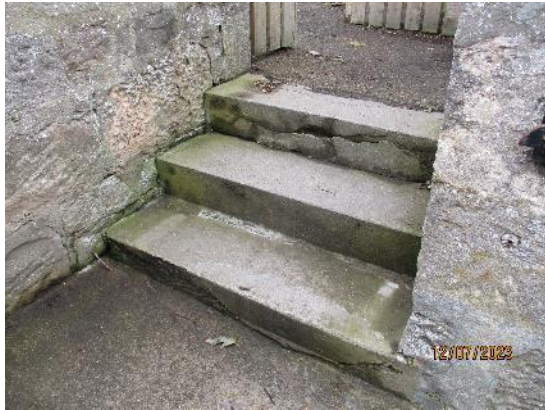
306. Concrete steps (North entrance)
