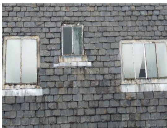
26. Various metal skylights
