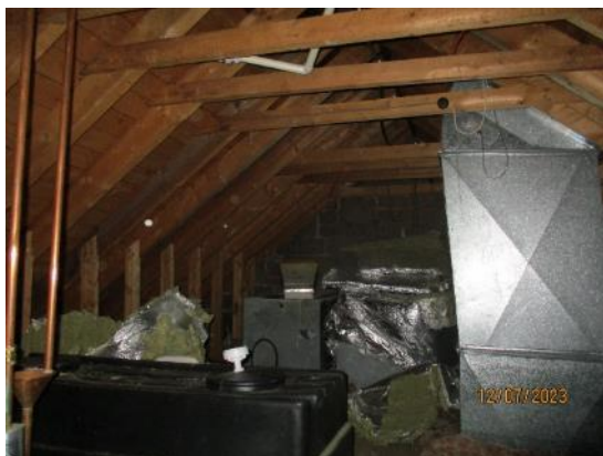
5. Timber roof trusses over Dining Hall
