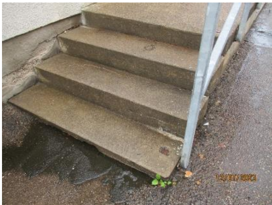
116. Concrete steps to Ding Hall
