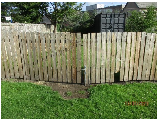
323. Timber boarded double gates
