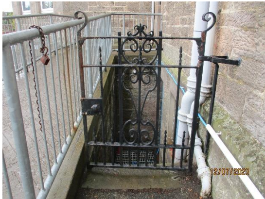
327. Metal decorative gate to Boiler Room
