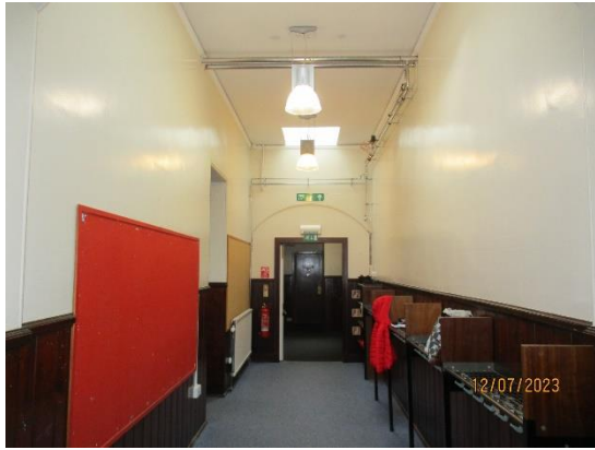
154. Lath & plaster walls
