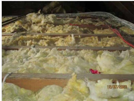
32. Insulation to school roofspace
