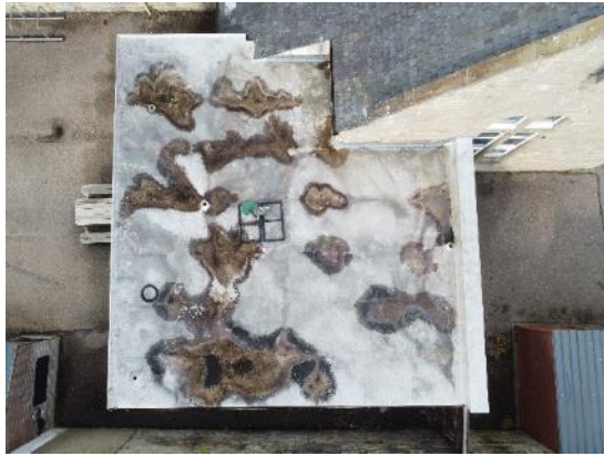
13. GRP roof over Girls toilet
