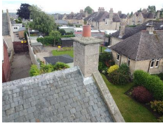
56. Stone chimney to Dining Hall
