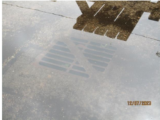
337. Blocked drainage
