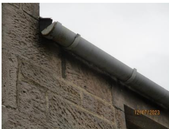
36. Cast iron gutters to school building
