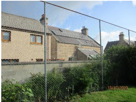
315. Chain link fencing to sports field
