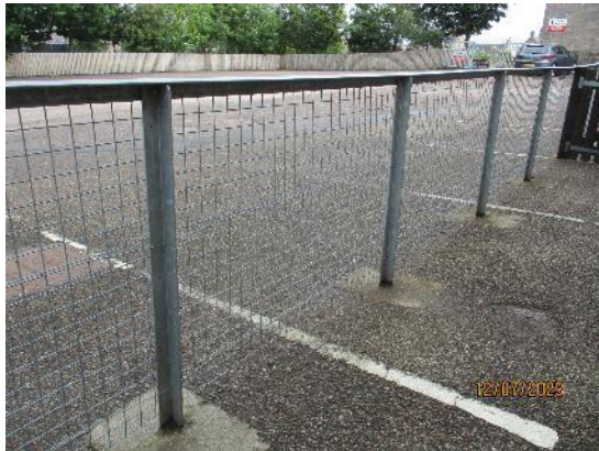
320. Galvanised mesh fence (car park)
