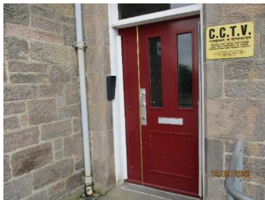
89. Timber school entrance door
