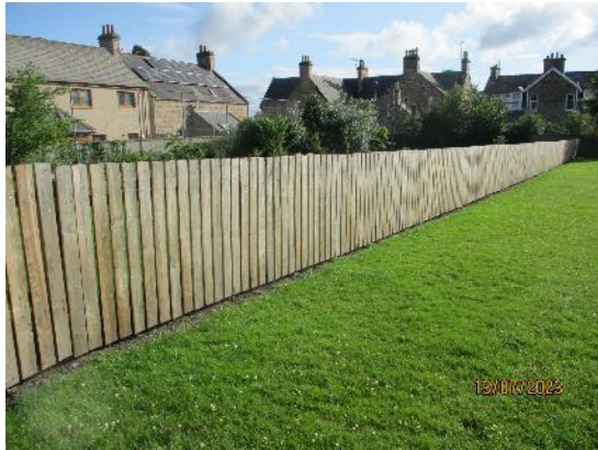
318. Timber boarded fence (sports field)
