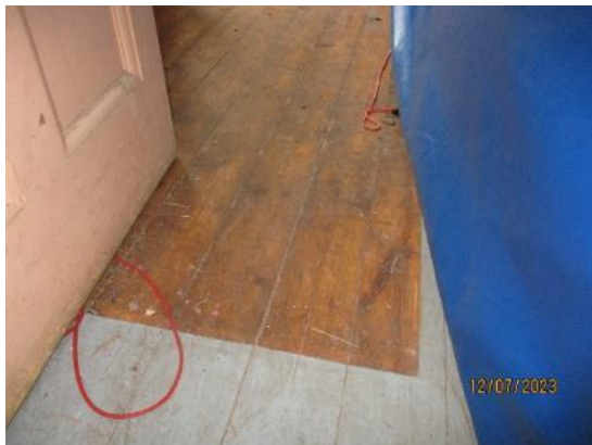
134. Timber floor boards
