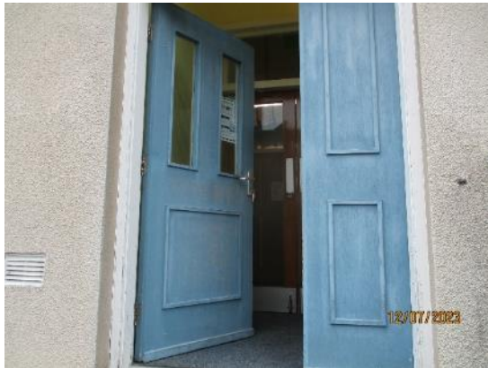
93. Timber Dining Hall entrance door
