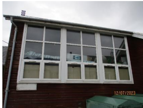
97. UPVC windows to Hut
