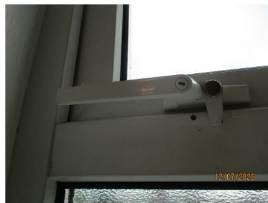
101. Lockable lever handles to windows
