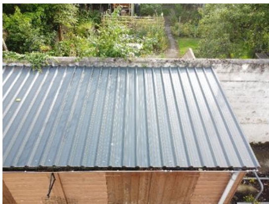
23. Metal profile roof
