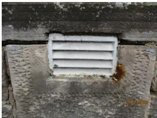
76. Underfloor ventilation to Dining Hall
