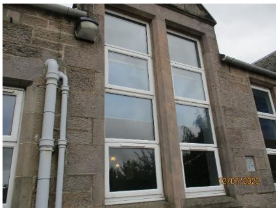
94. Large upvc windows to school
