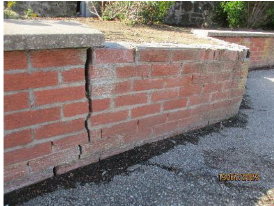
313. Damaged raised beds
