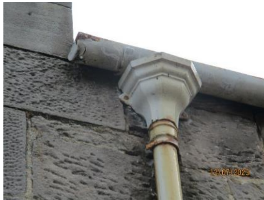
50. Cast iron hopper heads and downpipes to Dining Hall
