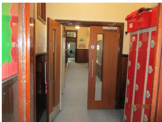
178. Timber veneered double doors
