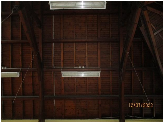
145. Timber linings to Games Hall
