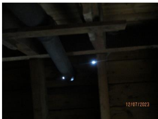
12. Daylight visible around vent pipe (see 10)
