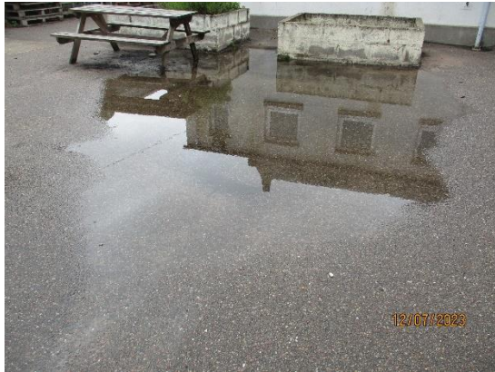
336. Surface water flooding (West playground)
