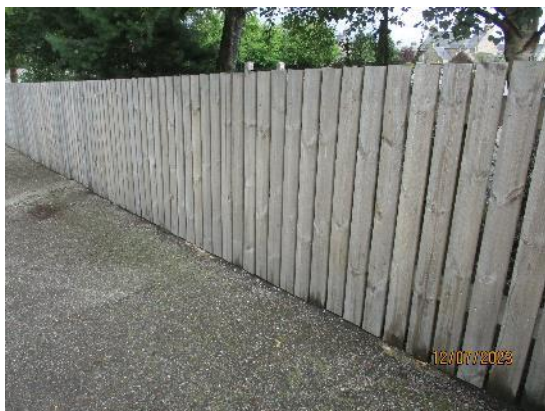
317. Timber boarded fence (car park)
