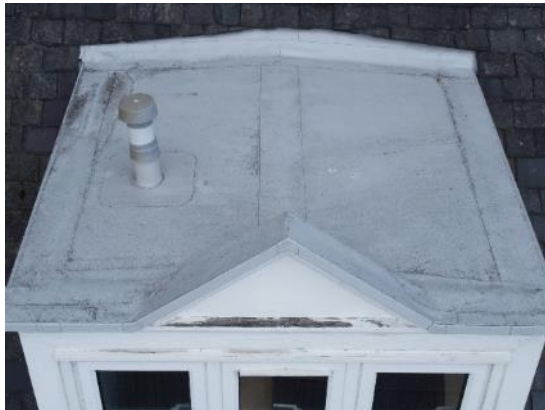
15. Single ply membrane to dormer roofs
