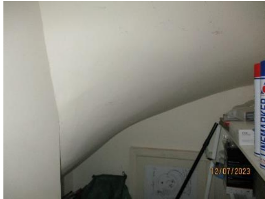
139. Plaster soffits to stairs
