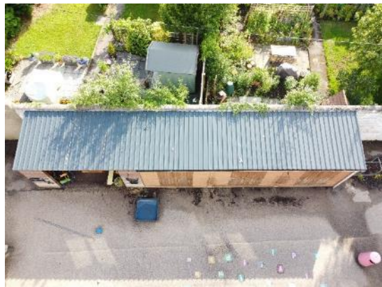
22. External stores – overview of metal profile roof
