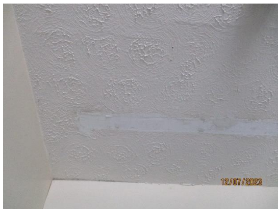
141. School – textured finish on lath & plaster
