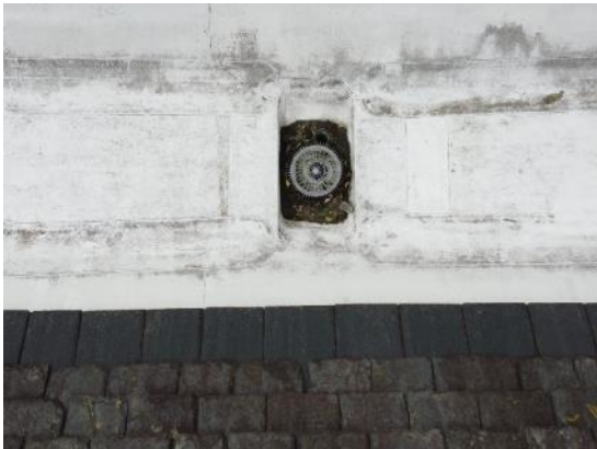
39. Valley gutter outlets
