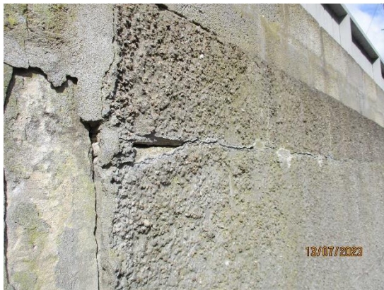
333. Horizontal cracking
