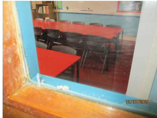
187. Plain glass to classroom doors
