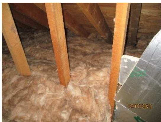
35. Insulation above Dining Hall
