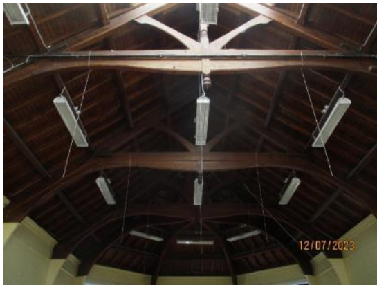
1. Exposed trusses in Hall
