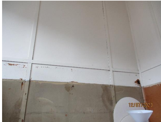
167. Fibreboard and timber straps in the Hut
