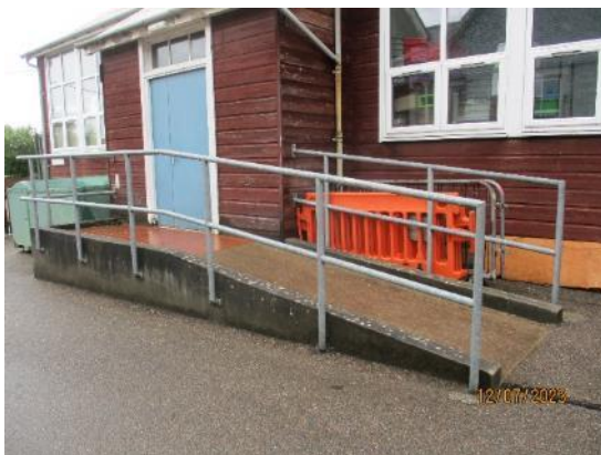
112. Steep concrete ramp to Hut
