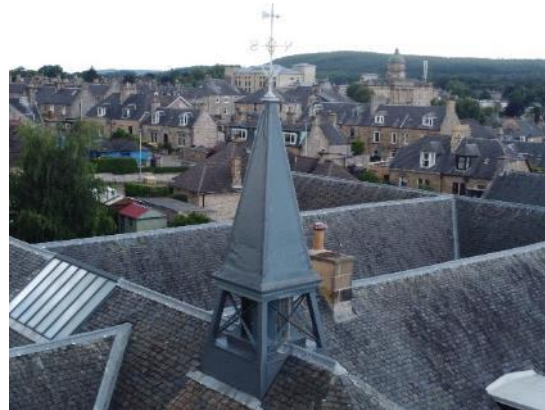
58. Timber framed bell tower
