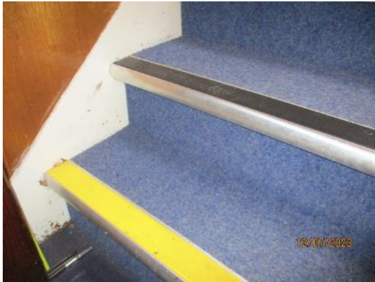
138. Carpet and aluminium nosings to stairs
