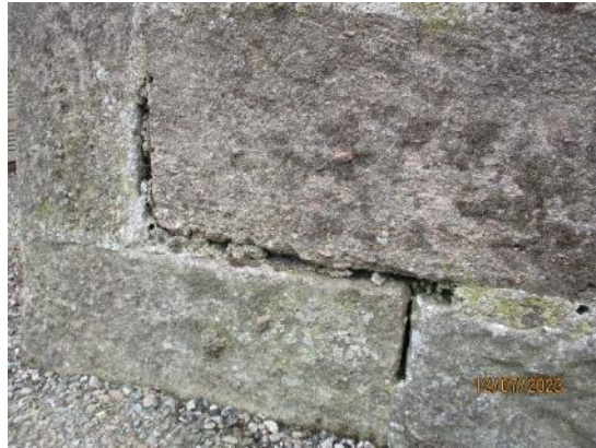
79. Isolated pointing required
