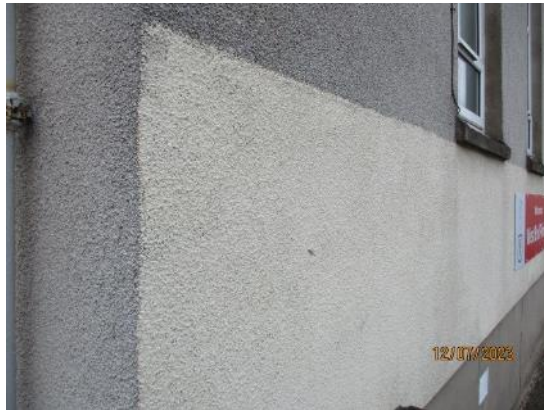
69. Masonry walls to Dining Hall
