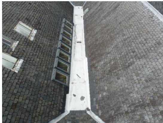
38. Valley gutter to school
