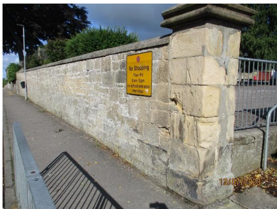
328. High stone boundary walls
