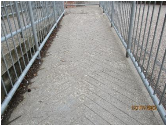
110. Concrete entrance ramp to school
