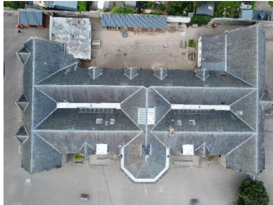
8. Main school overview of slated roof
