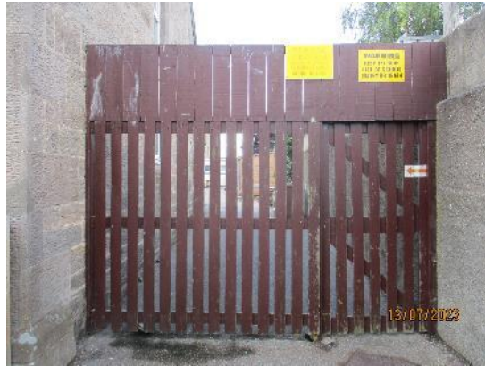
319. High timber boarded fence
