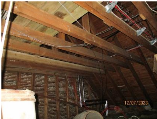
3. Timber trusses in school roofspace
