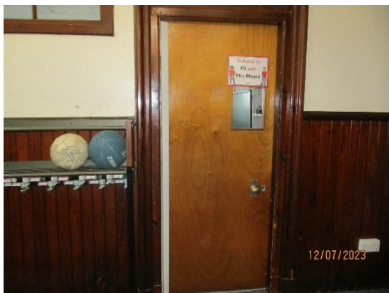
170. School – Timber hollow core doors
