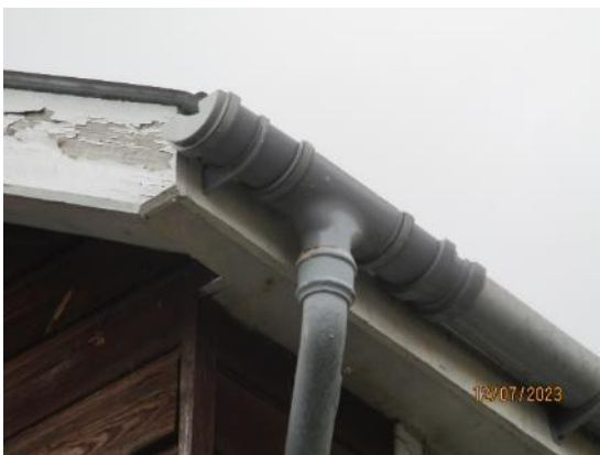
41. UPVC gutters to Hut
