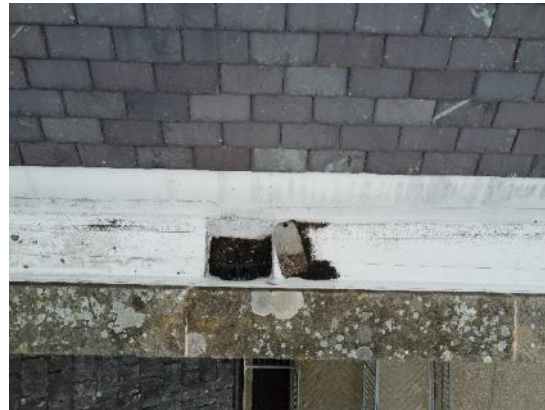
40. Slipped slate and blocked outlet above Games Hall
