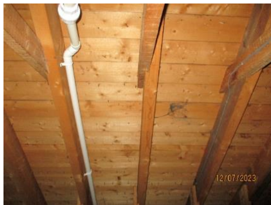
6. Timber sarking boards
