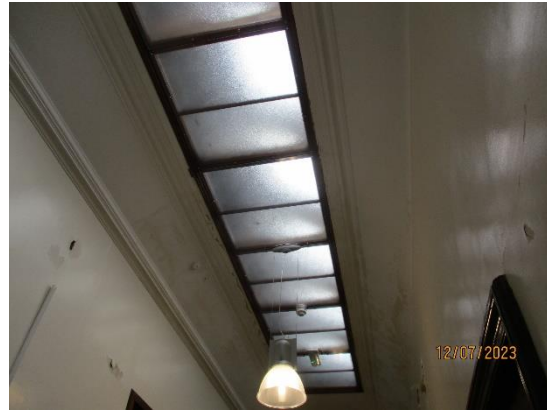
150. Borrowed lights below velux windows
