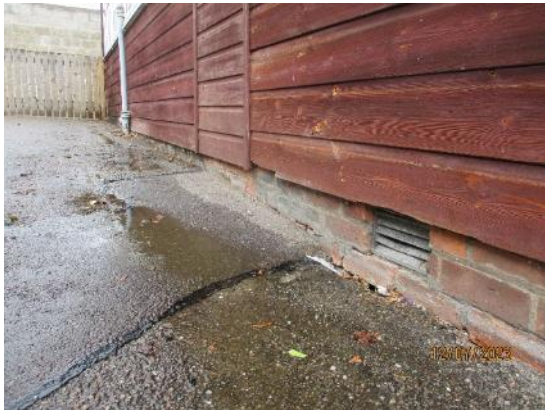
74. Reduced ground level to Hut
