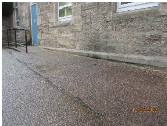
77. Reduced ground level to Dining Hall
