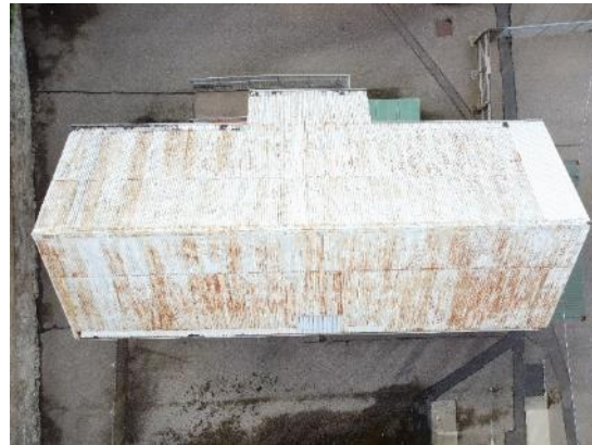
16. Hut corrugated iron roof - overview
