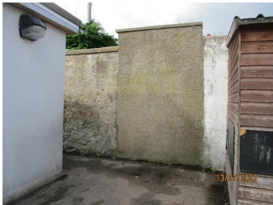
332. Concrete block walls
