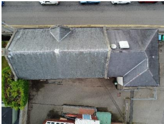
19. Dining block – overview of slated roof
