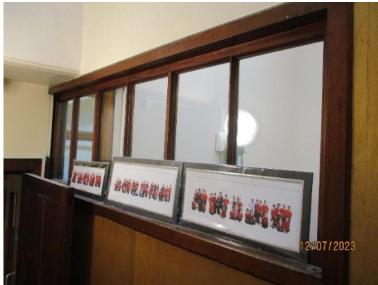
168. Timber borrowed lights in the school
