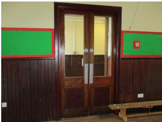
174. Timber panelled double doors
