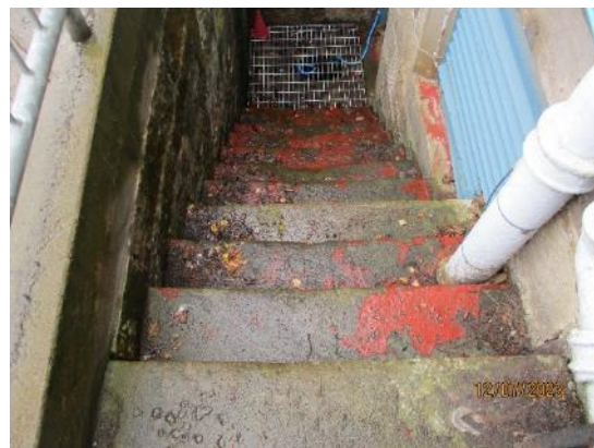
113. Stone/concrete steps to Boiler Room
