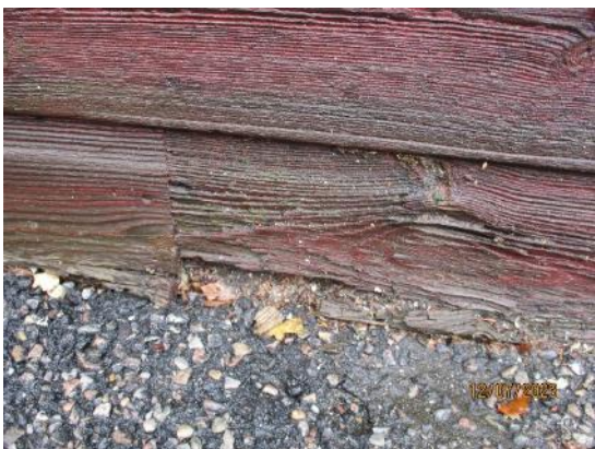
82. Saturated timber linings to Hut
