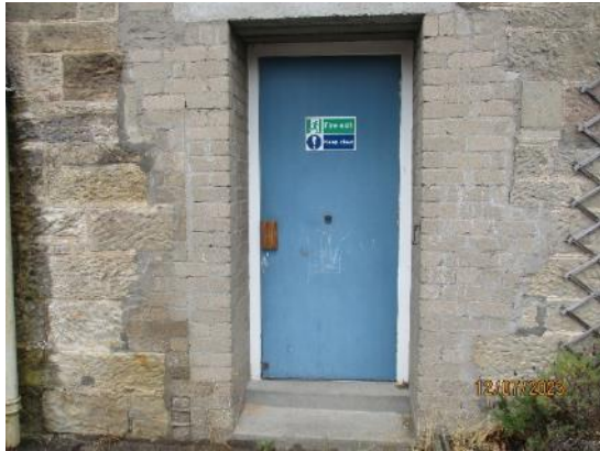
90. Timber fire escape doors
