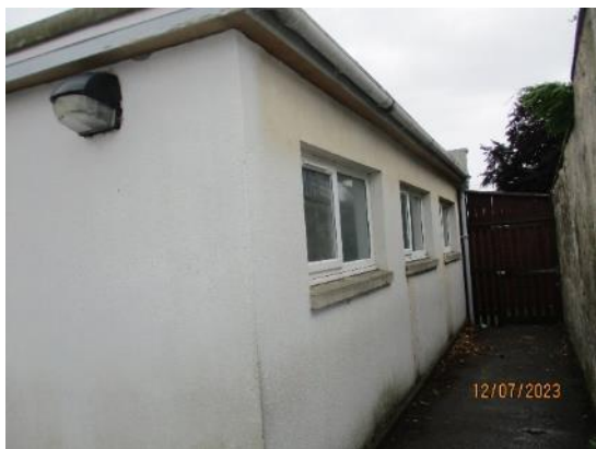
64. Masonry walls to school
