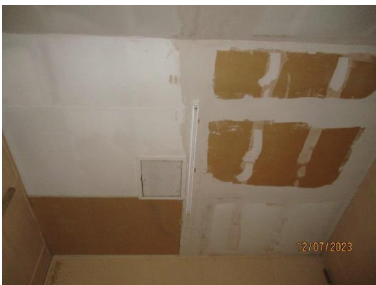
147. Fibreboard ceilings in the Hut
