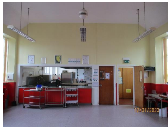
165. Lath & plaster in Dining Hall
