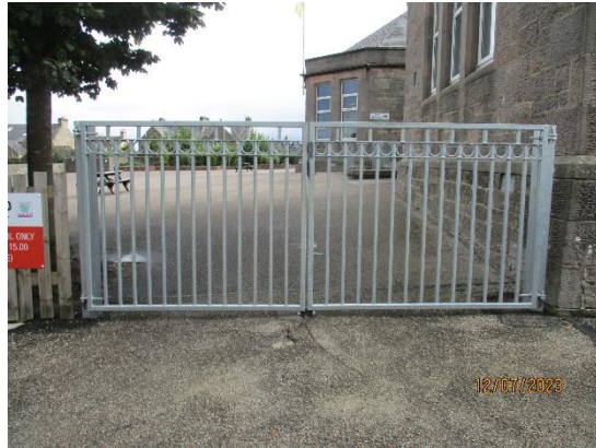
325. Galvanised bar vehicle gate
