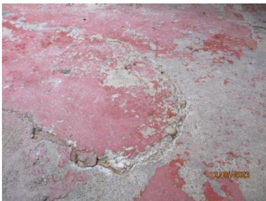
130. Boiler Room painted concrete floor
