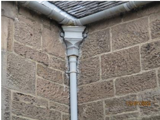
45. Cast iron hopper heads and downpipes
