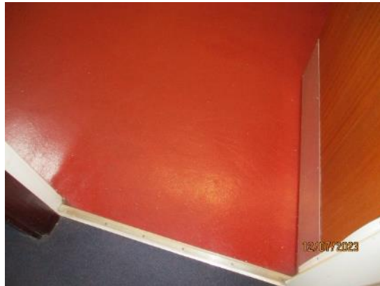
129. Painted concrete floors in the school
