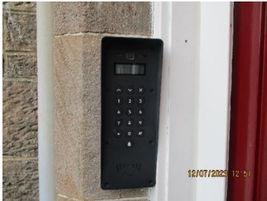
290. Paxton main entrance security door user video/audio unit.
