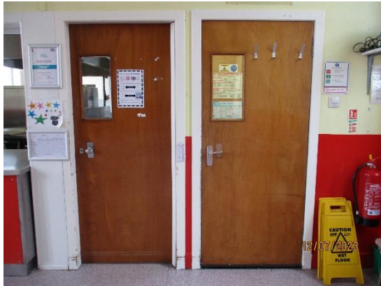
184. Timber hollow core doors in the Dining Hall
