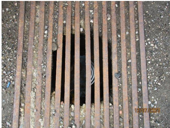
344. Metal can lid, blocking car park gully
