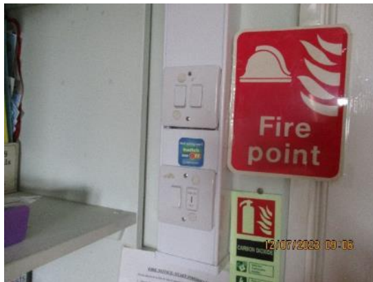
266. Light switches typical.
