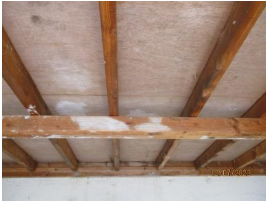
7. Timber rafters to External Stores
