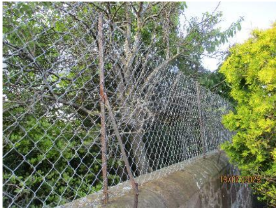
321. Chain link above walls (south)
