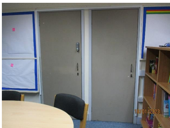
143. Timber hollow core cupboard doors
