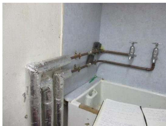
212. Pipework – hot and cold new. Main school 1/39
