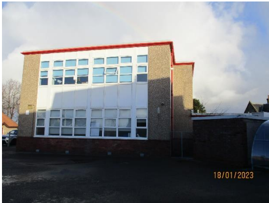
39. Concrete framed masonry walls
