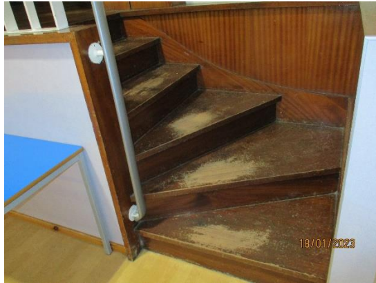
105. Timber stairs (Stage)
