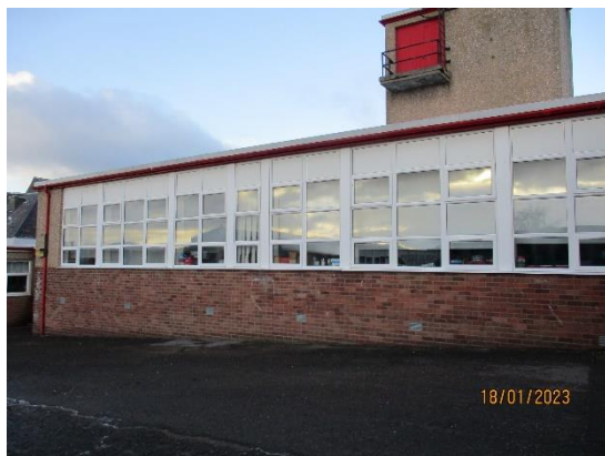
65. UPVC windows to school building
