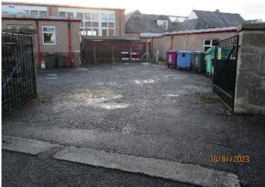
291. Rear tarmacadam car park
