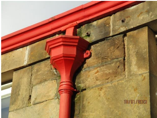
33. Cast iron hopper heads and downpipes
