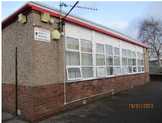
37. Brickwork external walls
