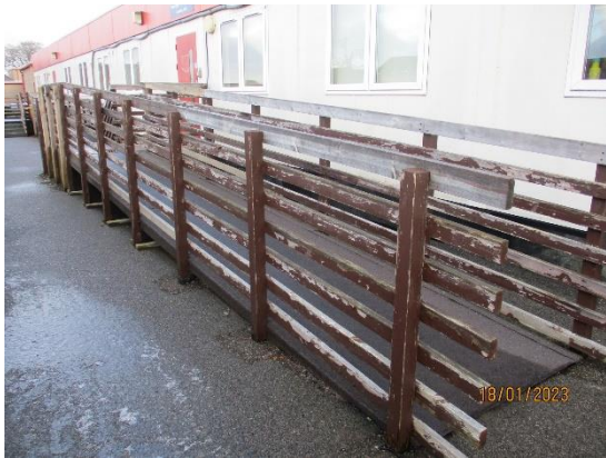
78. Timber guardrails and fencing
