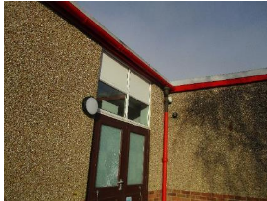
264. External lighting main school
