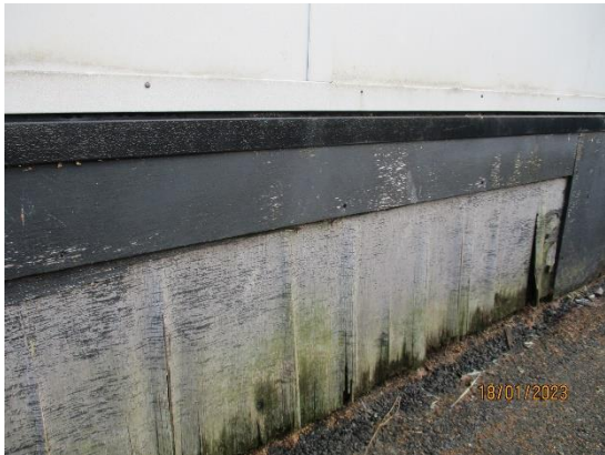
45. Plywood screening below ASN building
