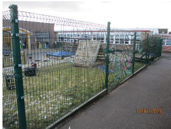
298. Security mesh fencing
