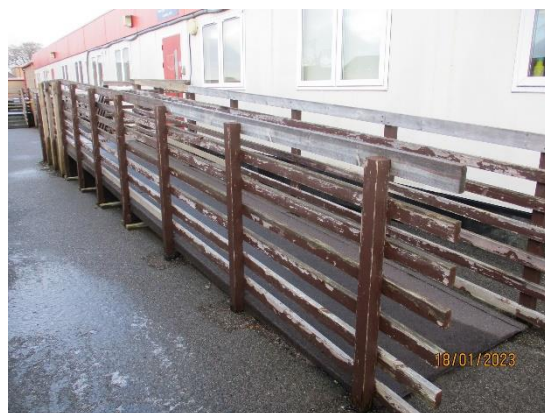
88. Timber guard rail
