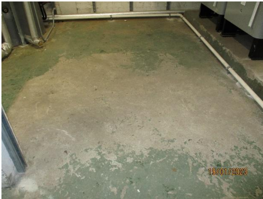
100. Painted concrete floors
