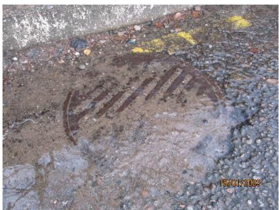
314. Blocked drainage
