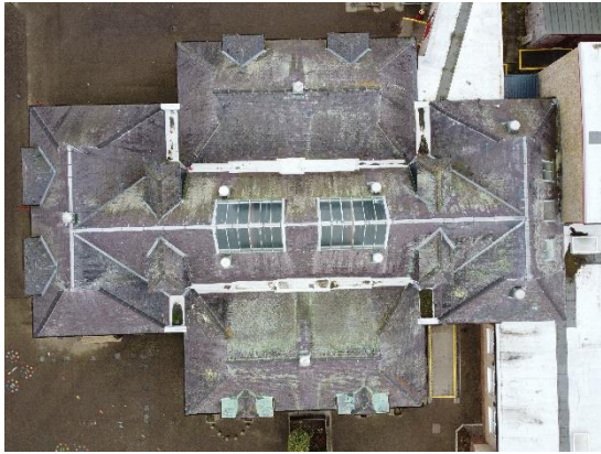
7. Natural slate to old building
