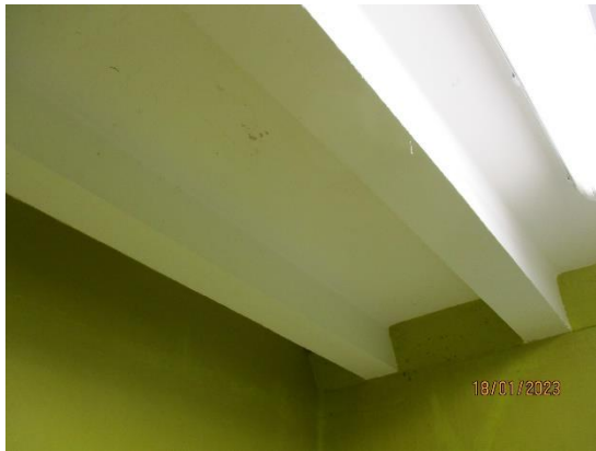
90. Concrete beam floors
