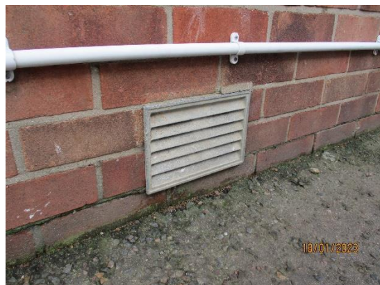
42. Ventilation below timber floors
