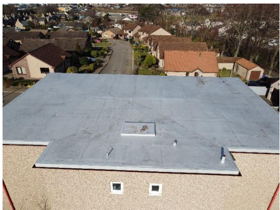
12. SPM to two storey building
