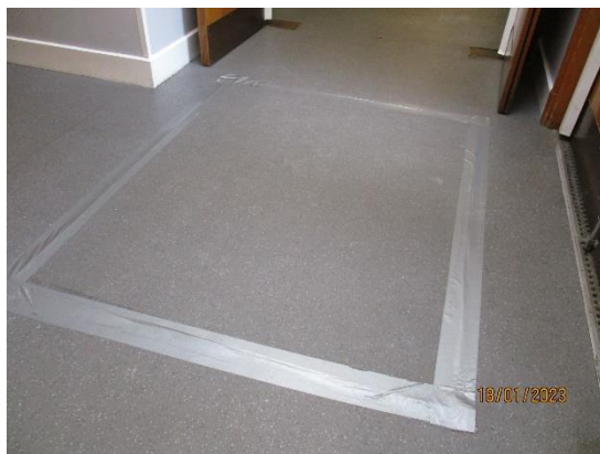
85. Tape repairs to vinyl
