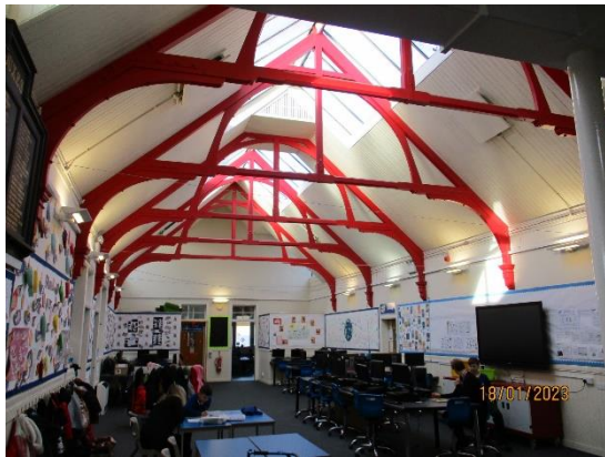
1. Old school central timber trusses
