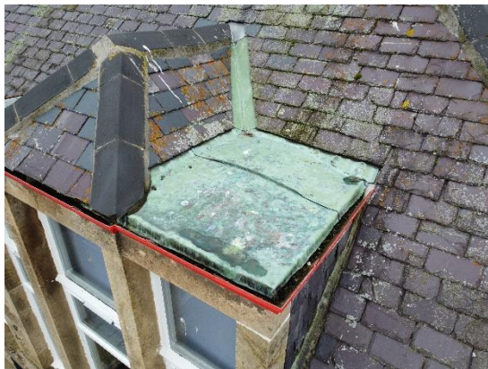
15. Copper to dormer roofs
