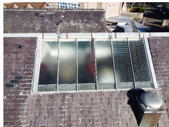
18. Skylights to old hall
