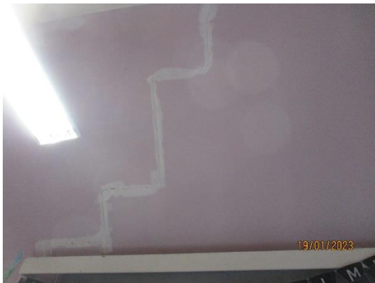
117. Previous repairs to cracks
