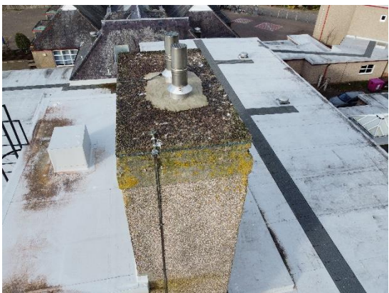
36. Water tank tower and boiler chimney
