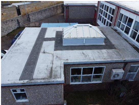
25. PVC cupola above Kitchen
