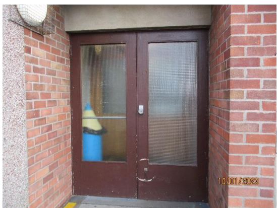
54. Timber glazed fire exits
