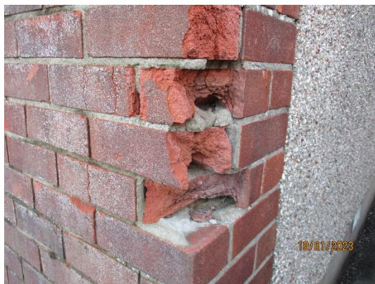
48. Damaged brickwork
