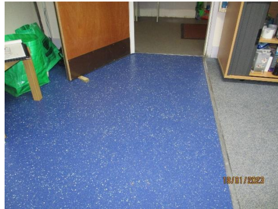
83. Sheet vinyl flooring to classrooms
