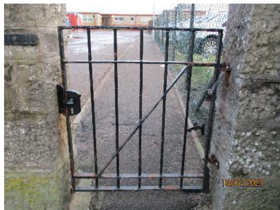
308. Metal bar gates
