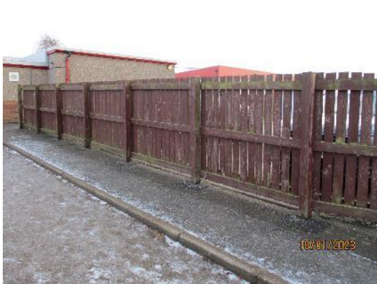
305. Timber boarded fencing
