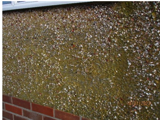
50. Spalling roughcast
