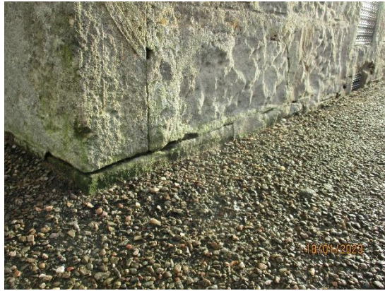
44. Ground level close to DPC
