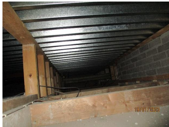
4. Decking below concrete slab roofs
