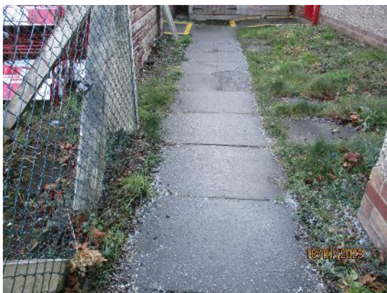
295. Paving slab footpaths
