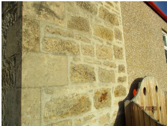
49. Stone walls to old building
