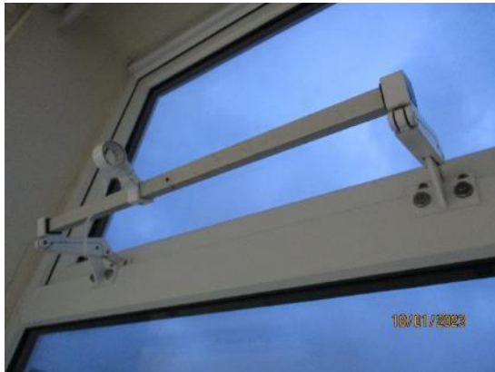
74. Cantilever top hung window ironmongery
