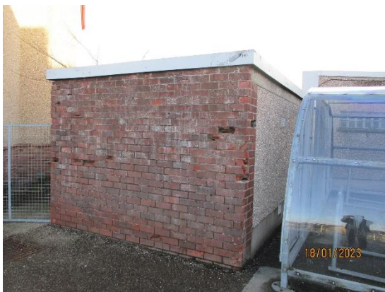
47. Brickwork to external store
