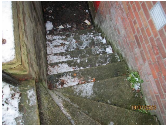
85. Concrete steps to Boiler House
