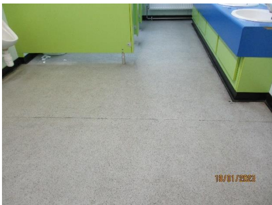
84. Sheet vinyl flooring to toilets
