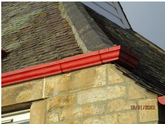
27. Cast iron ogee gutters
