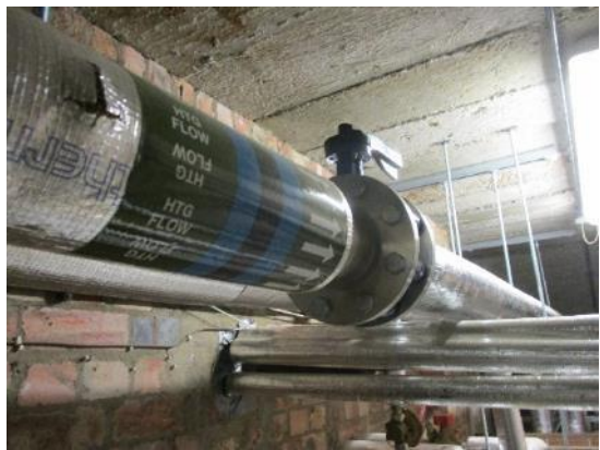
290. New heating pipework under school floor.
