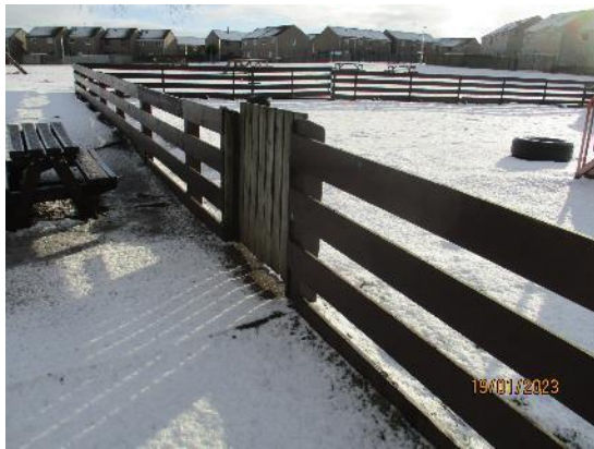
297. Timber post and rail fencing
