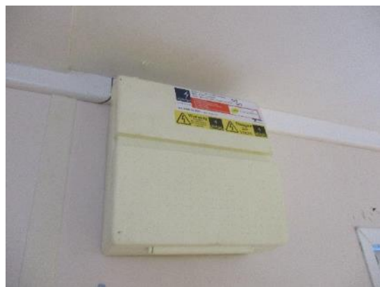
236. Consumer unit / RCD protection ASN building typical.
