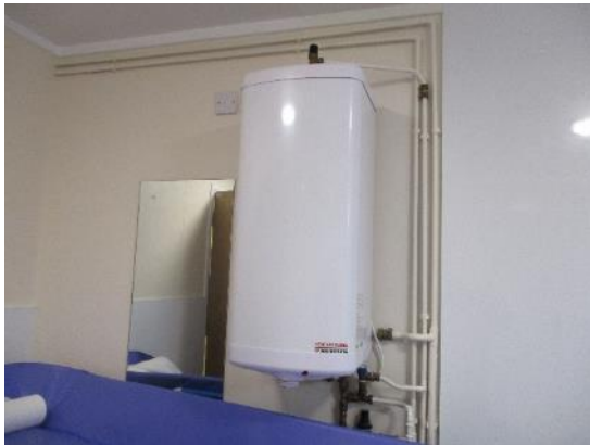
215. Point of use hot water storage unit. ASN building
