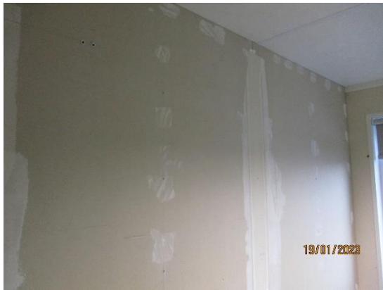
133. Plasterboard walls with no decoration
