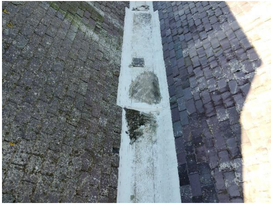
31. SPM valley gutters
