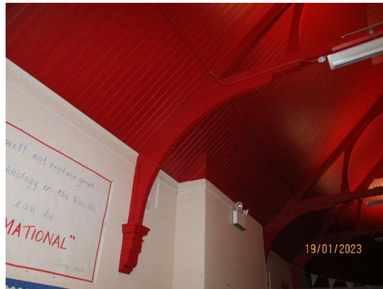
2. Trusses resting on stools
