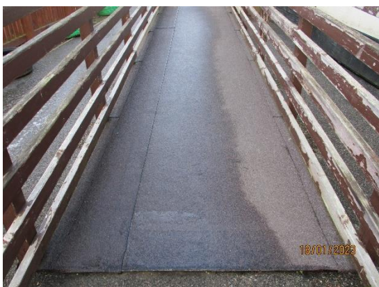
82. Timber ramps (ASN building)
