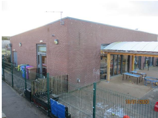
46. Brick walls to New Nursery
