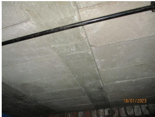
91. Beam & block floors
