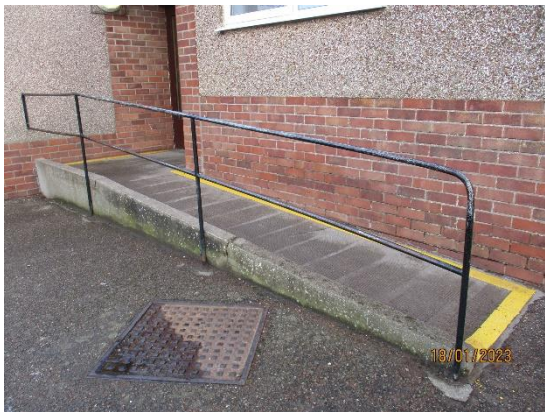
86. Metal tubular guard rail
