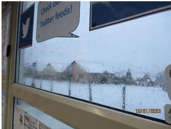
72. Blown double glazing units
