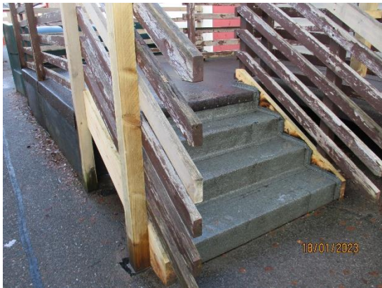
84. Timber steps (ASN building)
