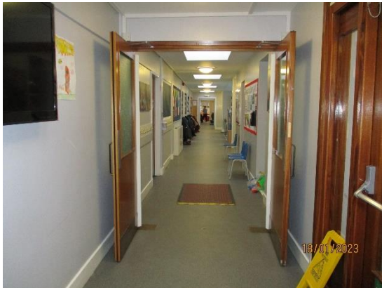
82. Sheet vinyl flooring to corridors
