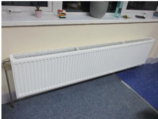
207. Radiator – main school 1/6 upgraded.
