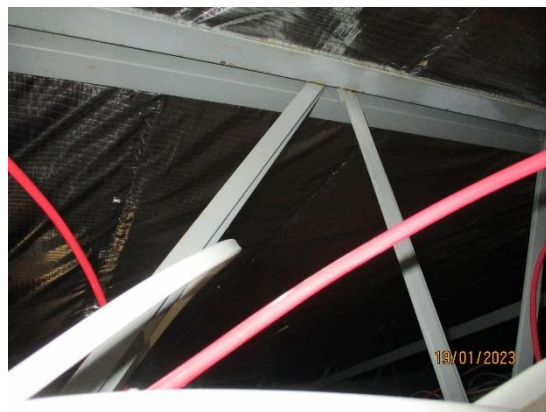
6. Steel roof joists to ASN building
