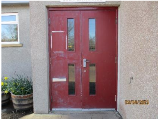
36. Timber front entrance doors
