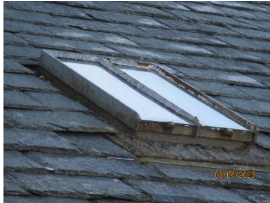
14. Metal skylights to external store
