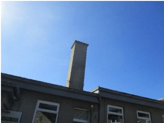
156. Boiler chimney – side view.
