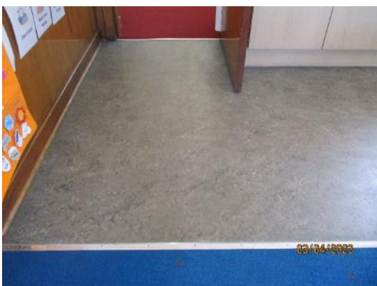
51. Sheet vinyl to sink areas
