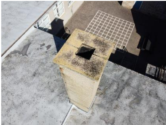
27. Concrete coping to boiler flue
