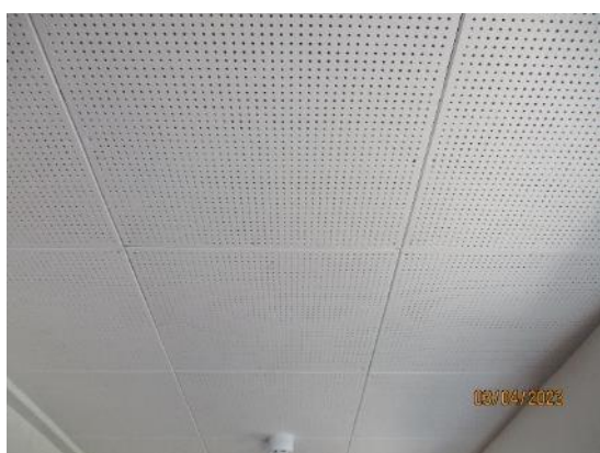
63. Fixed fibre tiles to most areas
