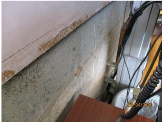
71. Blockwork internal walls
