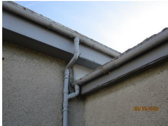
22. Cast iron downpipes
