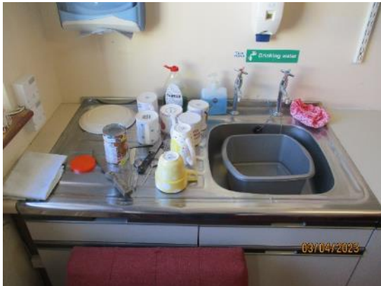
103. Stainless steel sink in Staff Room
