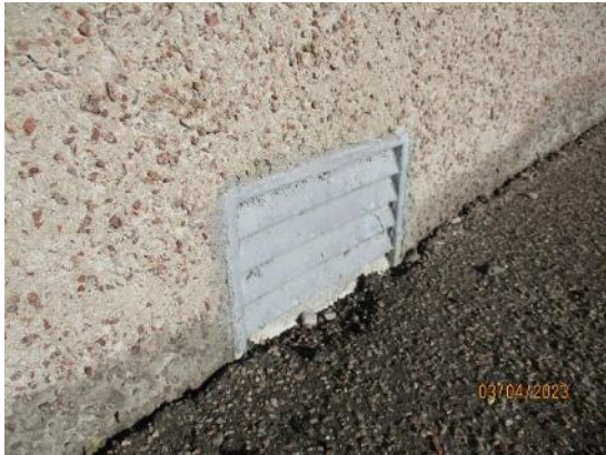
30. Under floor vents
