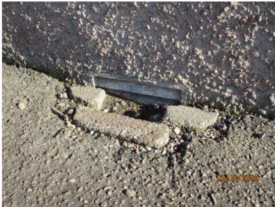
32. Ground level above vents
