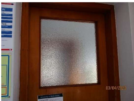
87. Glazing to classroom doors
