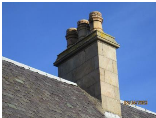
24. Stone chimneys with multiple clay pots
