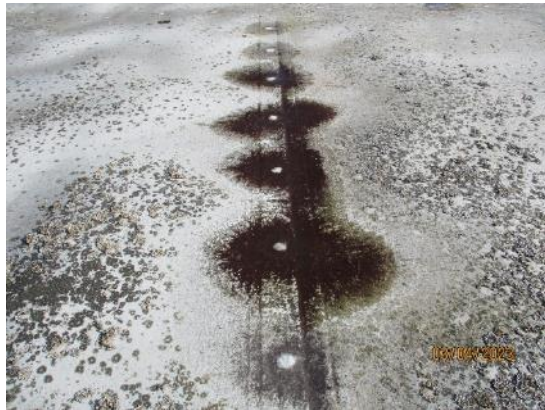
9. Fixings are raised and pronounced
