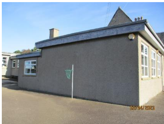
34. Roughcast walls to extension
