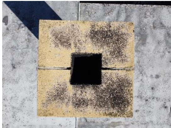
157. Boiler chimney termination. Aerial view from drone
