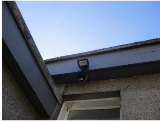
143. External lighting Kitchen entrance.
