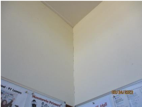
73. Lath and plaster walls
