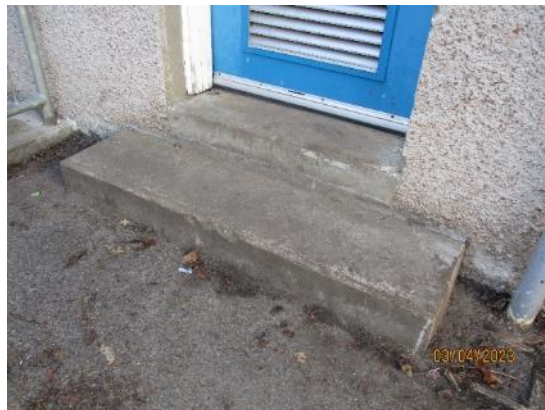
50. Concrete steps to boiler house
