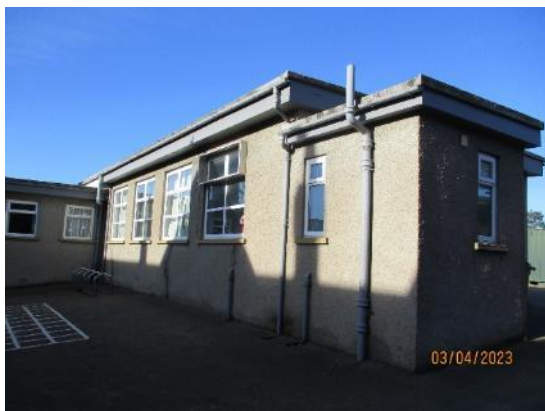
23. Cast iron soil vent pipes
