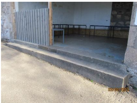
170. Concrete steps to external shelter
