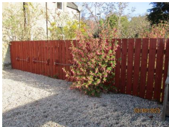
177. Timber boarded fence
