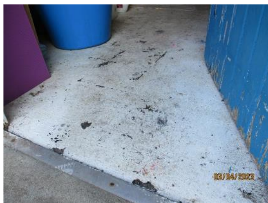
58. Concrete floor in external store
