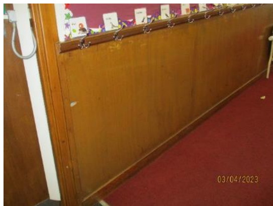
76. Timber panelling at low level
