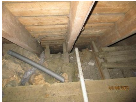
16. Partial insulation above ceilings
