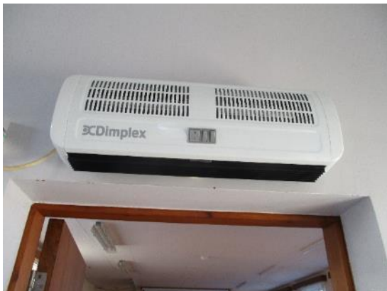
120. Electric Fan convector kitchen 1/11
