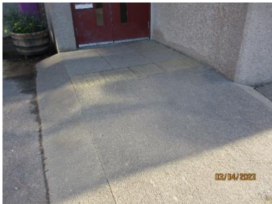
49. Concrete ramp to front entrance
