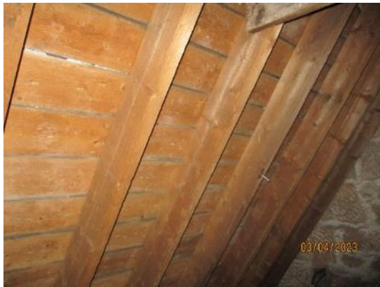
1. Timber rafters and sarking boards
