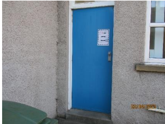
37. Timber fire escape doors
