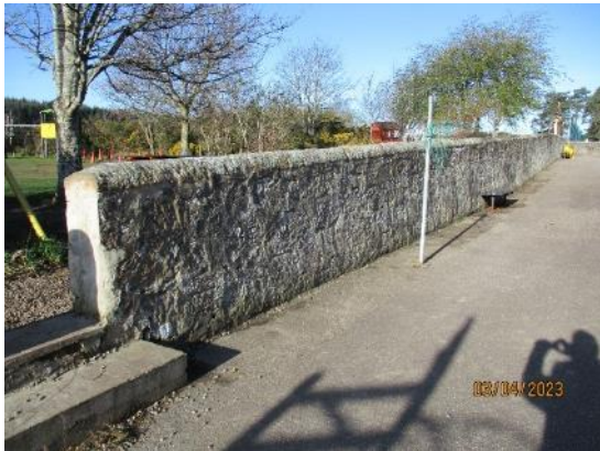
180. Natural stone playground perimeter wall
