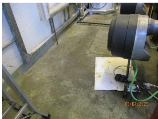
59. Concrete floor in Boiler Room
