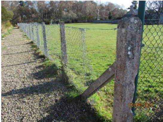
172. Concrete post and chain link fencing
