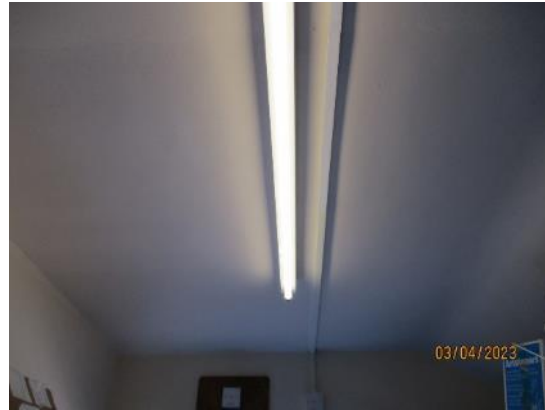
66. Lath and plaster ceiling in the external store
