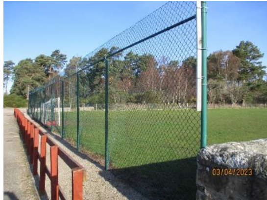
173. High chain link fencing
