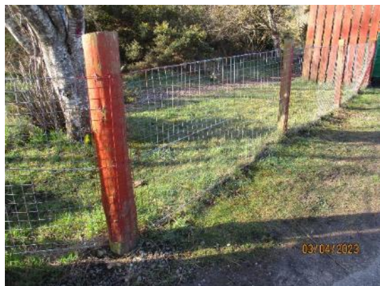
171. Timber post and wire mesh fencing
