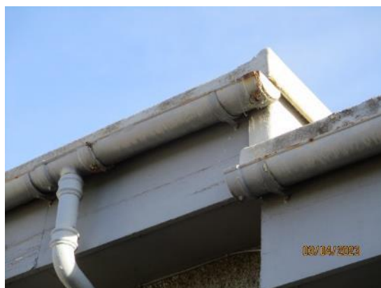
47. Cast iron rainwater goods
