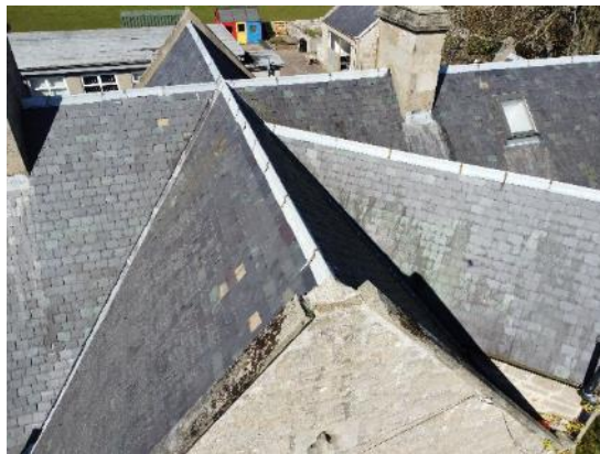
4. Slate roofs and zinc ridge
