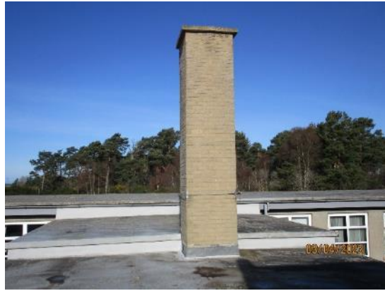
26. Brick boiler flue
