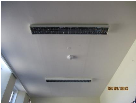
65. Lath and plaster ceilings in the old building
