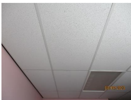
64. Suspended ceiling tiles to pupil toilets
