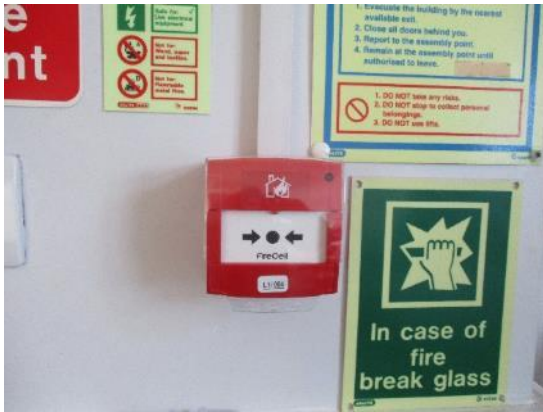
148. Fire alarm call point – wireless typical
