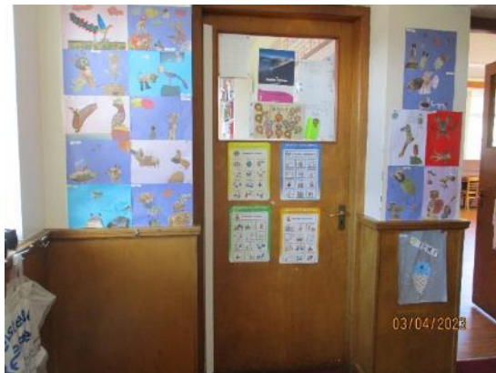
85. Timber hollow core classroom door
