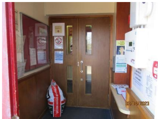
82. Timber double doors in corridor
