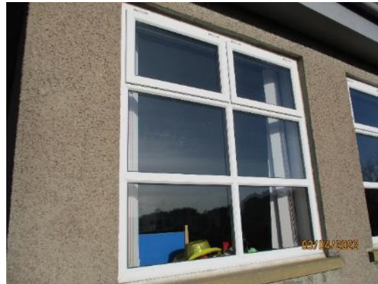
39. Large UPVC windows
