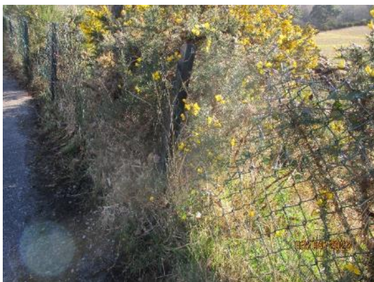
176. Galvanised post and chain link fence
