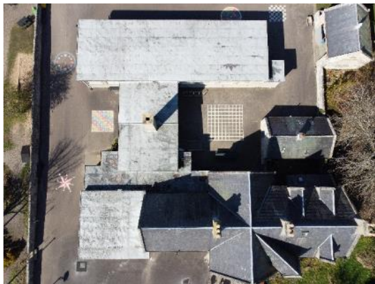
3. Overview of roofs
