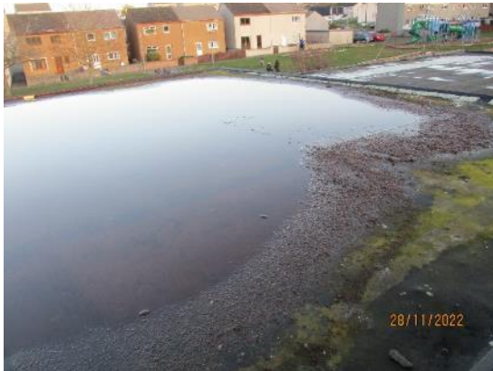
9. Significant ponding
