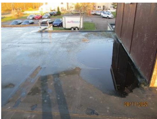
5. Inadequate falls
