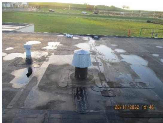
201. Roof extractor fans terminations typical
