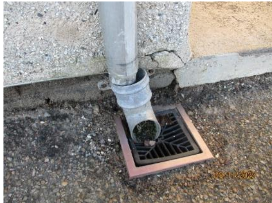
28. Displaced downpipe
