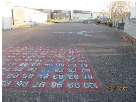
206. Rear tarmacadam playground
