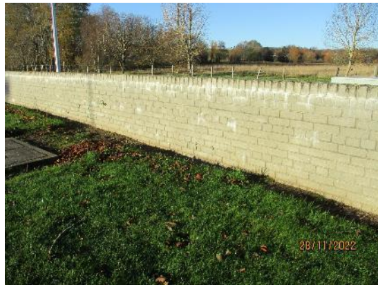
228. Brick wall to front
