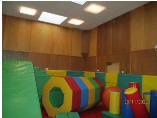
84. Timber lined walls (Soft Play)
