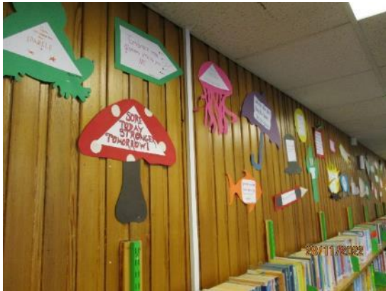
83. Timber linings (Library)
