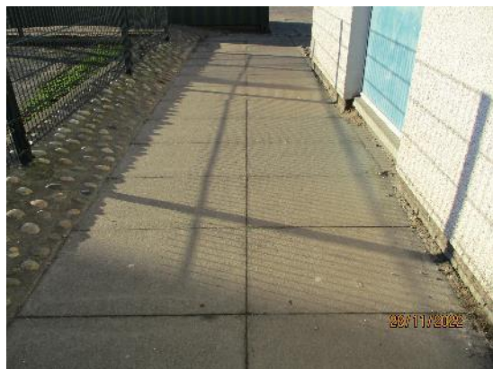
214. Paving slab footpaths
