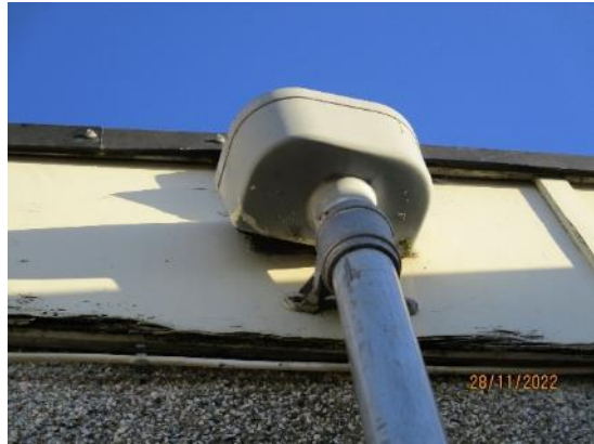
26. Insecure hopper heads
