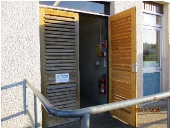
38. Timber louvre doors
