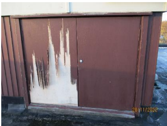
40. Timber tank house doors
