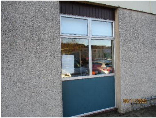
42. Typical aluminium window
