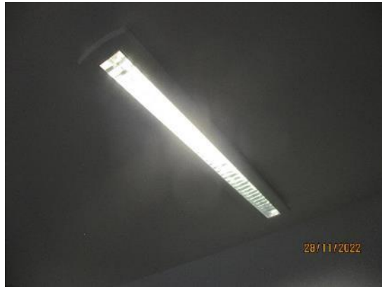
182. Emergency light – self contained variant.
