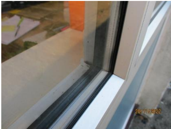
50. All windows are double glazed
