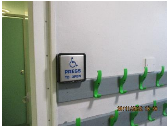
192. Automatic doors push pad operator 1/36a
