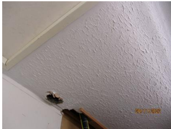
77. Textured finish to plasterboard ceilings
