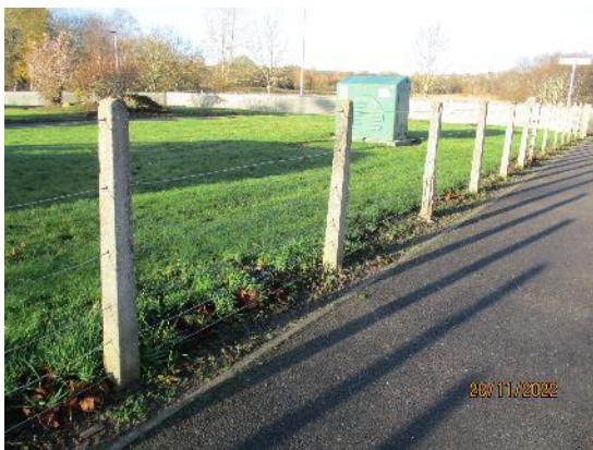
219. Concrete post and wire fence
