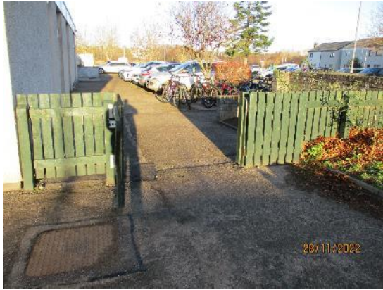
221. Timber boarded fence
