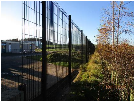
223. High metal security fencing
