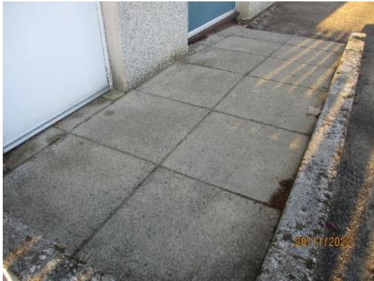
59. Paving slab ramps
