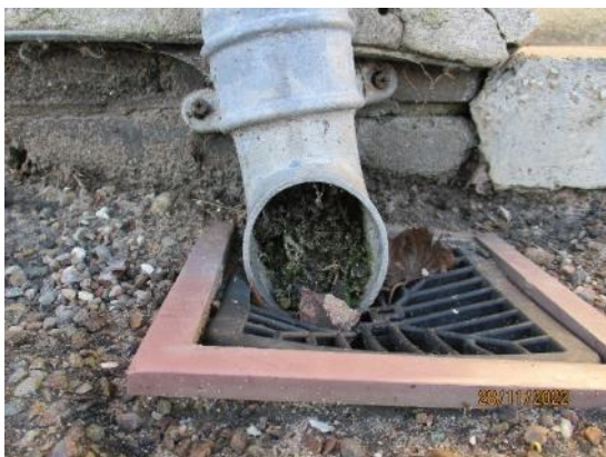
29. Blocked downpipe
