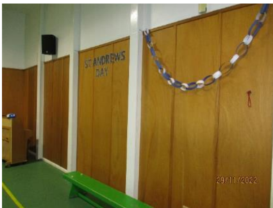
85. Timber lined walls (Games Hall)
