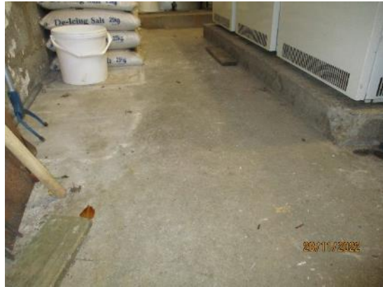
71. Concrete floor (Boiler Houses)
