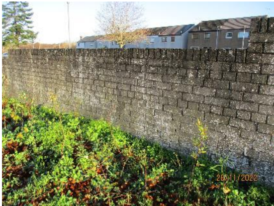
229. Brick wall to side
