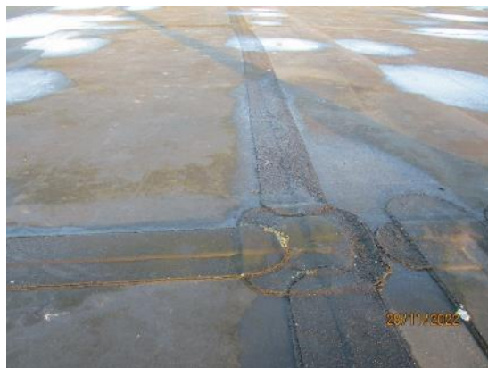
4. Previous patch repairs
