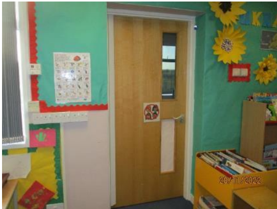
95. Veneered timber doors
