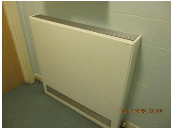
140. Radiator – LST type SEN zone typical.
