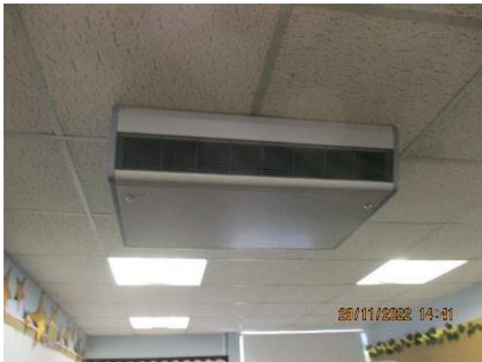
139. Fan convector heater SEN zone typical.
