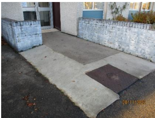
57. Concrete entrance ramp
