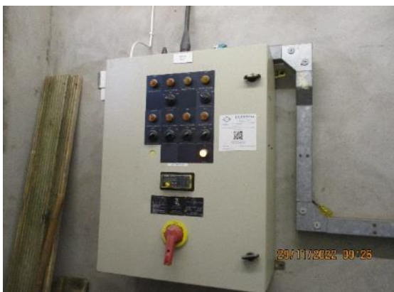
141. Heating control panel SEN zone 1/54
