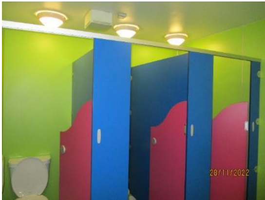
112. Composite cubicle partitions
