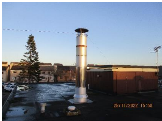
202. Roof – main school boiler flue system.
