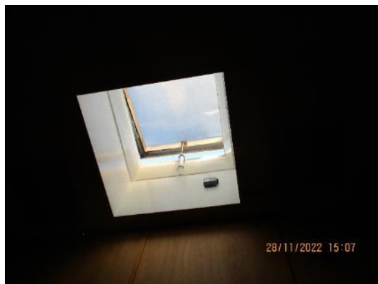
166. Electric motor operated roof lights. Typical.
