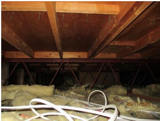
1. Steel lattice trusses and timber framed decking
