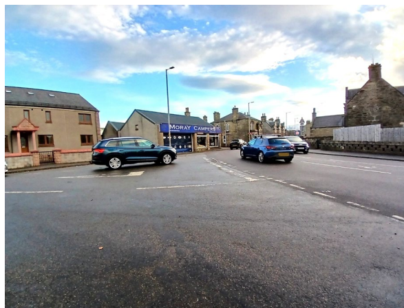
Large splay at junction with the width close to 30 meters, compared to 5.5 further into Drum Road.
