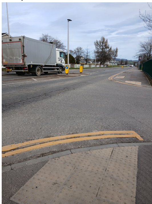
Entrance into Grammar School car park with wide corner radii and a lack of priority for pedestrians. The only crossing on this end of Banff Road is a pair of dropped kerbs with a central refuge just opposite the car park entrance.
