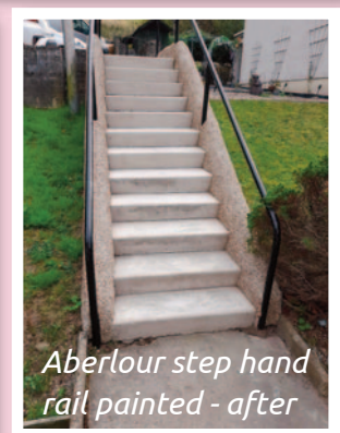
Aberlour step hand rail painted - before
