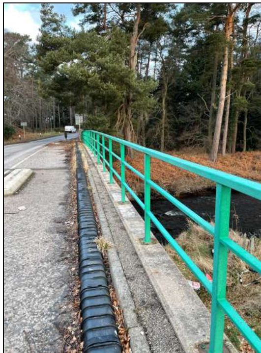
Fig 14. General view of north guardrail looking west
