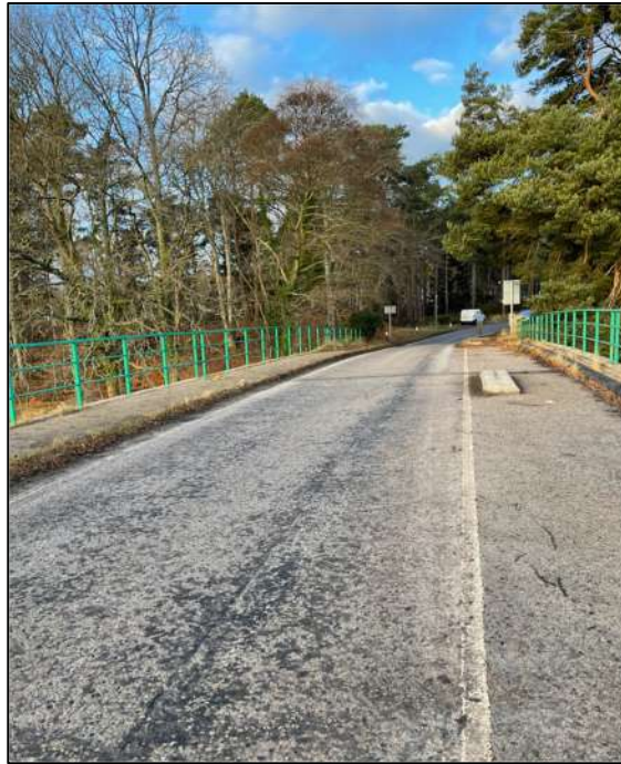
Fig 16. Road surface in good condition
