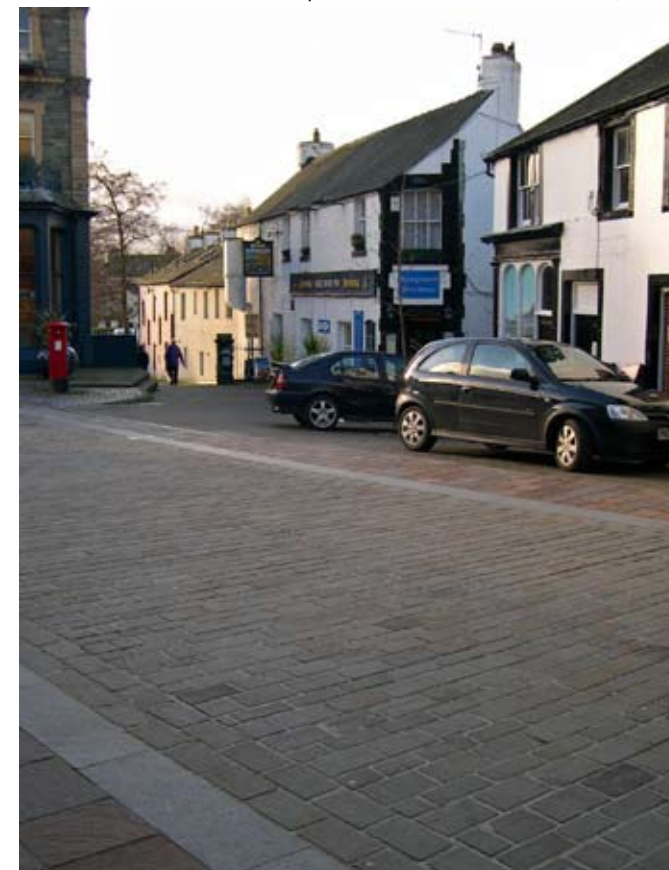
exemplar - shared surface in Keswick town centre, Cumbria
