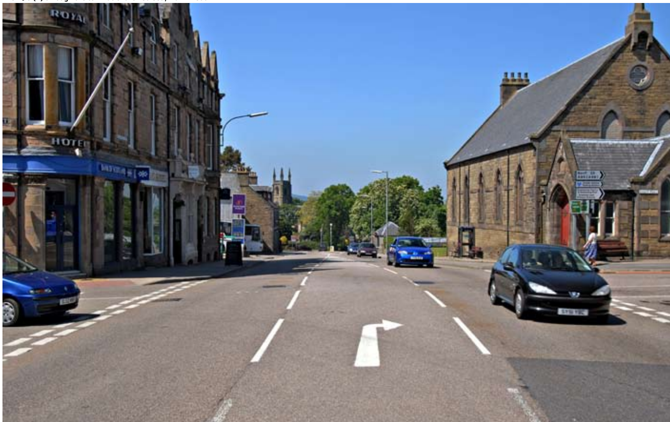
The A96 (T) through the town at Church Street / Banff Road
