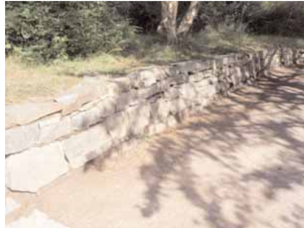
Stone boundary wall
