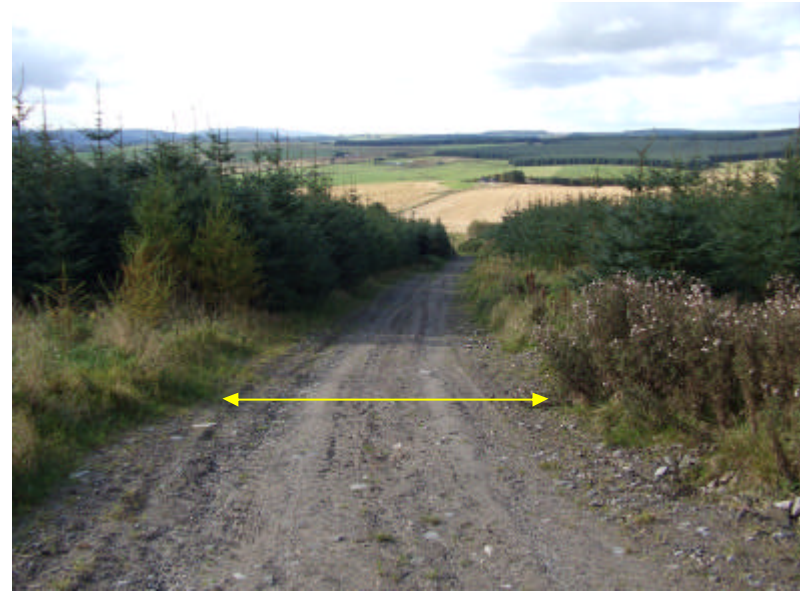
Photograph 10: Access track within the forest. The width of the lane at this section of the track is 3.6m as denoted by the yellow arrow. It will require widening of 20cm each side to bring it up to the access track specifications required by the turbine manufacturer, Enercon.
