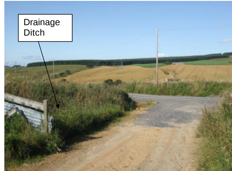
Photograph 4: Corner of track near Nethertown. This corner will be widened to 5.5m to allow the larger delivery lorries to pass. Following construction this will be returned to its current state by covering it with topsoil and seeding it appropriately. The existing drainage ditch will be re-routed to accommodate this corner infill.
