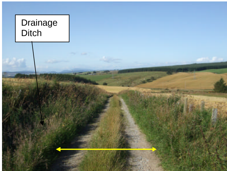
Photograph 5: Looking back down part of the access track already in place towards the B9018. Here the track is approximately 3.3m wide as denoted by the yellow arrow. It will require widening of 70cm to bring it up to the access track specifications required by the turbine manufacturer, Enercon. The drainage ditch on the left hand side of the photograph will remain unaffected.
