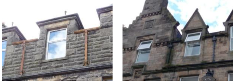
Damaged and poorly-maintained rainwater goods are common in the conservation area
