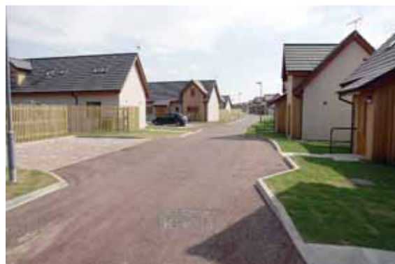
Canal Bank, Lossiemouth is a well designed Homezone, although the location and site conditions resulted in a cul de sac layout. Clear signage, a change in surface materials and segregated parking identify the area as a shared surface Homezone.
