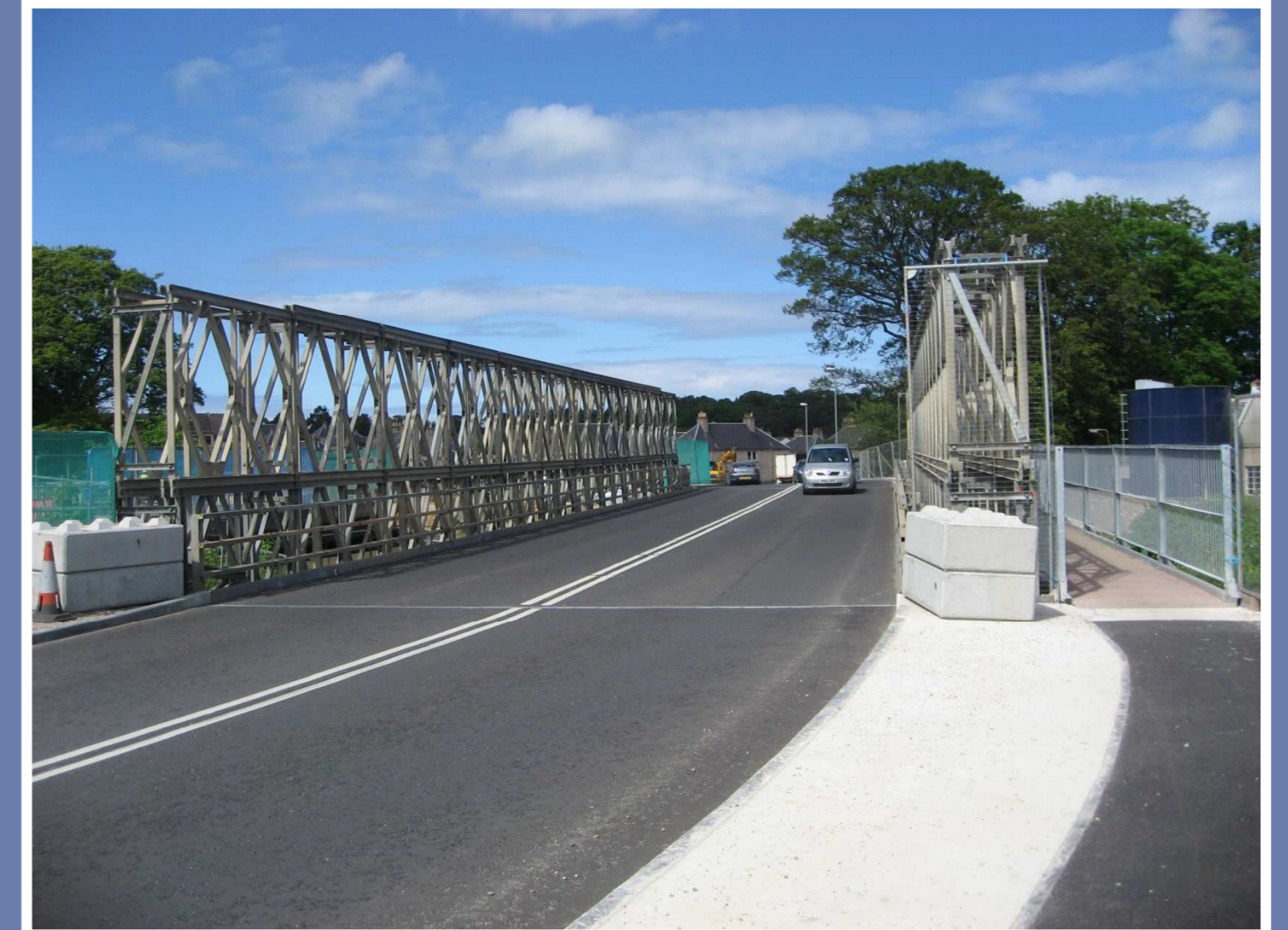
The temporary bridge
