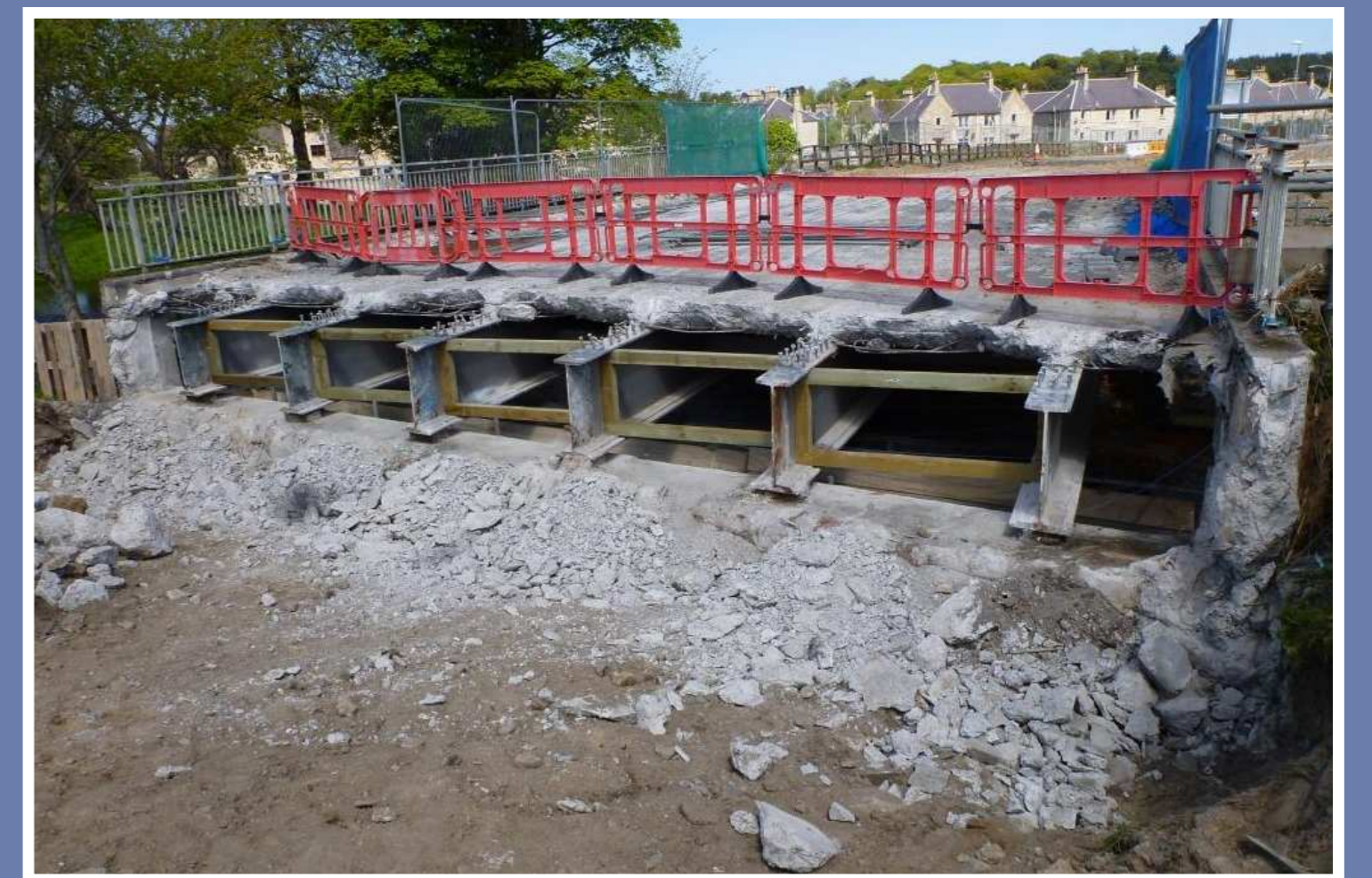
Demolition of the existing bridge
