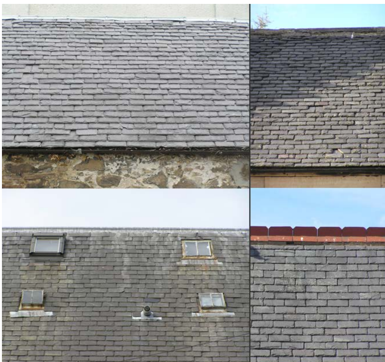
Blue slate roofs: the upper images show random face widths laid in diminishing courses; the lower images show regular machine dressed slates; ridges vary from lead, to stone and a decorative red clay ridge (bottom right)
