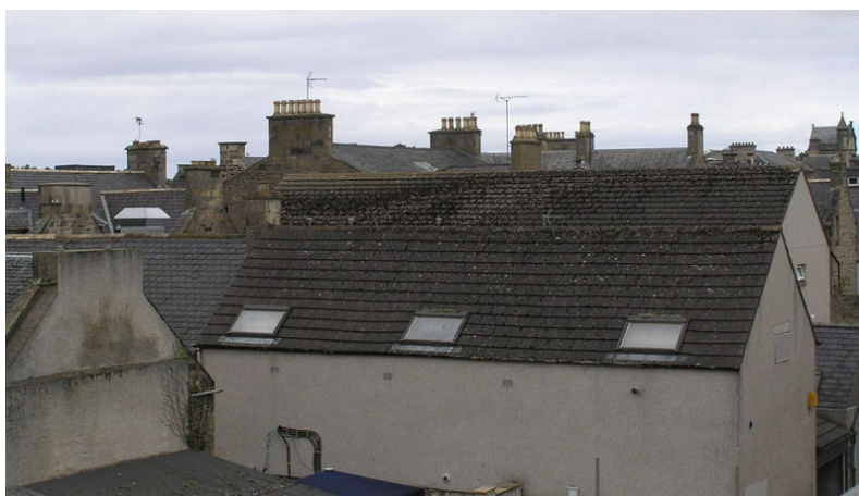
Concrete interlocking tile roofs appearing as alien finishes within a roofscape of predominantly blue slates
