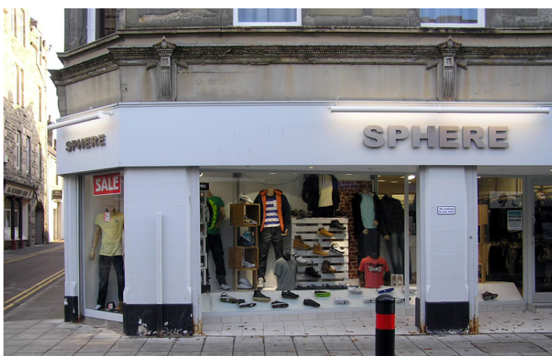
A shopfront marred only by the rusting guides for the security shutters and the modern shop fascia have been introduced below the original ornate one of timber, which is now at risk from not having been maintained
