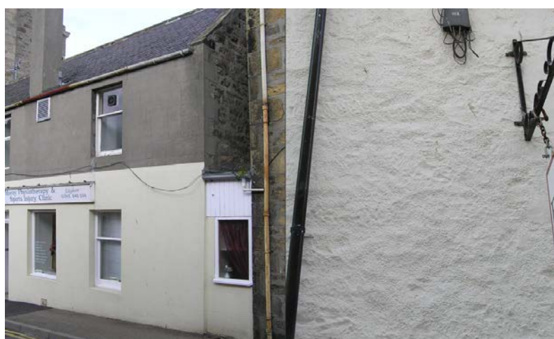
An early Portland cement smooth render, left, and possibly an early lime harl, right
