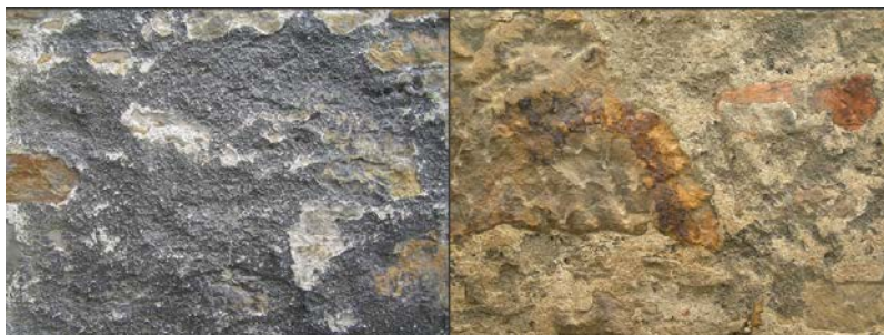
Rubble stonework with evidence of lime harling, or sneck harling
