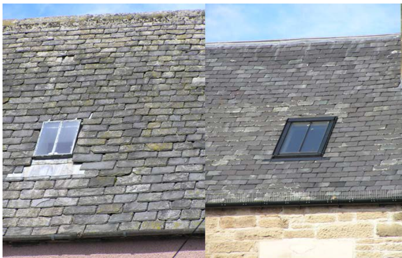
Traditional cast iron skylight (left) and modern conservation rooflight (right): although the top frame member is heavy the unit does not sit too high above the slates, and the middle astragal is slender, but there are less intrusive conservation rooflights than this on the market
