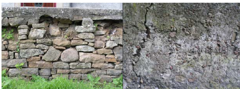
Unusual materials: boundary wall bonded with earth mortar and mass unreinforced concrete wall
