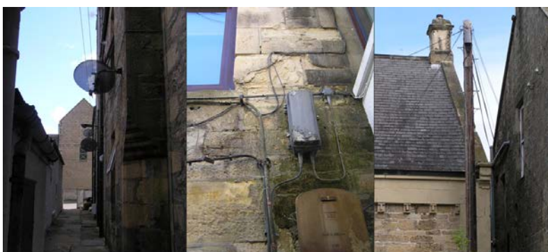
Satellite dishes, surface wiring and overhead lines
