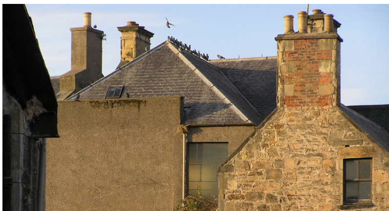
A hybrid brick and stone chimneyhead in which the soft stone has weathered worse than the brick – the stone chimneyhead in the background is in an advanced state of decay while the chimneyhead beside it has been taken down and rebuilt unattractively with a dense cement render finish
