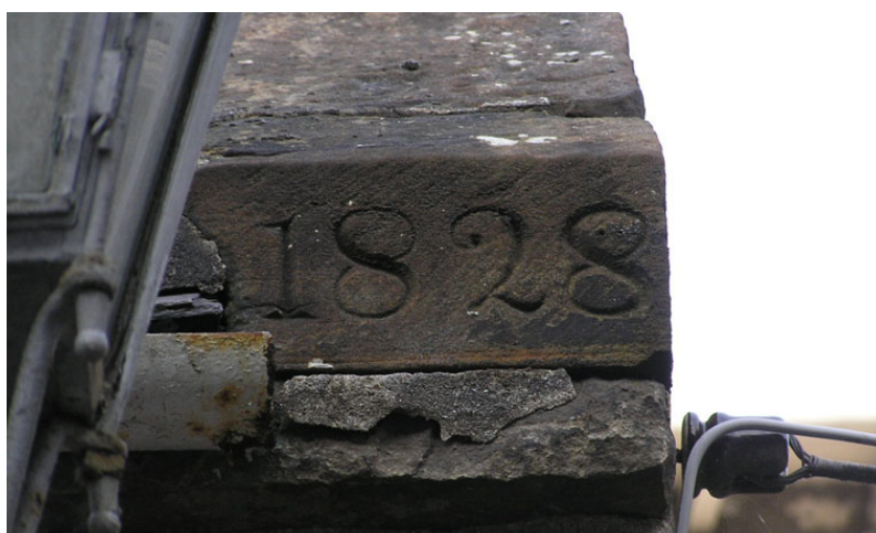
Gable with plain skews and a skewputt carrying the date 1828 (Braco's Close)
