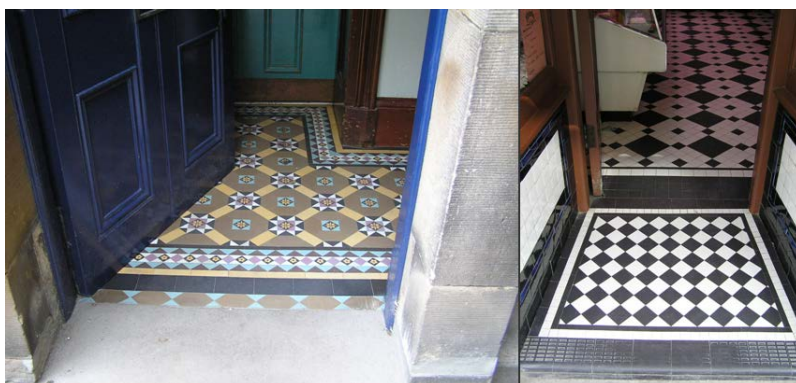
Encaustic tiled floors to door lobbies, late nineteenth century, left, and 1930s, right
