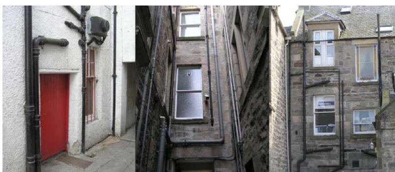
Unsightly soil and vent pipe systems to the rear of buildings on the forelands of the closes
