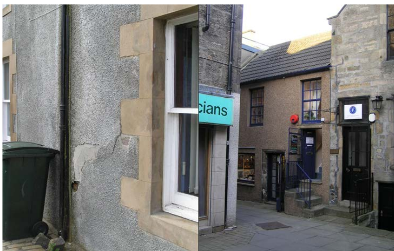
Wall finishes in the closes: an unattractive dense cement wet-dash harled finish with coloured cement quoins (which is failing) and a property rendered with a dry-dash finish and re-roofed with interlocking concrete roof tiles
